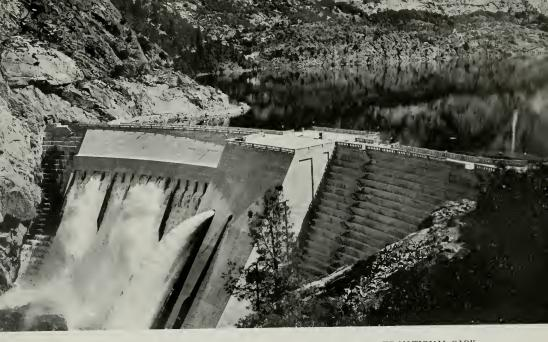
O'SHAUGHNESSY DAM ON TUOLUMNE RIVER IN YOSEMITE NATIONAL PARK The dam has a total height of 344 feet which will be increased to 430 feet at a cost of \$3,500,000. The present dam was completed in 1923 at a cost of \$7,000,000.
