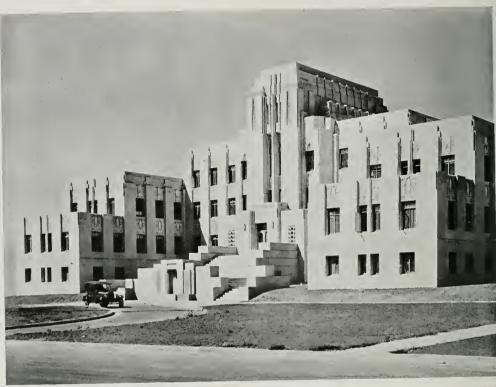
of the new solid section type—not cellular. It is attached by ties to vertical galvanized pencil rods which are anchored to the concrete and the intermediate space between tile and wall is slushed solid with mortar.
