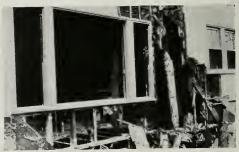
Fig. 4—The collapse of the wall and entrance of this home showed it to have been gutted by termites
