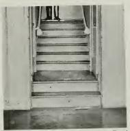
Fig. 2—The floor and stairs shown in Fig. 1 were found to have been gutted by these pests
