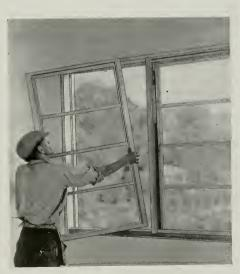
Carpenter attaches metal frame to simple wood sub-frame using ordinary wood-screws. Removable strip makes weights easily accessible.
