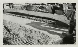
CLOSE-UP, SHOWING VIBRATING SCREEN IN OPERATION AND STEEL REINFORCEMENT
