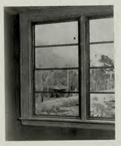
Installation completed and trim applied. Note narrow mullion and unobstrusive hardware. Sash may be raised or lowered with little finger.
