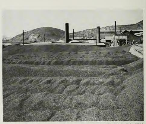
STOCK PILE OF GRAVELITE AT PLANT, POINT RICHMOND, CALIFORNIA This material mixed with cement makes a light weight concrete that is destined to revolutionize the present method of making structural concrete. Engineers say its use on the upper deck of the Bay Bridge will mean a saving of 20,000 tons in dead weight
