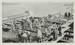
PLACING GRAVELITE CONCRETE IN UPPER DECK OF BRIDGE
