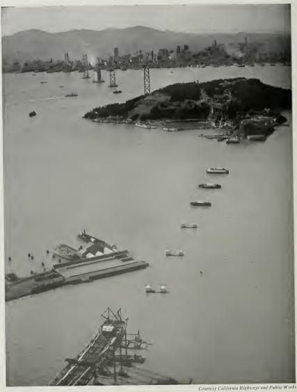
"STEPPING STONES" for the World's greatest bridge. In the foreground are seen the pier foundations for the East Bay crossing extending to Yerba Buena Island with a view of a traveling derrick erecting the last of the 288 foot spans of the Oakland shore superstructure. Beyond the island is seen the entire West Bay Crossing, with Tower W-5 under construction and the city of San Francisco in the background.
