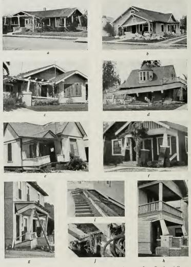
Fig. 1—(a-h) Typical examples of serious damage to frame houses at Long Beach and Compton. California, in the earthquake of March 10, 1933. Many of these failures were, in part, due to termite damage to under-pinning, as shown in details, i-j. The use of proper construction and wood, not attacked by termites, and fungi, would have prevented all but minor damage.
