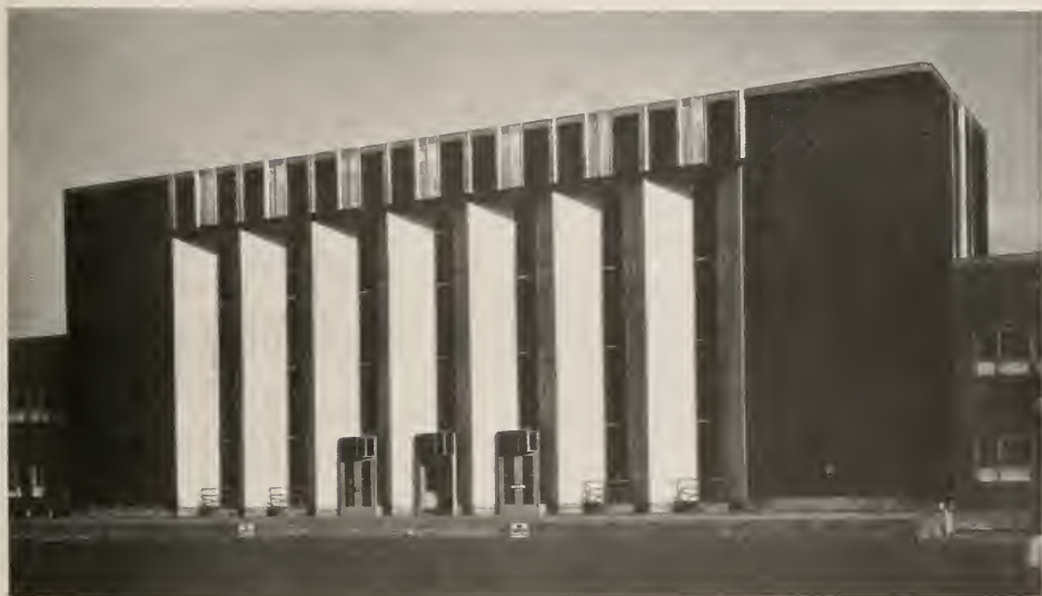
NIGHT ILLUMINATION OF MAIN FACADE, ADMINISTRATION BUILDING Edward H. Bennett, Hubert Burnham and John A. Holabird, Architects
