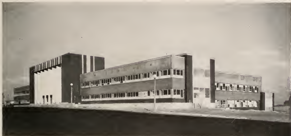
ADMINISTRATION BUILDING Edward H. Bennett, Hubert Burnham and John A. Holabird, Architects
