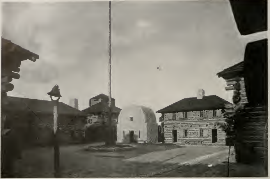
REPLICA OF FORT DEARBORN, CENTURY OF PROGRESS EXPOSITION
