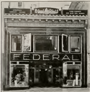
RECENT INSTALLATION OF DAY NITE SIGN Geary, near Mason Street, San Francisco
