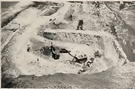
EXCAVATING FOR CABLE ANCHORAGE SAN FRANCISCO SIDE
