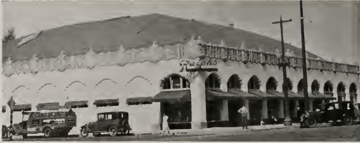
The ornamental concrete parapet shown in the above picture was cast in place in waste molds.
