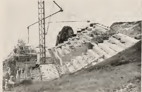
CABLE ANCHORAGE, MARIN SIDE, GOLDEN GATE BRIDGE
