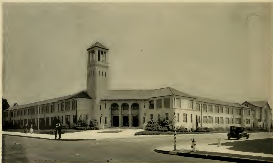
WOODROW WILSON HIGH SCHOOL, LONG BEACH, CALIFORNIA Reinforced concrete construction (except gymnasium which is not shown in the picture). Photograph taken after the earthquake of March 10th, 1933.
