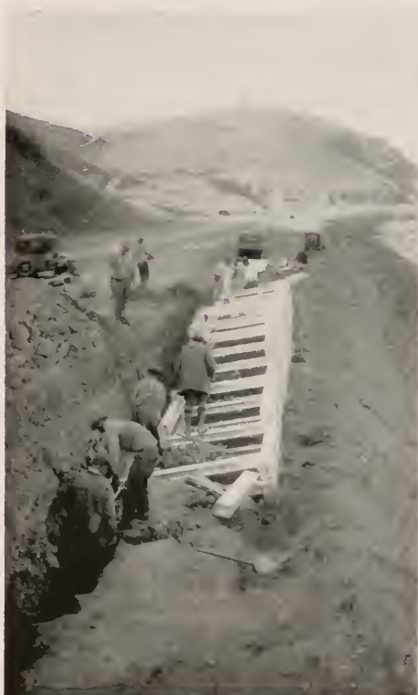
Metal crib wall, 114 feet long, installed by the California Division of Highways on Bayshore Highway, two miles south of the San Francisco-San Mateo County line.
