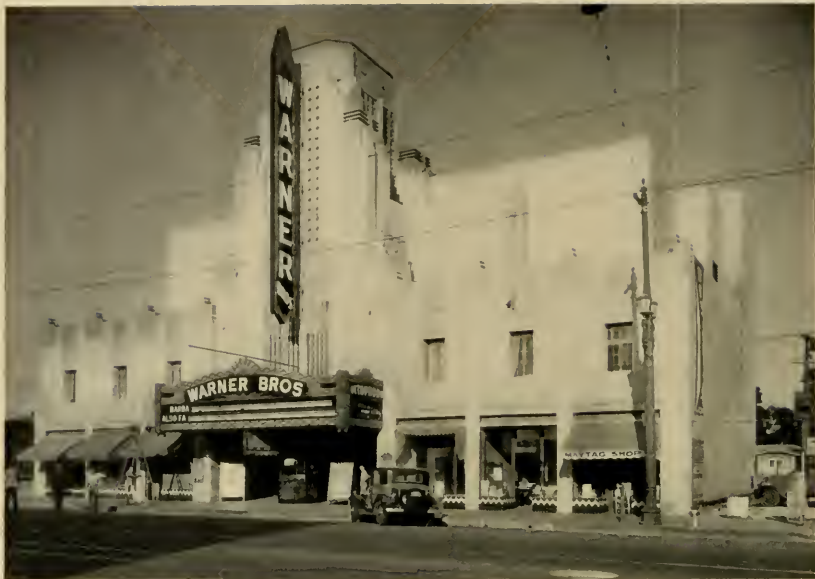
WARNER BROS. THEATER, HUNTINGTON PARK, CALIFORNIA Building is of reinforced concrete and was undamaged by the earthquake of March 10th, 1933. Signs in front announce auditorium safe for occupancy by order of Municipal Building Department. Photograph taken after the quake.
