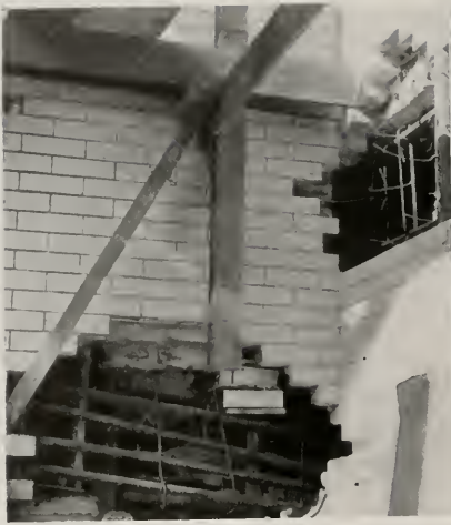
Above—View of preparation of walls and steel assembly at a wall corner.
