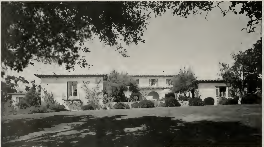
FRONT VIEW, HOUSE OF J. HENRY BEHRENS, SANTA BARBARA Reginald D. Johnson, Architect
