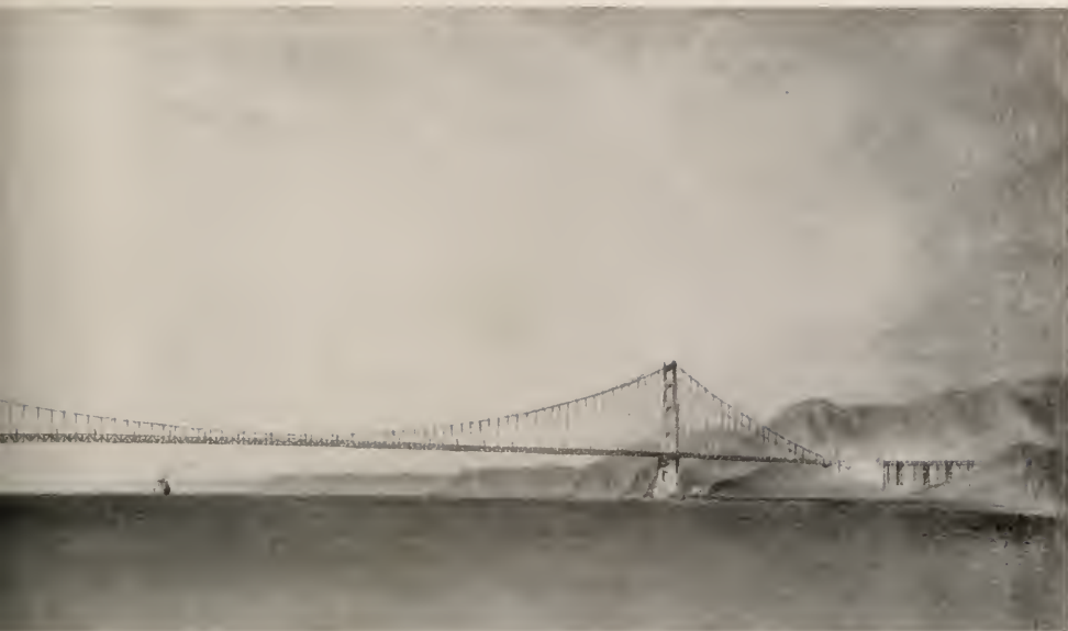
WITH A SINGLE CLEAR SPAN OF 4200 FEET, LONGEST SPAN IN THE WORLD
