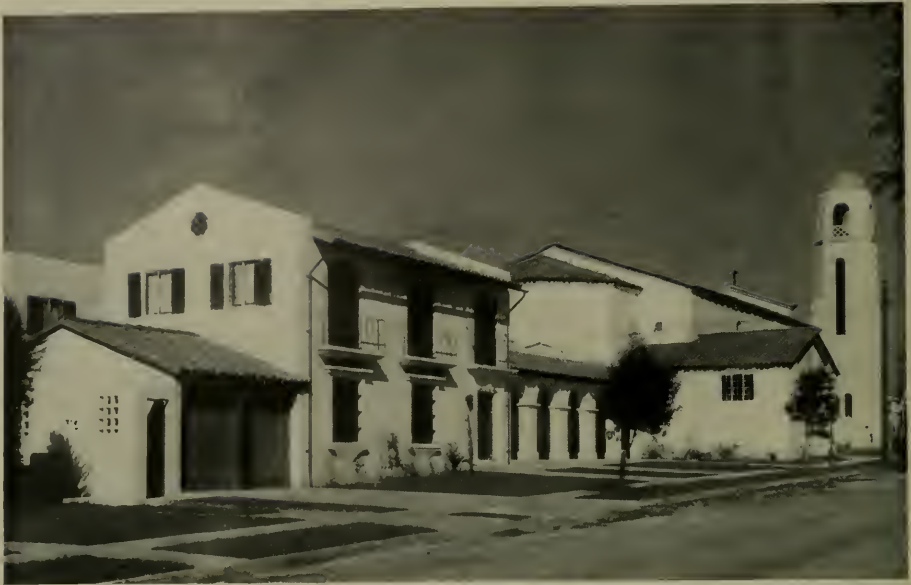
RECTORY AND CHURCH, HOLY SPIRIT PARISH, LOS ANGELES Newton and Murray, Architects
