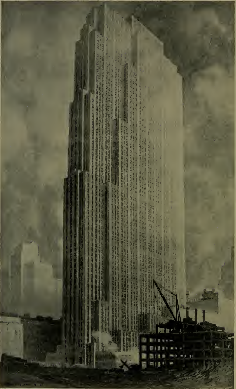
SEVENTY-STORY OFFICE BUILDING, ROCKEFELLER CENTER, NEW YORK CITY
