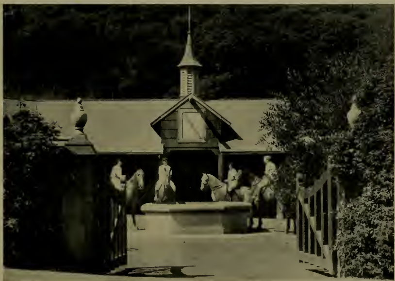
RIDING STABLE, MILLS COLLEGE W. H. Ratcliff, Jr., Architect
