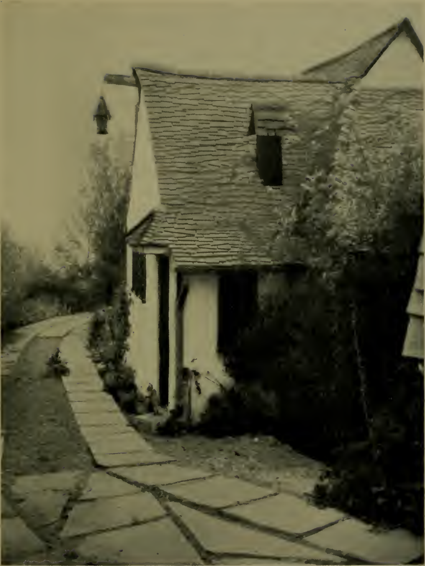
HOUSE FOR MR. AND MRS. CHARLES C. JOHNSON, BERKELEY, CALIFORNIA ARTHUR L. HERBERGER, ARCHITECT
