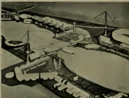
ARCHITECT'S DRAWING OF "THE SKY RIDE," CENTURY OF PROGRESS EXPOSITION, CHICAGO, ILL.
