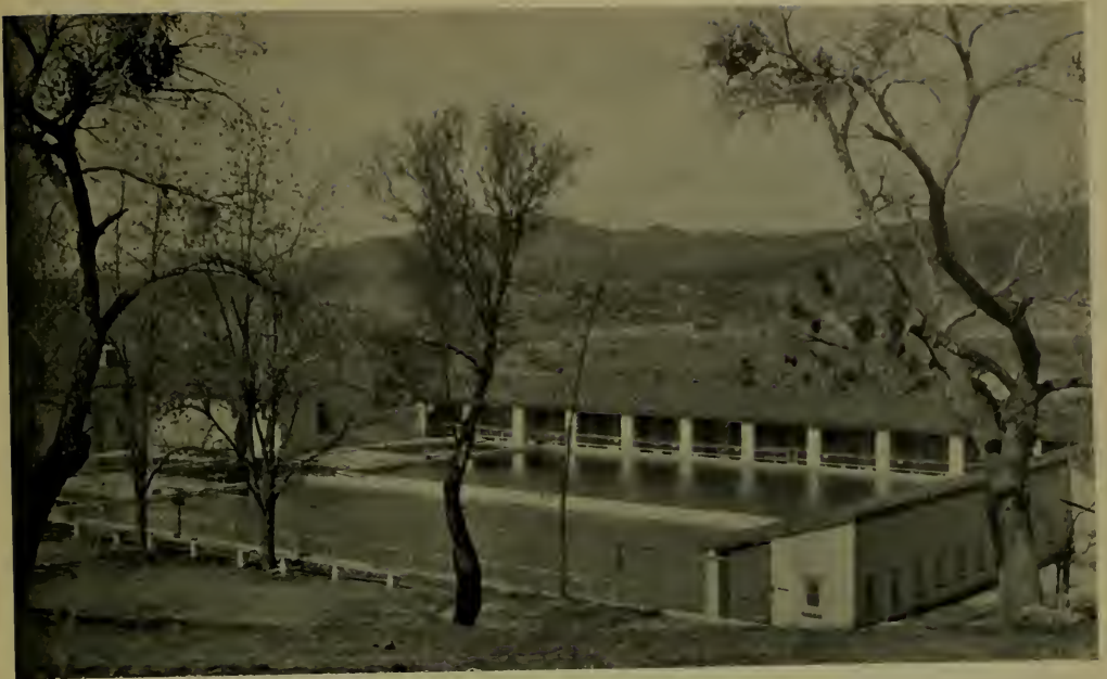
BUNGALOWS AND BATH HOUSE, WARNER HOT SPRINGS Gordon B. Kaufmann, Architect
