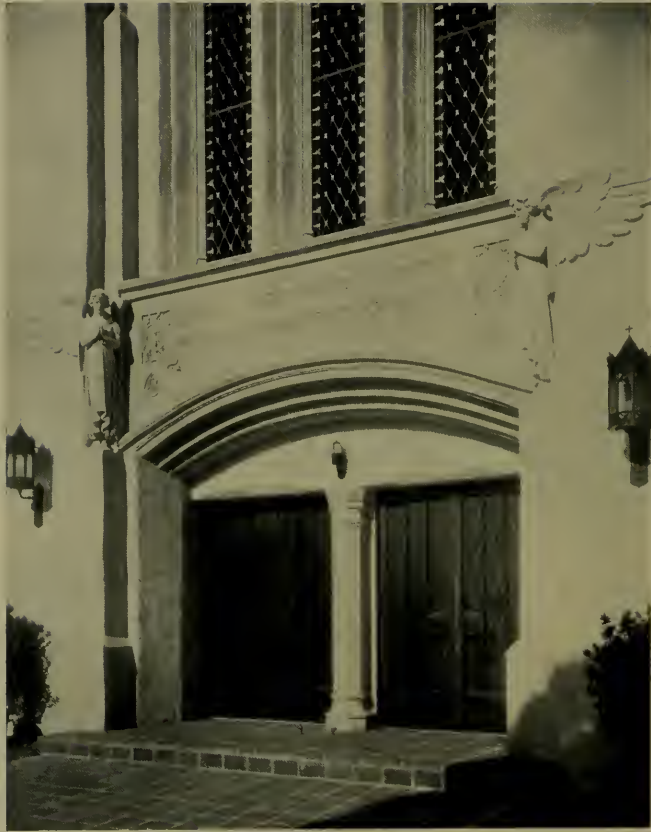
DETAIL OF ENTRANCE, GRACE LUTHERAN CHURCH, SAN DIEGO, CALIFORNIA
