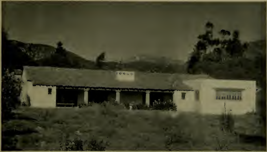
SOUTH ELEVATION, LA CANADA THURSDAY CLUB, LA CANADA, CALIFORNIA Newton and Murray, Architects
