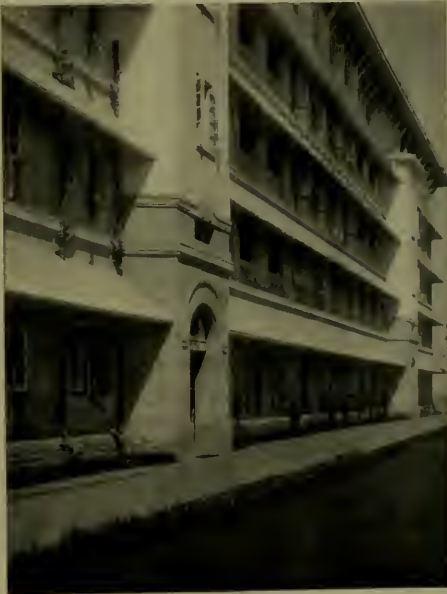
A CLOSE-UP OF THE "CHUIJAS", OR CORNICE, WHICH HELP TO MAKE LIFE MORE COMFORTABLE IN BOMBAY. THESE ARE CAST IN CONCRETE, WITH THE REST OF THE STRUCTURE
