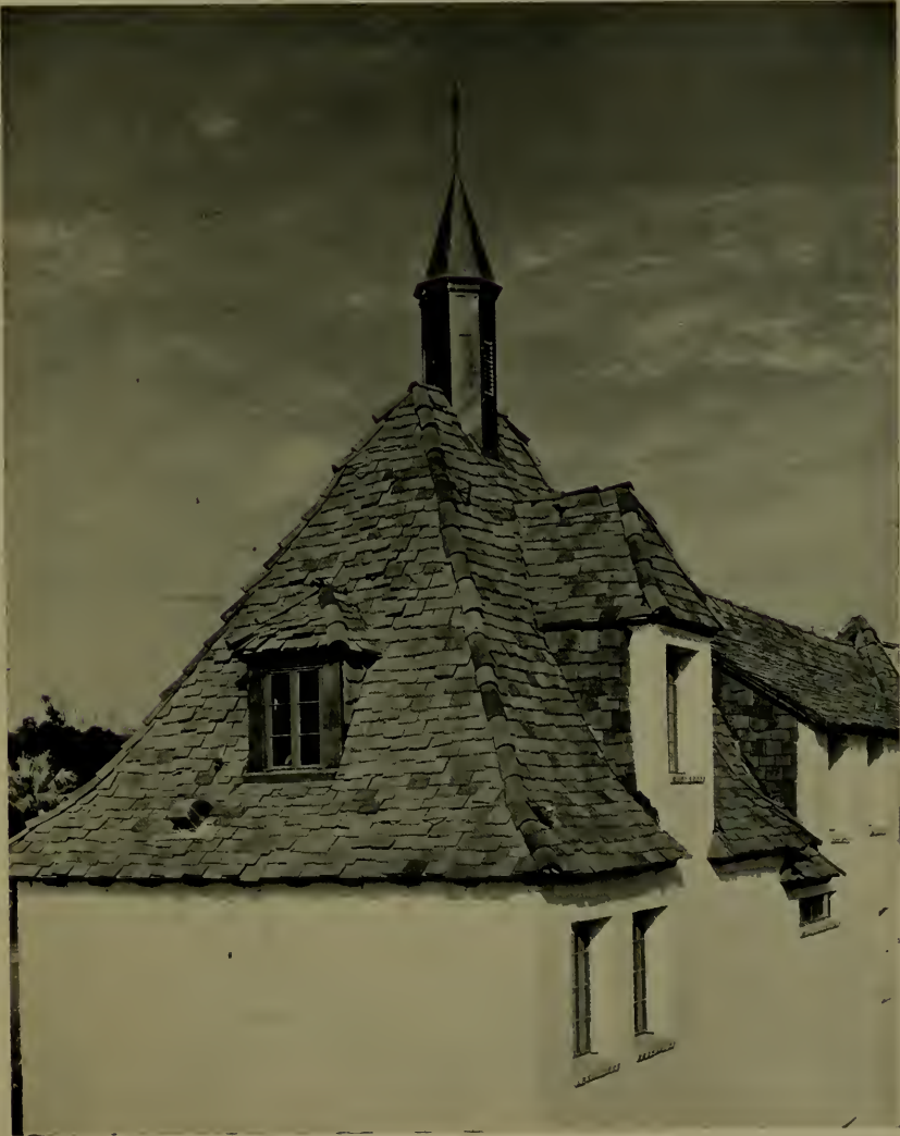
DAVIES STUDIO, LONG BEACH HUGH R. DAVIES, ARCHITECT
