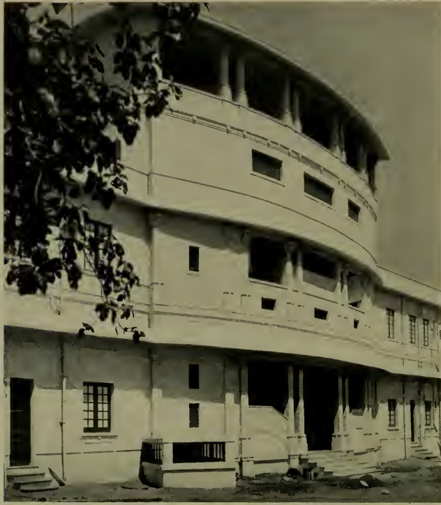
REMODELED PALACE OF THE LATE MAHARAJA SCINDIA AT WORLI, BOMBAY
