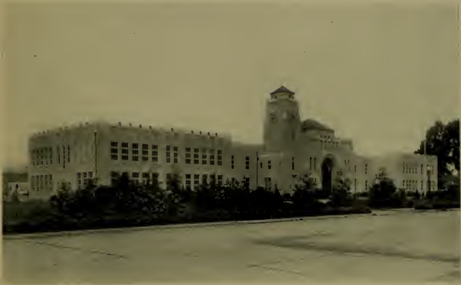
McKINLEY SCHOOL, REDWOOD CITY, CALIFORNIA Coffey and Rist, Architects
