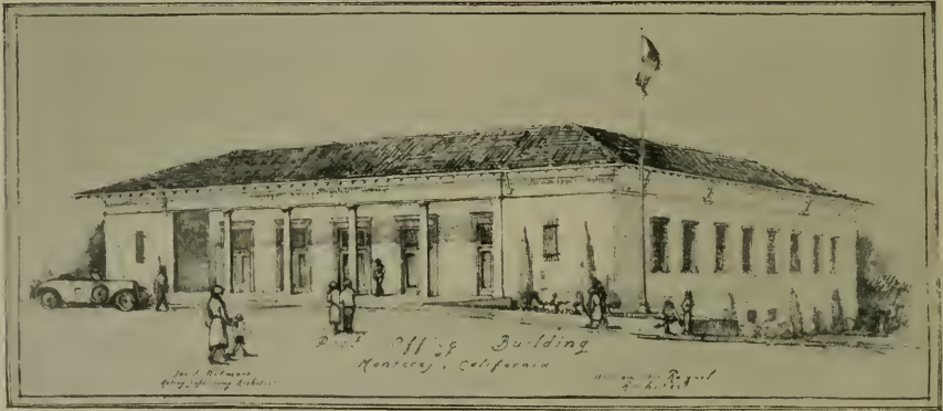
UNITED STATES POST OFFICE BUILDING, MONTEREY, CALIFORNIA William Otis Raiguel, Architect
