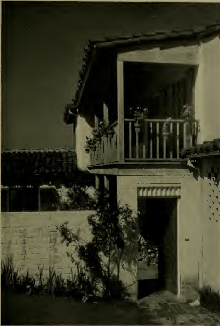
ENTRANCE DETAIL, RESIDENCE OF DR. CLYDE T. WETMORE, BERKELEY
