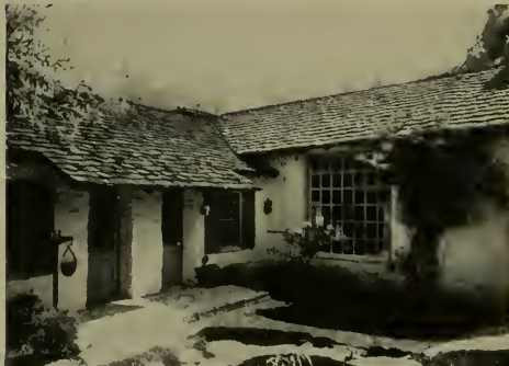
Adobe House, Pasadena, California. Roof of \frac{3}{4} " to 1" x 25" Hand Split Red Cedar tapered shakes machine-dipped in three shades (brown) of Cabot's Creosote Shingle and Wood Stains.
