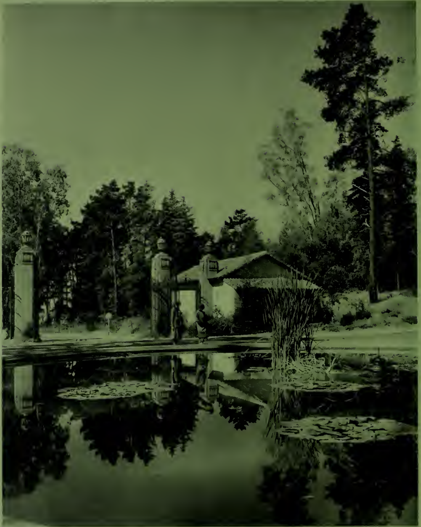
WETMORE GATE LODGE AND POOL, MILLS COLLEGE, OAKLAND, CALIFORNIA W. H. RATCLIFF, JR., ARCHITECT
