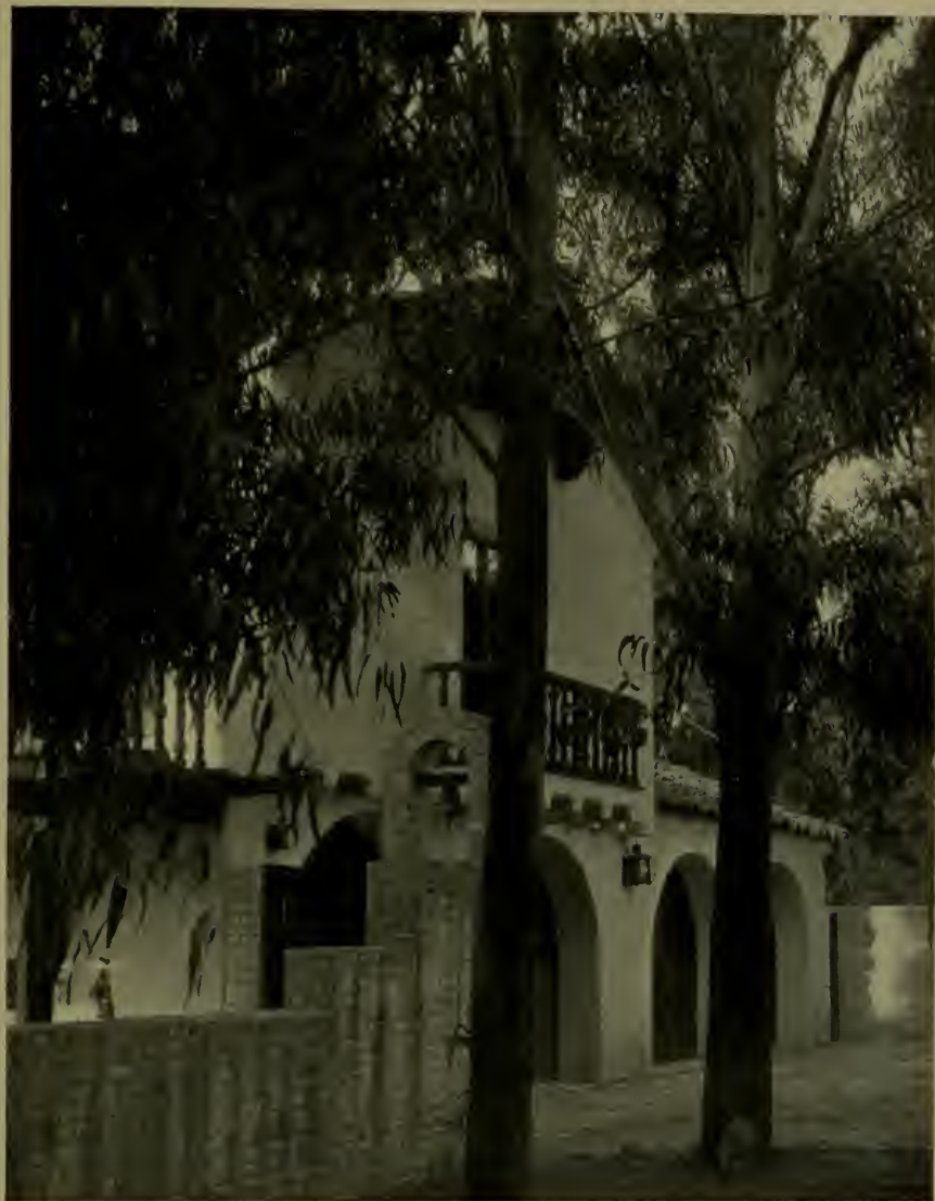
GARAGE ENTRANCE, RESIDENCE OF GEORGE FRIEND, ARLINGTON ESTATES, BERKELEY EDWIN LEWIS SNYDER, ARCHITECT
