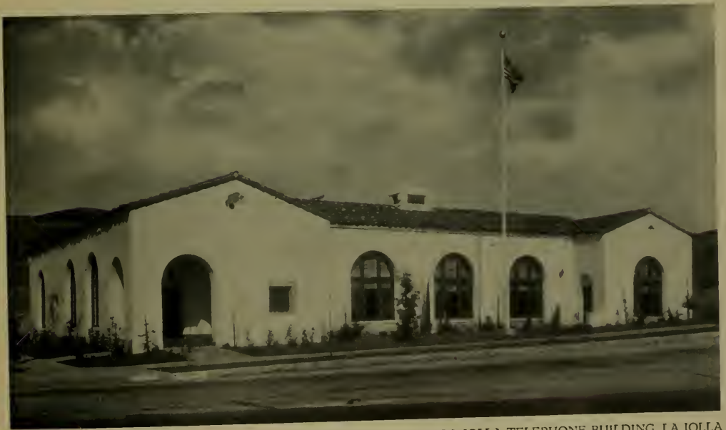
LA JOLLA TELEPHONE BUILDING, LA JOLLA G. R. Morrison, Building Engineer
