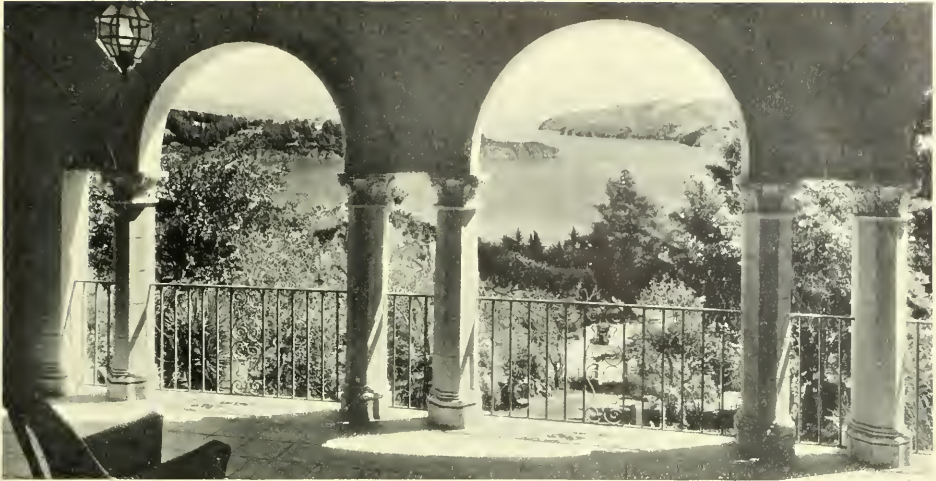
OBSERVATION PORCH, ALTA MIRA HOTEL, SAUSALITO, CALIFORNIA Fabre & Hildebrand, Architects
