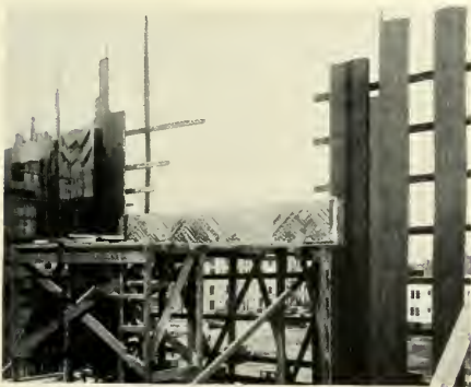
PLASTER WASTE-MOLD SET IN PLACE
