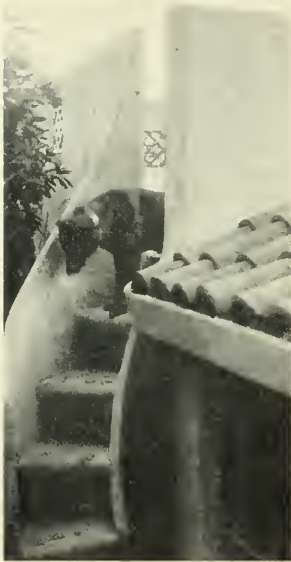
Spiral stair to roof terrace, treads, risers and rails made of stucco. The terrace parapet also of stucco. The terrace parapet also of stucco, is about 11 1/4" thick, 4" high and 8" long, reinforced with netting and 3/8" rods. Tests have proven that it has ample strength.
