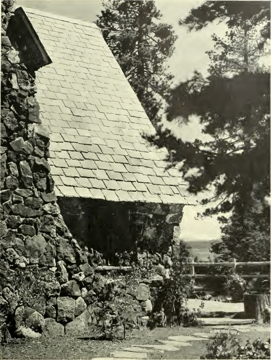
Slate Roof by General Roofing Company
