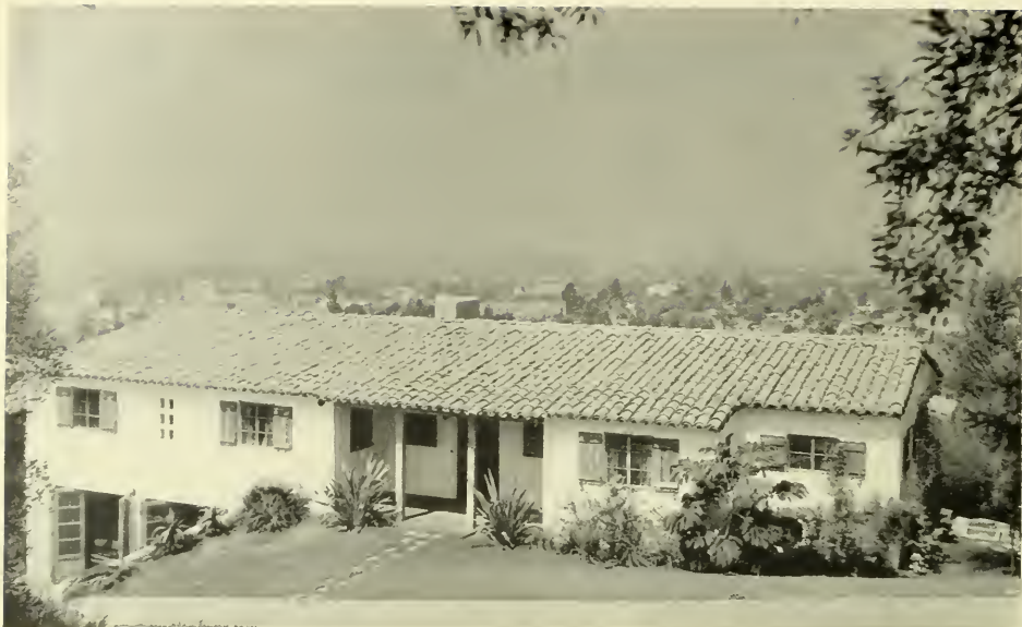
RESIDENCE OF F. W. LAKE, WHITTIER, CALIFORNIA H. Roy Kelley, Architect
