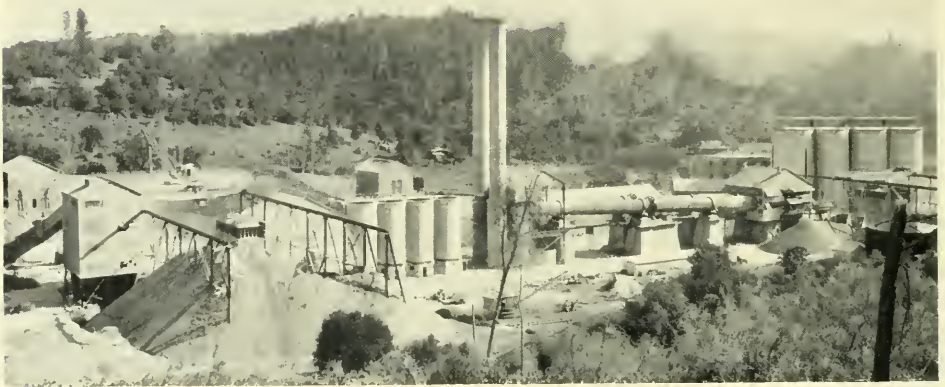
PLANT OF THE CALAVERAS CEMENT COMPANY OF SAN FRANCISCO
