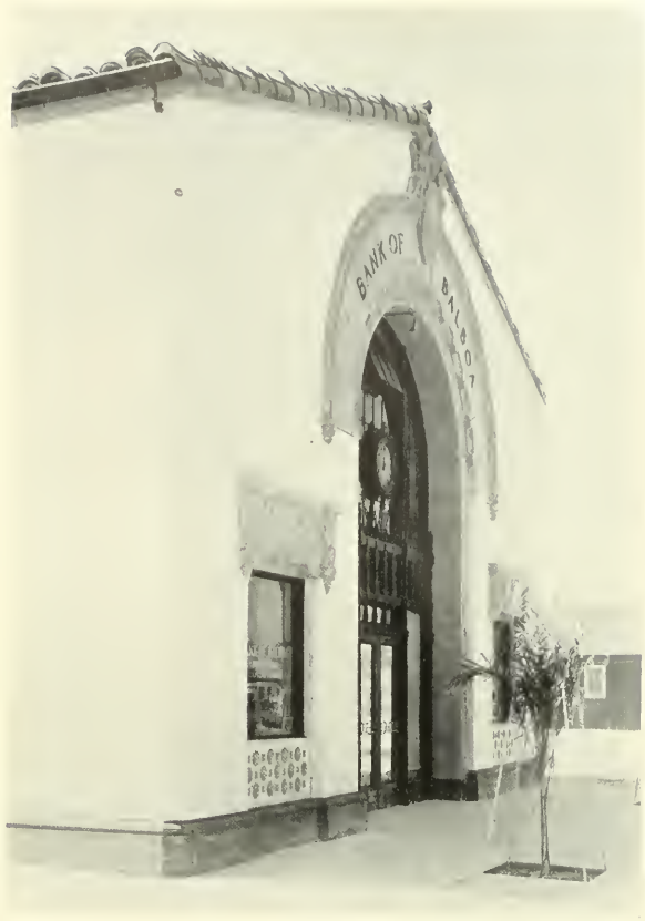
An early example of exposed concrete employing plaster molds and ordinary board forms BANK OF BALBOA, BALBOA, CALIFORNIA McGraw, Walls & Clements, Architects, Los Angeles.
