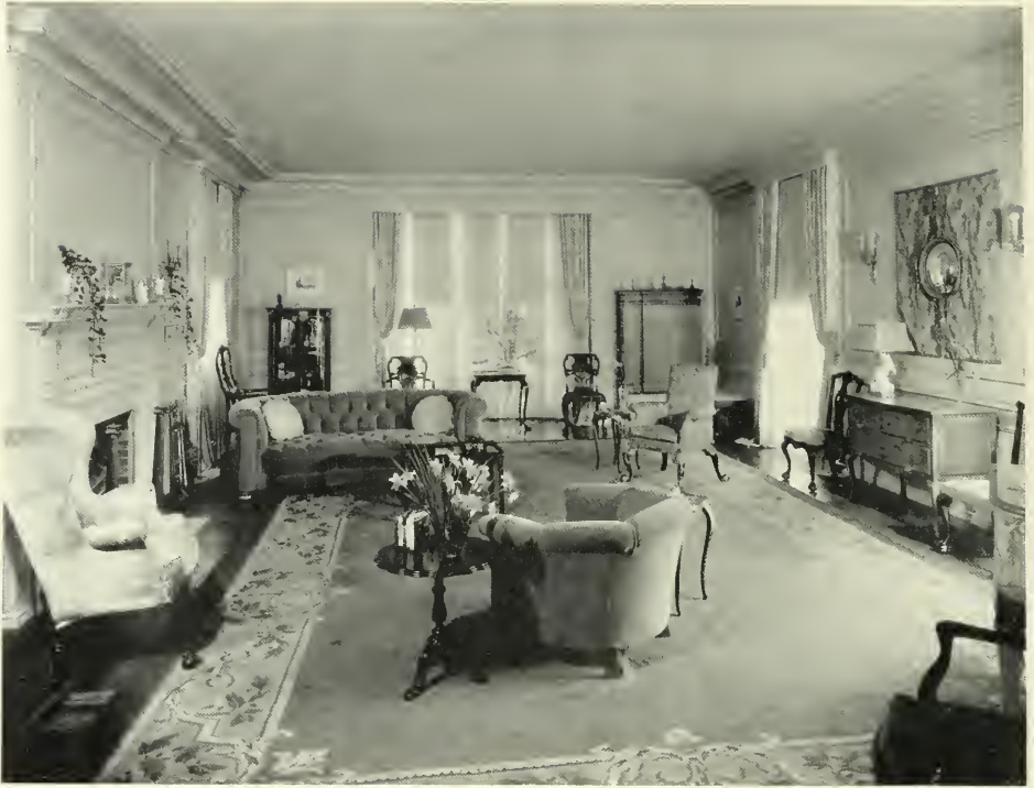
LIVING ROOM, RESIDENCE OF R. S. RHEEM, PIEDMONT, CALIFORNIA Alben Froberg, Architect
