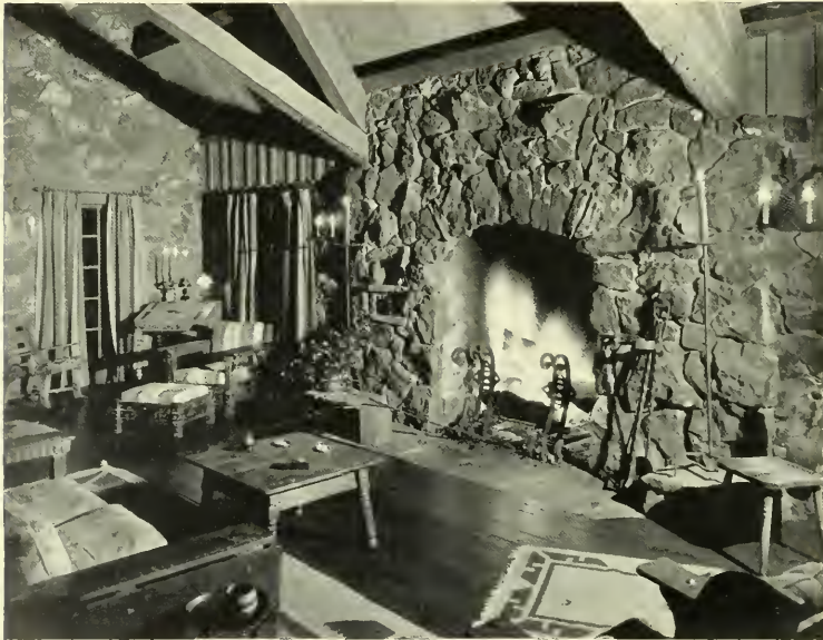
DETAIL OF FIREPLACE, HOUSE OF MRS. LAURA B. WESTPHAL, LAKE TAHOE Kent and Hass, Architects
