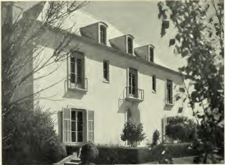
RESIDENCE OF ALBERT L. GUERARD, STANFORD UNIVERSITY John K. Branner, Architect
