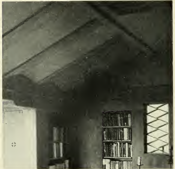
Detail of living room. Ceiling panels of fibre-board, in V form to improve acoustics. Rafters and girders of concrete (Method C). Book cases recessed in wall-hollows. Leaded sash plastered in without frame. Pivoted Fabricrete door with perforated tile as handle. General illumination of room is through ceiling panels consisting of stucco grilles glazed with flat Phillipine shell.
