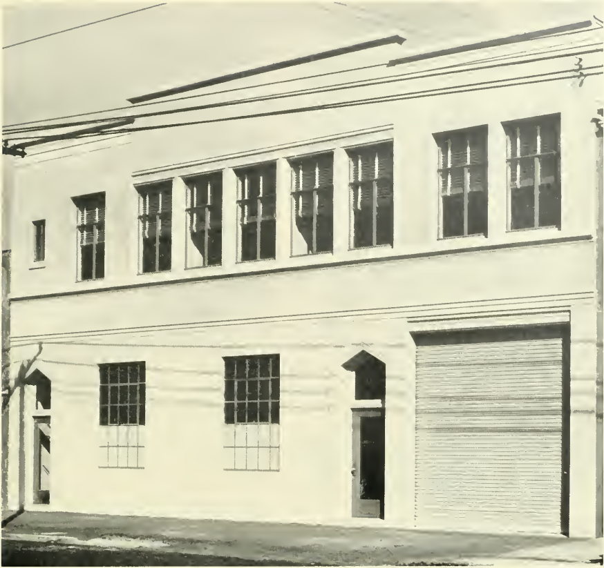
OFFICE AND WAREHOUSE FOR LARSEN & LARSEN, SAN FRANCISCO Kent and Hass, Architects
