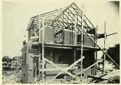
Steel frame in place and part of the outer brick work in position
