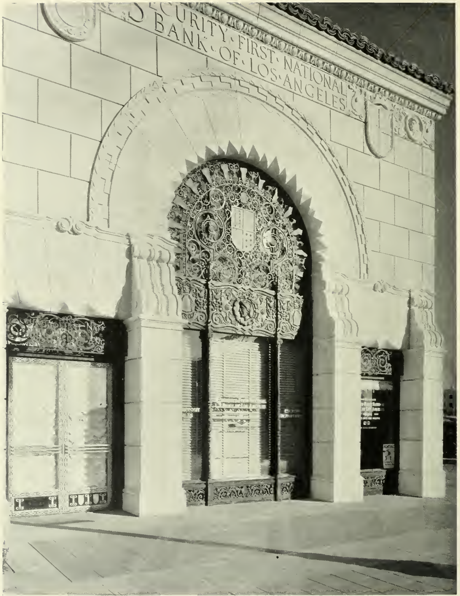
Fibre board lined forms and plaster molds were used
