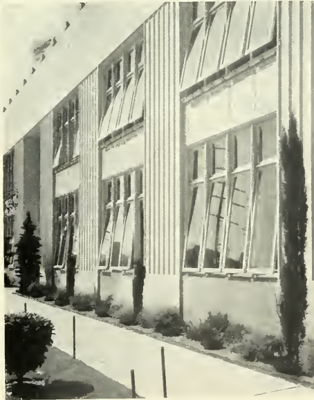
DETAIL OF FACADE, TIMES BUILDING, SEATTLE R. C. Reamer, Architect
