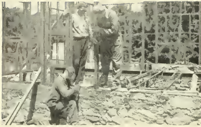
Welder at work making joint at foundations
