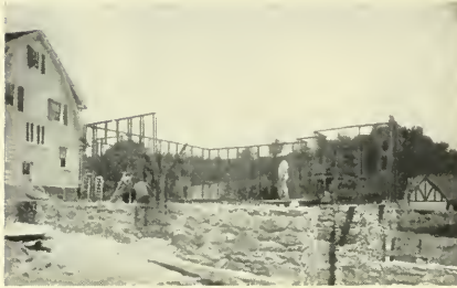
Steel frame on foundations in early stages of construction
