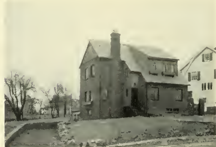
General View of the completed dwelling
