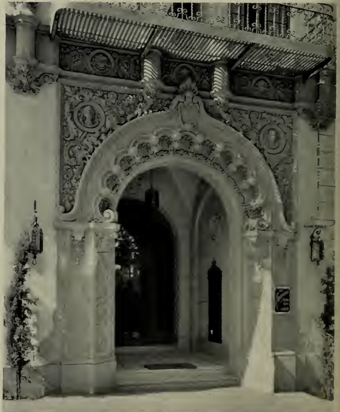
DETAIL, ENTRANCE, JEANNE ARMS APARTMENTS Albert H. Larsen, Architect
