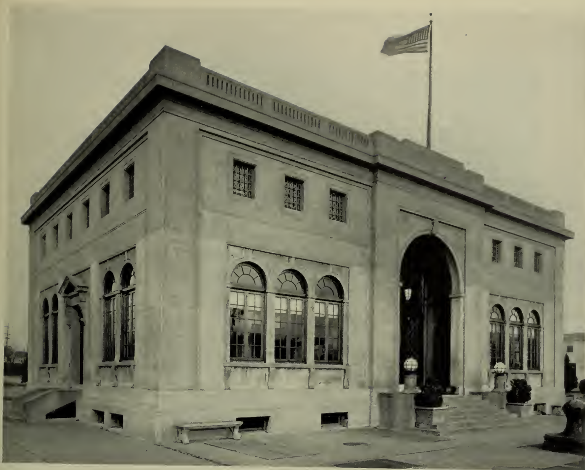
OPERATING HOUSE, U. S. GOVERNMENT LOCKS, BALLARD, WASHINGTON
