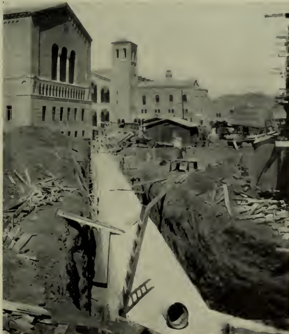
SERVICE TUNNEL, UNIVERSITY OF CALIFORNIA AT LOS ANGELES
