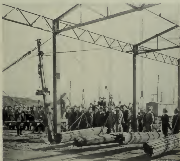
IMPACT LOAD PRODUCING SUDDEN HORIZONTAL PULL OF OVER 2000 POUNDS AT WELDED CON- NECTION OF TRUSS
