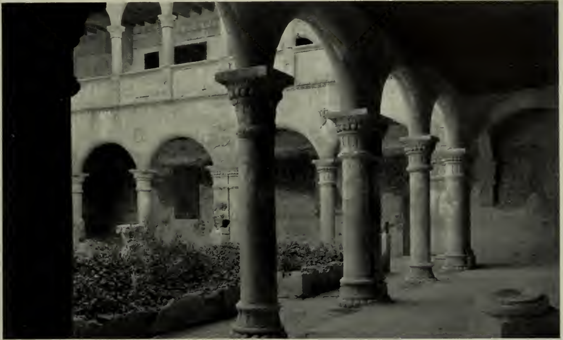
MAJOR CLOISTER, CONVENT OF SAN AUGUSTIN ACOLMAN, NEAR SAN JUAN TEOTIHUACAN. NOTE FORCEFUL BEAUTY IN STONE CARVING
