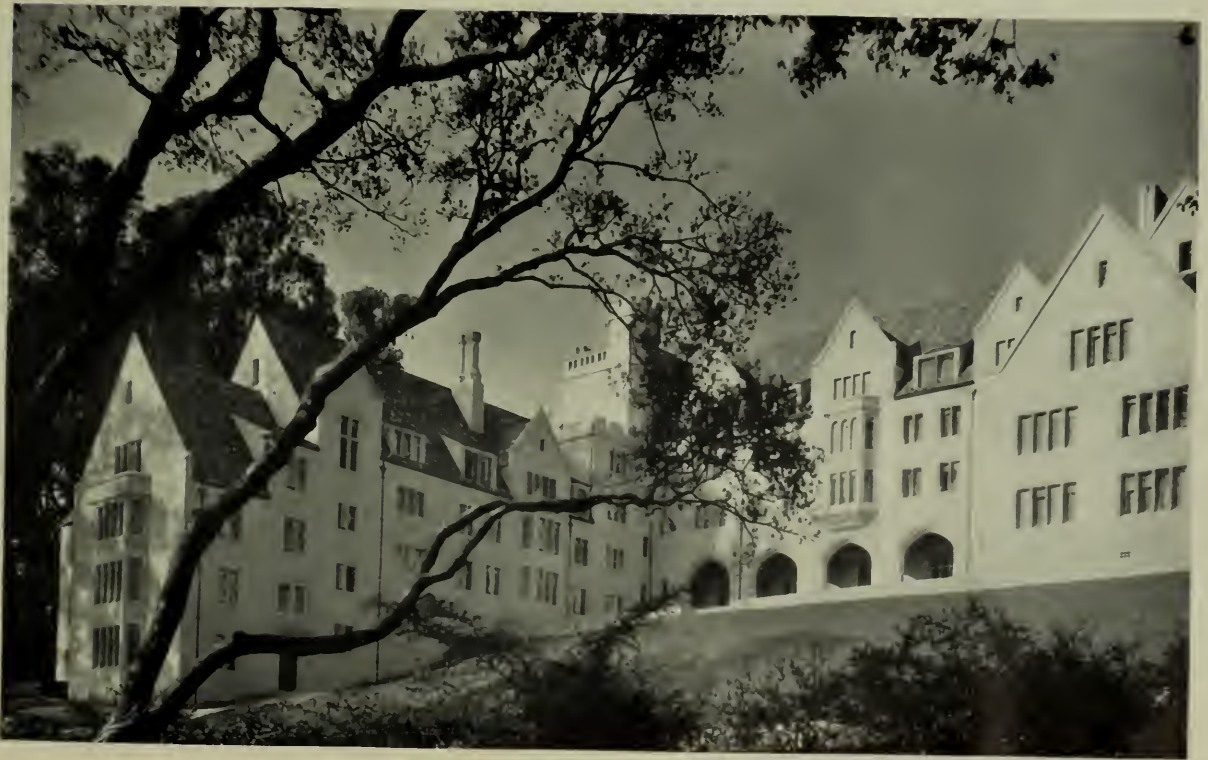
BOWLES HALL, UNIVERSITY OF CALIFORNIA, BERKELEY GEORGE W. KELHAM, ARCHITECT
