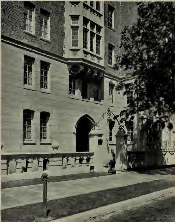
ENTRANCE, TUDOR HALL APARTMENTS Miller and Warnecke, Architects
