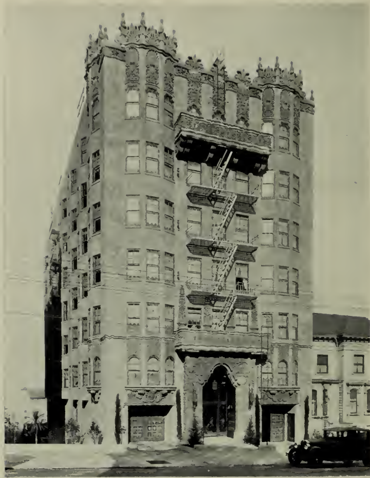
APARTMENT HOUSE, PACIFIC AVENUE NEAR LAGUNA, SAN FRANCISCO Douglas Dacre Stone, Architect
