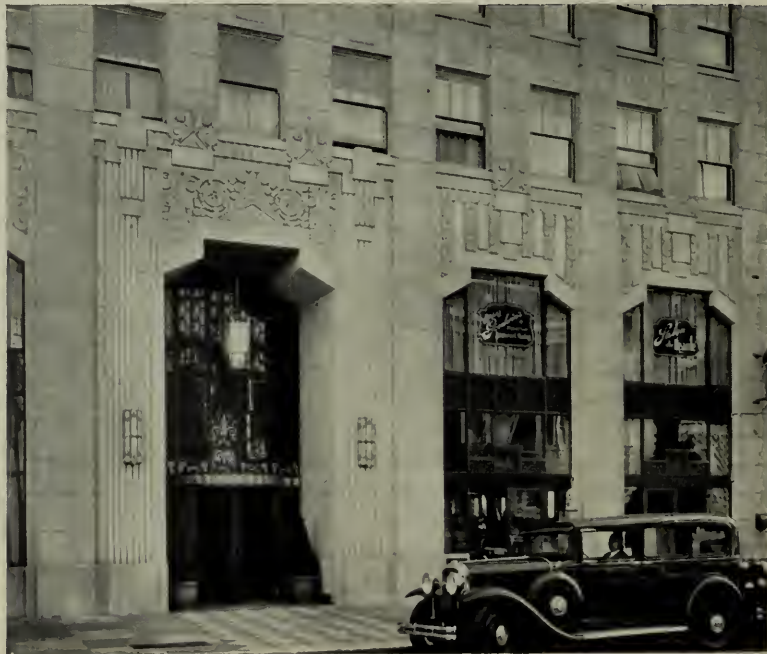
DETAIL, LOWER STORIES, ALEXANDER HAMILTON APARTMENTS, SAN FRANCISCO Albert H. Larsen, Architect
