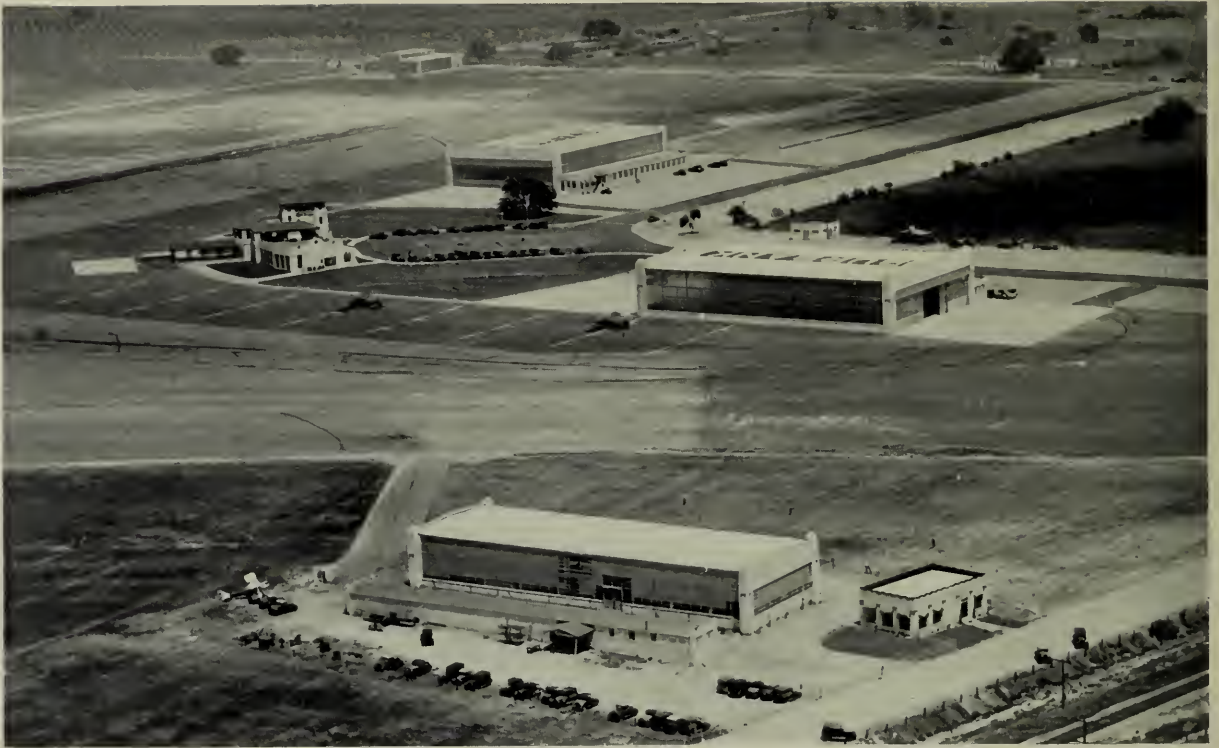
UNITED AIRPORT LANDING FIELD, BURBANK, CALIFORNIA The Austin Company, Designers and Builders
