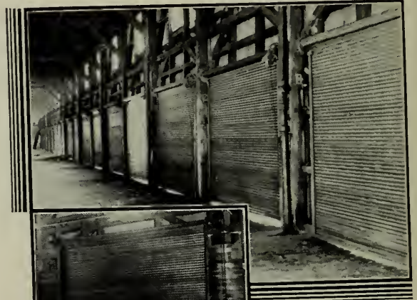
(Upper View) Kinnear Rolling Doors installed in 1897 in the P.C.C. & St. L. R. R. freight house at Columbus, Ohio. (Lower View) A 35 year old counterweighted Kinnear Door still in perfect operating condition.
