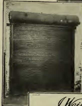
Unretouched photographs, taken April 8th, 1930, of the Kinneair Automatic Rolling Doors installed in the Weiskopf Building in 1912, as they appear after eighteen years of continuous service and fire protection duty.
