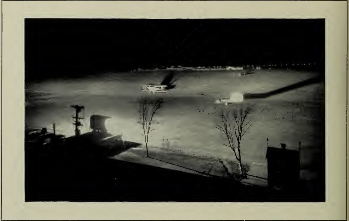
NIGHT VIEW OF BOLLING FIELD, WASHINGTON, D. C. Lighted with General Electric, Type ALH 24 Kw. Floodlight
