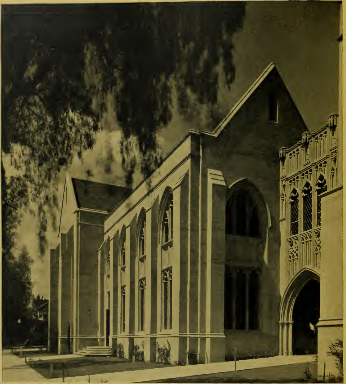
Methodist Episcopal Church, Hollywood, California. Thomas P. Barber, Architect
