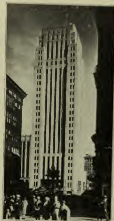
RAND TOWER, MINNEAPOLIS Holabird & Root, Architects
