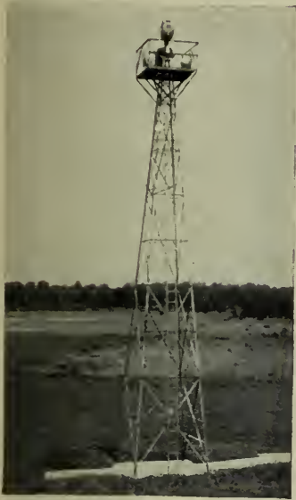
Beacon and On-course Lights Mounted on Steel Tower
