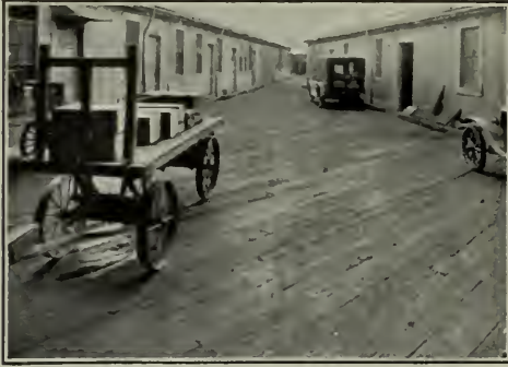
San Francisco Ferry Building Dock—floored with Port Orford Cedar nine years ago. Constant jar and the wear of steel-tired trucks have affected it but little.
