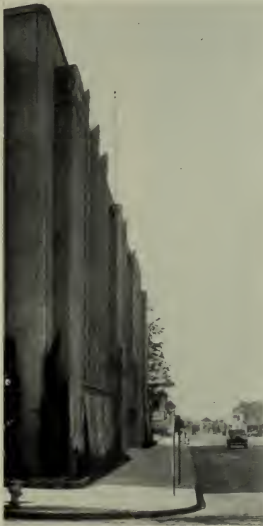
KITTRIDGE STREET FRONTAGE LIBRARY BUILDING, BERKELEY
