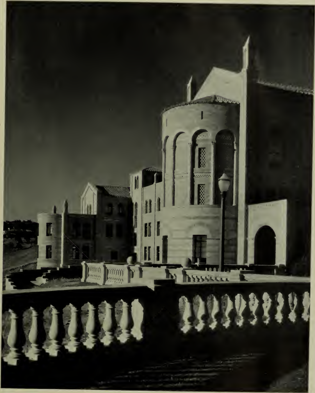
ROYCE HALL, UNIVERSITY OF CALIFORNIA AT LOS ANGELES ALLISON AND ALLISON, ARCHITECTS GEORGE W. KELHAM, SUPERVISING ARCHITECT
