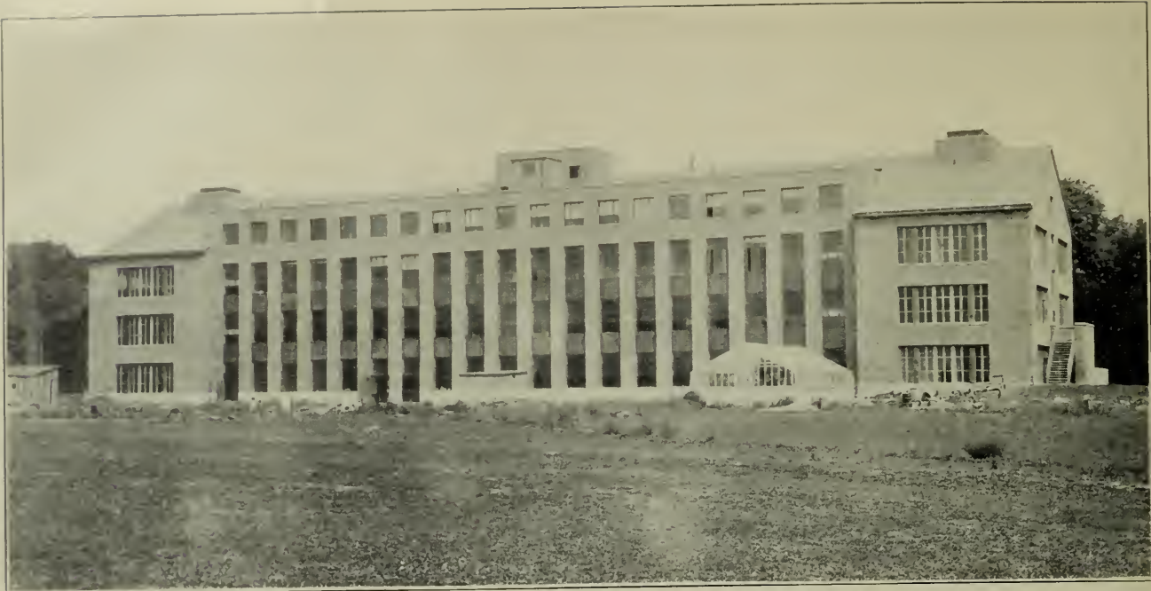
In this General Science Building of Antioch College, Yellow Springs, Ohio, 28 tons of 16, 18 and 22 gauge galvanized INGOT IRON was used for the duct work, which carries moisture and corrosive chemical fumes from 27 laboratories. INGOT IRON was chosen on the strength of its eminent past performance under all kinds of corrosive conditions.
