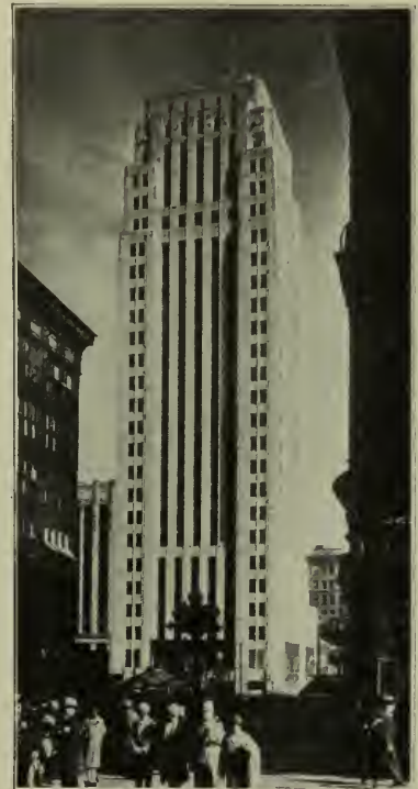
RAND TOWER, MINNEAPOLIS Holabird & Root, Architects
