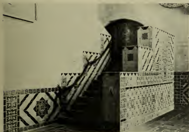
Stairway of Tunisian Tile with Floors and Steps of Fallston Tile Santa Barbara Courthouse Wm. Mooser, Architect
