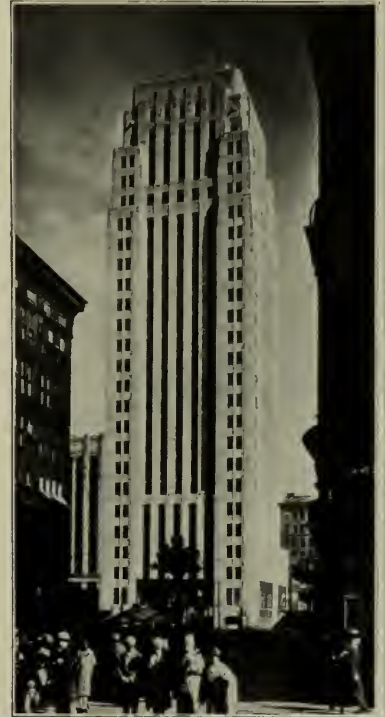
RAND TOWER, MINNEAPOLIS Holabird & Root, Architects
