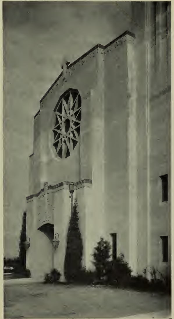
DETAILS, FRONT OF CHURCH, SHOWING CONCRETE TEXTURE SURFACE AND TERRA COTTA LINTEL
