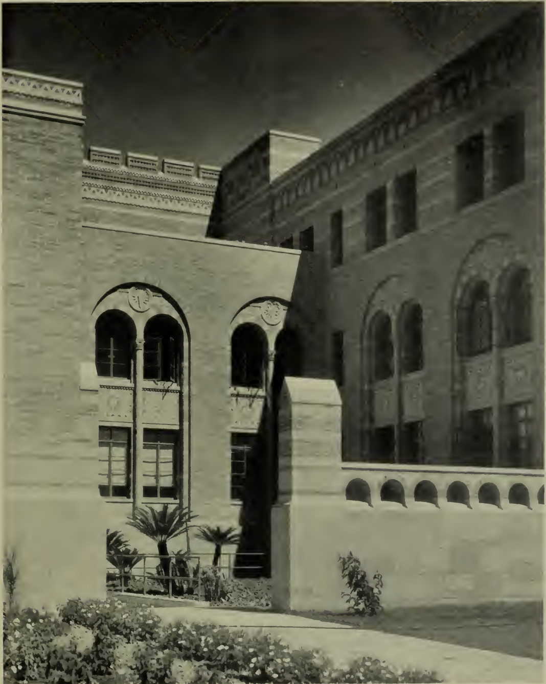
PHYSICS BUILDING, UNIVERSITY OF CALIFORNIA AT LOS ANGELES
