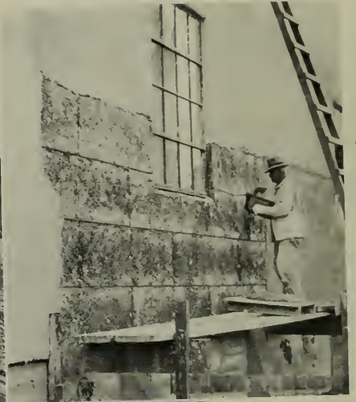
Applying the Finish Coat to Fireproof Wall of "Thermax"
