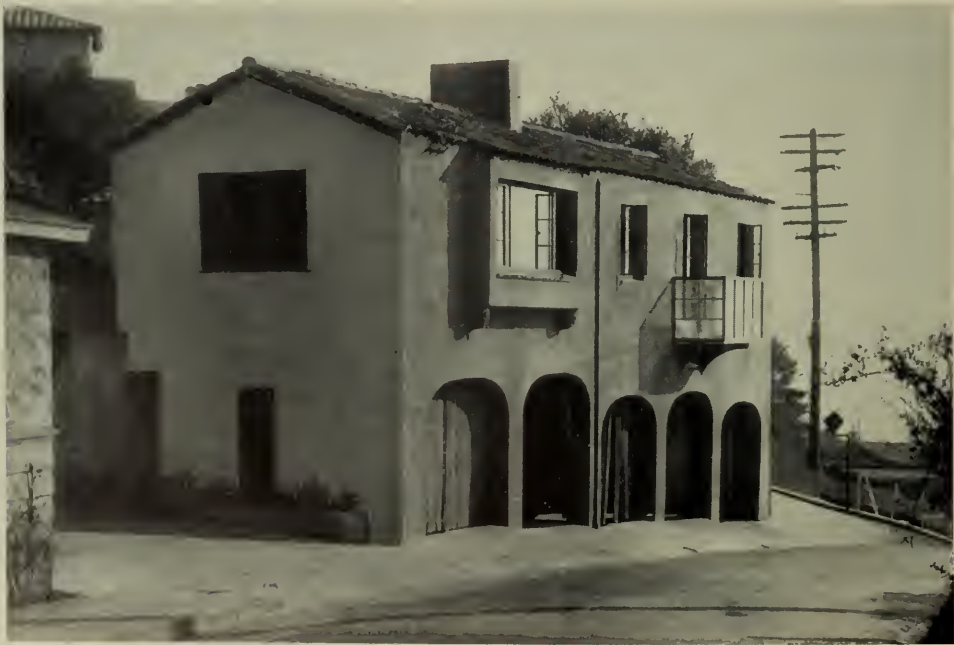
GARAGES AND APARTMENT AT 6 MOSSWOOD ROAD, BERKELEY NEARING COMPLETION, FEBRUARY, 1931
