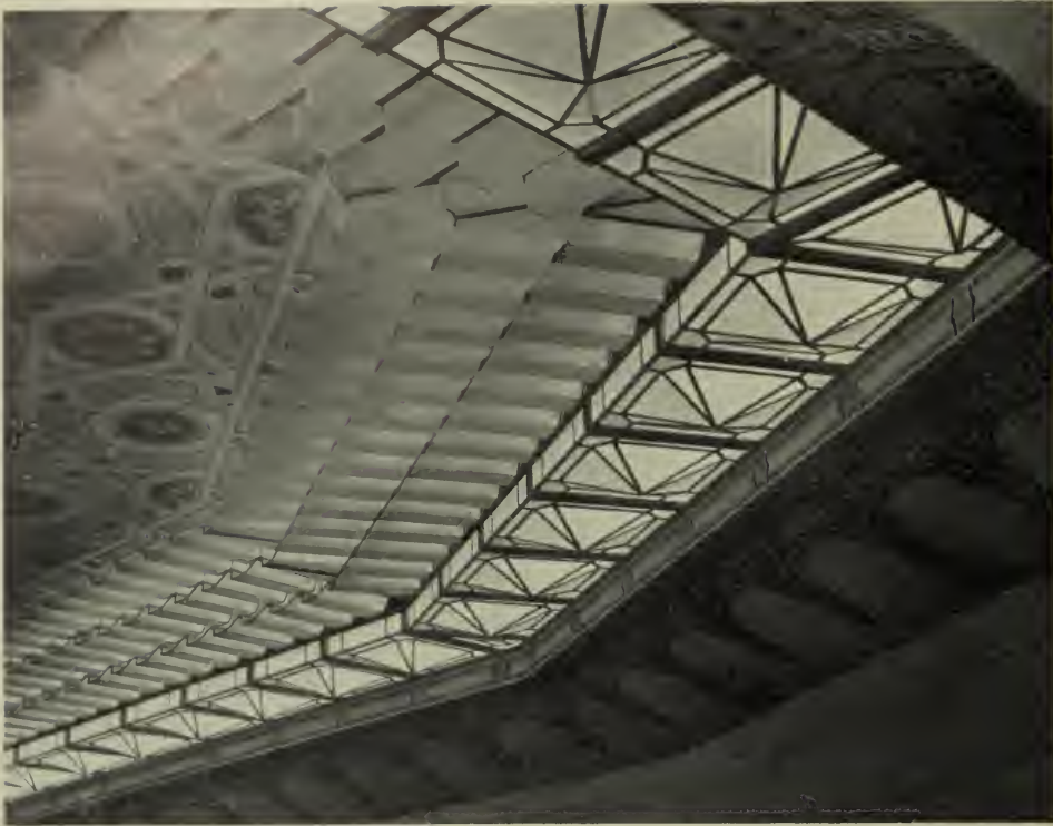
CRYSTAL-LIKE LIGHTING IN CEILING OF BOARD ROOM, STOCK EXCHANGE LOS ANGELES
