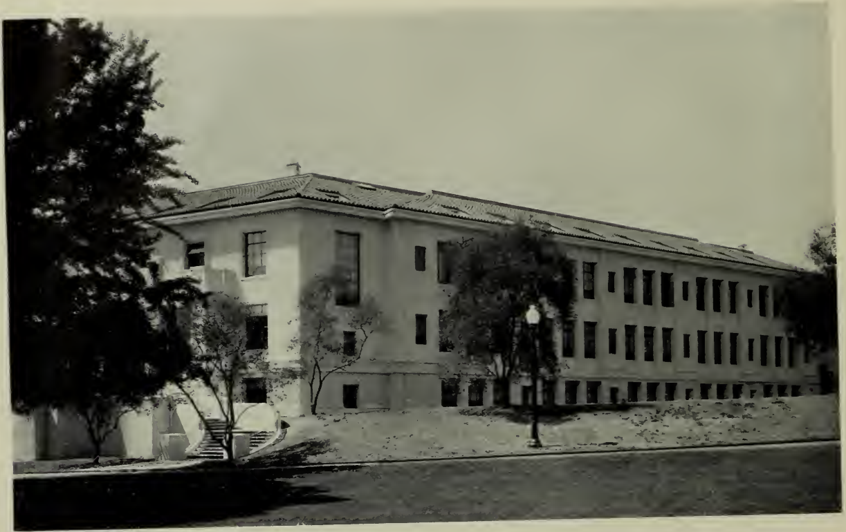
GIANNINI HALL, UNIVERSITY OF CALIFORNIA, BERKELEY William C. Hays, Architect
