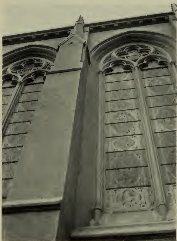
DETAIL OF BUTTRESS, GRACE CATHEDRAL CHAPEL, SAN FRANCISCO
