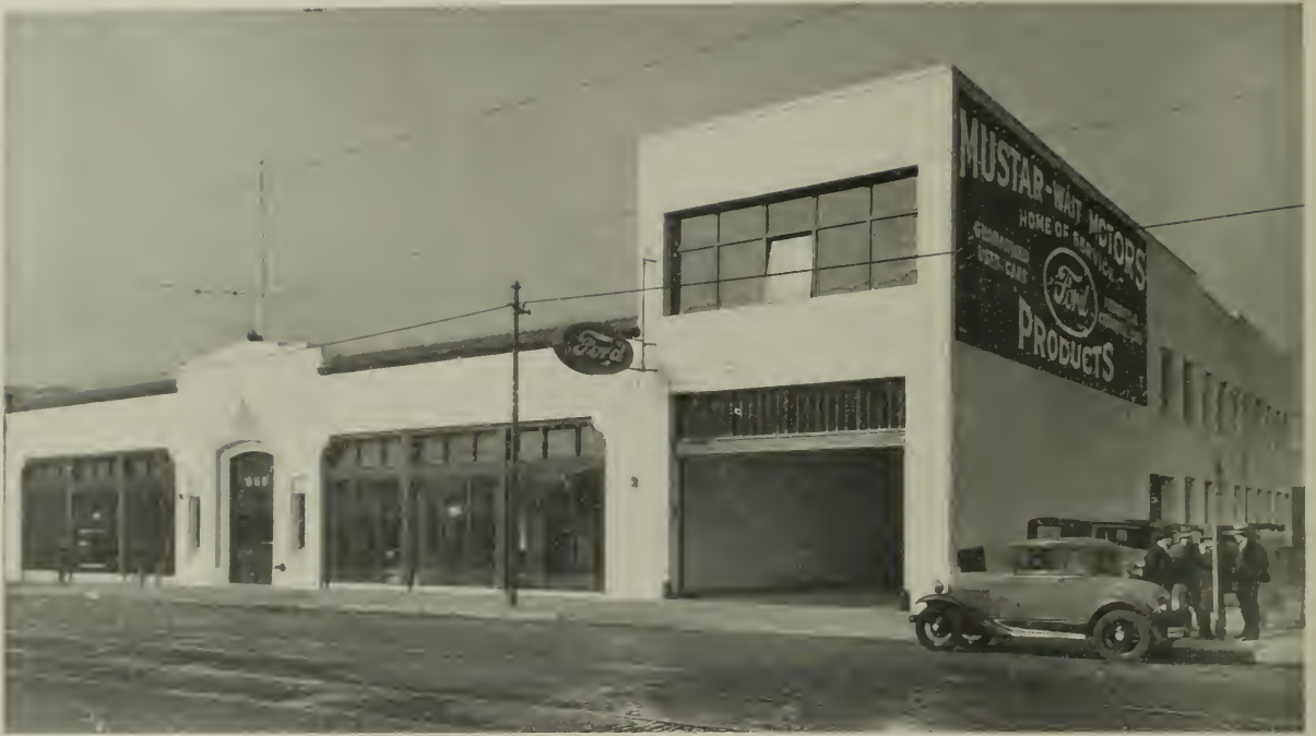
REMODELED BUILDING, 860 HOWARD STREET, SAN FRANCISCO Villadsen Bros., Engineers and Contractors
