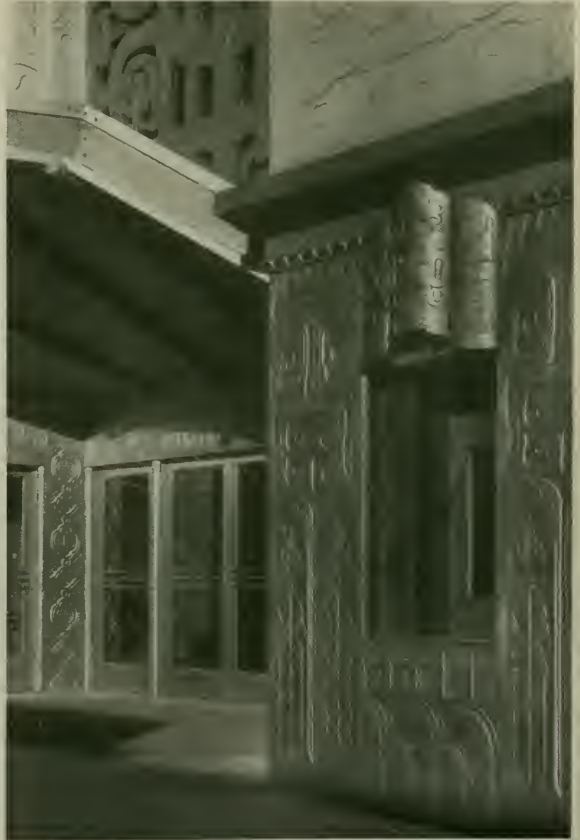
ENTRANCE DETAIL, FOUR FIFTY SUTTER J. R. Miller and T. L. Pfeuger, Architects
