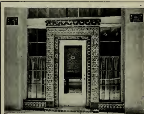
Detail of Entrance, Rossman Warehouse, San Francisco FRED K. H. MEYER, Architect
