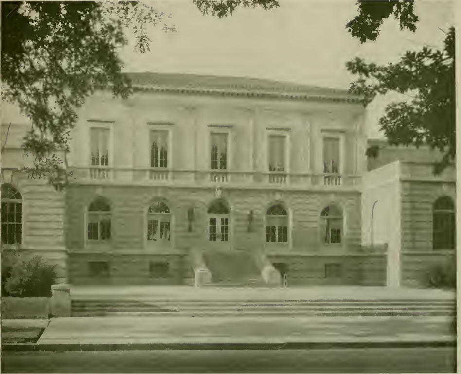
MOREY JUNIOR HIGH SCHOOL, DENVER, COLORADO William E. Fisher and Arthur A. Fisher, Architects
