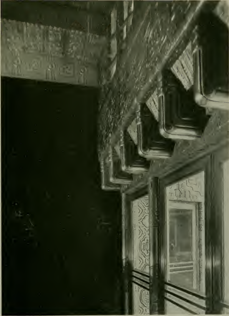
FORMS IN METAL, FOUR FIFTY SUTTER, SAN FRANCISCO J. R. Miller and T. L. Pflueger, Architects
