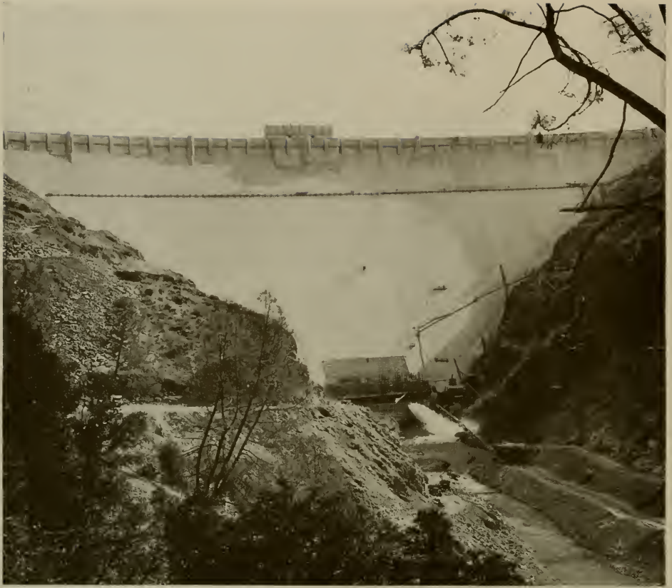
CLOSE-UP OF PARDEE DAM UNDER CONSTRUCTION
