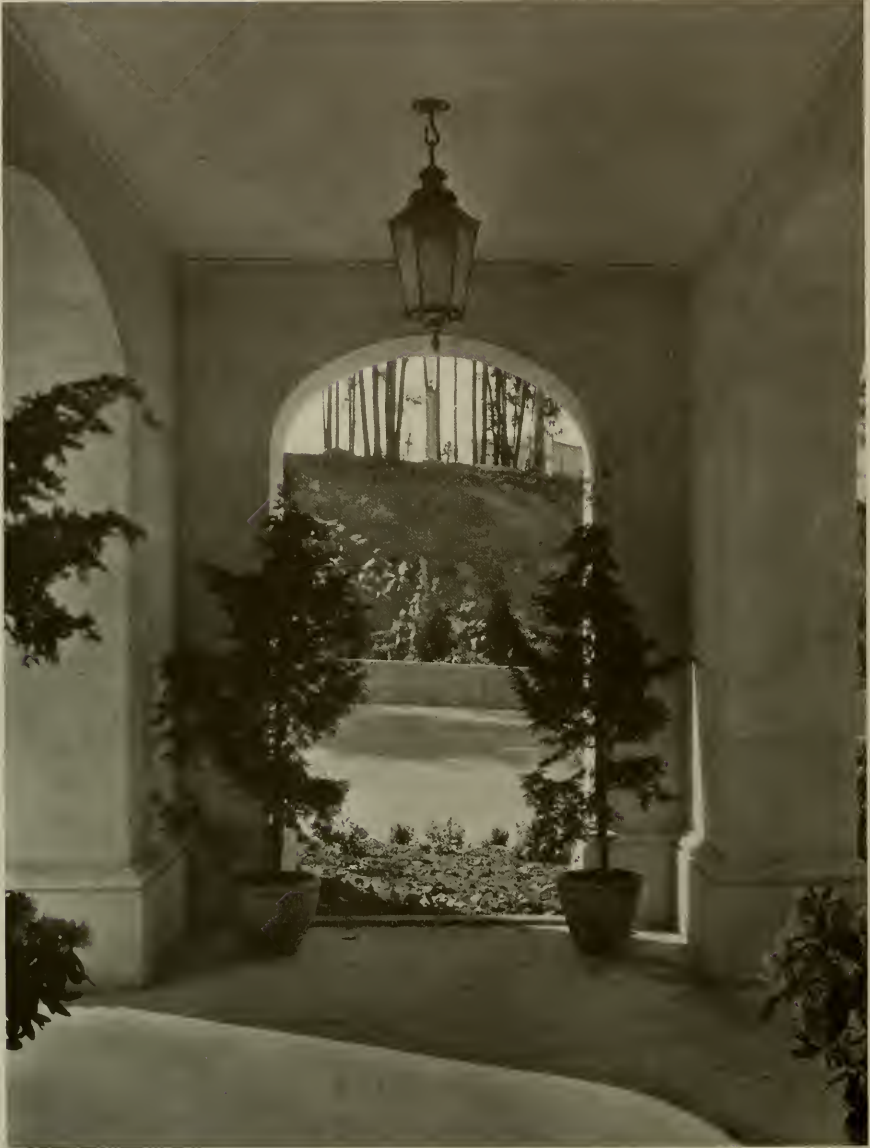
PORTE COCHERE, CHRISTIAN SCIENCE SANATORIUM, SAN FRANCISCO HENRY H. GUTTERSON, ARCHITECT
