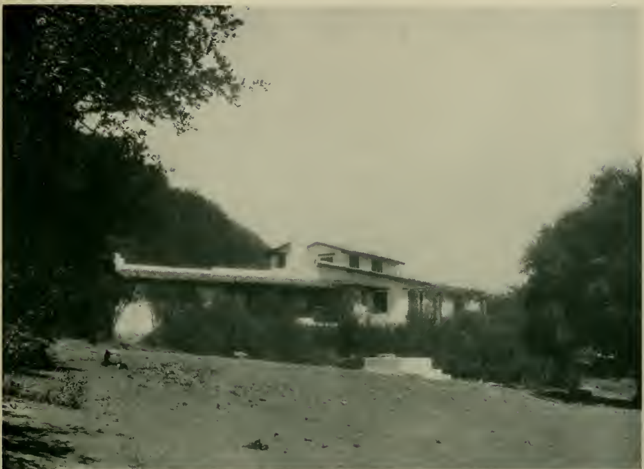
RANCH HOUSE FOR MAJOR L. H. FRENCH, LAS TURAS LAKE John Byers, Architect
