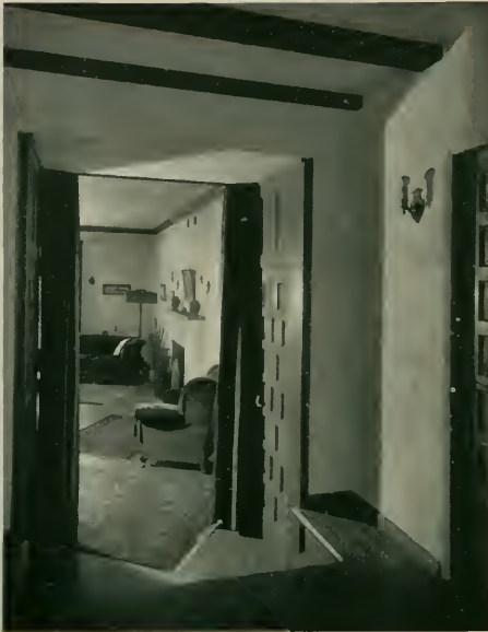
HALLWAY, RESIDENCE OF FRED S. McCORD Masten and Hurd, Architects
