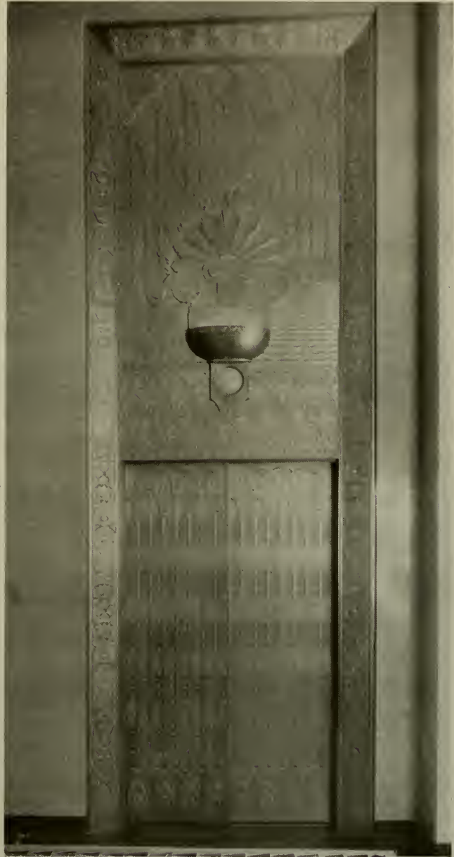
DETAIL, ELEVATOR DOOR, SHELL BUILDING, SAN FRANCISCO Geo. W. Kelham, Architect
