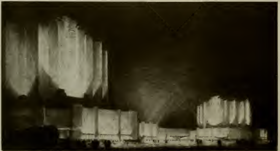
TRAVEL AND TRANSPORTATION BUILDING, 1933 WORLD'S FAIR, CHICAGO, ILLINOIS
