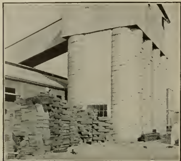
Battery of eight storage bins for crushed slate. Port Orford Cedar was chosen for this job because of its durability, because it shrinks but little.
