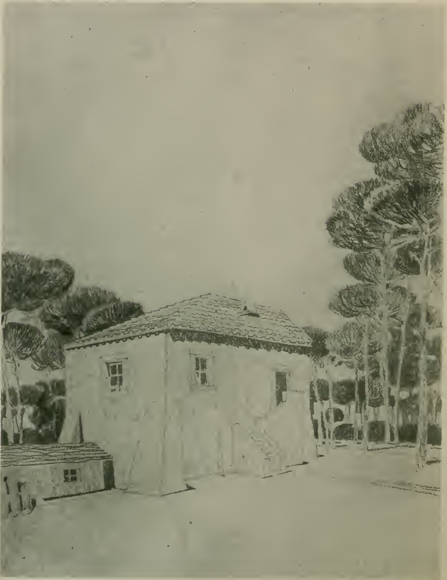
FARM HOUSE NEAR ROME
