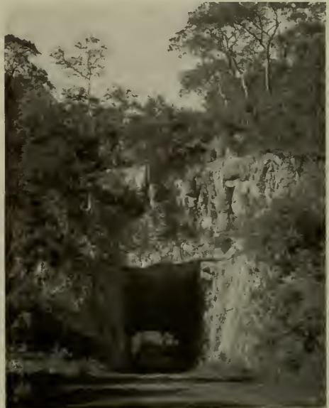
Tunnel cut through solid stone, in wild Zopelote Canyon, in the State of Guerrero, on the major highway from Mexico City to Acapulco, one of the finest natural harbors on the Pacific. Photograph, courtesy of National Highway Commission of Mexico.
