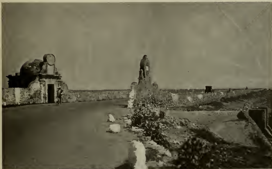
Sluice Gate House with dome on the left and Shrine, on the right, built of stone, and Spanish Colonial in design. On the Pachuca Highway which passes between two long stone dykes. Photograph by the author.
