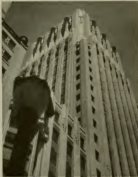
VERTICAL VIEW OF TOWER, SHELL BUILDING Geo. W. Kelham, Architect
