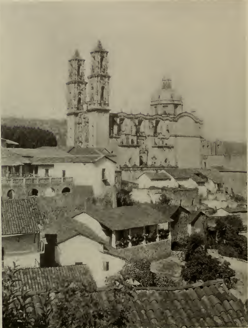
The Parochial Church of Taxco, built by Jose de la Borda, was completed in 1757. The stone is of a warm buff color tinged with pink and the carvings are rich, both on the exterior and interior. The dome is of polychrome glazed tile in yellow, green and blue. Photograph by author.
