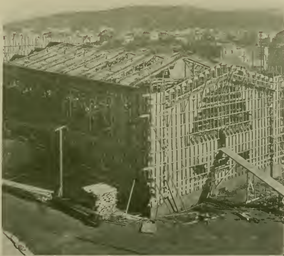
CONCRETE ARCH FRAMING OVER GYMNASIUM
