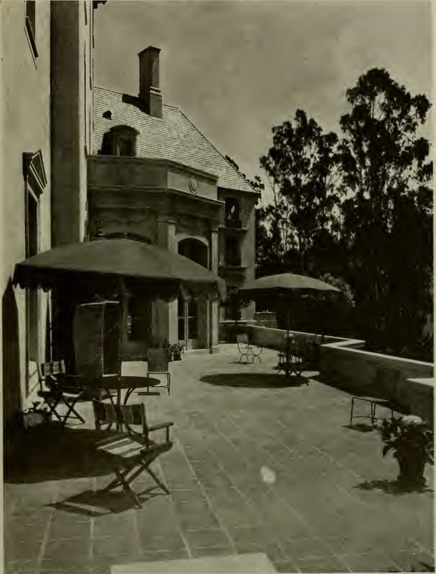
MAIN FLOOR TERRACE, CHRISTIAN SCIENCE SANATORIUM, SAN FRANCISCO HENRY H. GUTTERSON, ARCHITECT
