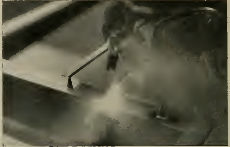
ARC WELDING TO PURLINS, WORKING FROM TOP OF ROOF
