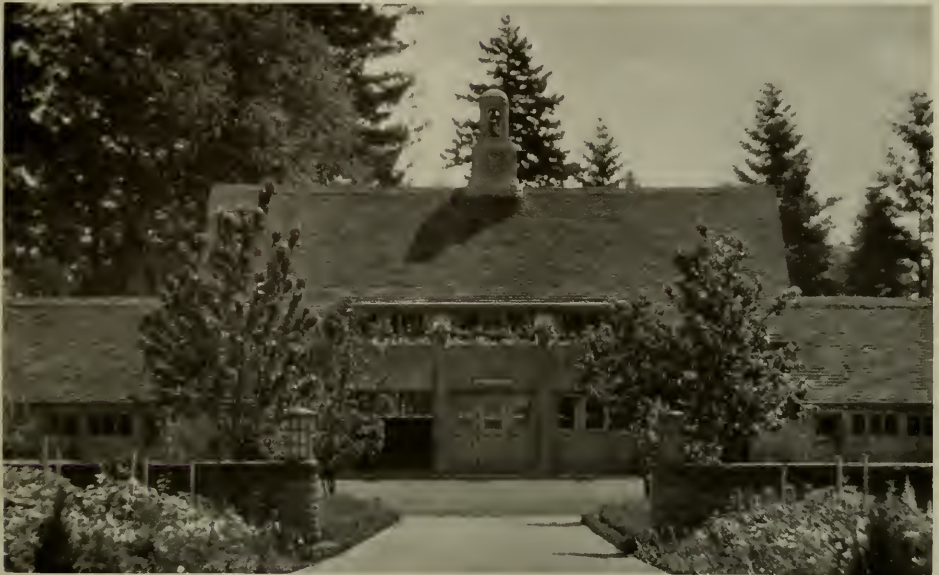
GARAGE ENTRANCE, ESTATE OF M. LLOYD FRANK, PORTLAND Herman Brookman, Architect
