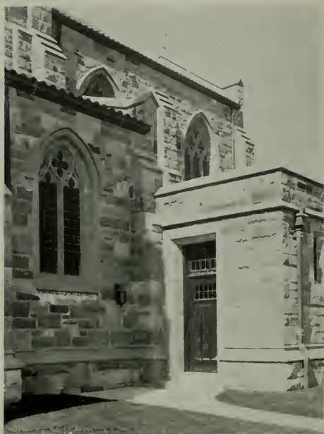
VIEW SHOWING EFFECT OF CONCRETE TRIM STONE IN FIELD OF NATURAL SANDSTONE
