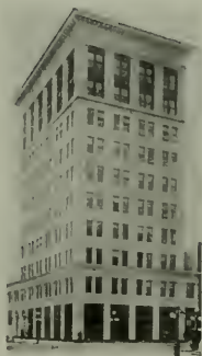
CALIFORNIA FRUIT BUILDING, SACRAMENTO CHARLES S. KAISER , Architect This building is Waterproofed and Coated with
