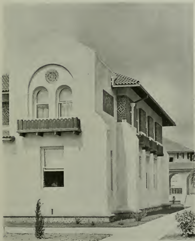
DETAIL, END OF TREATMENT BUILDING, AGNEW STATE HOSPITAL
