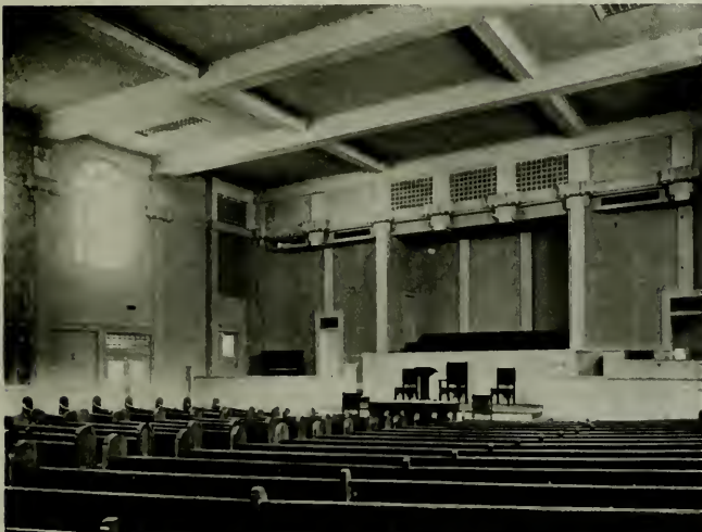
INTERIOR, CENTRAL CHRISTIAN CHURCH, PHOENIX, ARIZONA Robert H. Orr, Architect
