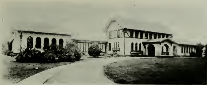
RECEIVING BUILDING, STATE HOSPITAL, NAPA
