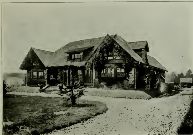
THE SHINGLE ROOF LOOKS WELL ON A HOUSE OF THIS TYPE
