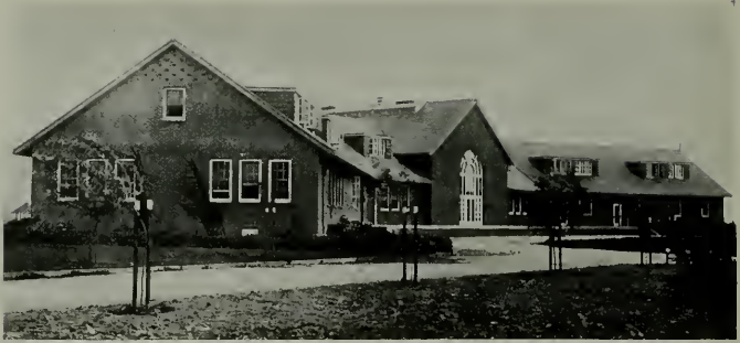
KITCHEN BUILDING, NORWALK STATE HOSPITAL
