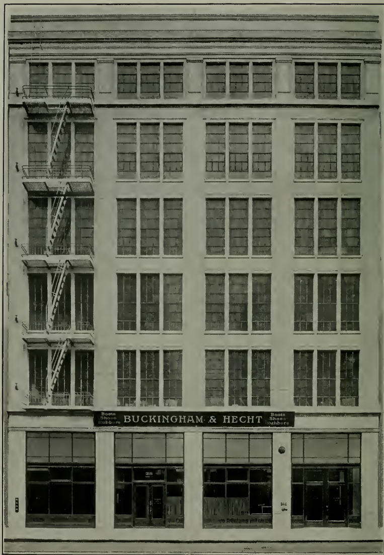
BUILDING FOR BUCKINGHAM & HECHT BAKEWELL & BROWN, ARCHITECTS
