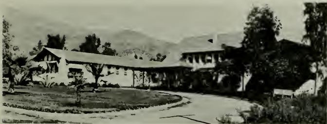
RECEIVING BUILDING, SOUTHERN CALIFORNIA STATE HOSPITAL
