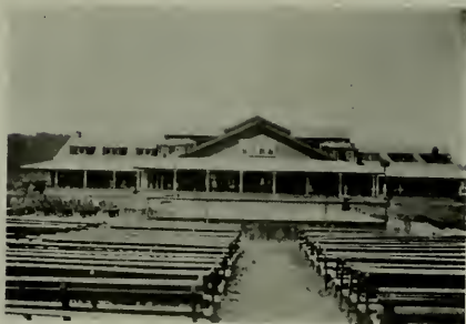
COMMUNITY HOUSE, CAMP SHERMAN, CHILLICOTHE, OHIO
