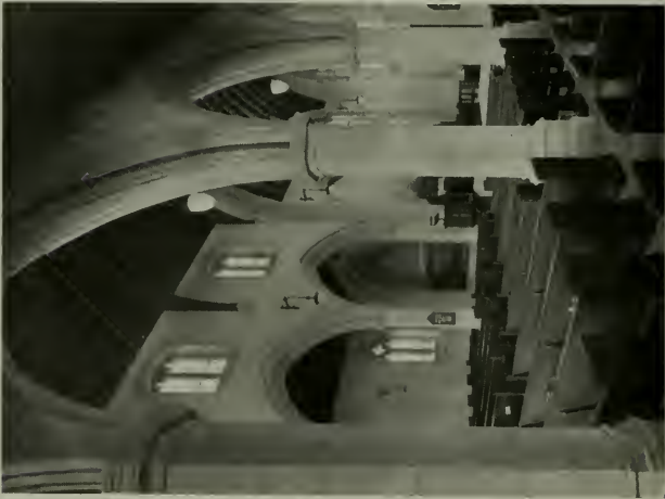
INTERIOR OF SANTA BARBARA CHURCH, SHOWING TRIM OF CONCRETE STONE Frohman & Martin, Architects
