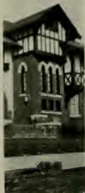
Here, the masonry character of the walls makes slate the consistent roof covering.
