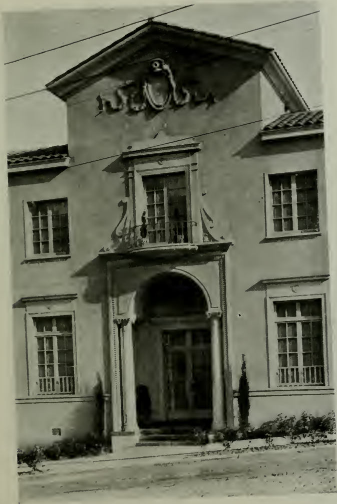
MISS BURKE'S SCHOOL. MAIN ENTRANCE DETAIL
