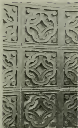
THE METHODIST CHINESE MISSION, MAIN ENTRANCE. DETAILS OF VAULT, SOFFIT AND KEY BLOCK.
