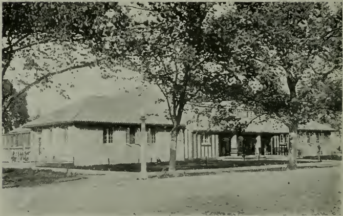
WARD BUILDING, STATE HOSPITAL, STOCKTON
