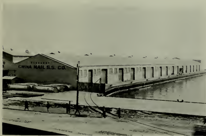
PIER 29, SAN FRANCISCO WATER FRONT Built by Clinton Construction Company
