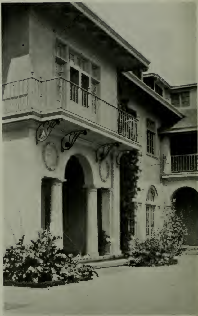
MISS RANSOM AND MISS BRIDGES' SCHOOL, PIEDMONT. DETAIL OF FORECOURT JULIA MORGAN, ARCHITECT
