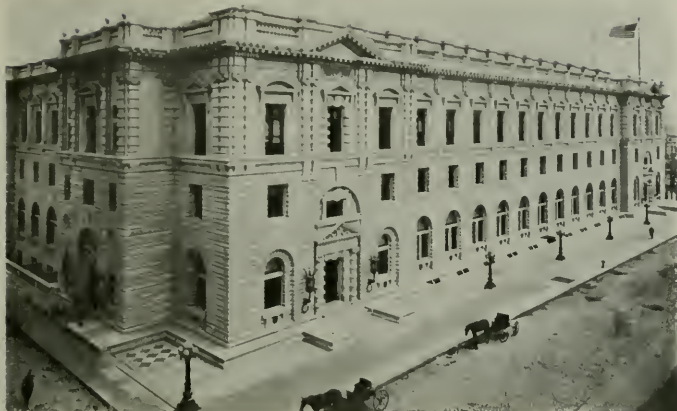
UNITED STATES POSTOFFICE AND COURT HOUSE, SAN FRANCISCO James Knox Taylor, Supervising Architect
