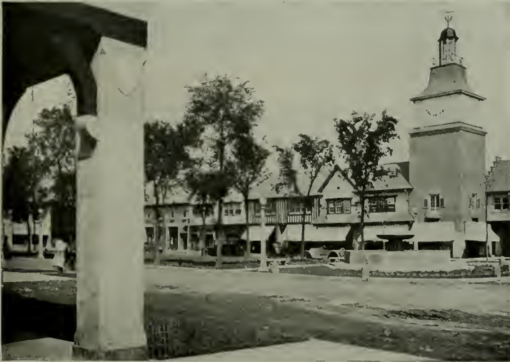
VIEW OF MARKET SQUARE, LAKE FOREST, ILL. Howard Shaw, Architect This shows how the tower relieves the whole design and with the corresponding tower across the Square, creates an imposing entrance
