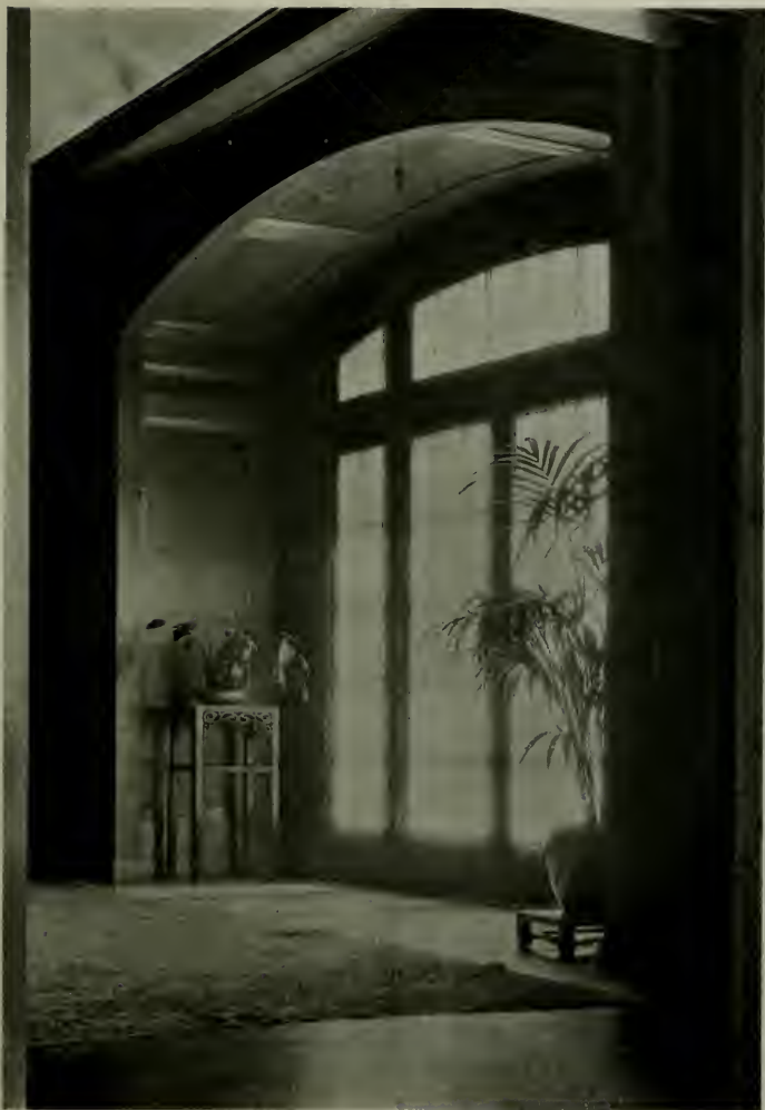
RESIDENCE OF MR. ABRAHAM ROSENBERG. ENTRANCE HALL
