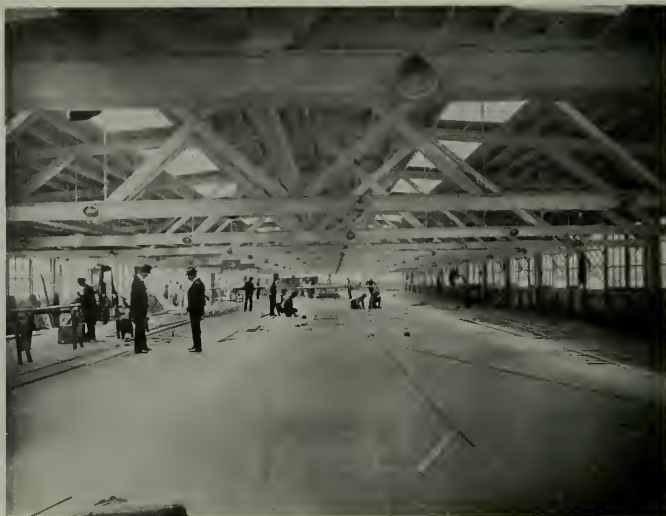
MOLDING LOFT, MOORE SHIPBUILDING WORKS, OAKLAND
