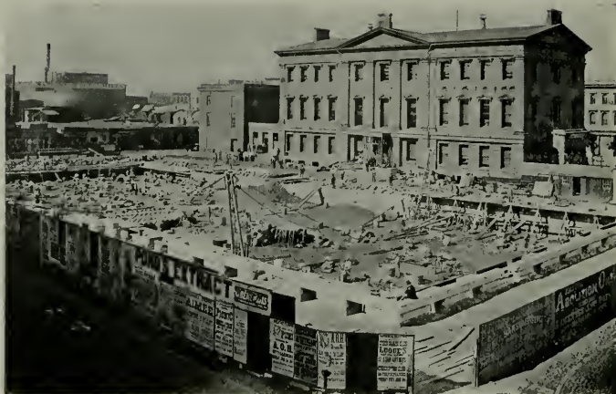
UNITED STATES APPRAISERS' BUILDING (IN COURSE OF CONSTRUCTION), JUNE 20, 1874
