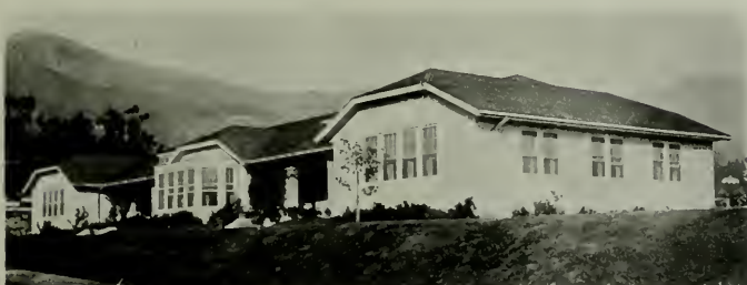
TYPICAL COTTAGE, SOUTHERN CALIFORNIA STATE HOSPITAL
