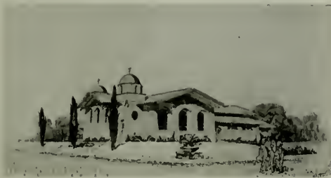
FIRST PRESBYTERIAN CHURCH, MADERA H. M. Patterson, Architect
