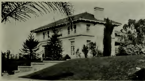
A ROOF OF CALIFORNIA MISSION TILE
