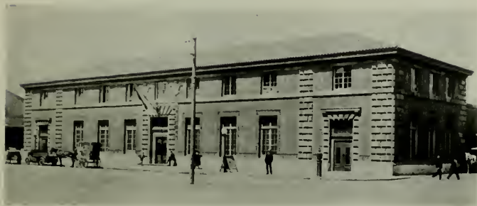
FERRY POST OFFICE BUILDING, SAN FRANCISCO
