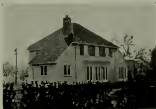
MANOR HOUSE, MENDOCINO STATE HOSPITAL
