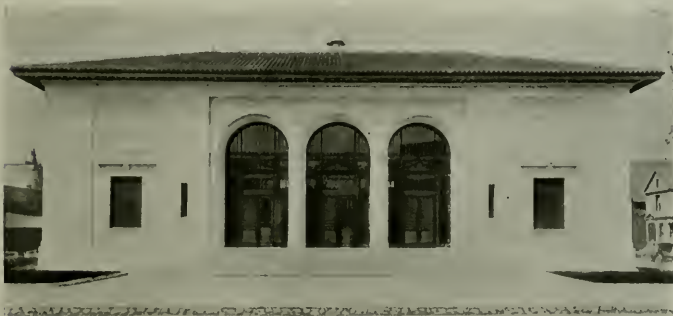
UNITED STATES POSTOFFICE, ALAMEDA, CALIFORNIA Oscar Wenderoth, Supervising Architect
