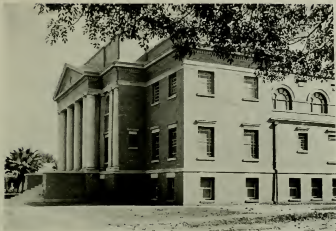
CENTRAL CHRISTIAN CHURCH, PHOENIX, ARIZONA Robert H. Orr, Architect
