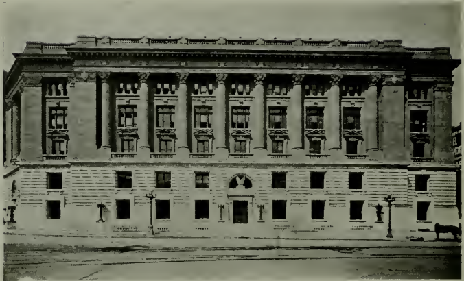
UNITED STATES POSTOFFICE, COURT HOUSE AND CUSTOM HOUSE, LOS ANGELES James Knox Taylor, Supervising Architect
