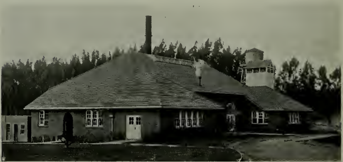
POWER HOUSE, NORWALK STATE HOSPITAL
