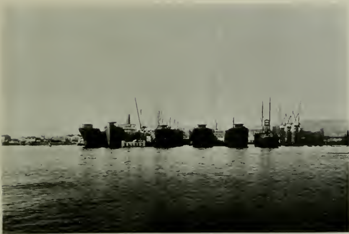
HULLS AT FITTING-UP BERTHS, AWAITING MACHINERY MOORE SHIPBUILDING WORKS, OAKLAND
