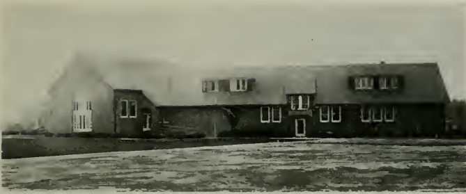
KITCHEN BUILDING, NORWALK STATE HOSPITAL
