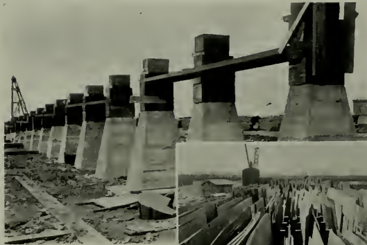
Concrete bases for shipway. This is one of only three yards in the world so equipped.
