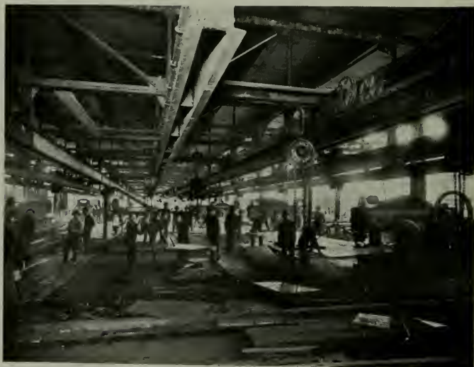
INTERIOR PUNCH SHED, MOORE SHIPBUILDING WORKS, OAKLAND Leland S. Rosener, C. E.
