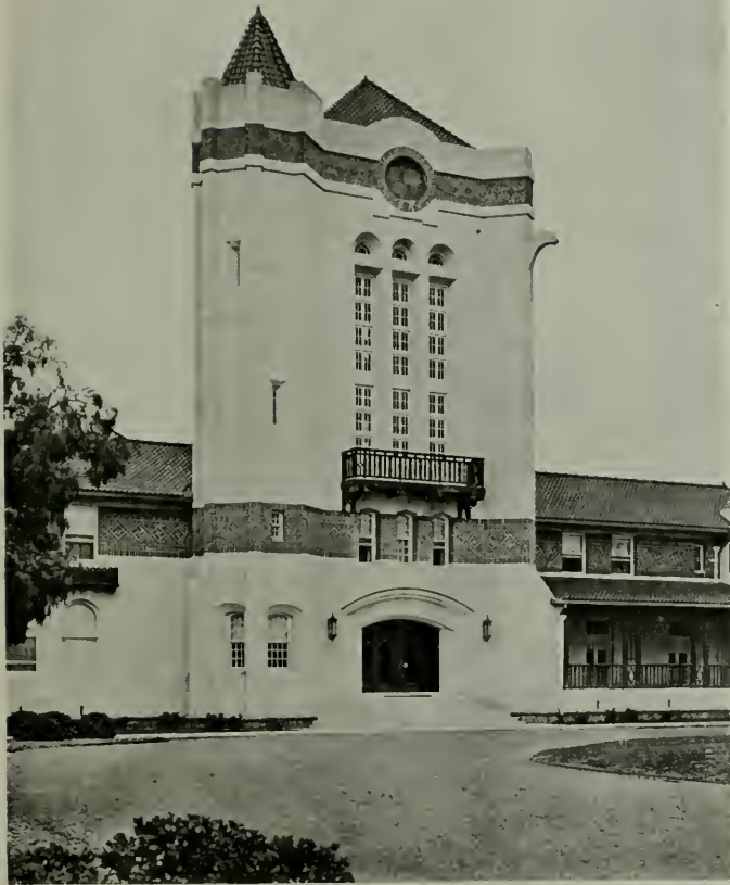
TOWER, AGNEW STATE HOSPITAL
