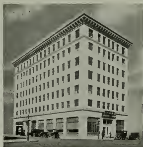
Citizens Savings Bank Building, Pasadena Parkinson & Bergstrom, Architects The banking rooms of this modern bank and office building are equipped with
