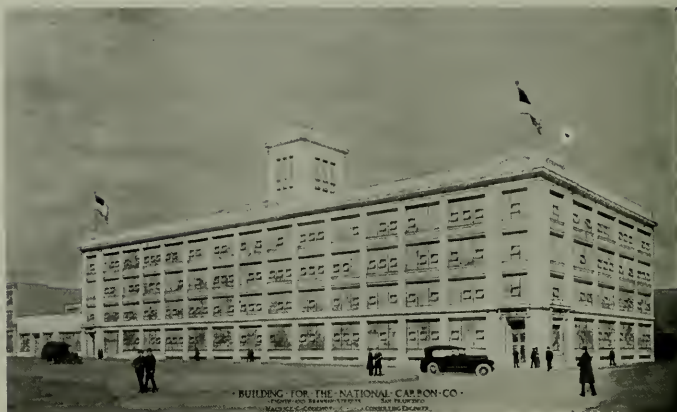
BUILDING FOR THE NATIONAL CARBON CO., SAN FRANCISCO
