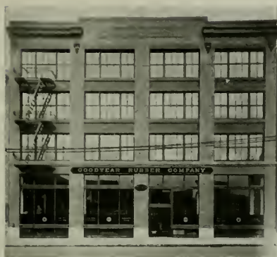
BUILDING FOR GOODYEAR RUBBER COMPANY, SAN FRANCISCO, A. M. MILWAIN, ARCHITECT
