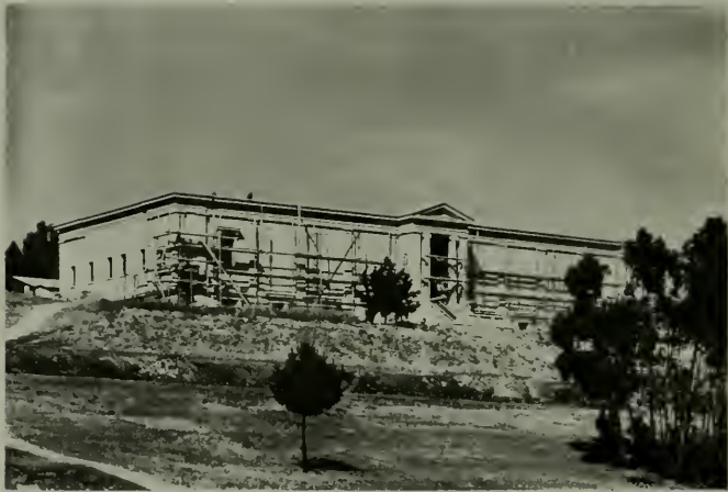
PROGRESS PICTURE, EVERGREEN MAUSOLEUM Haven-court, Oakland B. J. S. Cahill, Architect
