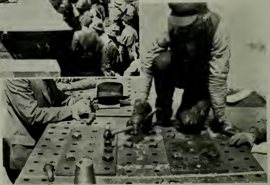
Laying first keel, less than four months after ground was broken for Pacific Coast Shipbuilding Plant, Hay Point.
