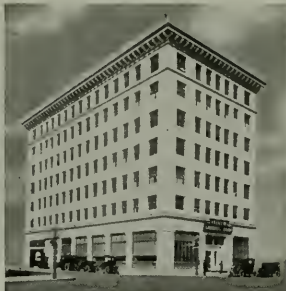
Citizens Savings Bank Building, Pasadena Parkinson & Bergstrom, Architects The banking rooms of this modern bank and office building are equipped with
