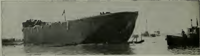
The Concrete Ship "Faith." Length, 336 feet. Beam, 44 feet. Capacity 5,000 tons. San Francisco Shipbuilding Co., Builders
