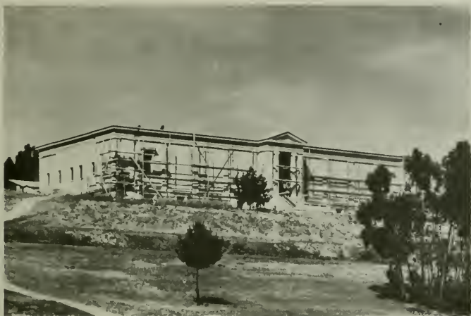
PROGRESS PICTURE, EVERGREEN MAUSOLEUM
