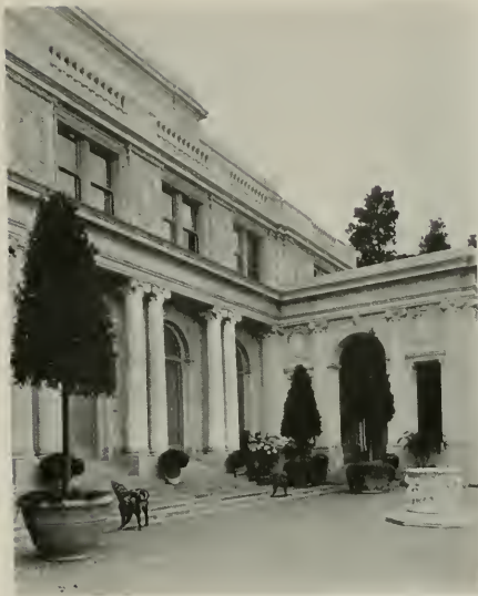
COURT, COUNTRY HOUSE OF MR. TEMPLETON CROCKER, HILLSBOROUGH. Willis Polk & Co., Architects.
