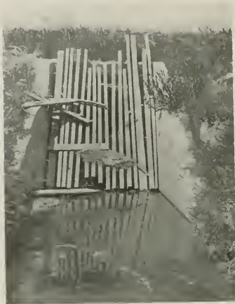
FIG. 7.—Wooden grating for catching debris. Automatic Drainage Gate, Ralph Bull ranch, near Arcata, California, on Humboldt Bay.
