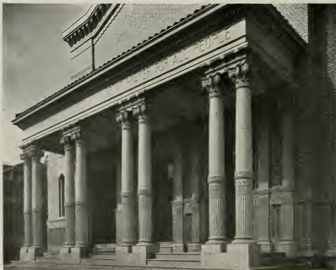
COLONNADE, SYNAGOGUE FOR FIRST HEBREW CONGREGATION, OAKLAND G. Albert Lansburgh, Architect
