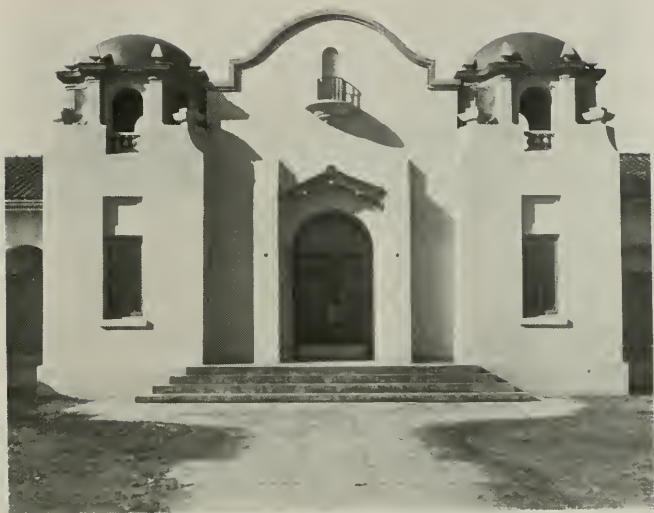
DETAIL OF ENTRANCE, CARRUTHERS UNION HIGH SCHOOL, Ernest J. Kump, Architect.
