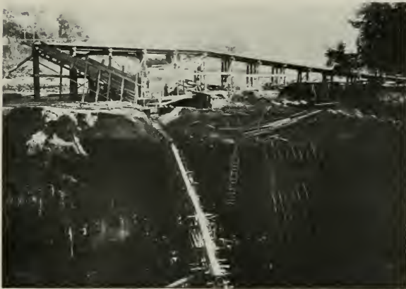
MATERIAL BUNKERS AND CONCRETE CHUTE, LAGUNA HONDA STATION, TWIN PEAKS TUNNEL.
