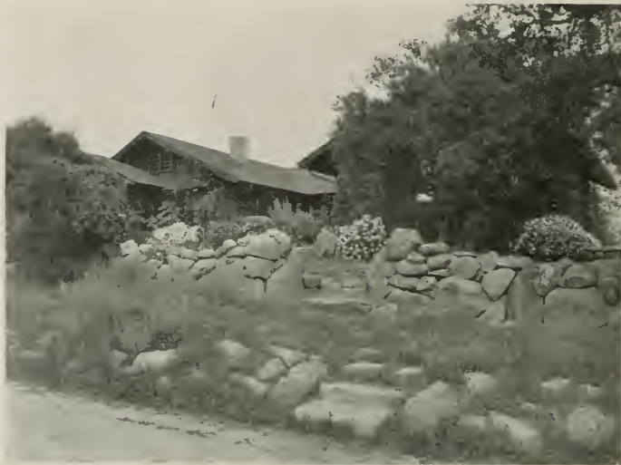
BUNGALOW OF MR. E. D. LIBBEY, NORDHOFF, CALIFORNIA Myron Hunt and Elmer Grey, Architects
