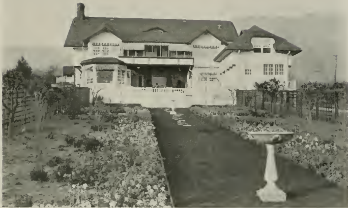
GARDEN FRONT, RESIDENCE OF MRS. E. M. NEUSTADT, ALTADENA Elmer Grey, Architect
