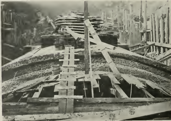
CONCRETE ARCH IN TUNNEL SECTION CONSTRUCTED IN OPEN CUT, SHOWING KEY AND ROUGHED SURFACE FORMING CONSTRUCTION.
