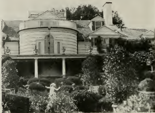
FIG. 1. Day view of the residence of J. L. Breese, showing the arrangement of the projector units on the roof of the porch for lighting this garden, and also in the foreground the two box lights for lighting the fountain.
