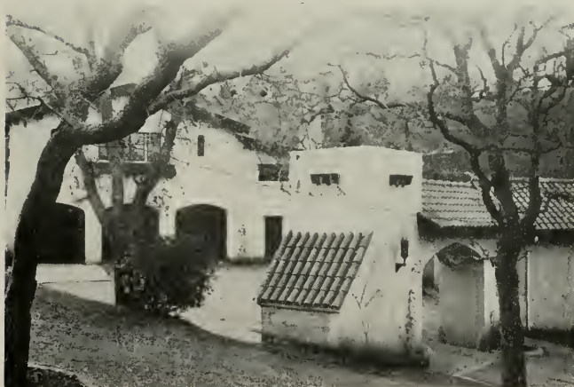
GARAGE COURT, W. B. WELLMAN RESIDENCE, LOS ALTOS Henry C. Smith, Architect
