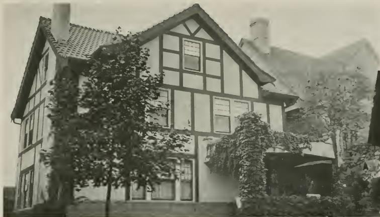
Handsome Residence with Stucco Exterior Finish on a Base of Armco Iron Lath
