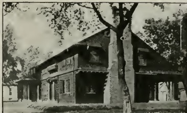
Stained with Cabot's Creosote Stains (burglar-brown walls, moss-green roof). Clinton P. Shockley, Architect, Waterloo, Ia.
