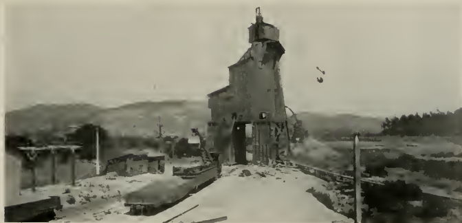
GENERAL VIEW OF PLANT AND GRAVEL DEPOSITS
