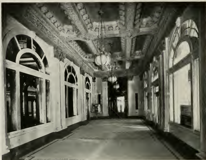
ENTRANCE LOBBY, STANDARD OIL BUILDING, SAN FRANCISCO Benj. G. McDougall, Architect
