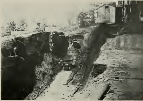
OPEN CUT EXCAVATION FOR SUBWAY SECTION, TWIN PEAKS TUNNEL.
