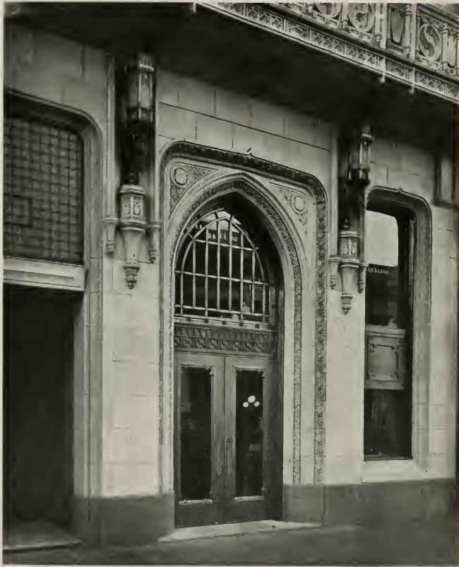
BROADWAY ENTRANCE, FEDERAL REALTY BUILDING, OAKLAND BENJ. G. McDOUGALL, ARCHITECT
