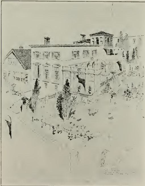
RESIDENCE DR. C. CAGLIERI Albert Farr, Architect
