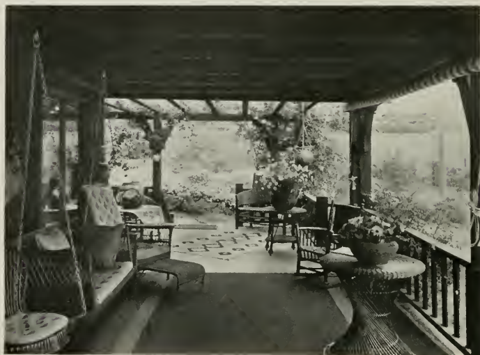
BUNGALOW OF MR. E. D. LIBBEY, NORDHOFF, CALIFORNIA Myron Hunt and Elmer Grey, Architects
