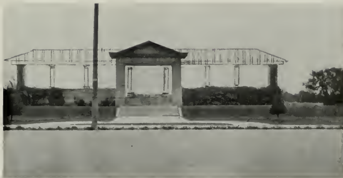
FRONT ELEVATION OF PRESENT STRUCTURE, MUNICIPAL PARK, FULLERTON, CAL.
