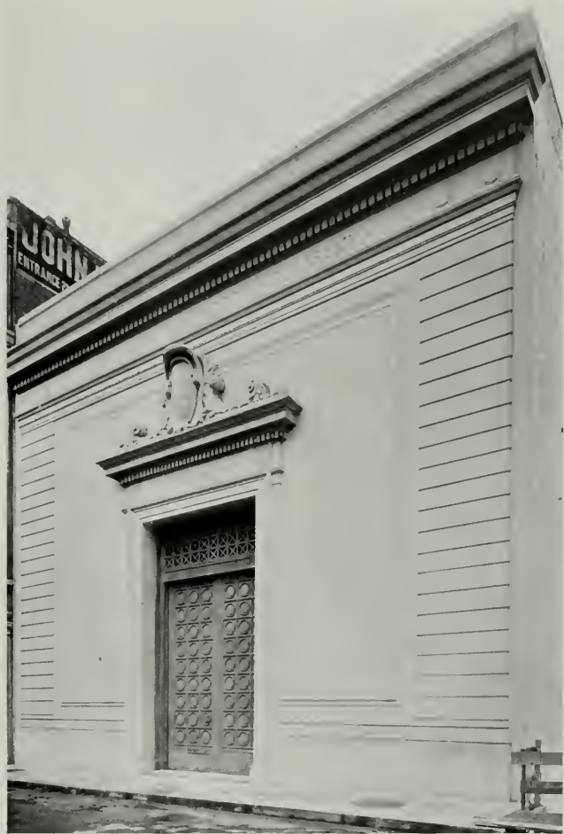
STATION "J," PACIFIC GAS & ELECTRIC COMPANY FREDERICK H. MEYER, ARCHITECT
