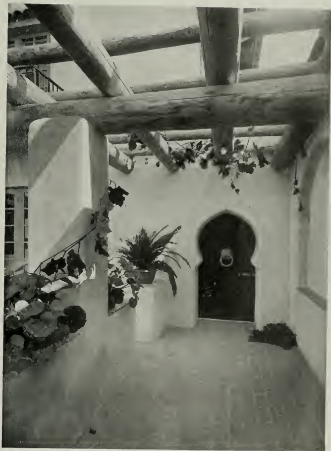
DOORWAY, HOUSE OF JUDGE A. H. SWEET, SAN DIEGO FRANK MEAD AND RICHARD S. REQUA, ARCHITECTS
