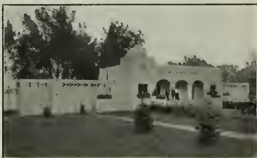
Berkeley Lake City and Denver County Bath House Stained with Cabot's Stucco Stains E. H. Moorman, Architect, Denver, Colo.
