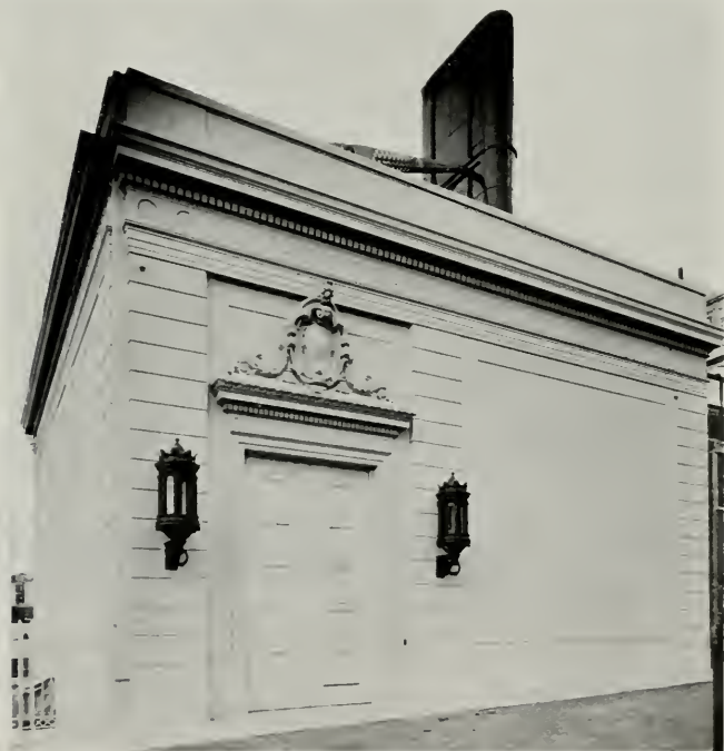
STATION "S," SAN FRANCISCO GAS & ELECTRIC CO. Frederick H. Meyer, Architect
