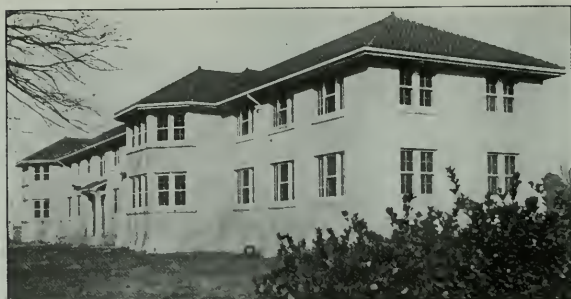
WARD 25, STOCKTON STATE HOSPITAL, STOCKTON, CALIFORNIA
