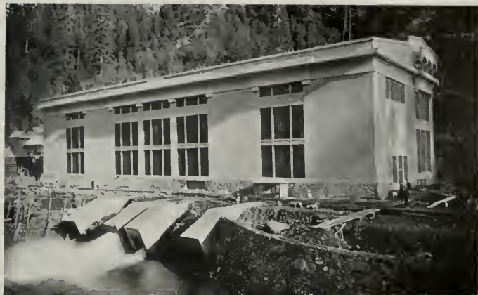
DRUM POWER HOUSE, HYDRO-ELECTRIC PLANT Designed by Ivan C. Frickstad
