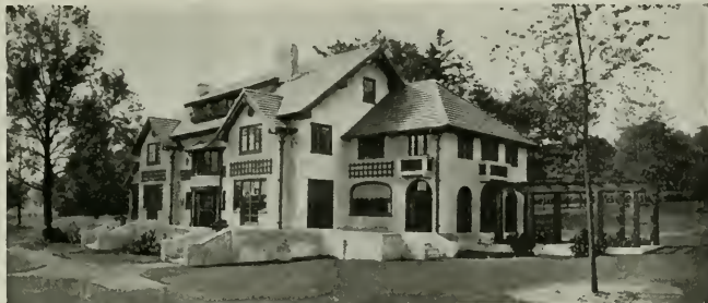
This Beautiful Home is finished in White Portland Cement.
