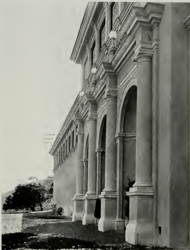
DETAIL OF FACADE. CORDELIA SUB-STATION DESIGNED BY IVAN C. FRICKSTAD H. C. VENSANO, ENGINEER
