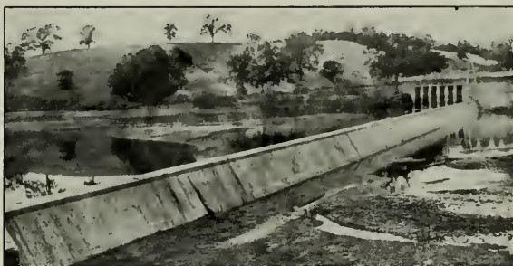
CAPAY DIVERTING DAM, YOLO WATER AND POWER COMPANY
