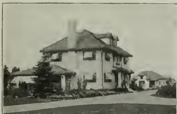
Residence at Wakefield, Mass., stained with Cabot's Cement Stains. H. A. Perkins, Architect, Boston.
