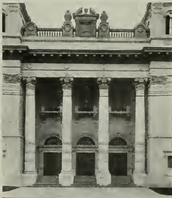
Detail of Entrance, First M. E. Church, Oakland, Norman F. Mersh, Architect. Columns are of Portland Stone.
