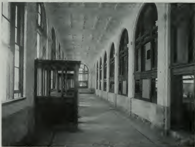
MAIN LOBBY. LOOKING EAST, POSTOFFICE BUILDING, BERKELEY
