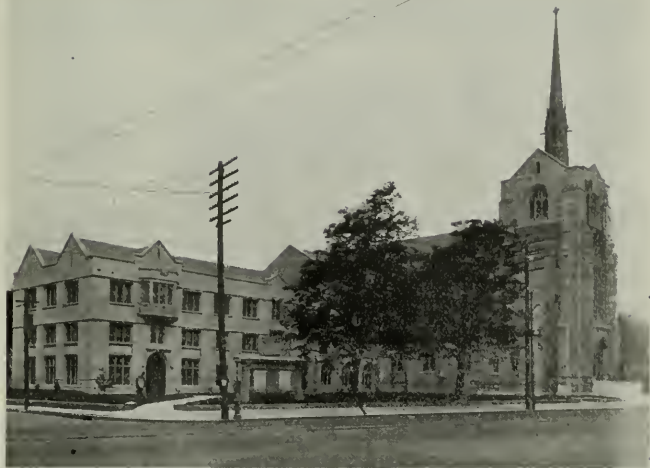
FIRST PRESBYTERIAN CHURCH, OAKLAND, CONSTRUCTED ENTIRELY OF PORTLAND STONE AND GRANITE W. C. Hays, Architect
