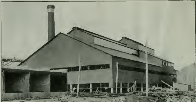
From a photograph of Atlantic Coast Lumber Co., Georgetown, S. C. This is the largest fire-proof lumber plant in the world and its roofing and side walls are Armco Iron
