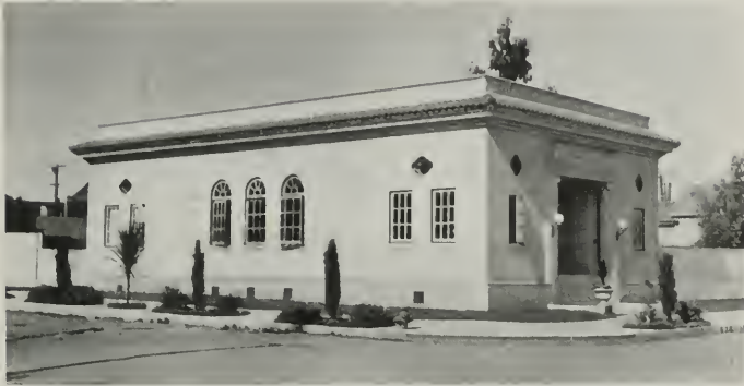
SAN MATEO SUB-STATION, SAN MATEO, CALIFORNIA Designed by Ivan C. Frickstad
