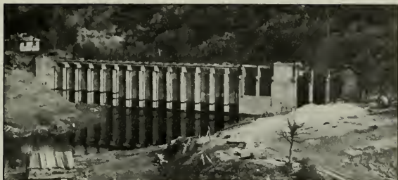
IMPOUNDING DAM, CACHE CREEK, AT OUTLET
