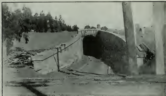
BELT LINE R.R. TUNNEL, WEST PORTAL, SAN FRANCISCO HARBOR FRONT
