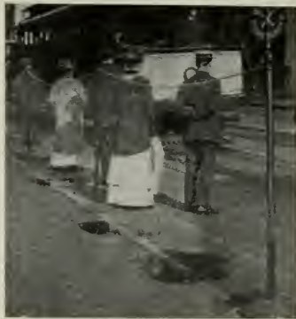
SAFETY ZONE for street car passengers, showing the lines D and E of the diagram and the posts, signs and chains to emphasize line E. A similar post with base and a semaphore, lettered "Stop-Stop," "Go-Go," stands by the traffic policeman near the center of the intersection, and signals the traffic to wait or to proceed, aided also by the policeman's whistle and arm in case of slow, impatient or inattentive drivers.
