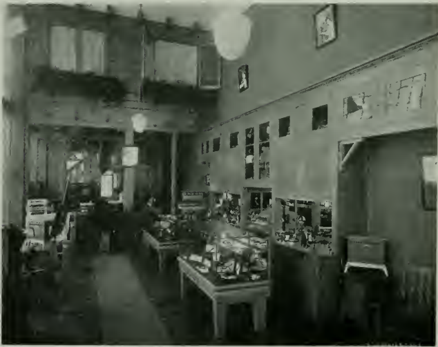
DISPLAY ROOM AND OFFICES, GENERAL ELECTRICAL CONSTRUCTION COMPANY
