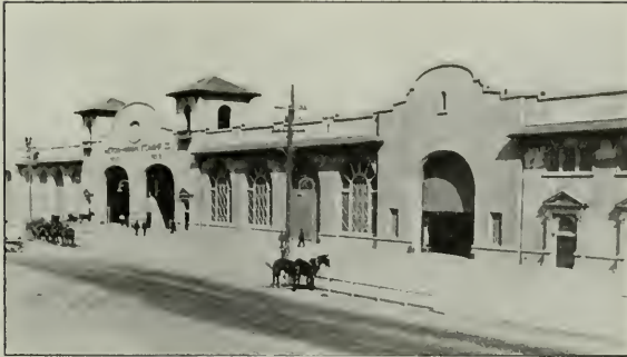
PIERS 30 AND 35, SAN FRANCISCO HARBOR FRONT
