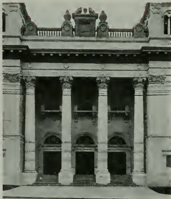
Detail of Entrance, First M. E. Church, Oakland, Norman F. Marsh, Architect. Columns are of Portland Stone.
