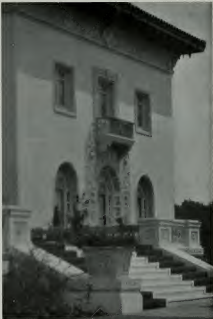
FRONT MOTIF, HOUSE OF MR. LOUIS SARONI, SAN FRANCISCO MACDONALD AND MACDONALD, ARCHITECTS
