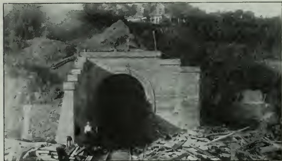
BELT LINE R.R. TUNNEL, EAST PORTAL, SAN FRANCISCO HARBOR FRONT
