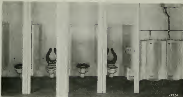
PHOTOGRAPH OF TOILET INSTALLATION IN STOCKTON SCHOOLS
