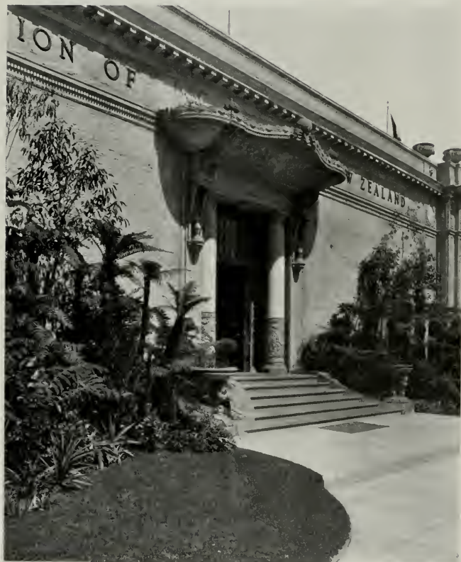
DETAIL OF ENTRANCE, BUILDING FOR THE DOMINION OF NEW ZEALAND LEWIS P. HOBART, ARCHITECT
