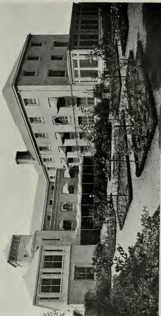
GARDEN ELEVATION, RED CROSS HOSPITAL, SAN MATEO, CALIFORNIA LEWIS P. HOBART, ARCHITECT
