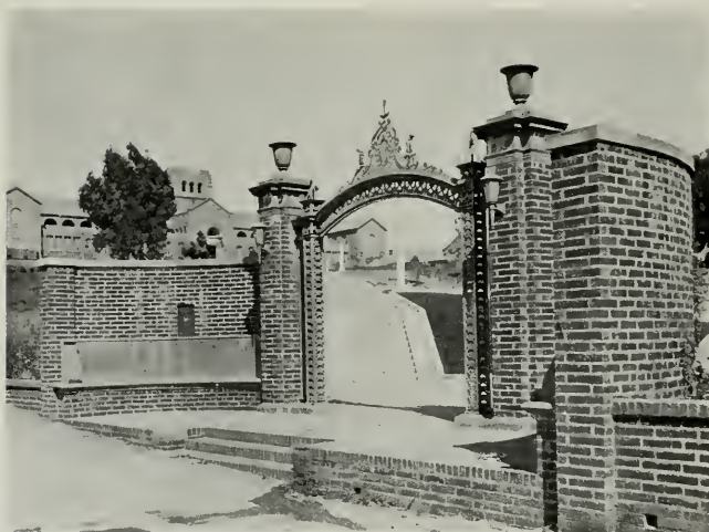
FAWTER MEMORIAL GATE, HIGH SCHOOL GROUP, SANTA MONICA Allison & Allison, Architects
