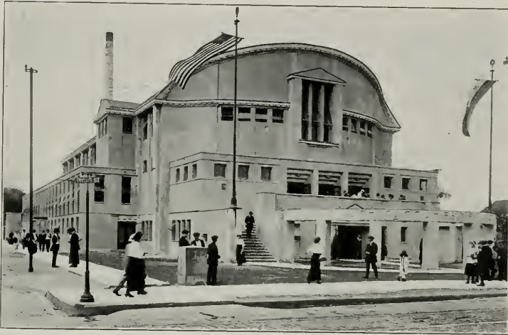
TAYLOR STREET FRONT OF CHICAGO HEBREW INSTITUTE Ottenheimer, Stern & Reichert, Architects
