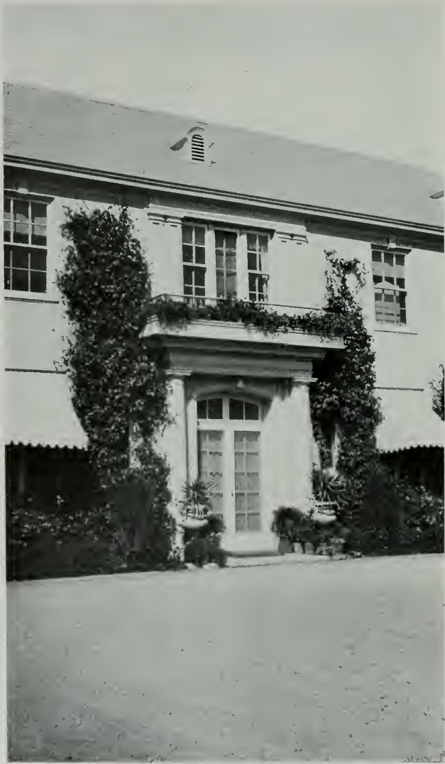
ENTRANCE DETAIL, HOUSE OF THOS. DRISCOLL, ESQ. LEWIS P. HOBART, ARCHITECT
