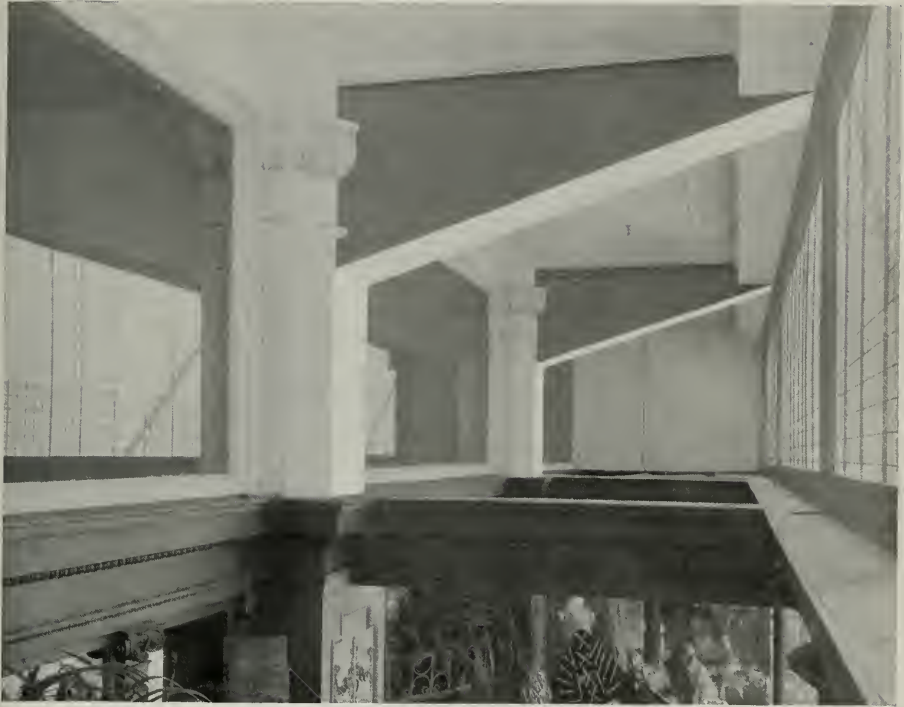
Fig. 11—SHOWING CANTILEVER CONSTRUCTION, HALE BROS.' DEPARTMENT STORE
