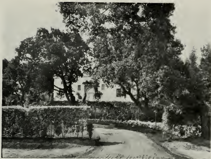
HOUSE, DR. W. C. CHIDESTER, SAN MATEO, CALIFORNIA Lewis P. Hobart, Architect
