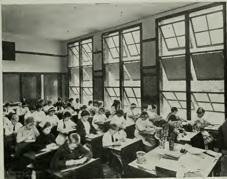
Typical interior of class rooms showing SIMPLEX WINDOWS
