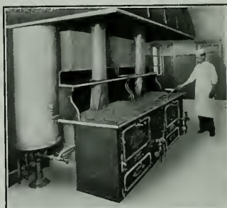
Cruze Oil Burners Operating Kitchen Ranges in Government Barracks at Fort Winfield Scott
