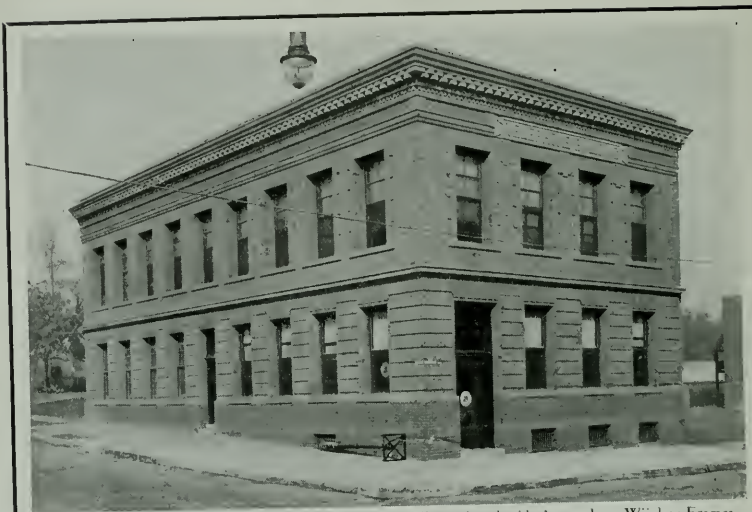
A Telephone Building of the Bell System at Galesburg, Ill., equipped with Armco Iron Window Frames
