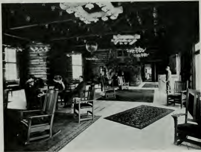
INTERIOR, PEBBLE BEACH LODGE, MONTEREY, CALIFORNIA Lewis P. Hobart, Architect
