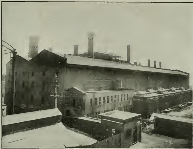
Station A, Pacific Gas & Electric Company, San Francisco
