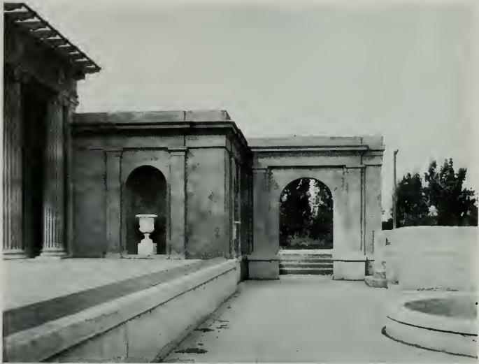
OPEN AIR THEATER, BAKERSFIELD, CALIFORNIA Lewis P. Hobart, Architect
