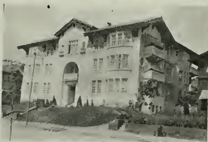
CHANNING APARTMENTS Berkeley W. H. Ratcliff, Jr., Architect
