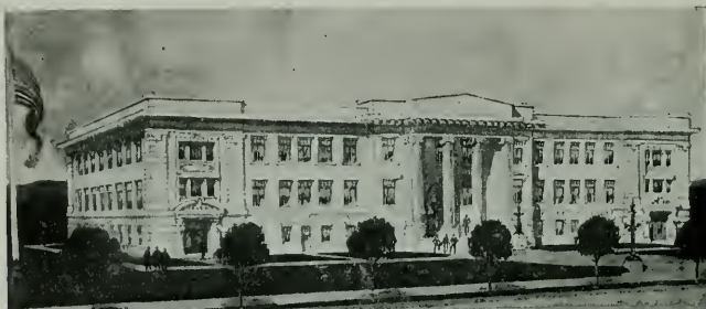
TOPLIGHT SHADES USED IN THE ARMIJO UNION HIGH SCHOOL, FAIRFIELD, CAL., HENRY C. SMITH, Architect.
