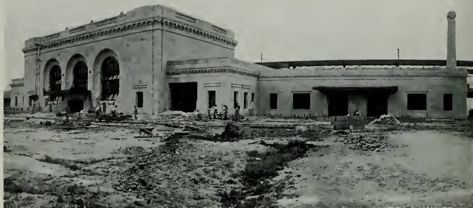
SOUTHERN PACIFIC RAILROAD STATION, OAKLAND, CALIFORNIA
