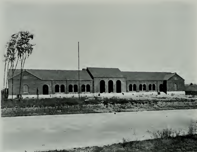
FREMONT AVENUE SCHOOL, ALHAMBRA Allison & Allison, Architects
