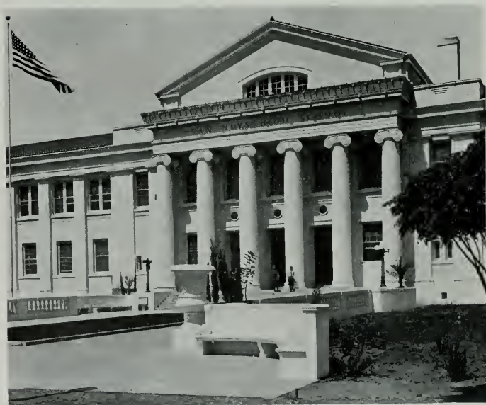
DETAIL, MAIN BUILDING, VAN NUYS HIGH SCHOOL Allison & Allison, Architects
