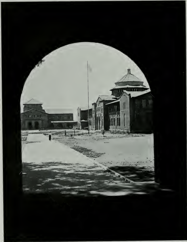
VIEW FROM TRAINING SCHOOL, LOS ANGELES STATE NORMAL GROUP ALLISON & ALLISON ARCHITECTS W. F. McCLURE, STATE ENGINEER
