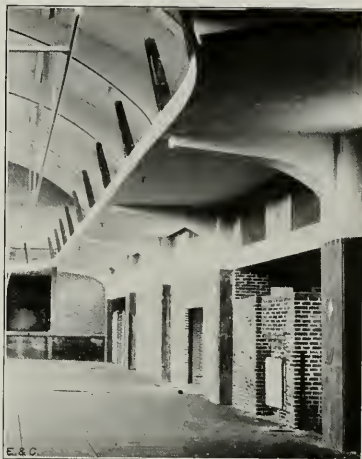
FIG. 8—INTERIOR VIEW OF PORTION OF MAIN GYMNASIUM OF CHICAGO HEBREW INSTITUTE
