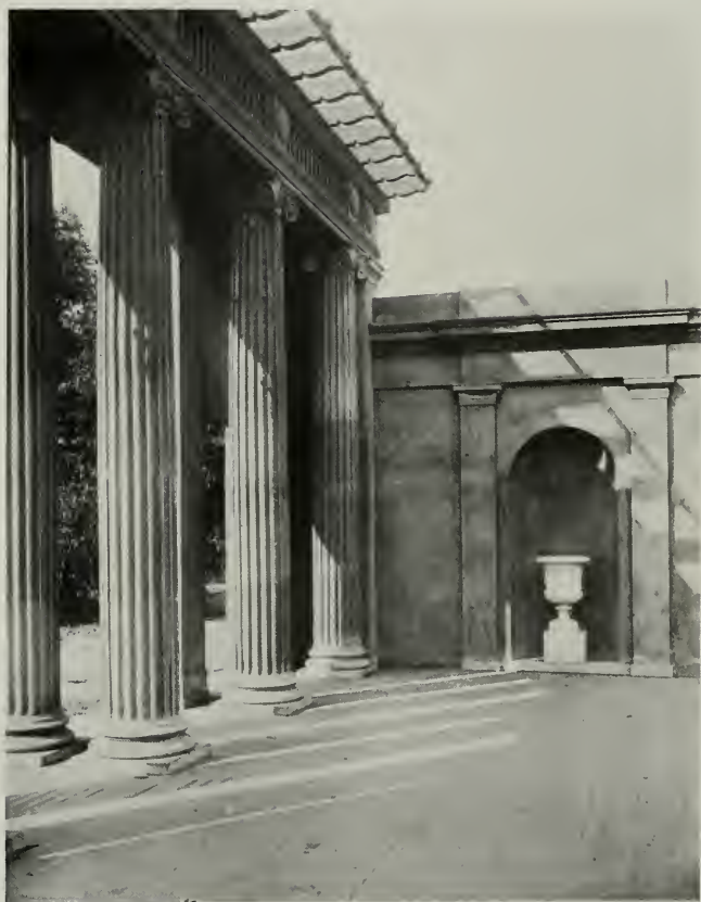
OPEN AIR THEATER, BAKERSFIELD, CALIFORNIA LEWIS P. HOBART, ARCHITECT
