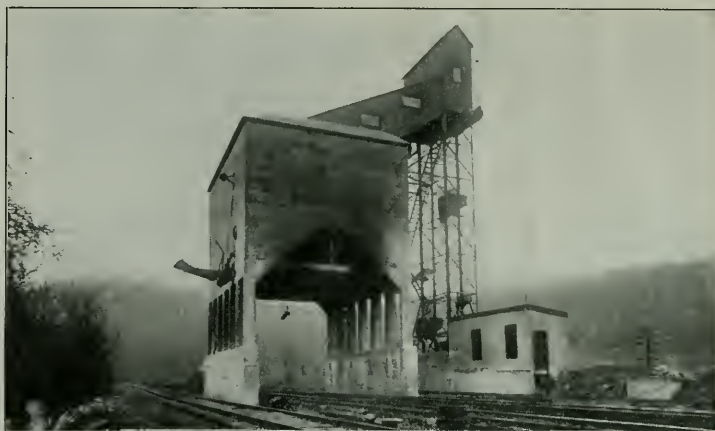
Locomotive Coaling Plant at Sir John's Run, W. Va. Designed and built for the B. & O. Railroad by The Roberts & Schaefer Co., Chicago. Armco Iron Roofing and Siding used.
