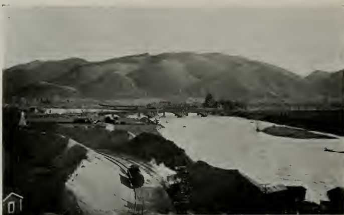
(Fig. C)—Storage piles of rock, sand and gravel
