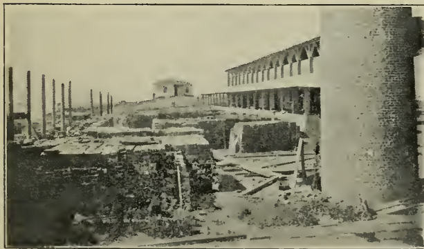
PAVING AND RED PRESSED BRICK AT VALLEJO BRICK & TILE CO.'S VALLEJO YARD
