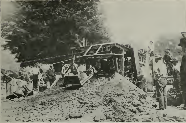
THE YOUNGER EXCAVATOR IN OPERATION
