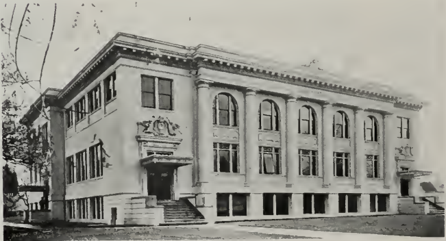
SANTA ROSA HIGH SCHOOL Wm. H. Weeks, Architect
