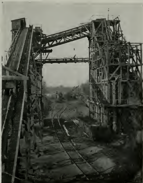
(Fig. A)—View of plant, showing belt-conveyor and storage bins
