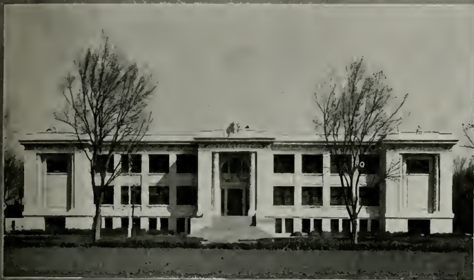
THE WOODLAND HIGH SCHOOL, W. H. Weeks, architect, is equipped by us with
