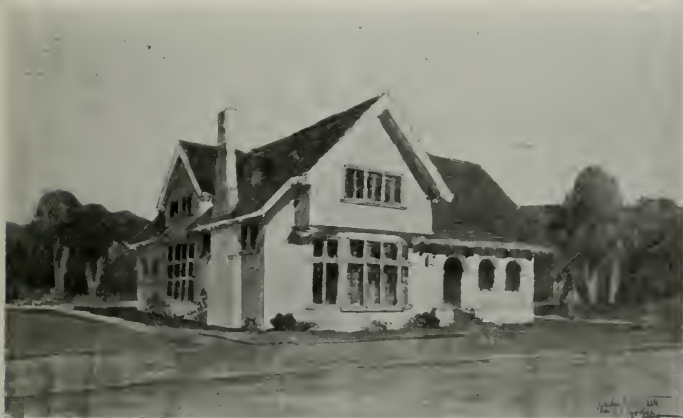
HOUSE FOR MR. GEORGE A. MOORE, ROSS, CALIFORNIA W. Garden Mitchell and Charles E. Hodges, Architects
