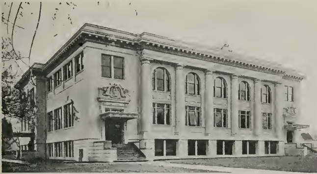
SANTA ROSA HIGH SCHOOL, SANTA ROSA CALIFORNIA MR. WILLIAM H. WEEKS, Architect
