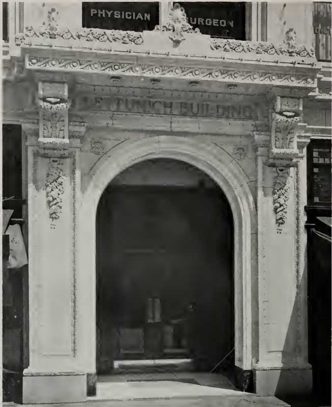
ENTRANCE, LETTUNICH BUILDING, WATSONVILLE Wm. H. Weeks, Architect
