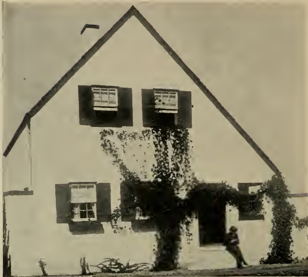
CONCRETE COTTAGE WITH 8-IN. WALLS BUILT AT A COST OF $2,700
