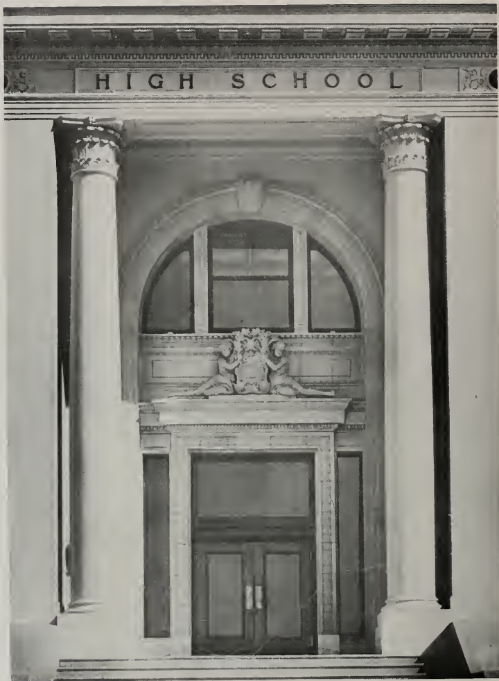
DETAIL OF ENTRANCE, WOODLAND HIGH SCHOOL WILLIAM H. WEEKS, ARCHITECT
