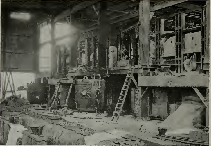
CASTING SIDE OF MOULDING ROOM, PACIFIC COAST STEEL COMPANY
