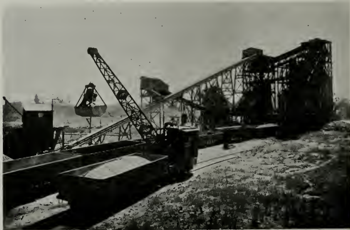
(Fig. D)—Port of plant of Niles Sand, Gravel & Rock Company, showing bunkers, loading facilities and locomotive crane in operation
