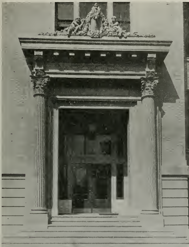
Detail of Entrance, Willows High School
