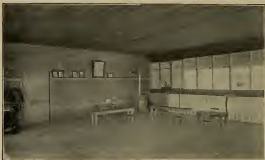
INTERIOR—PASADENA OPEN-AIR CLASS ROOM Elmer Grey, Architect
