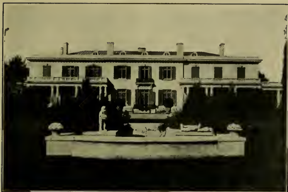
RESIDENCE, BURLINGAME, CALIFORNIA Louis P. Hobart, Architect
