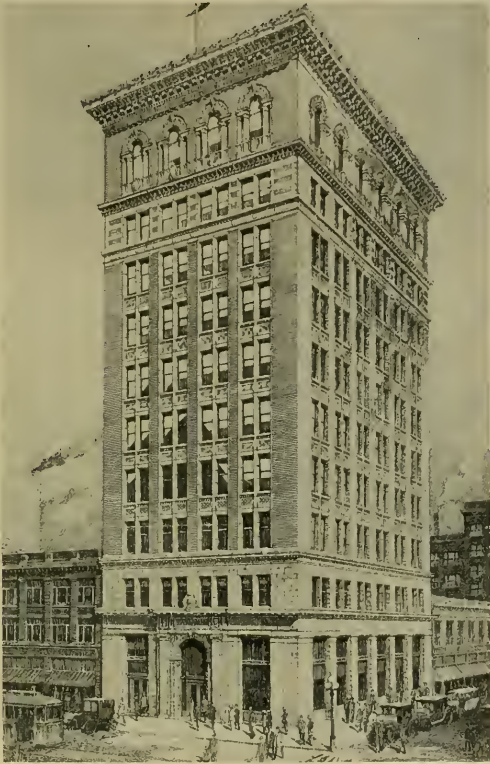
COMMERCIAL & SAVINGS BANK BLDG., STOCKTON, CALIFORNIA L. B. Dutton, Architect Stone & Wright, Associate Architects P. J. Walker, Builder
