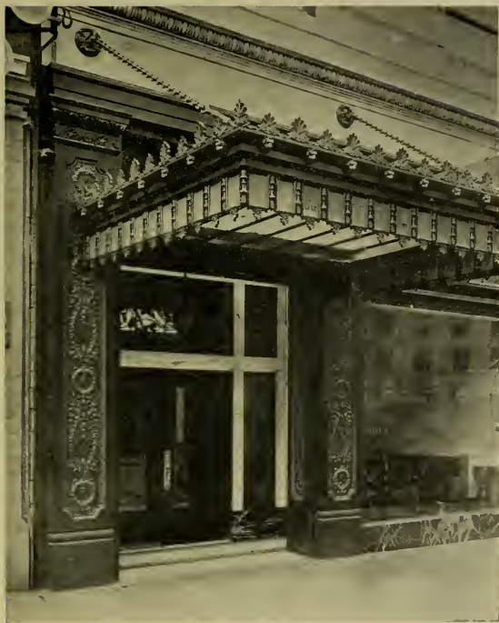
CAST IRON ENTRANCE AND MARQUISE TO HOTEL GLENN, SAN FRANCISCO WILLIAM H. WEEKS, ARCHITECT
