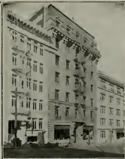
HOTEL WELLINGTON, San Francisco, Cal. Frederick Boese, Architect
