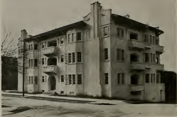
GLEN GARRY APARTMENTS, BERKELEY W. H. RATCLIFF, JR., Architect
