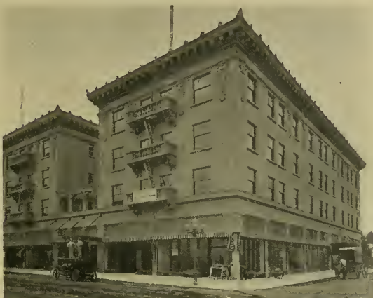
MONTGOMERY HOTEL, SAN JOSE, CAL., WILLIAM BINDER, ARCHITECT
