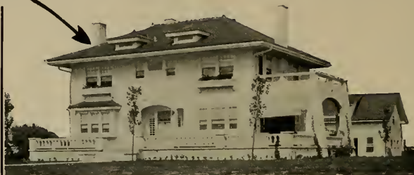
STUCCO HOUSE AND TILE ROOF
