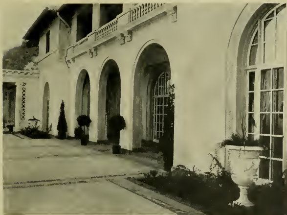
FACADE, COUNTRY HOUSE OF HON. JAS. D. PHELAN William Curlett & Son and C. E. Gottschalk, Architects Golden Gate cement used exclusively
