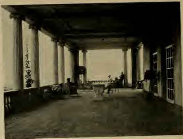
TILED PORCH, COUNTRY HOUSE OF HON. JAS. D. PHELAN William Curlett & Son and C. E. Gottschalk, Architects
