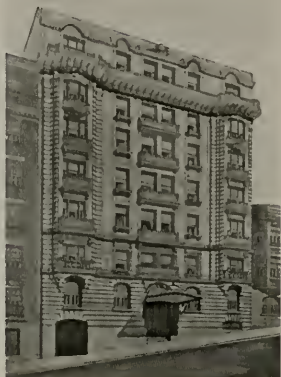
APARTMENT HOUSE FOR A. W. WILSON AND J. MARTIN, NOB HILL, SAN FRANCISCO.
