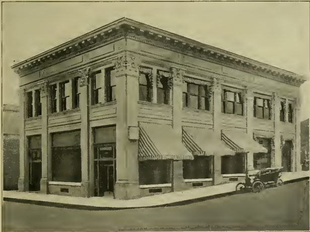
STATE BANK BUILDING, SAN PEDRO Edelman & Barnett, Architects
