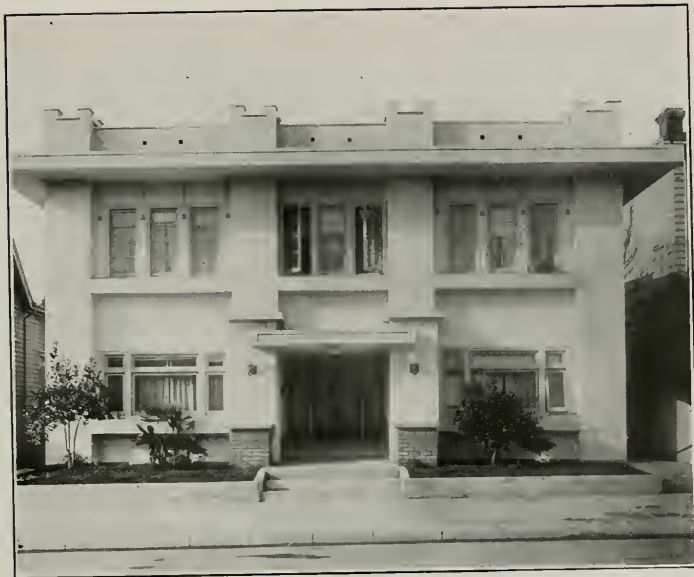
WOLFE APARTMENTS, SAN JOSE, CALIFORNIA
