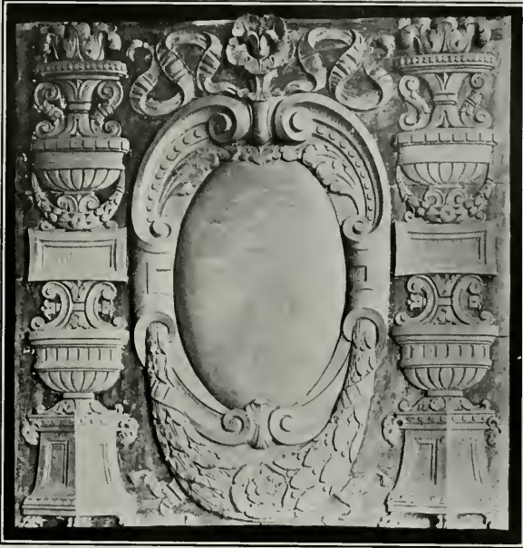
TERRA COTTA DETAIL, NORTHWESTERN BANK BUILDING, PORTLAND, OREGON
