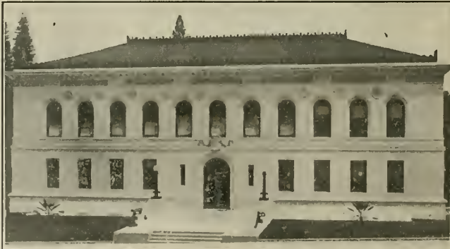
ELDORADO COUNTY COURT HOUSE, PLACERVILLE, CALIFORNIA
