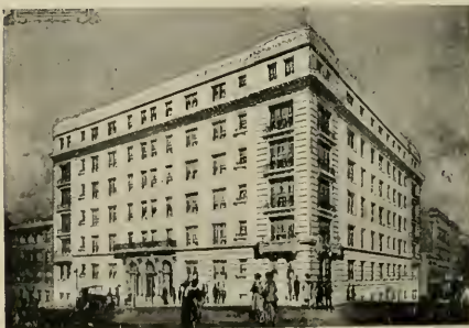
SMEIDELL APARTMENTS, SAN FRANCISCO Frederick H. Meyer, Architect
