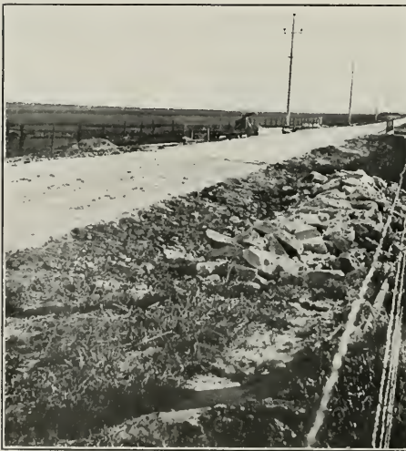
STATE ROAD NEAR LINCOLN Flood waters caused destruction
