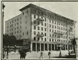
Temporary City Hall, San Francisco Wright, Rushford & Cahill, Architects
