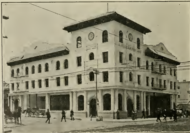
MISSION SAVINGS BANK BLDG., SAN FRANCISCO. Crim & Scott, Architects. EQUIPPED WITH
