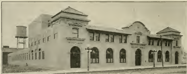
SUNSET PUBLISHING CO., SAN FRANCISCO (HY-RIB Exterior Walls)
