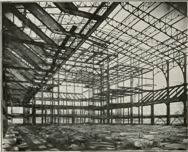
Fig. 8.—A CLOSE VIEW OF STRUCTURAL STEEL WORK
