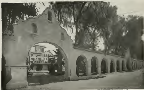
Fig. 9.—GLENWOOD INN, RIVERSIDE CAL.. LOOKING FROM THE STREET INTO THE COURTYARD
