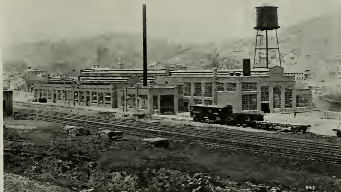
FIREPROOF MANUFACTURING PLANT OF THE GURNEY ELECTRIC ELEVATOR COMPANY
