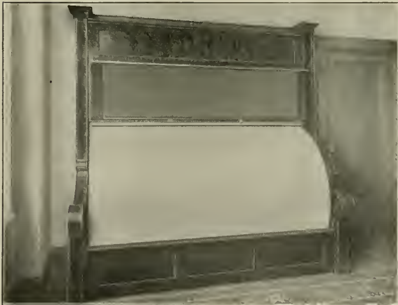
REVOLVING WALL TURNED INSIDE, LEAVING OCCUPANT IN OPEN AIR, AS SHOWN IN FOLLOWING ILLUSTRATION
