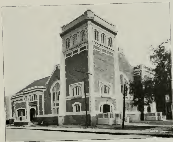
Fig. 24.—CONCRETE BLOCKS IN THE CONSTRUCTION OF THE NORMAL PARK METHODIST CHURCH, CHICAGO
