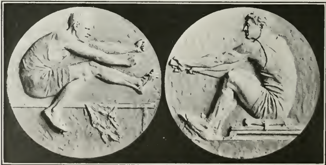
TERRA COTTA DETAIL, LOS ANGELES ATHLETIC CLUB BUILDING Parkinson & Bergstrom, Architects
