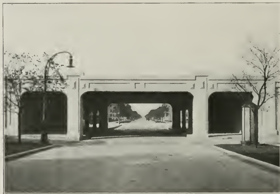
Fig. 18.—SACRAMENTO BOULEVARD VIADUCT, BALTIMORE AND OHIO RAILROAD, CHICAGO
