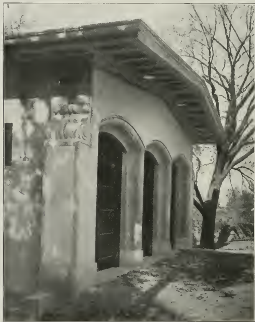
Fig. 6.—WESTERN FIRE STATION, WESTON, MASS.
