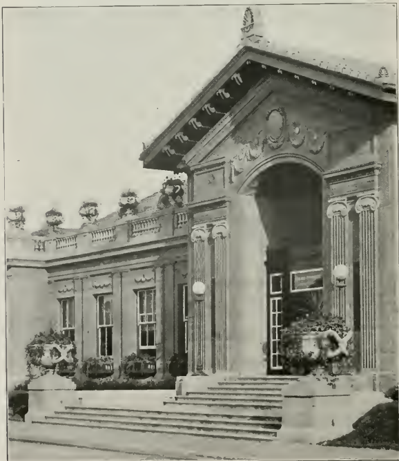
Fig. 4.—ENTRANCE DETAIL. ADMINISTRATION BUILDING, WASHINGTON PARK, CHICAGO
