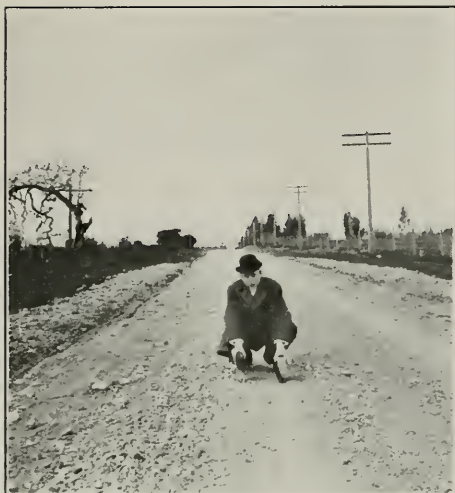
STATE ROAD NEAR HEALDSBURG Concrete torn up for about 700 feet—too thin. Photo taken March 1, 1914
