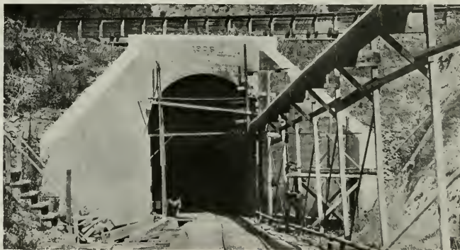
WESTERN PACIFIC RAILWAY TUNNEL PORTAL AND LINING
