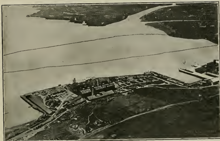
AEROPLANE VIEW OF STEIGER TERRA COTTA & POTTERY WORKS SOUTH SAN FRANCISCO
