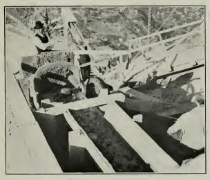
Belt Conveyor Discharging Wet Concrete-Speed 400 Feet Per Minute
