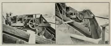
Belt Conveyor at Rest, Showing Wet Concrete on Belt
