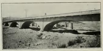
Reinforced Concrete Bridge, Niles, Col., 110-Foot Arches, with 18-Inch Concrete Slabs
