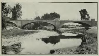
Concrete Bridge on the San Jose-Oakland Road Over Coyote Creek. Three 70-Foot Spans J. G. McMillan, Engineer
