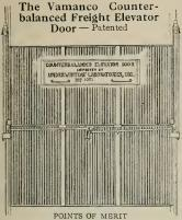
Obtains the lowest possible rate of insurance. Occupies but 3 inches in the shalt. Acts as a gate and fireproof door combined. All parts are in plain view at all times. Any ordinary mechanic can repair it. Its construction makes it easy to operate, it is not expensive. Insures a closed shaft at all times. No strings to break or get out of order. It is absolutely freproof. Manufactured by
