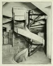
Showing Fire-door and Smoke Baffle under ceiling,
