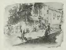
No. 6A Mixer with Gravity Distributing Chute on paving work at Chico, California.
