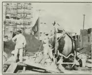
Foote Batch Mixer with Power Loading Skip, on building construction Lange & Bergstrom, Contractors.
