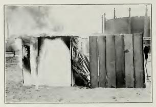
Fig. 2, Showing Fall of Unpainted Wall Against Pointed One
