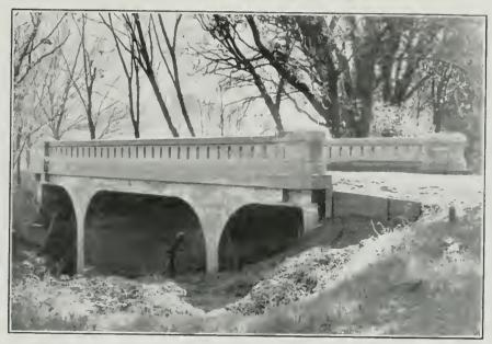
Reinforce Concrete Flat Slab Bridge, City of Ress, Morin Colony, California
