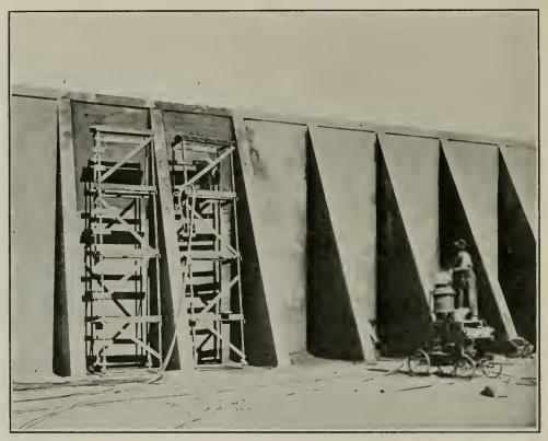
Cement Gun at Work on Twin Peaks Reservoir
