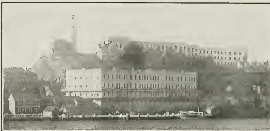
U. S. Government Buildings, Alcatraz Island, San Francisco Bay
