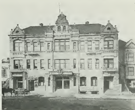
TURN-VEREIN BUILDING, SAN FRANCISCO, CAL. Foundations and Swimming Pool Waterproofed with CERESIT
