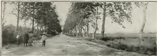
Oakland Road, California. Richmond Road Oil used as a binder.
