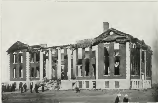
The Same Building After a Fire on February 4. Absence of Fireproof Floors was Responsible for the Extensive Damage. A few Thousand Dollars Spent for Concrete or Hollow Tile Fireproofing Would Have Confined the Fire to at Least One Floor, if not to a Single Room.
