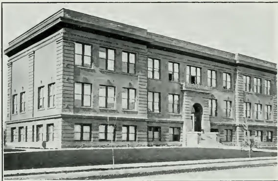
Santa Clara High School Building
