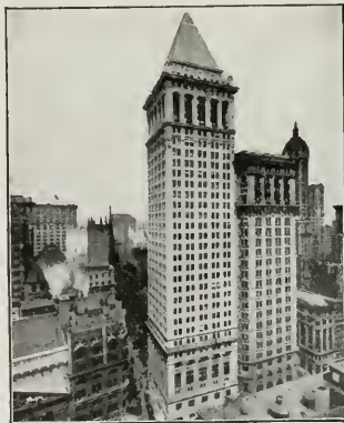
BANKERS TRUST CO. BLDG., NEW YORK Trowbridge & Livingston, Architects Marc Eiditz & Sons, Contractors
