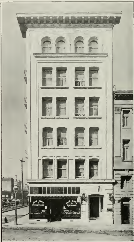
WILSON BUILDING, SAN FRANCISCO
