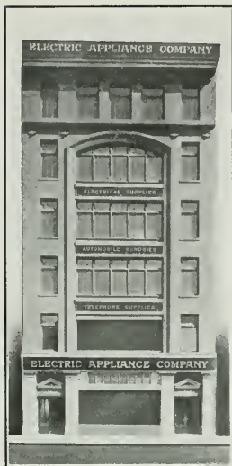
New Home of Electric Appliance Company
