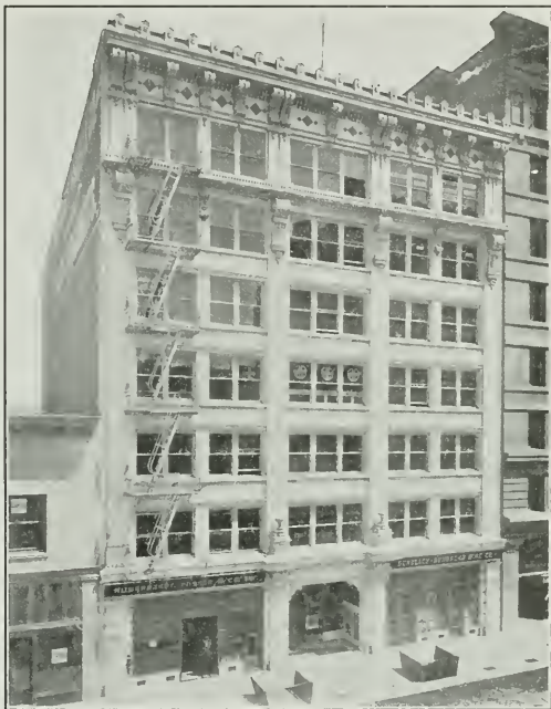
MARVIN BUILDING, SAN FRANCISCO, C. A. MEUSSDORFFER, ARCHITECT
