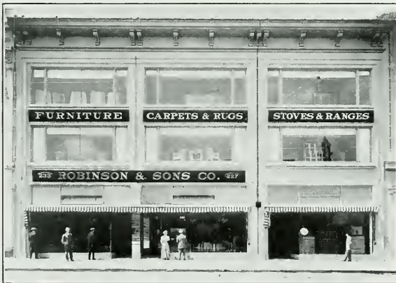
Robinson-Binder Building, San Jose
