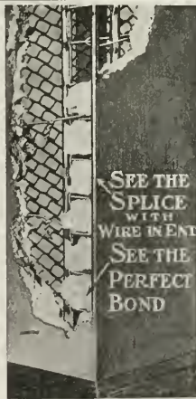
A Corner in Plaster.
