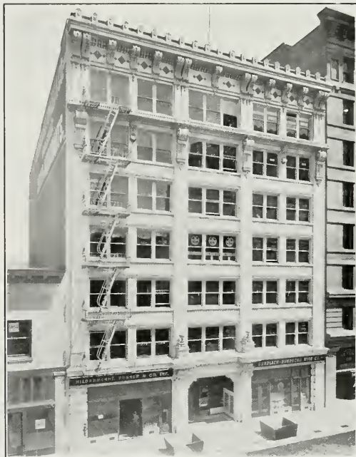
Merchants' Trust Building, San Francisco C. L. Vennard, Architect
