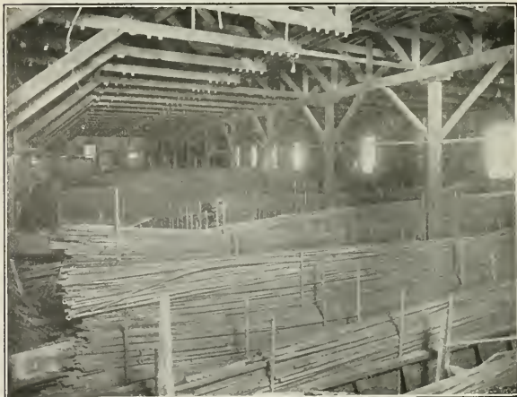
This Photograph shows over 1500 Tons of Reinforcing Steel in Woods & Huddart's Warehouse
