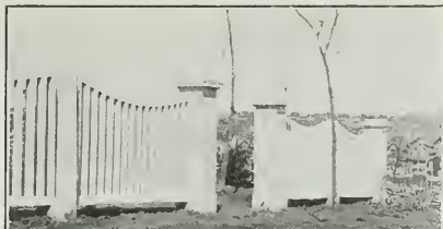
Upper Cut Shows Concrete Fence
