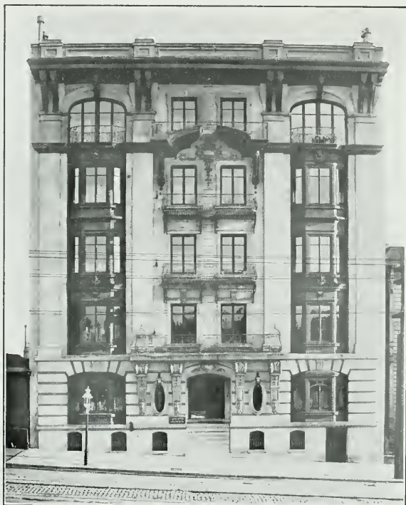
The Lafayette Apartments, San Francisco, Nat. C. Goodwin, Owner C. A. Meussdorffer, Architect
