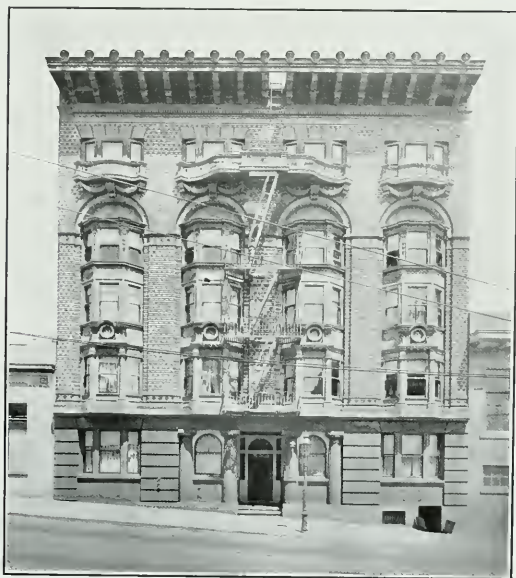
Empress Apartments, San Francisco C. A. Meussdorffer, Architect
