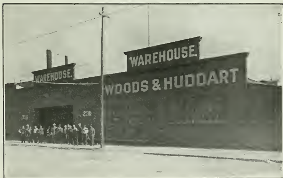
Woods & Huddart Warehouse where Rudgear High Tensile Steel Bars are Stored for Immediate Delivery
