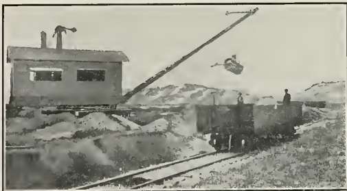
Electric Excavator with Two Yard Bucket.
