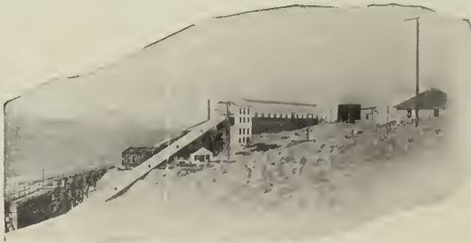
Crusher House and Ore Conveyor, Goldfield Consolidated Mines Company.
