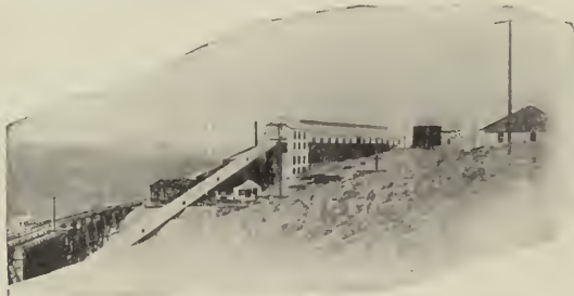
Crusher House and Ore Conveyer, Goldfield Consolidated Mines Company.
