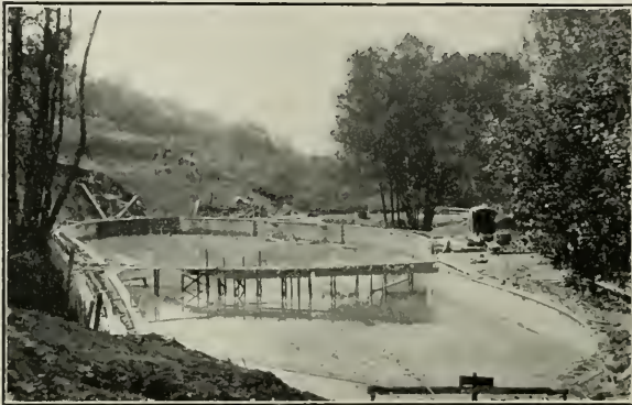
CONCRETE SWIMMING TANK. UNIVERSITY OF CALIFORNIA BERKELEY, CAL. WATERPROOFED WITH MEDUSA COMPOUND
