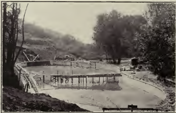
CONCRETE SWIMMING TANK, UNIVERSITY OF CALIFORNIA BERKELEY, CAL.
