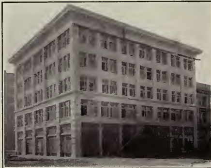
SAUNDERS BUILDING SAN FRANCISCO
