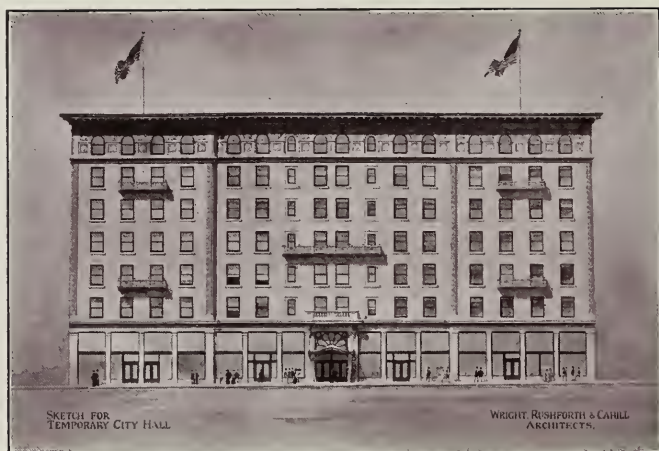
Temporary City Hall, San Francisco. Contract for the Concrete Work Alone Amounted to Nearly $200,000. Foundations, Curtain Walls, Floors and Roof Are All of Concrete Wright, Rushforth & Cohill, Architects
