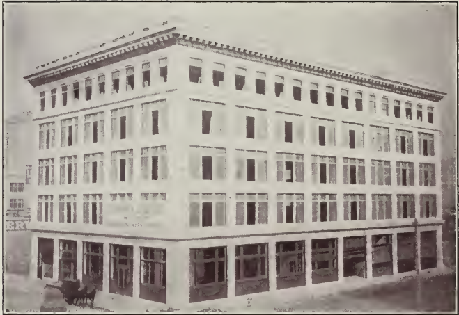
Tillmann & Bendel Building, San Francisco. One of the First Concrete Buildings for Wholesale Purposes Completed after the Fire. The Kahn System of Reinforcement Is Used MacDonald & Applegarth, Architects.
