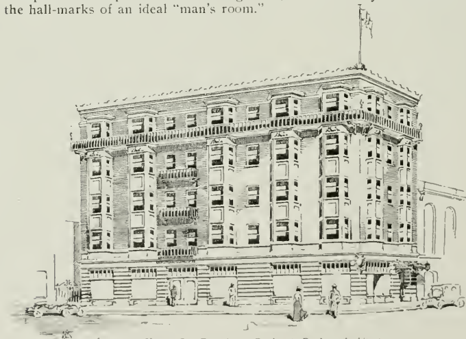
Apartment House, San Francisco. Bugbee & Bugbee Architects
