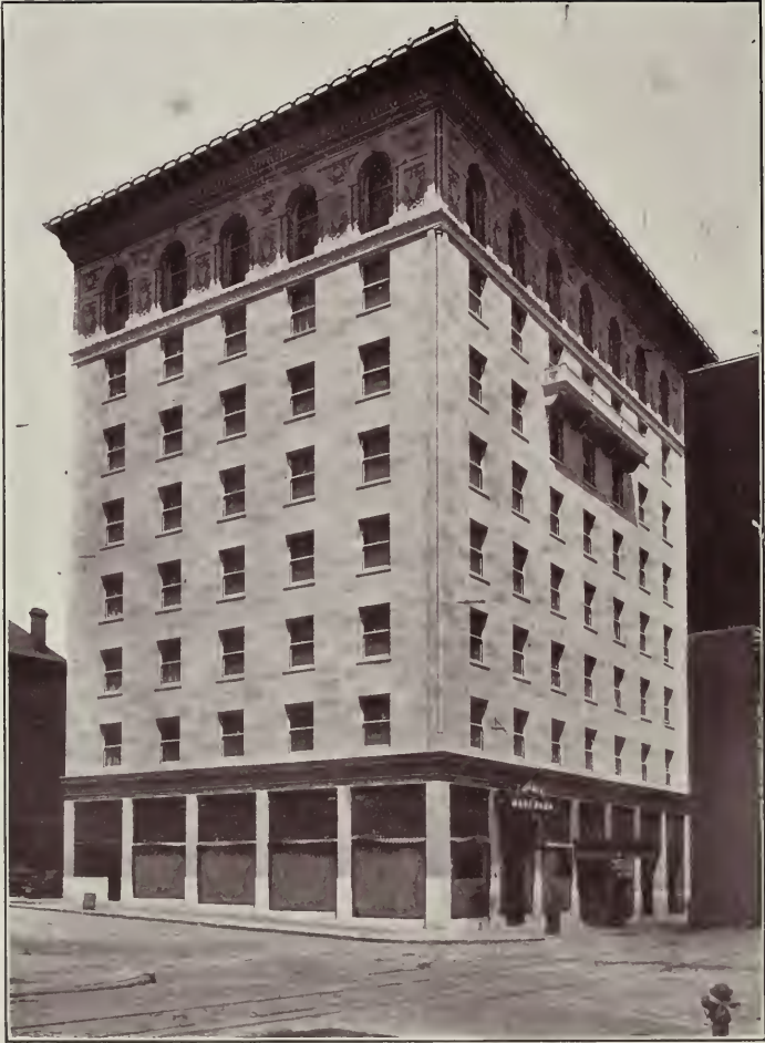
Hotel San Marco San Francisco. Built Entirely of Reinforced Concrete MacDonall & Applegarth Architects
