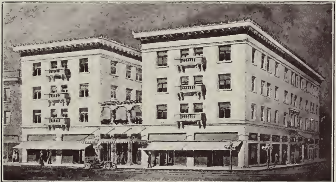
Montgomery Hotel, San Jose. An All-concrete Structure, Reinforced with Deformed Steel Bars. This Building Is Nearing Completion and Will Cost Close to $200,000 William Binder, Architect
