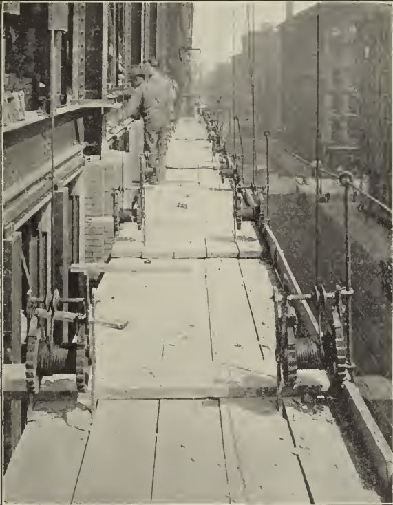
Masons' Suspended Platforms Worked Individually as Units
