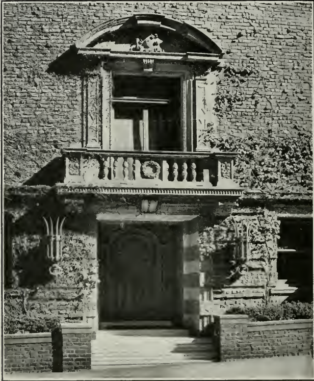
Entrance, Residence of Mr. W. B. Bourn, San Francisco, California
