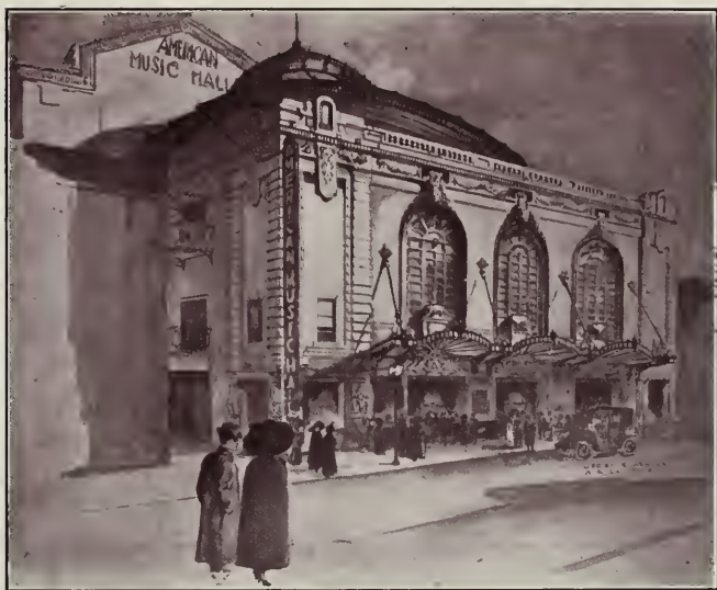
American Music Hall, San Francisco. Steel Frame and Concrete Walls Henry Ives Cobb, Architect
