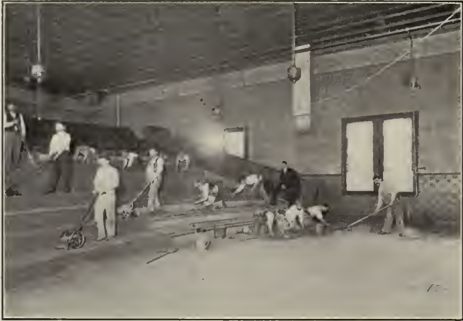
Laying "Kompolite" in Erie Railroad's Fruit Auction Room, Pier 20, New York
