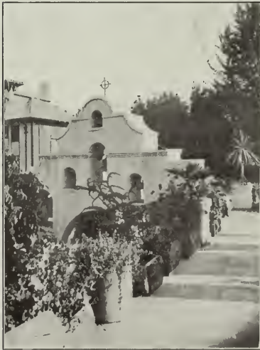
View of Campanile from Balcony
