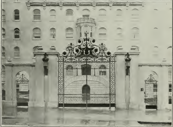
Completed Section and Entrance Gates, St. Mary's Hospital, San Francisco, California.*
