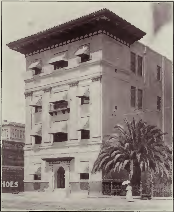
Pacific Telephone Building, San Jose. Steel Frame and Concrete Walls
