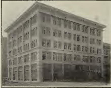
SAUNDERS BUILDING, SAN FRANCISCO
