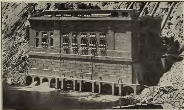
Ferrocinclave roof and floors. Power House, Great Western Power Co., California
