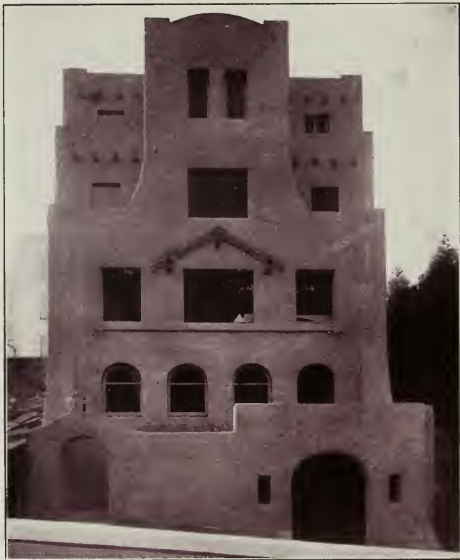
Residence, San Francisco. Unique Design in the Indian Pueblo Style. Exterior of Rough Pebble Cement Chas. F. Whittlesey, Architect
