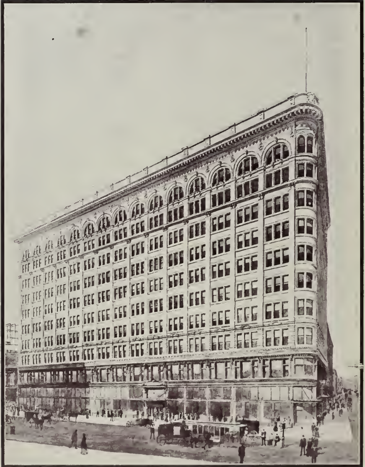
James D. Phelan Building, San Francisco Fireproofed Throughout with Concrete. Exterior of Terra Cotta Tile William Curlett & Son, Architects
