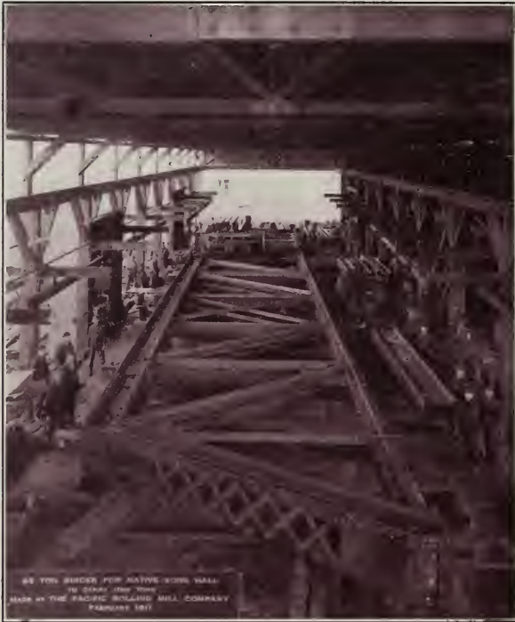
Eighty-two Foot Truss made by Pacific Rolling Mills for Native Sons' Building, San Francisco
