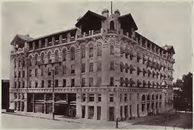
Sacramento Hotel, Sacramento, Col. An All-Reinforced Concrete Structure Sellon & Hemmings, Architects
