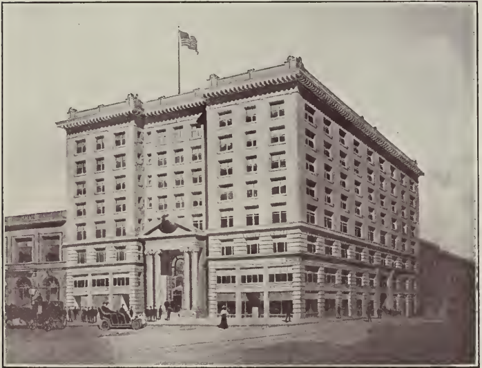
Y. M. C. A. Building, San Francisco, Steel Frame and Reinforced Concrete Walls McDougall Bros., Architects
