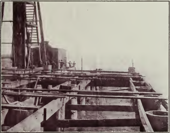
Showing Method of Building Concrete Coissons for Pier Improvements, San Francisco Water Front
