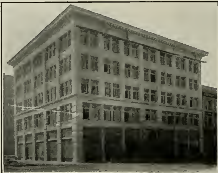
SAUNDERS BUILDING SAN FRANCISCO
