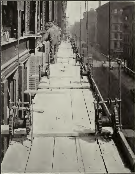
Suspended Platforms Worked Individually as Units
