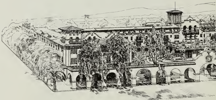
General Panoramic View of Glenwood Mission Inn, Riverside
