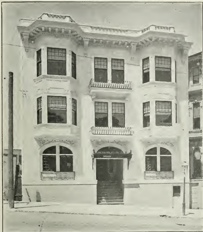
The Laurel Apartments, San Francisco John Tschabold, Painter Crim & Scott, Architects Wallace C. Boswell, Contractor The frame of this building was erected in twelve days
