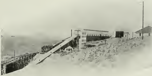
Crusher House and Ore Conveyor, Goldfield Consolidated Mines Company.
