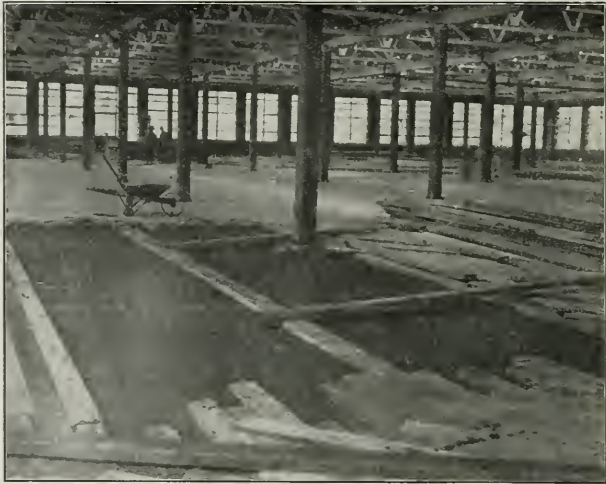
Blake & Johnson Plant, Waterville, Conn. Tar Sub-Floor in Process of Construction.
