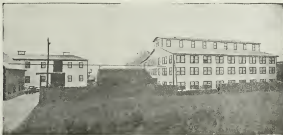
Plant of Woburn Machine Company, Woburn, Mass., showing fire-proof and time proof roofing and siding of ASBESTOS PROTECTED METAL
