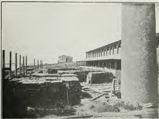
Finished Product Sorted and Piled in Yard Ready for Shipment
