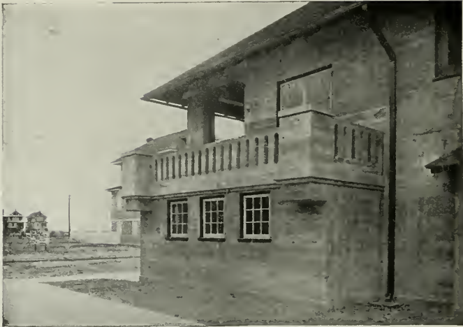
Fig. I.—Detail View Showing Texture of Walls and Substantial Concrete Posts and Balustrade of Porch (The large square posts are hollow, with drainage at the bottom, and will be utilized for plants)
