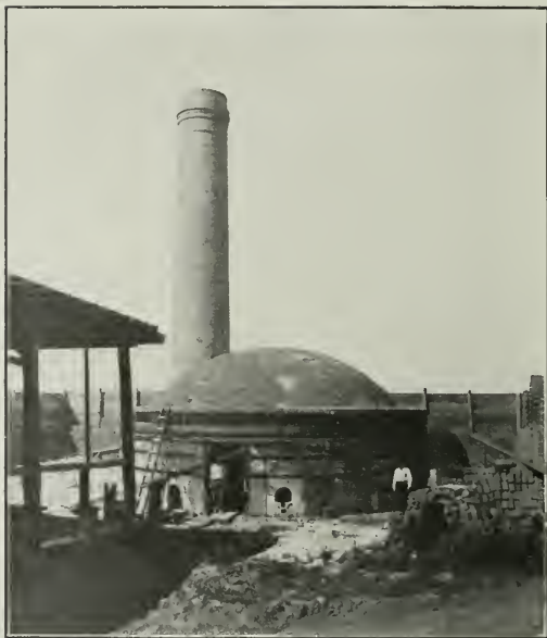
Bee Hive Type of Kiln, Vallejo Brick & Tile Company
