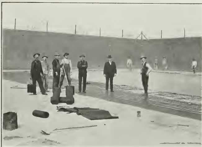
Waterproofing Concrete Bottom of Medford's Municipal Reservoir
