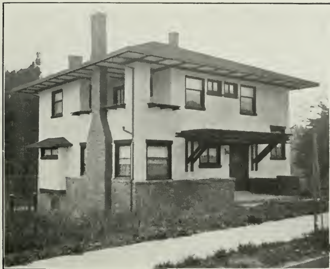
An Oakland Home Finished in Medusa Cement and Monterey White Sand A. W. Smith, Architect
