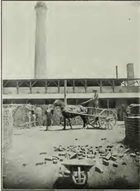
In the Yards of the Vallejo Plant
