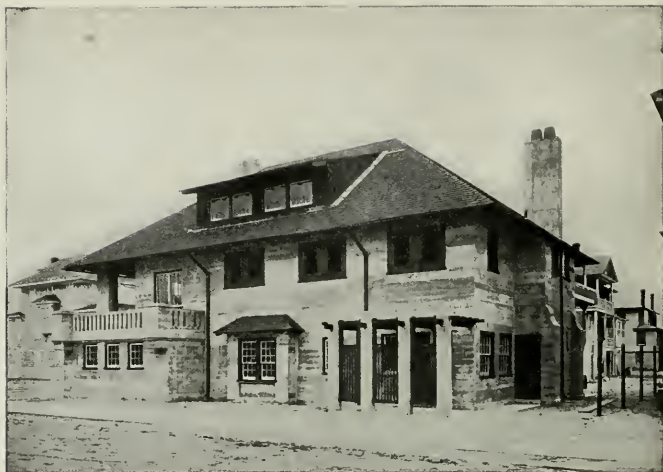
Fig. III.—Side and Rear View Showing Massive Chimney Construction and Interesting Treatment of Concrete Columns
