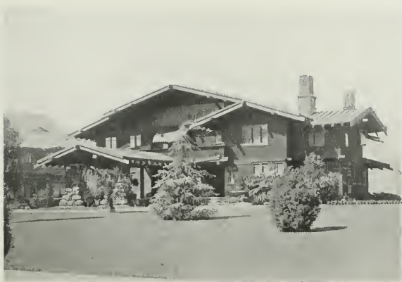
The Cole Bungalow, Pasadena, Cal. Greene & Greene, Architects
