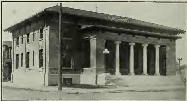
Post Office Building, Santa Rosa, Cal. James Knox Taylor, Supervising Architect, Treasury Department.
