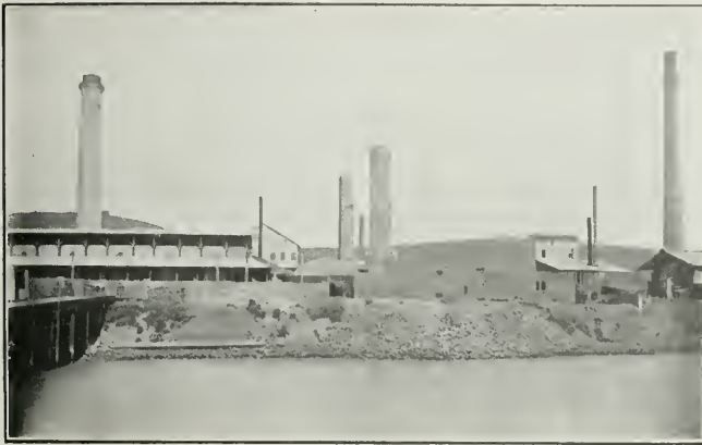
Part of Vallejo Plant from Water Front
