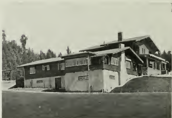
House of Messrs. Glasscock and Edwards, Pasadena, Cal.
