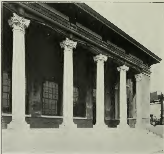
Post Office Building, Santa Rosa, Cal.—Detail of Colonnade James Knox Taylor, Supervising Architect, Treasury Department
