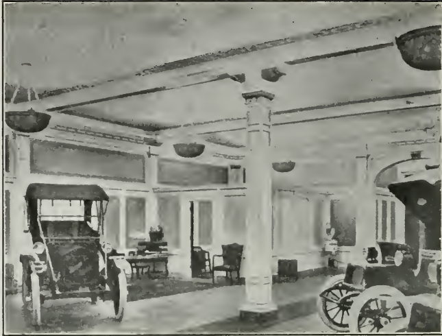
Showing Reflectors, No Exposed Lamps Visible, in a New York Garage
