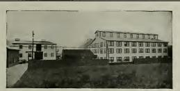
Plant of Woburn Machine Company, Woburn, Mass., showing fire-proof and fume-proof roofing and siding of ASBESTOS PROTECTED METAL
