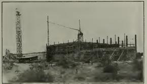
Precooling Ice Plant for Santa Fe Railroad, San Bernardino, Colifornia Showing Gravity System Delivering Concrete 502 Feet From the Mixing Plant
