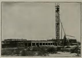
Precooling Ice Plant for the Santa Fe Railroad, San Bernardino, California—Square Tower, 172 Feet High, 20-Foot Boom with 40-Foot Auxiliary Boom to Support Distributing Pipe
