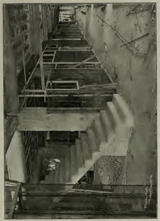
Photo Showing Metal Partitions Before Plastering
