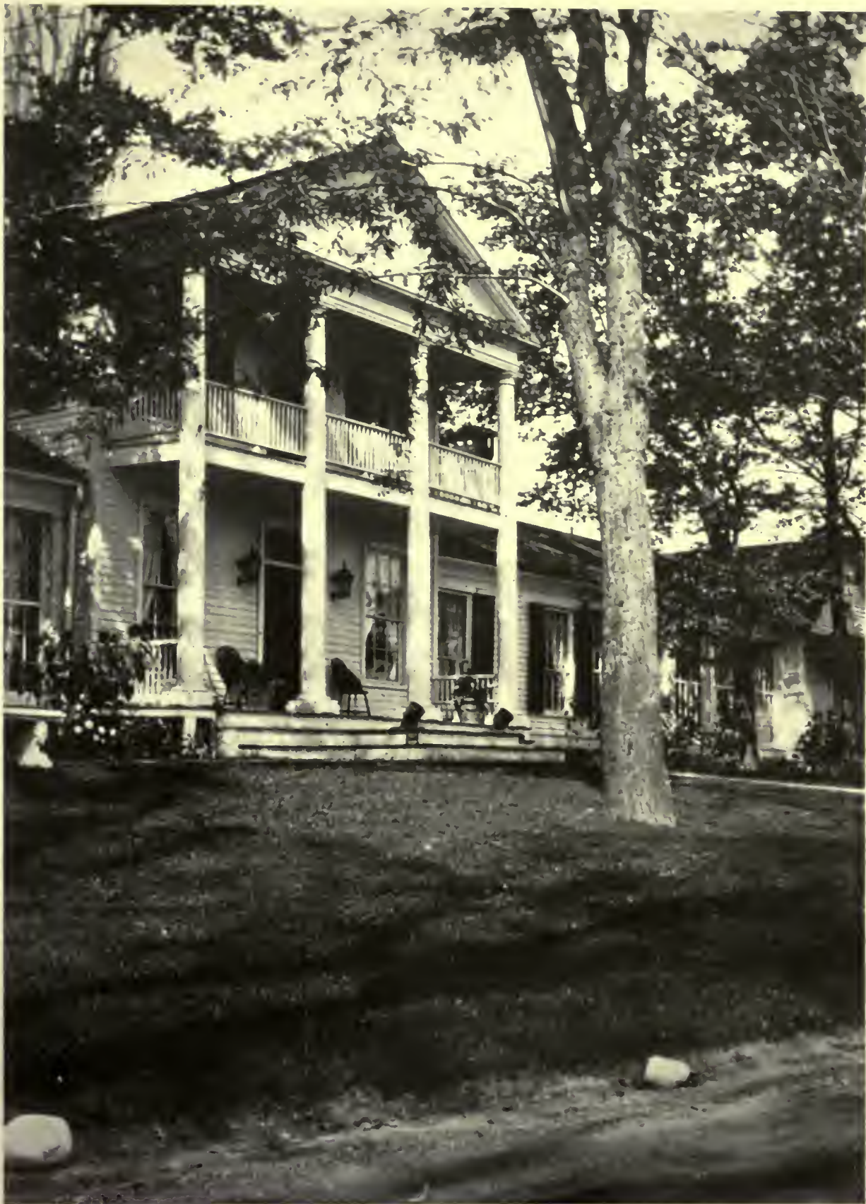
HOUSE OF S. H. P. PELL, ESQ., FORT TICONDEROGA, N. Y. ALFRED C. BOSSOM, ARCHITECT
