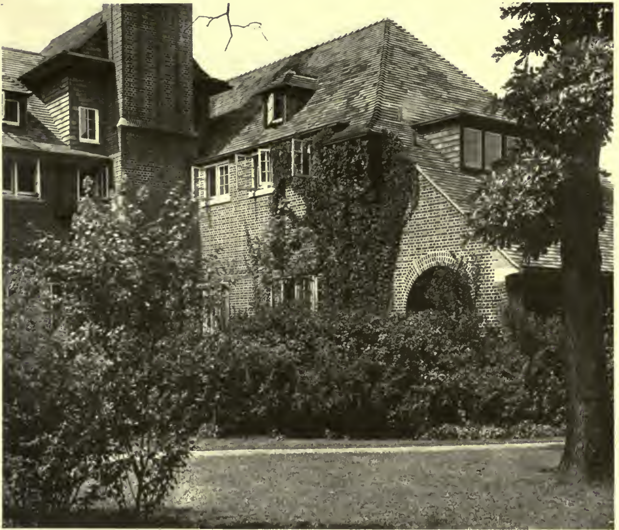
DETROIT GOLF CLUB, DETROIT, MICH. ALBERT KAHN, ARCHITECT
