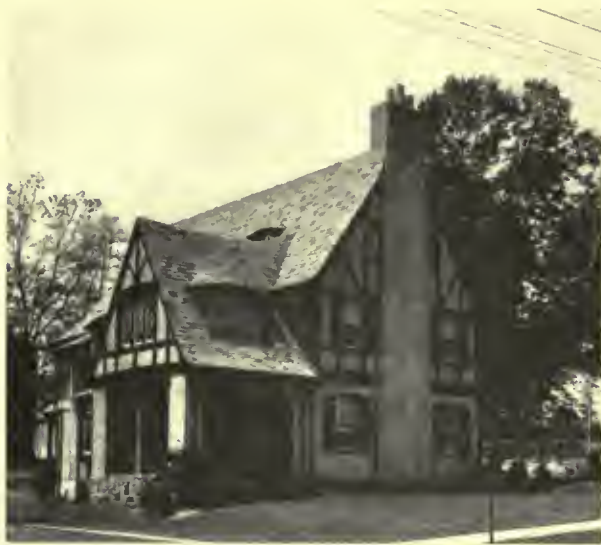
Slate roof with curved surfaces. Kew Gardens, L. I. Walter McQuade, Architect. The selection of vari-colored slates, for this roof is particularly appropriate for half-timbered construction
