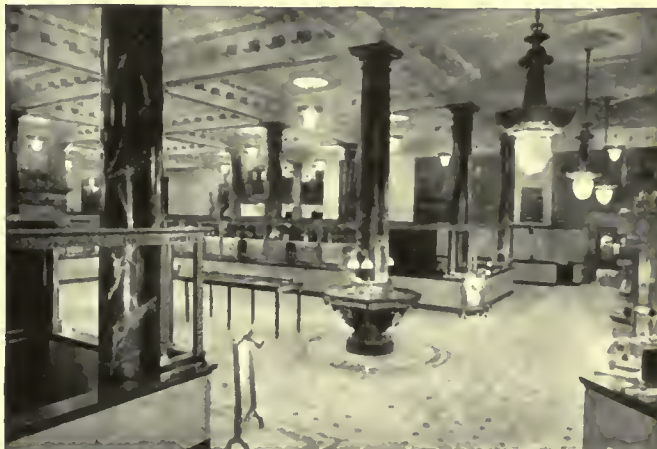
Remodeled fixture with one 300-watt Mazda lamp and three hidden 40-watt bulbs—420 watts—four foot-candles.
