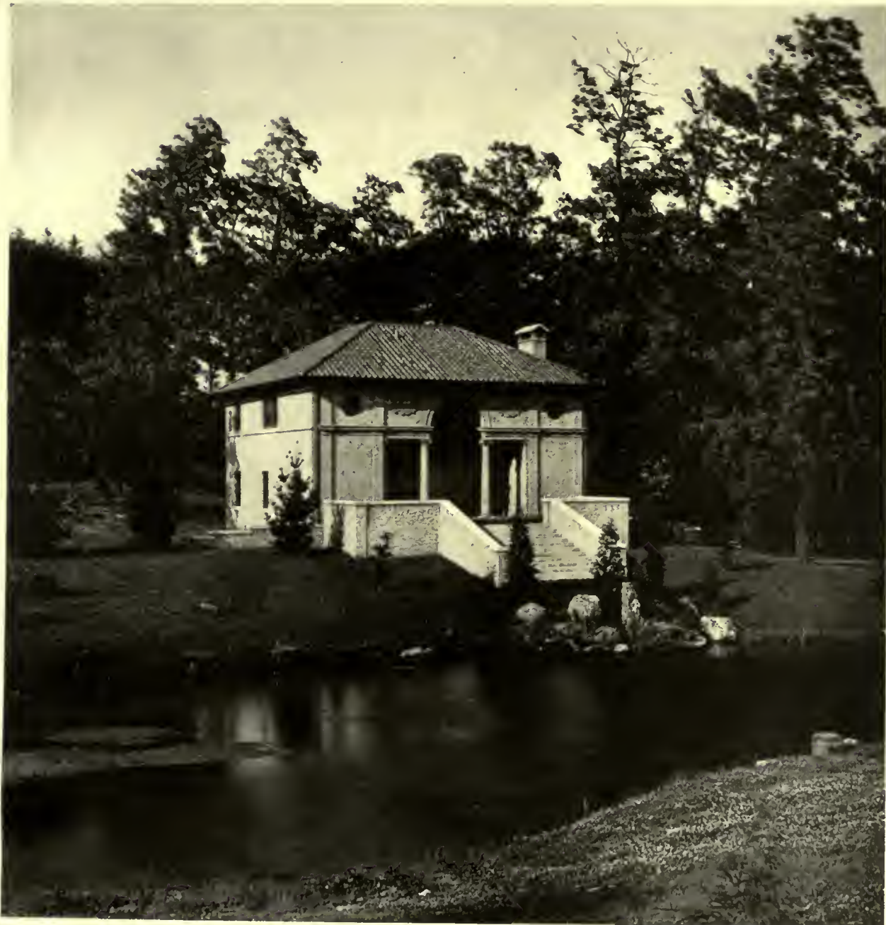
GARAGE OF A. E. BURR, ESQ., SCARSDALE, N. Y. A. J. BODKER, ARCHITECT
