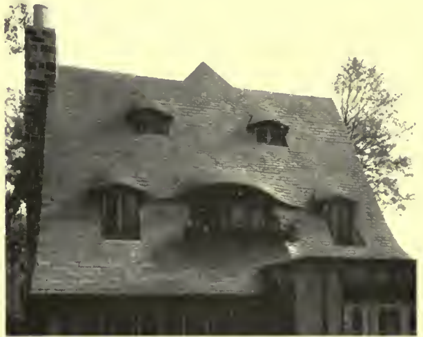
A roof which illustrates the possibilities of slate as a material for broken surfaces. Glenwolde, L. I. Walter McQuade, Architect
