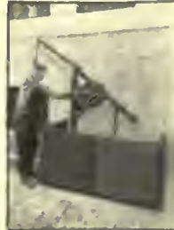
Operator "dips" overhead crane, descends iron ladder and lowers hoisting head.
