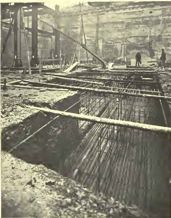
REINFORCEMENT IN COLUMN FOOTINGS BUSH BUILDINGS, LONDON
