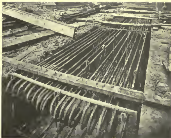
REINFORCEMENT IN COLUMN FOOTINGS SHOWING HOOK ANCHORAGE—BUSH BUILDINGS, LONDON
