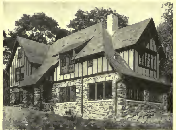
Residence of Mr. V. A. Wiss, Morris Plains, N. J. Stone walls, stucco walls and a slate roof make a fire resistant house
