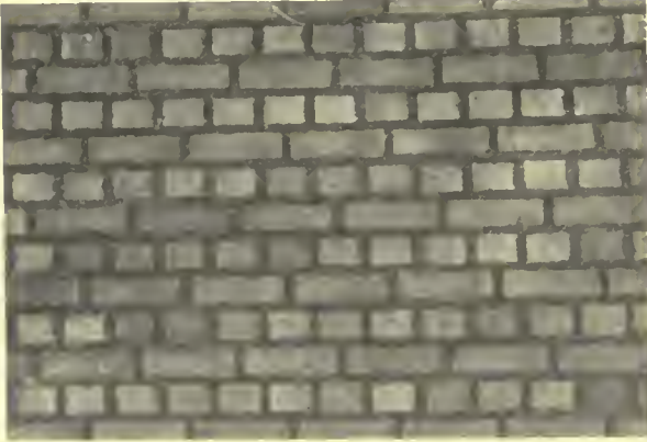
A WALL OF CONCRETE BRICK WITH FLUSH JOINTS
