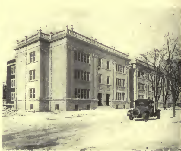
Apartment houses in Brookline, Mass., in which all floors are carried on light steel joists. Partitions are of plaster on metal lath carried on metal studding
