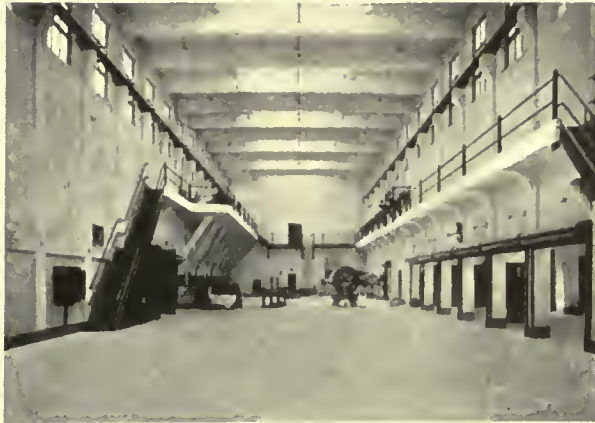
The architectural possibilities of reinforced concrete. Cantilevered columns to carry travelling cranes and working platforms in a high narrow room spanned by deep beams suggest medieval halls.
