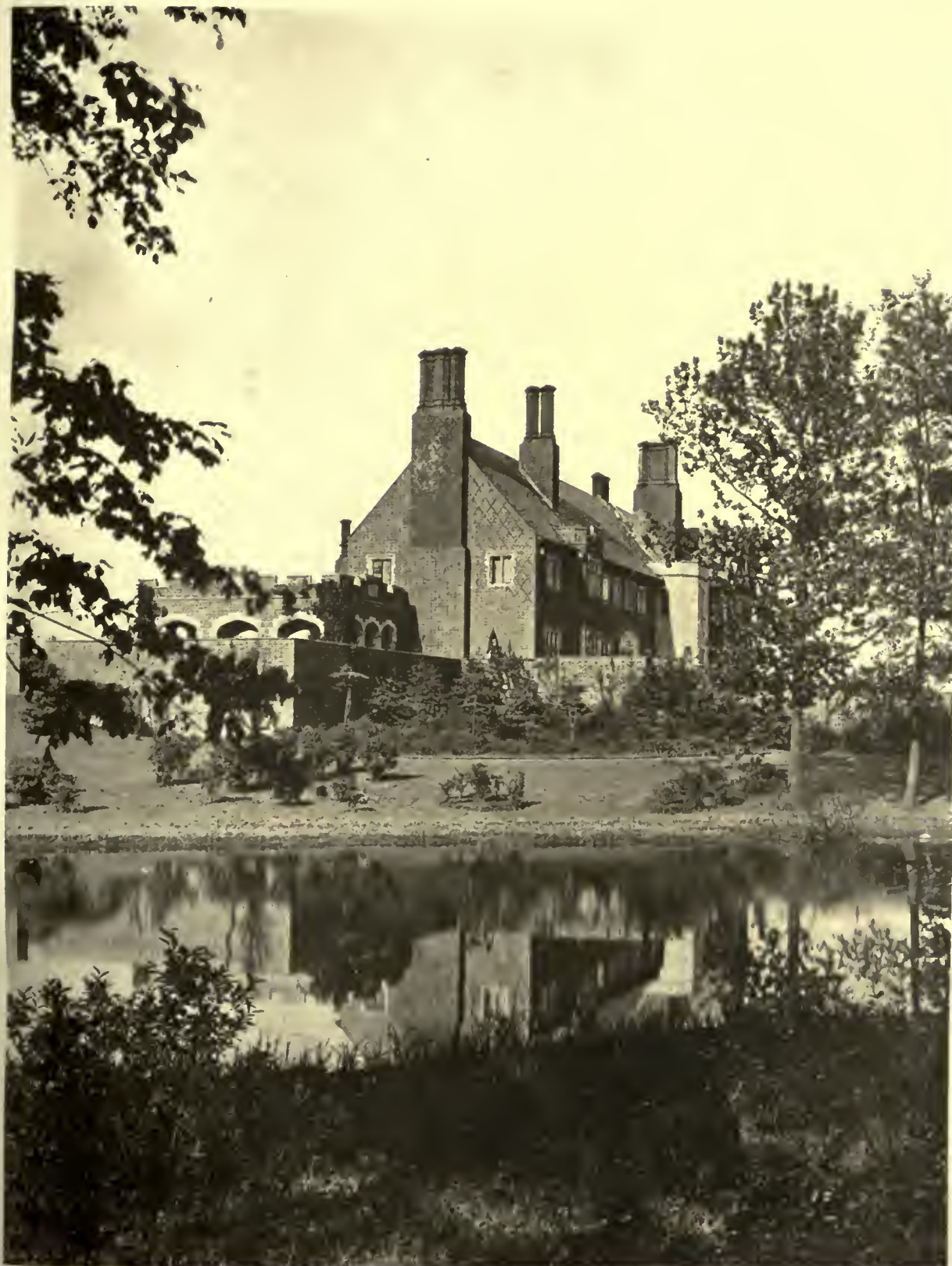
WEST ELEVATION, LOOKING ACROSS POND
