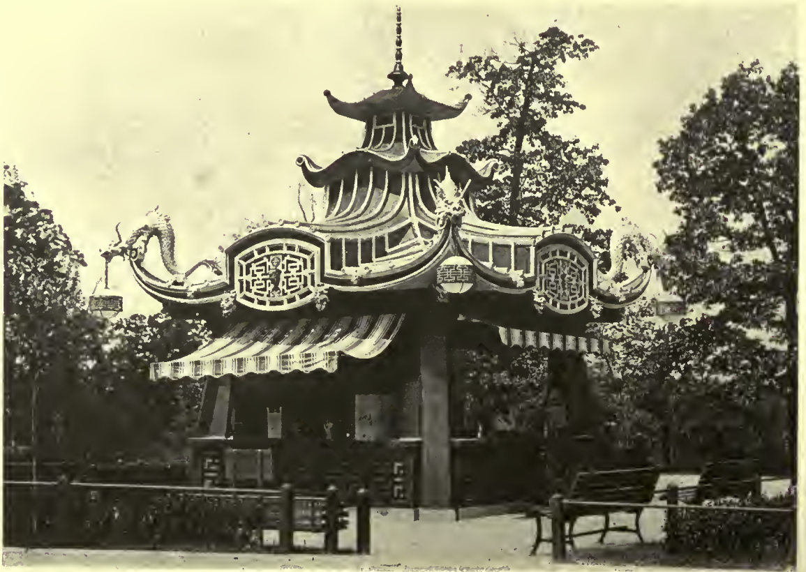
CHINESE PAVILLION IN ST. LOUIS (MO.) ZOOLOGICAL GARDENS T. B. BARNETT & CO., ARCHITECTS
