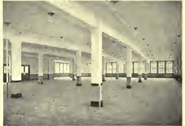
Reinforced concrete. Top floor of an administration building. Long span slabs on beams carried by columns. No intermediate girders. Square columns are inferior to round columns in case of fire.
