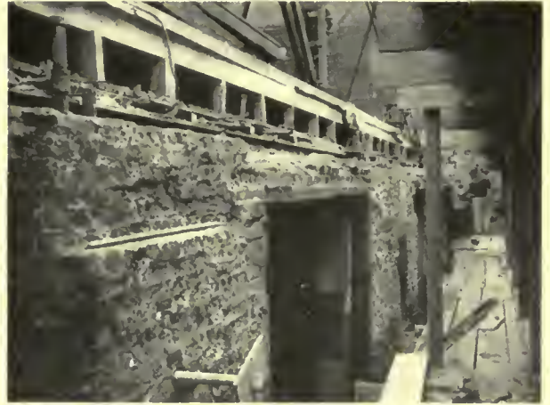
Old brick walls prepared for the stone facing
