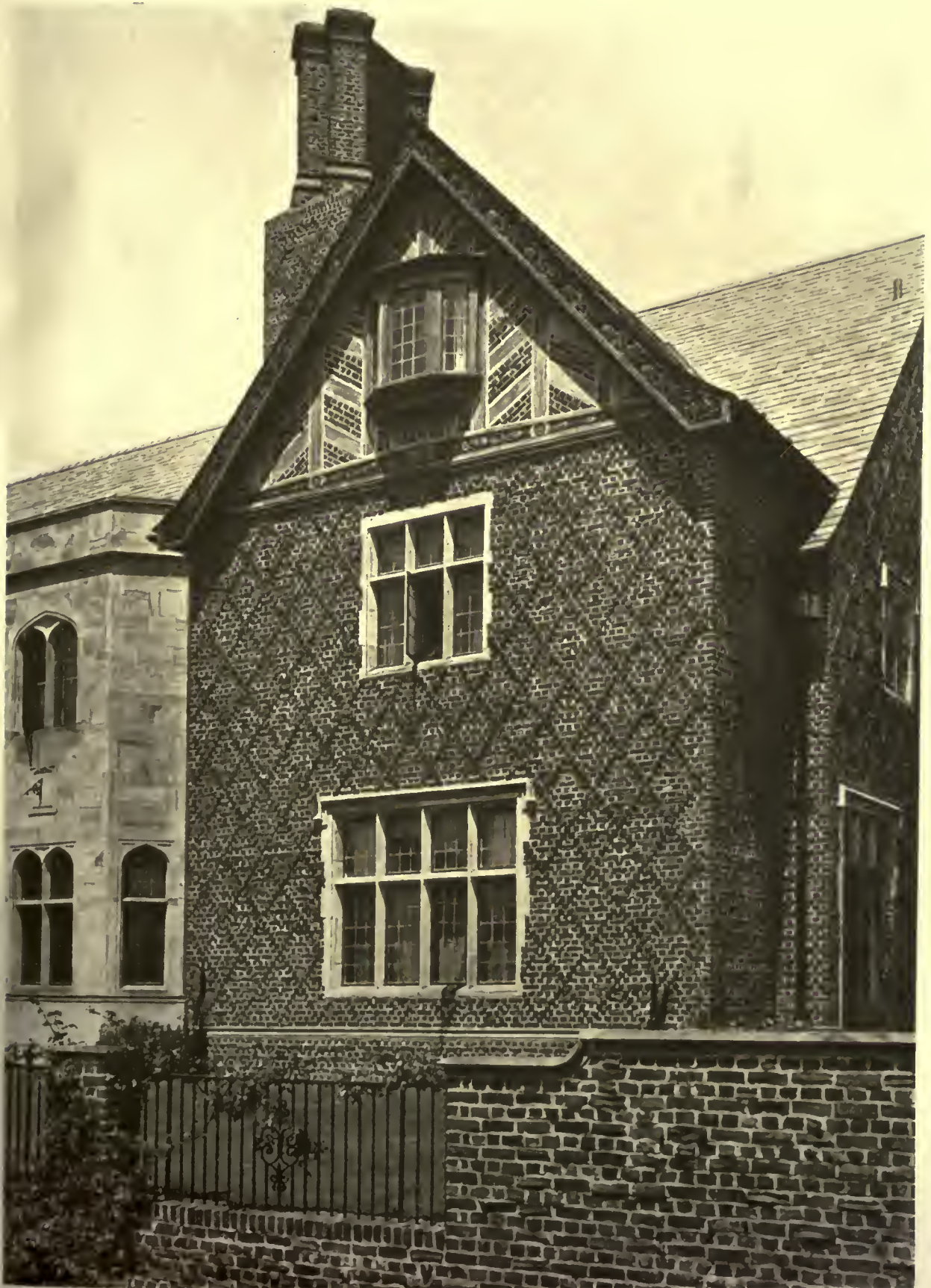
GABLE OF DINING ROOM
