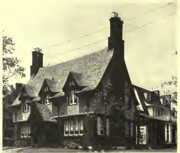
A fine example of slate roof with broken and curved surfaces. Kew Gardens, L. I. Walter McQuade, Architect
