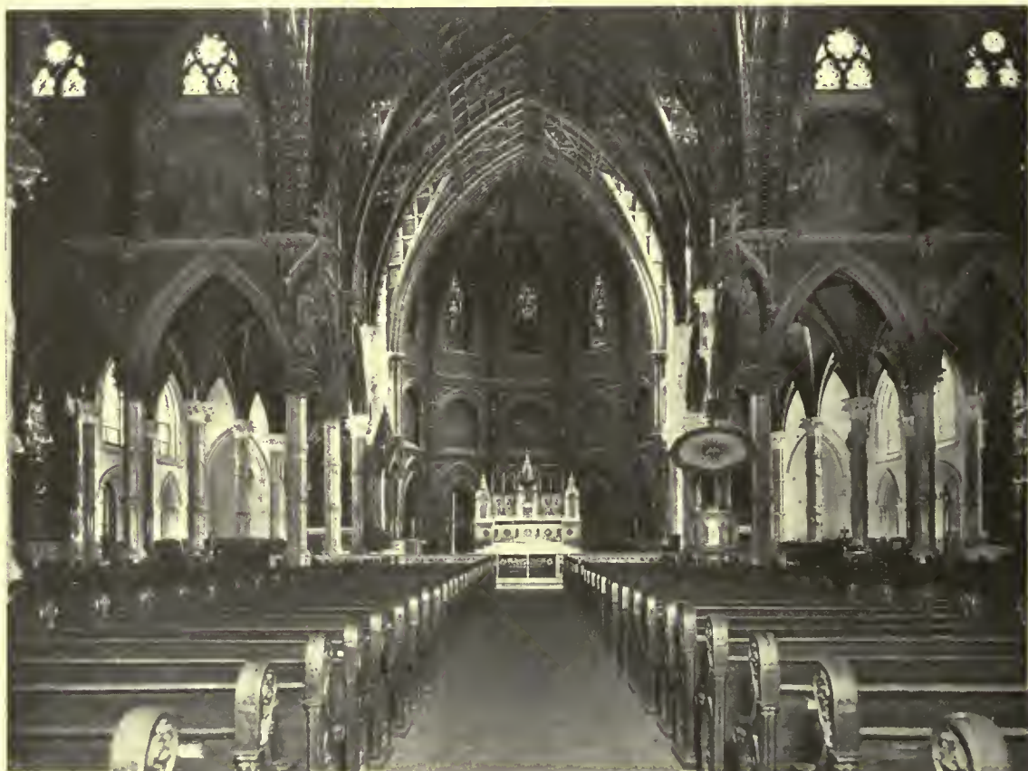
INTERIOR VIEW OF HOLY NAME CATHEDRAL, CHICAGO; AFTER ENLARGEMENT, BEFORE NEW WORK WAS DECORATED
