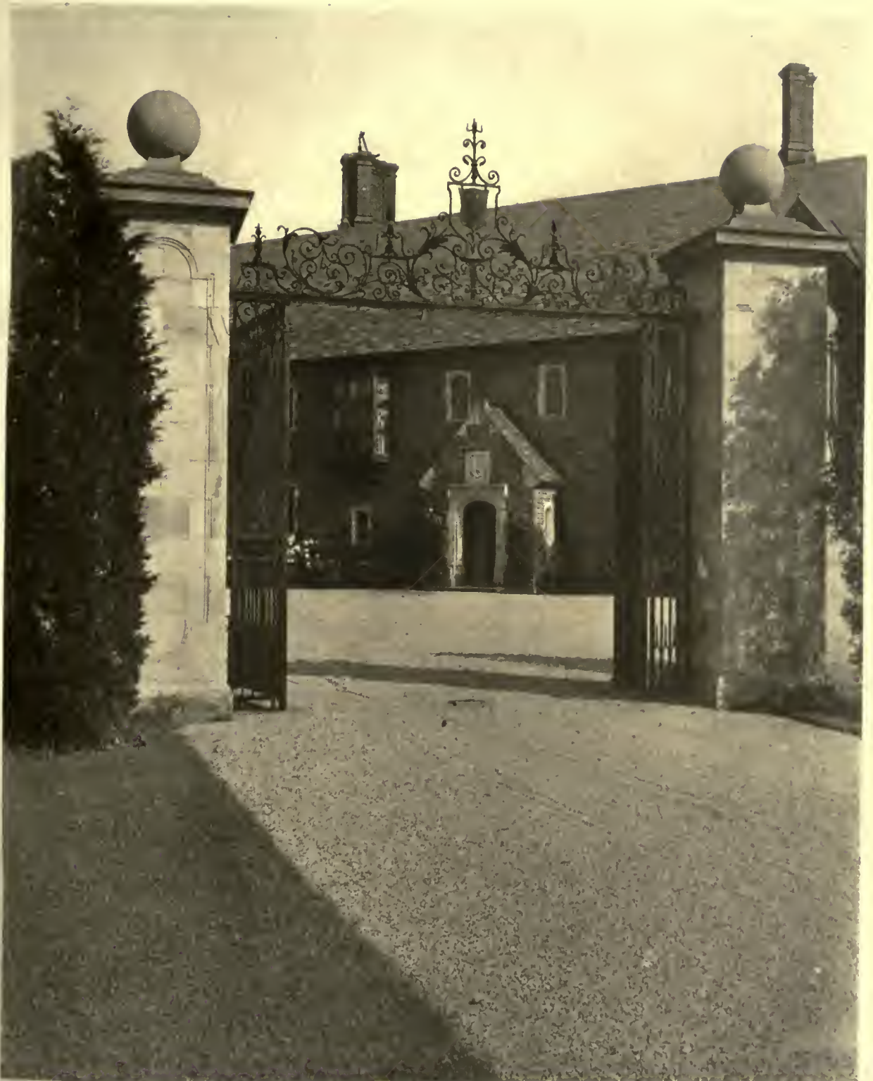
VISTA INTO COURT THROUGH ENTRANCE GATES
