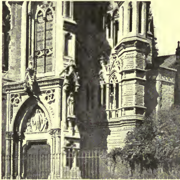
Details of Principal Facade of the Church of St. John, Barcelona John Martorell, Architect
