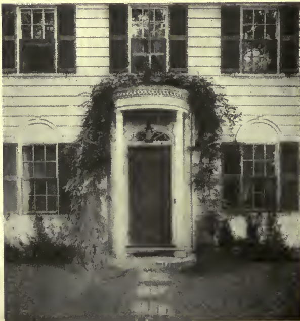
Door Detail—Residence of Miss E. S. Cushing, Waban, Mass. Grandgent & Elwell, Architects
