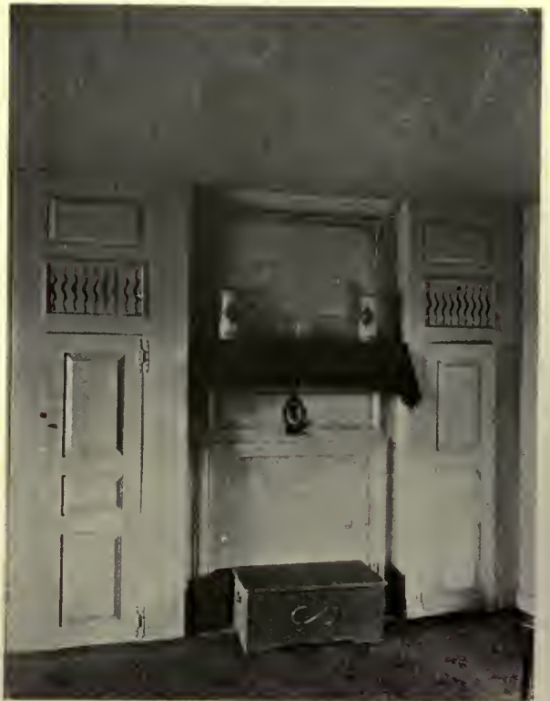
Cupboards with ventilating perforations, Pledger House, near Salem
