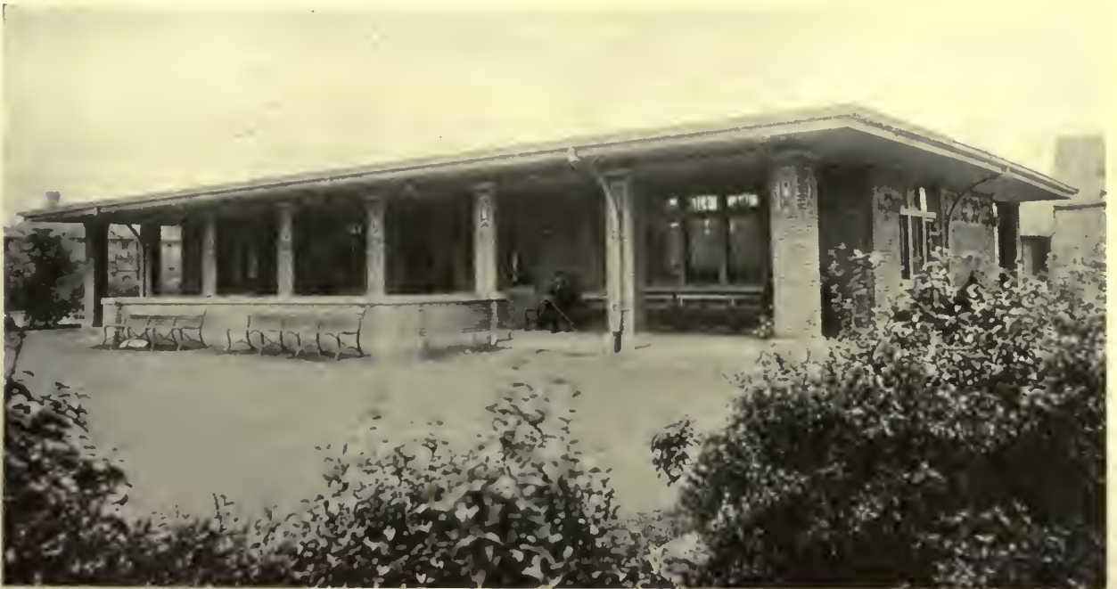
REST BUILDING OF CONCRETE BRICK IN A MILWAUKEE PUBLIC PARK ALFRED C. CLAS, ARCHITECT
