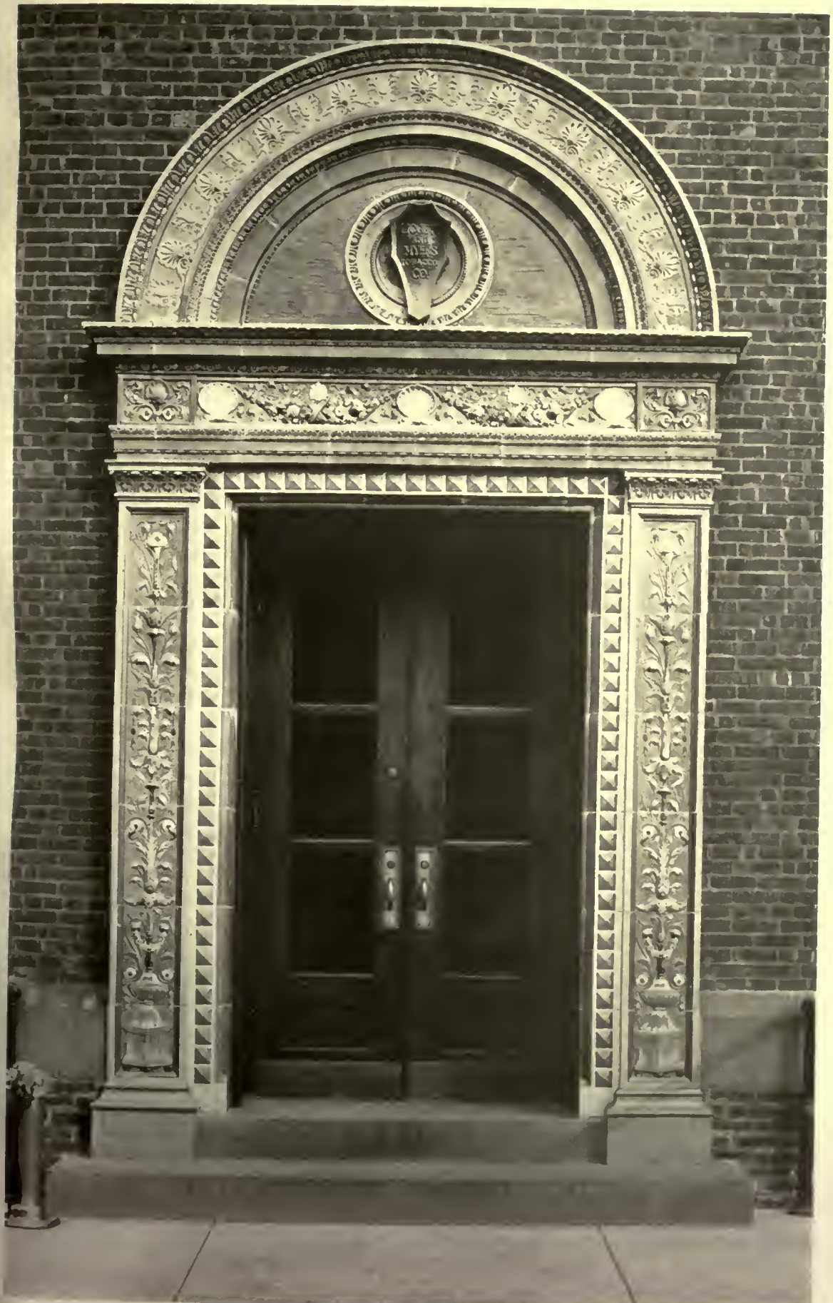
POLYCHROME TERRA COTTA DOORWAY
