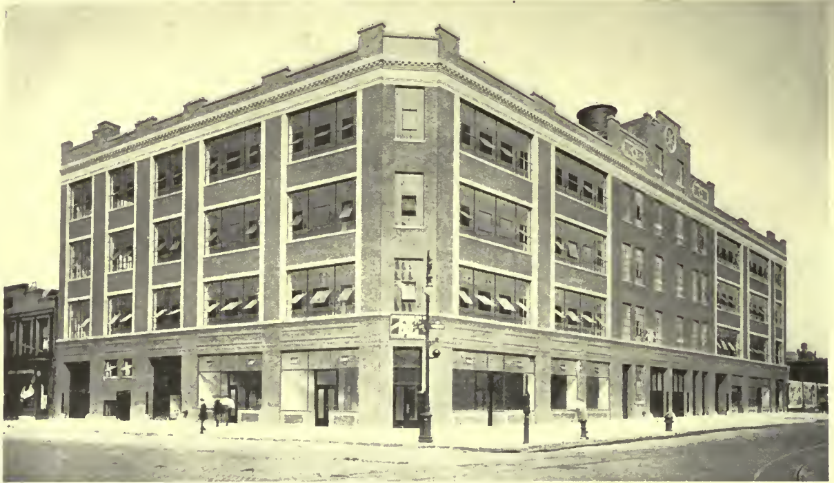
Garage, 23rd Street and 13th Avenue, New York City. Chelsea Moore Co., Owners. W. M. Farrar, Architect Standard Concrete Steel Co., Engineers and Builders.
