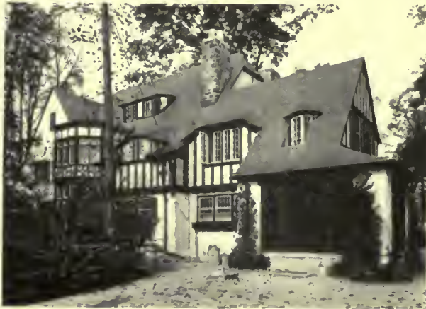
Residence with slate roof, Glenwolde, L. I. Walter McQuade, Architect
