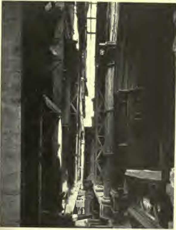
VIEW OF SANCTUARY OF HOLY NAME CATHEDRAL, CHICAGO, DURING ALTERATIONS. TAKEN FROM INTERIOR WHEN GAP WAS ABOUT THREE FEET WIDE
