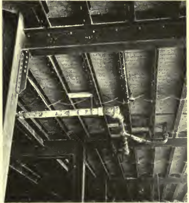
Underside of pressed steel floor
