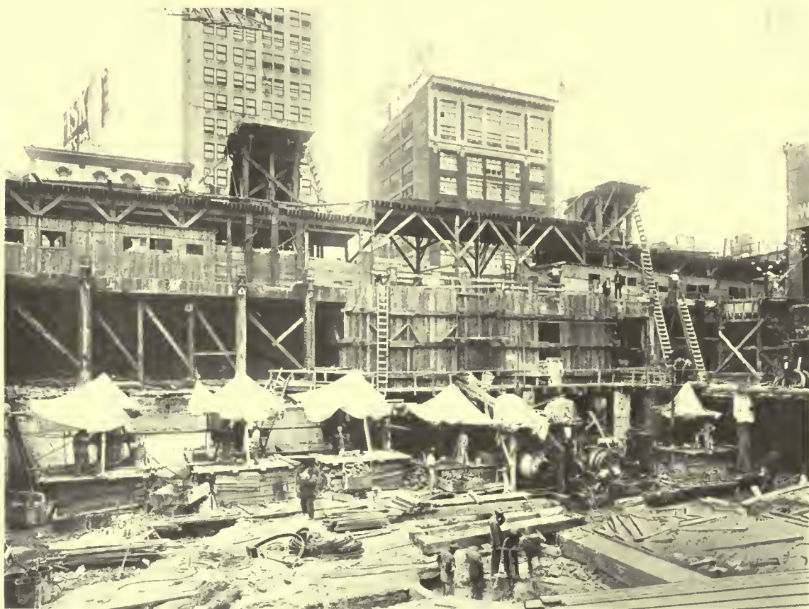
STARTING THE CAISSONS FOR BANK AND OFFICE BUILDING ON THE SITE OF THE OLD HOTEL PONTCHARTRAIN, DETROIT. IN THE FOREGROUND THE CONCRETE MAT IS BEING CUT FOR A CAISSON
