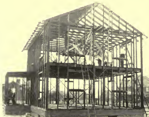
Frame work of metal lumber house ready for lath. Rear view
