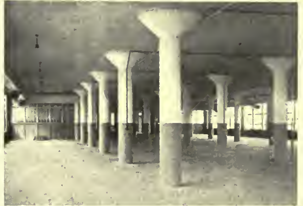
Reinforced concrete. Girderless floor carried on large column capitals without drop heads.
