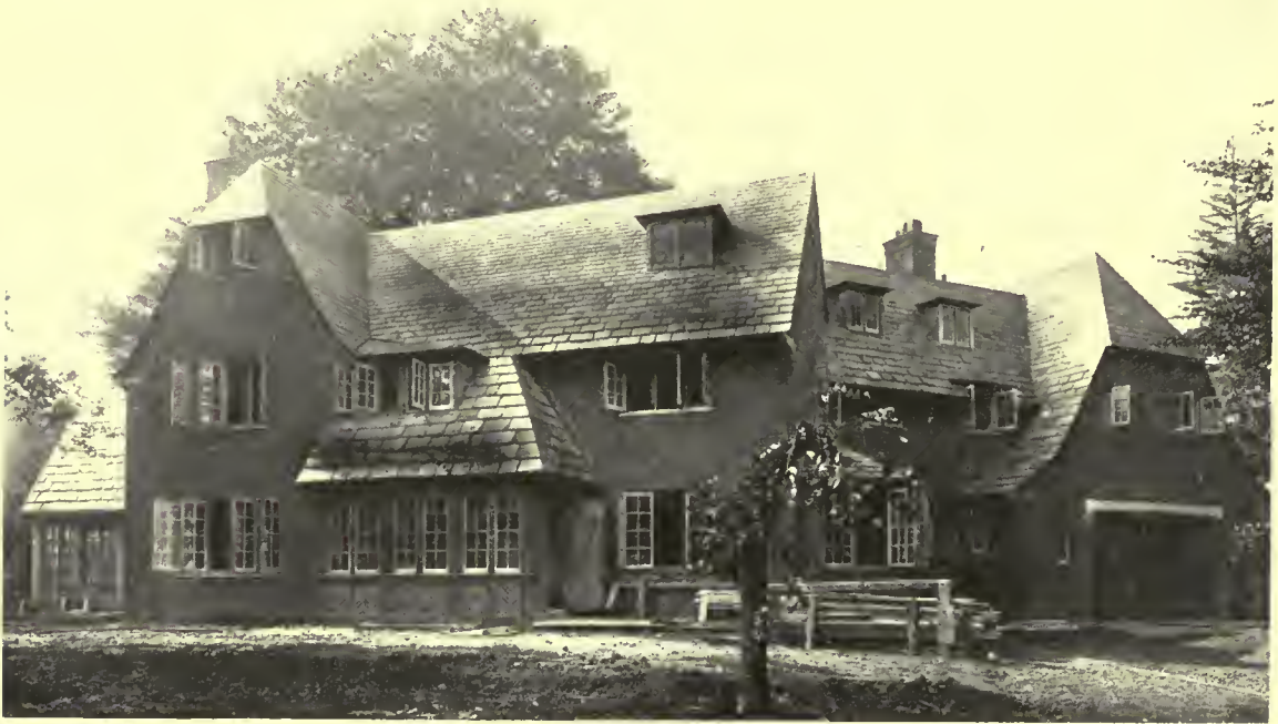
Residence of Mr. E. B. Meyerowitz, So. Orange, N. J. The permanent character of slate roofing permits it to be laid on varying pitches without changing the head-lap
