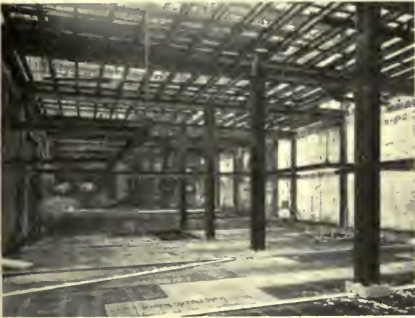
Telephone Exchange, Akron, Ohio. Brick bearing walls. Interior was of ordinary wood joist floor construction, wood studding and wood lath. Gutted by fire the interior was reconstructed with structural steel and steel lumber joists
