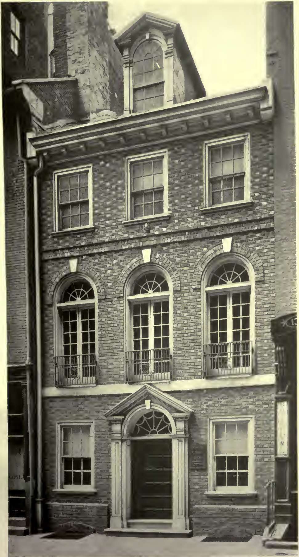
BUILDING AT 132 SOUTH FOURTH STREET, PHILADELPHIA, PA. ALTERATIONS BY C. A. ZIEGLER, ARCHITECT
