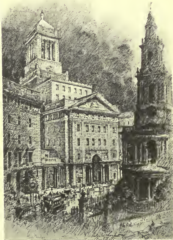
PERSPECTIVE VIEW OF BUILDING AND CHURCH OF ST. MARY LE STRAND, SHOWING "SQUARE" TOWER AND STREET FRONT OF BUILDING LIMITED TO THE LEGAL HEIGHT OF EIGHTY FEET TO CORNICE LINE
