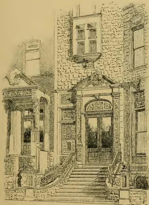
DOORWAY AT FIFTH AVENUE AND SIXTY-SEVENTH STREET.
