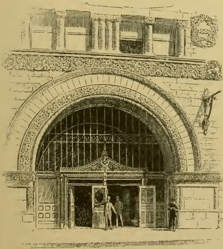
ENTRANCE TO THE PHENIX BUILDING.
