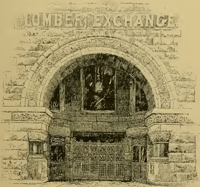
LUMBER EXCHANGE, MINNEAPOLIS.
