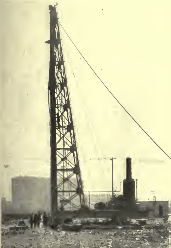
ALL METAL PILE DRIVER AND 60-H.P. ENGINE.
