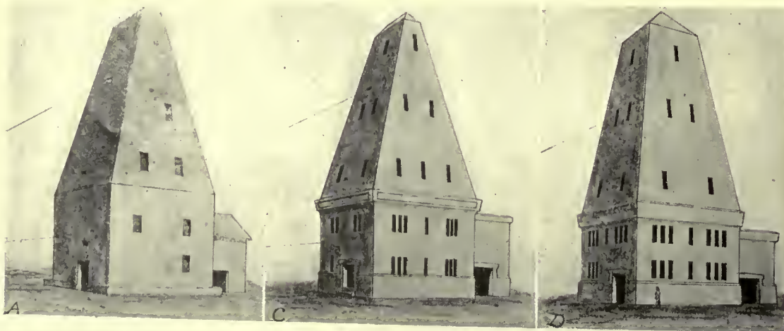
A—THE ORIGINAL DESIGN. C—DESIGN OF CONSTRUCTION ENGINEERS, RETAINING THE RECTANGULAR TOP. D.—THE RESTUDIED DESIGN WITH SQUARE TOP. SEE OTHER PLATES FOR FINAL DESIGNS AS COMPLETED BY THE ARCHITECT
