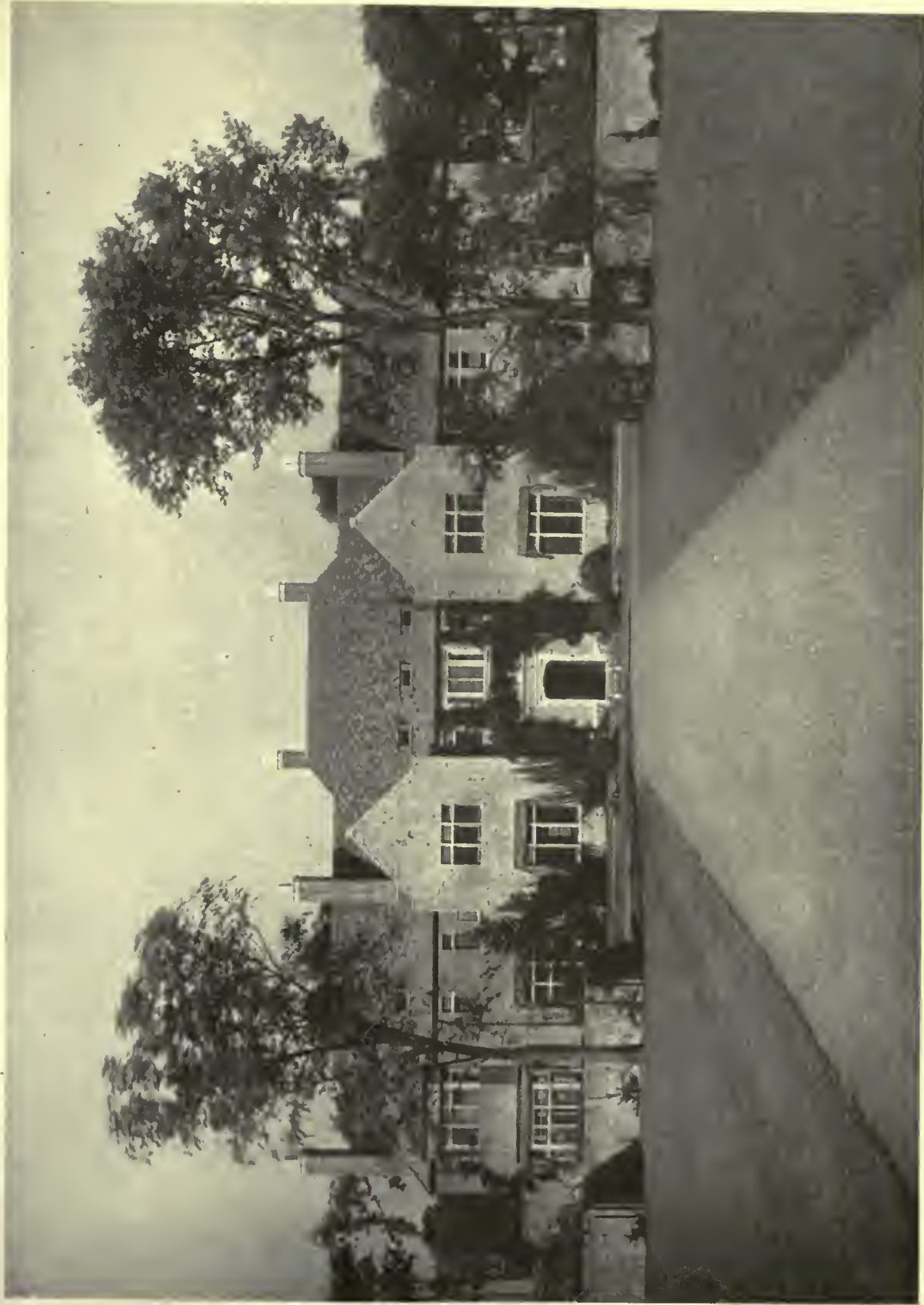
HOUSE OF A. G. MILBANK, HUNTINGTON, LONG ISLAND JOHN MEAD HOWELLS, ARCHITECT
