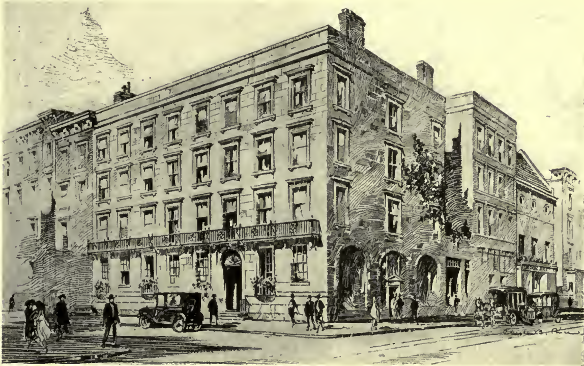
A GROUP OF REMODELED HOUSES ON MADISON AVENUE, NEW YORK FREDERIC R. KING, ARCHITECT
