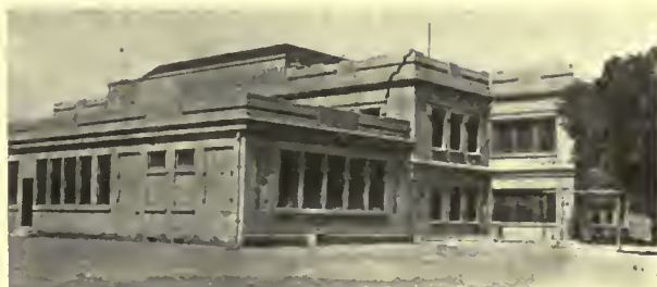
INGLEWOOD GRAMMAR SCHOOL. One-Story Annex in the foreground is practically undamaged.
