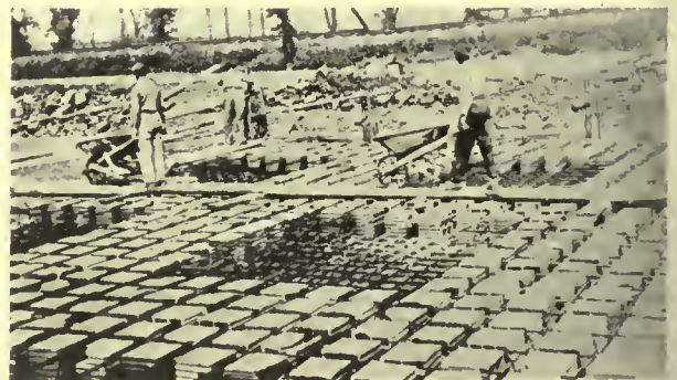
CONSTRUCTION OF FOOTINGS
