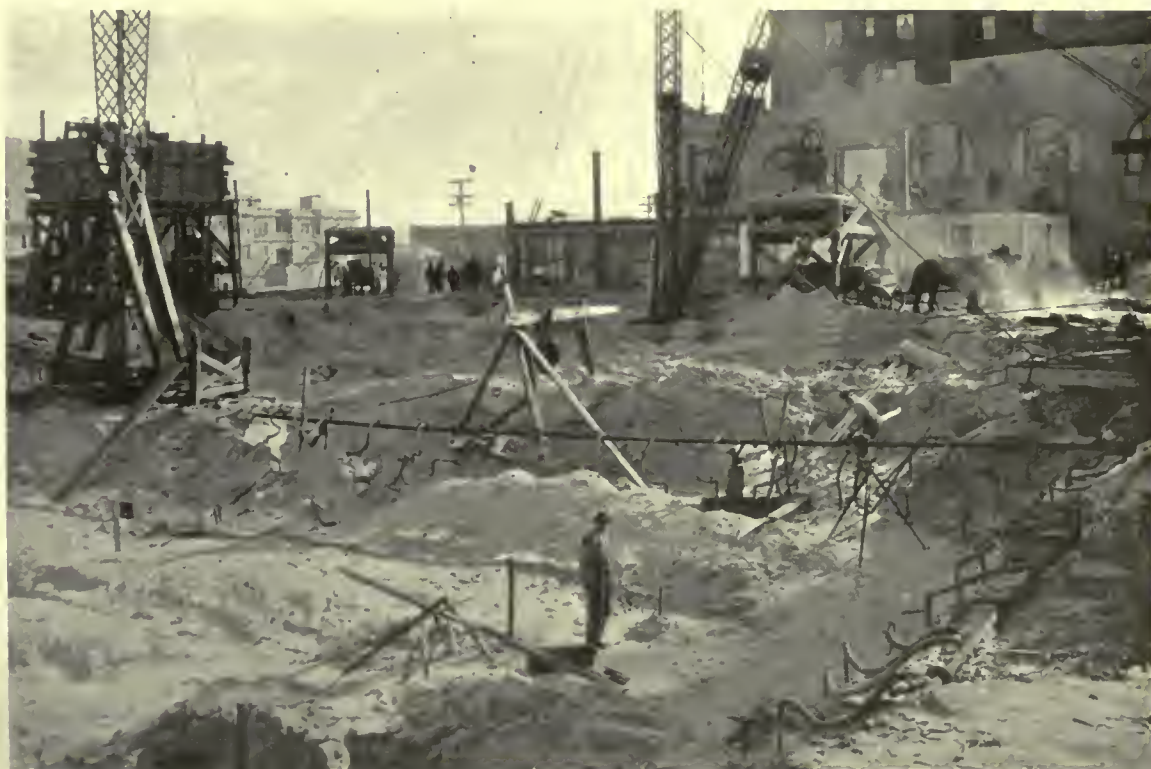
EXCAVATION IN PROGRESS, AMBASSADOR HOTEL ANNEX, ATLANTIC CITY, N. J. This photograph was taken December 15, 1919. The tops of the well points and connecting pipe line used to drain the excavation are plainly visible.
