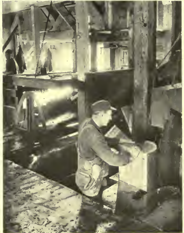
FIG. 4. QUARTER SECTIONS BEING TRIMMED
