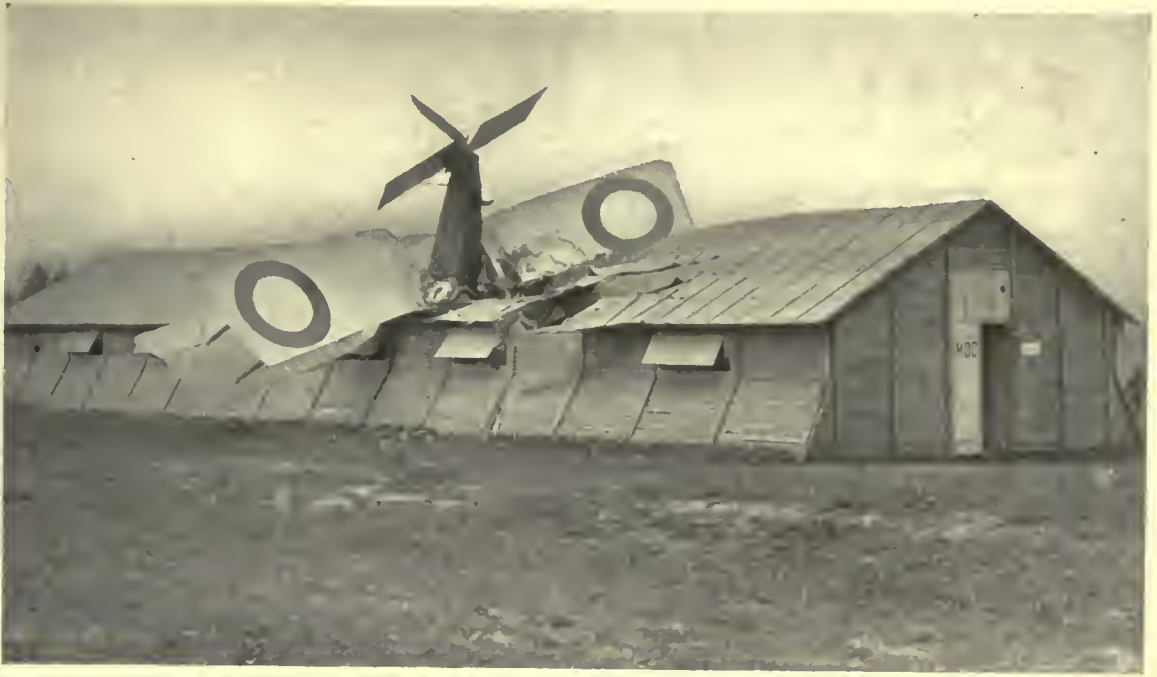
HARRIAN TYPE BARRACK WITH AN UNEXPECTED VISITOR
