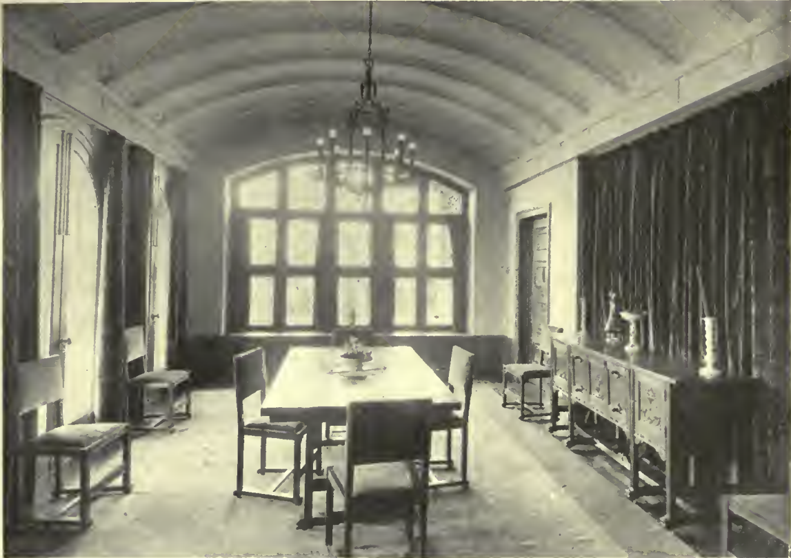
DINING ROOM Finished in cement plaster, stippled between ceiling beams
