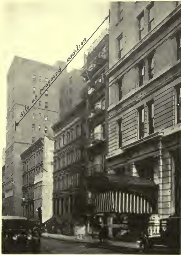
WESTERLY END OF FIFTY-EIGHTH STREET FRONTAGE OF PLAZA HOTEL, SHOWING EXISTING CONDITIONS AT SITE OF PROPOSED ADDITION
