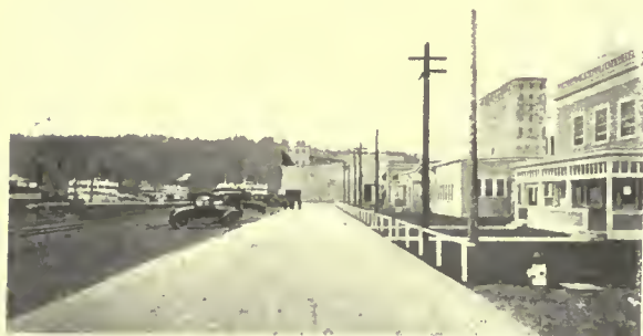
MAIN ENTRANCE TO TERMINAL
