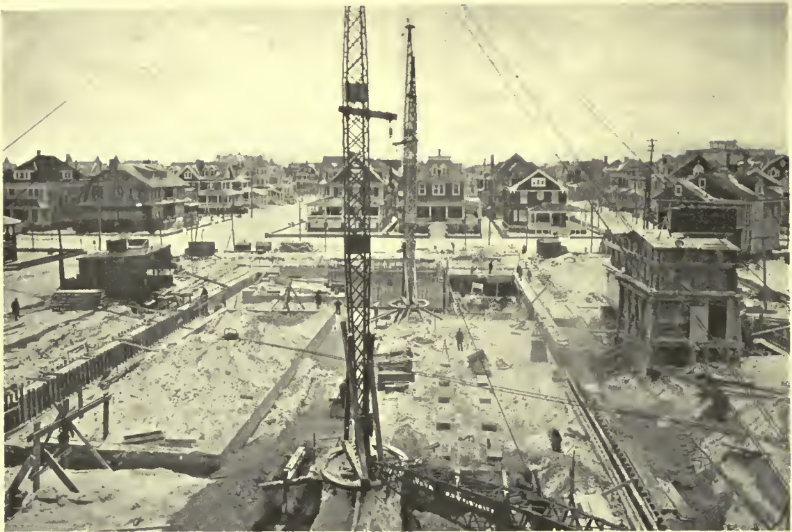
GENERAL VIEW OF THE SITE DURING CONSTRUCTION OF FOUNDATIONS
