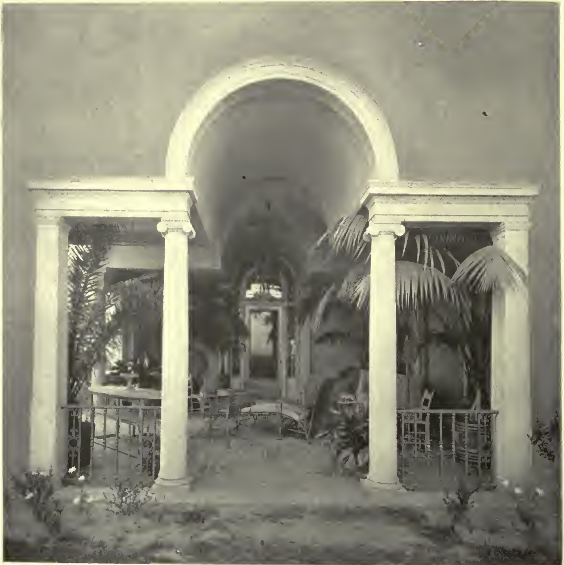
LOGGIA IN HOUSE OF GEORGE E. CRANMER, DENVER, COLORADO
