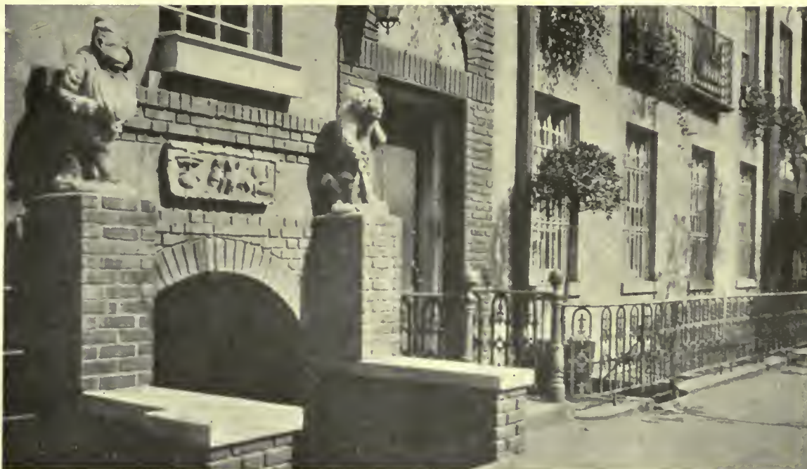
ENTRANCE DETAIL—ALTERATION TO HOUSE ON EAST 19th STREET, NEW YORK FREDERICK J. STERNER, ARCHITECT
