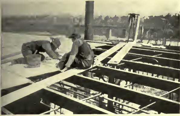
ROOF CONSTRUCTION—STEEL CHANNELS AND POROUS SLABS
