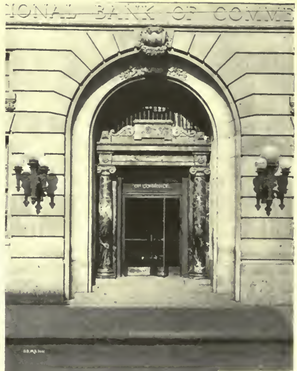
MAIN ENTRANCE TO A BANK BUILDING
