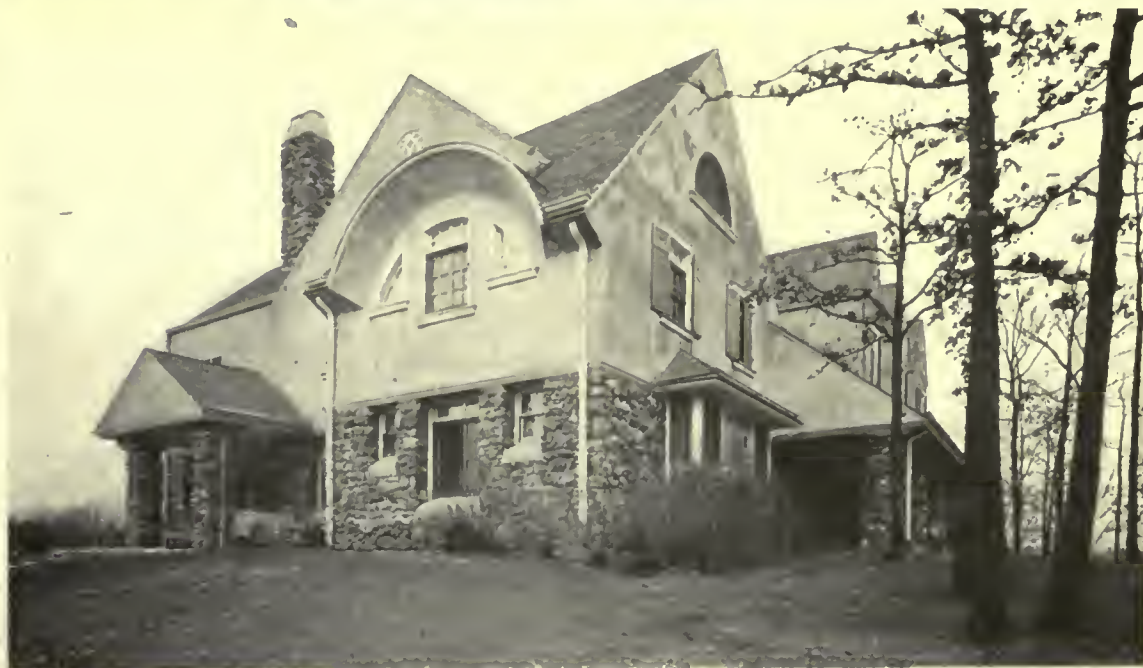
HOUSE OF GEORGE S. JOHNS, ST. LOUIS COUNTY, MO. T. P. BARNETT CO., ARCHITECTS
