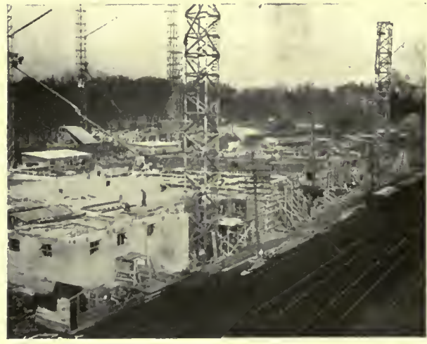
THE LOWELL TEXTILE MILL AND STOREHOUSE IN COURSE OF CONSTRUCTION
