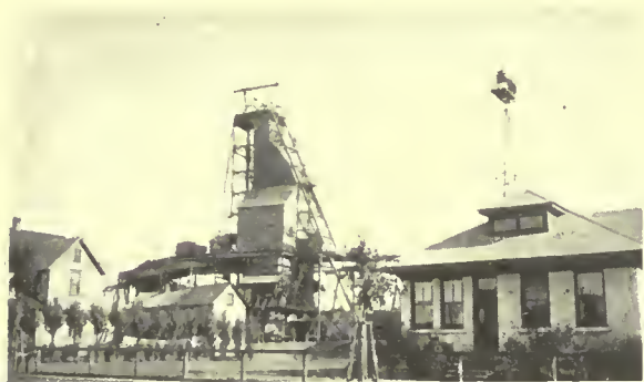
A STRUCTURAL STEEL HEAD-FRAME
