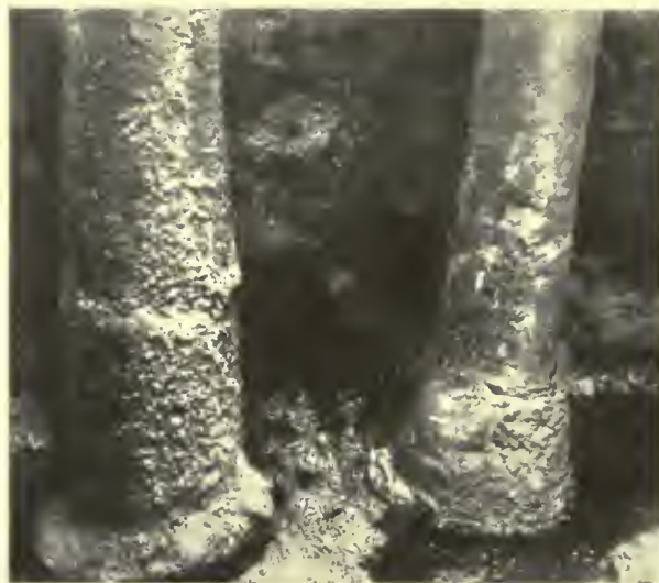
TWO PEDESTAL PILES, EXCAVATED FOR INSPECTION
