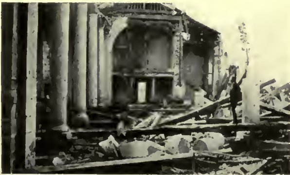
NEUVILLY-MEUSE. THE CHURCH BEYOND REPAIR
