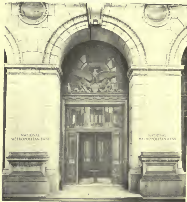
REVOLVING DOOR USED IN LARGE OPENING Space on Each Side and Above Revolving Door Filled With Glass Panels. Note the Heavy Exterior Doors Which Are Closed and Locked after Banking Hours.
