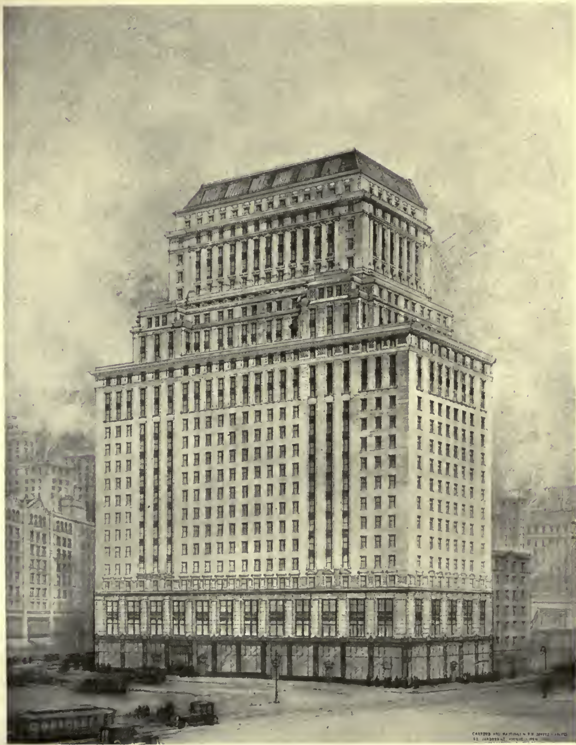
FISK BUILDING, NEW YORK CITY CARRERE & HASTINGS AND R. H. SHREVE, ARCHITECTS
