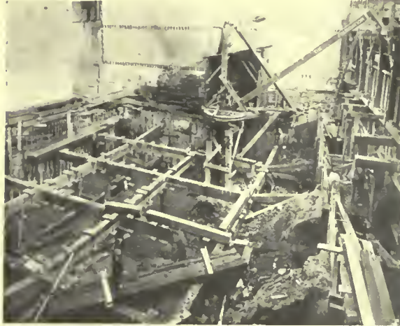
EARLY STAGES OF FOUNDATION WORK, SEABOARD BANK BUILDING, NEW YORK CITY
