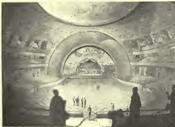
INTERIOR VIEW OF MODEL FOR COLISEUM, SAN ANTONIO, TEXAS
