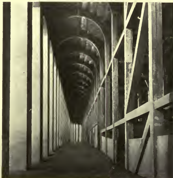
VIEW SHOWING SUPPORTING CONSTRUCTION
