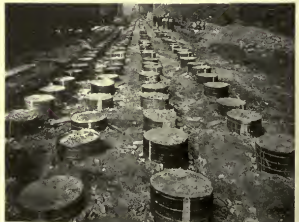
GROUP OF RAYMOND CONCRETE PILES READY FOR CONCRETE CAP
