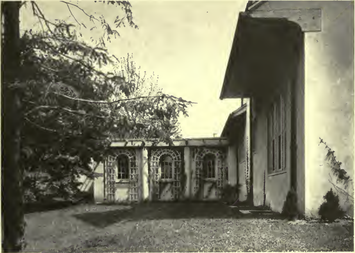
VIEW SHOWING GARAGE
