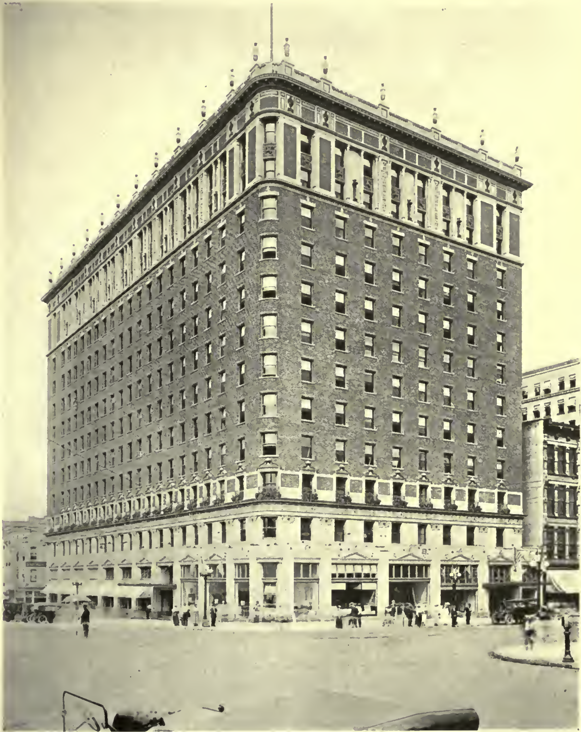
HOTEL DESHLER, COLUMBUS, OHIO HOLABIRD & ROCHE, ARCHITECTS
