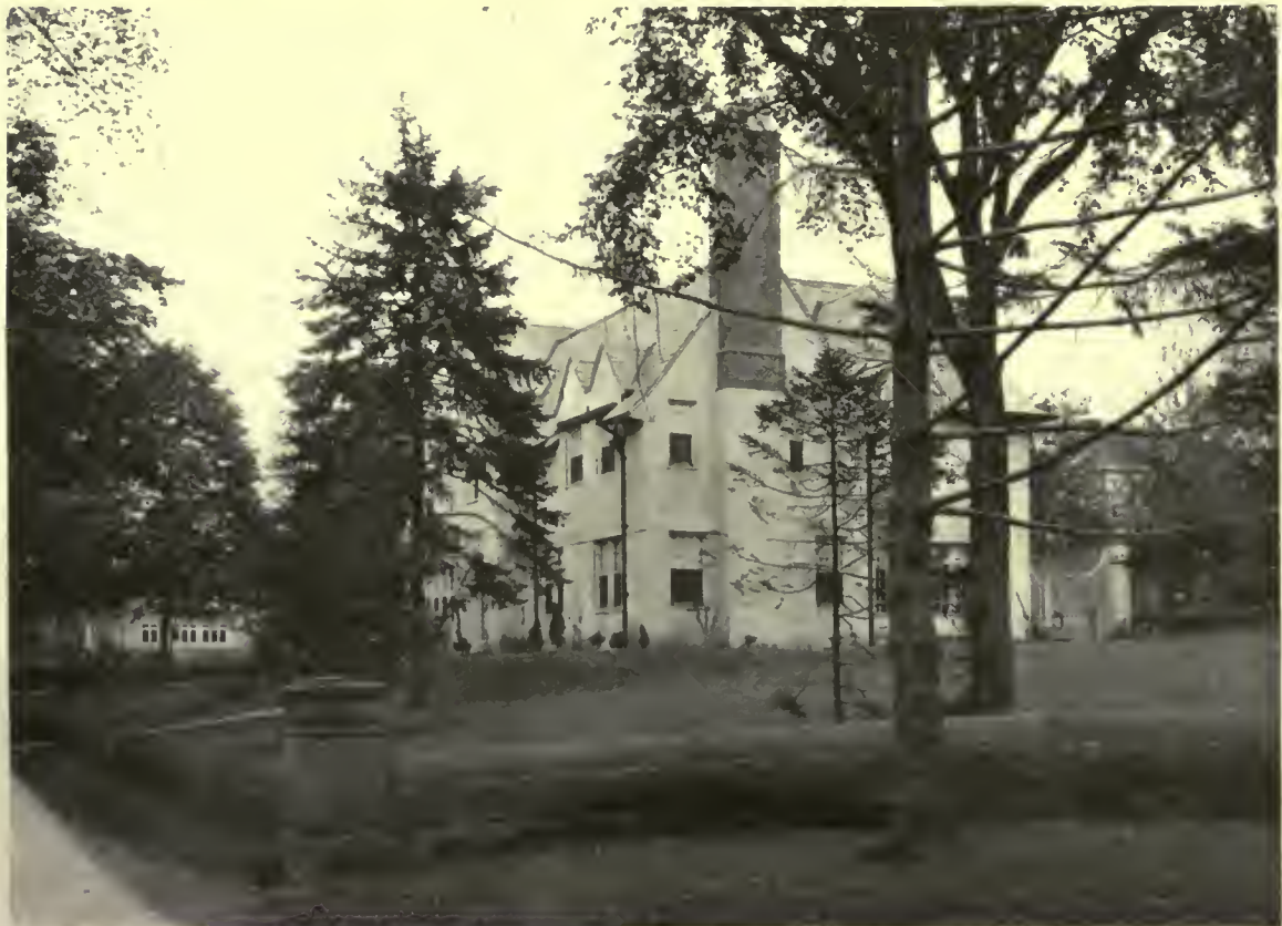
HOUSE OF B. D. BENSON, PASSAIC, N. J. JOHN F. JACKSON, ARCHITECT
