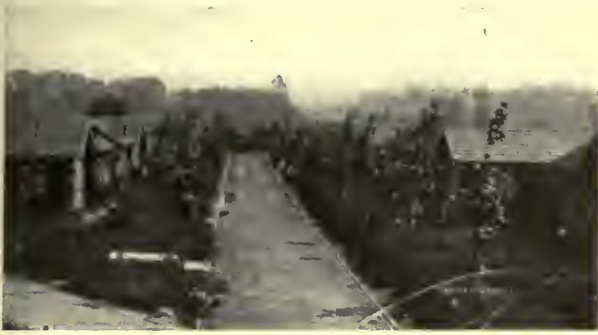
A RECONSTRUCTED CITÉ IN THE MARNE, BUILT BEFORE THE ARMISTICE BY THE SOCIÉTÉ DES AMIS. BRICKS WERE AVAILABLE FOR THIS SCHEME
