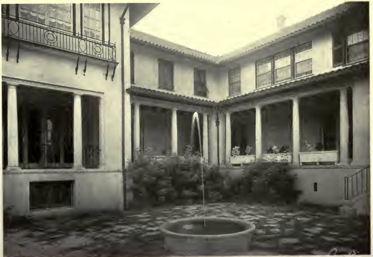
VIEW IN COURT HOUSE OF MRS. C. P. ADAMS, DALLAS, TEXAS H. B. THOMSON, ARCHITECT
