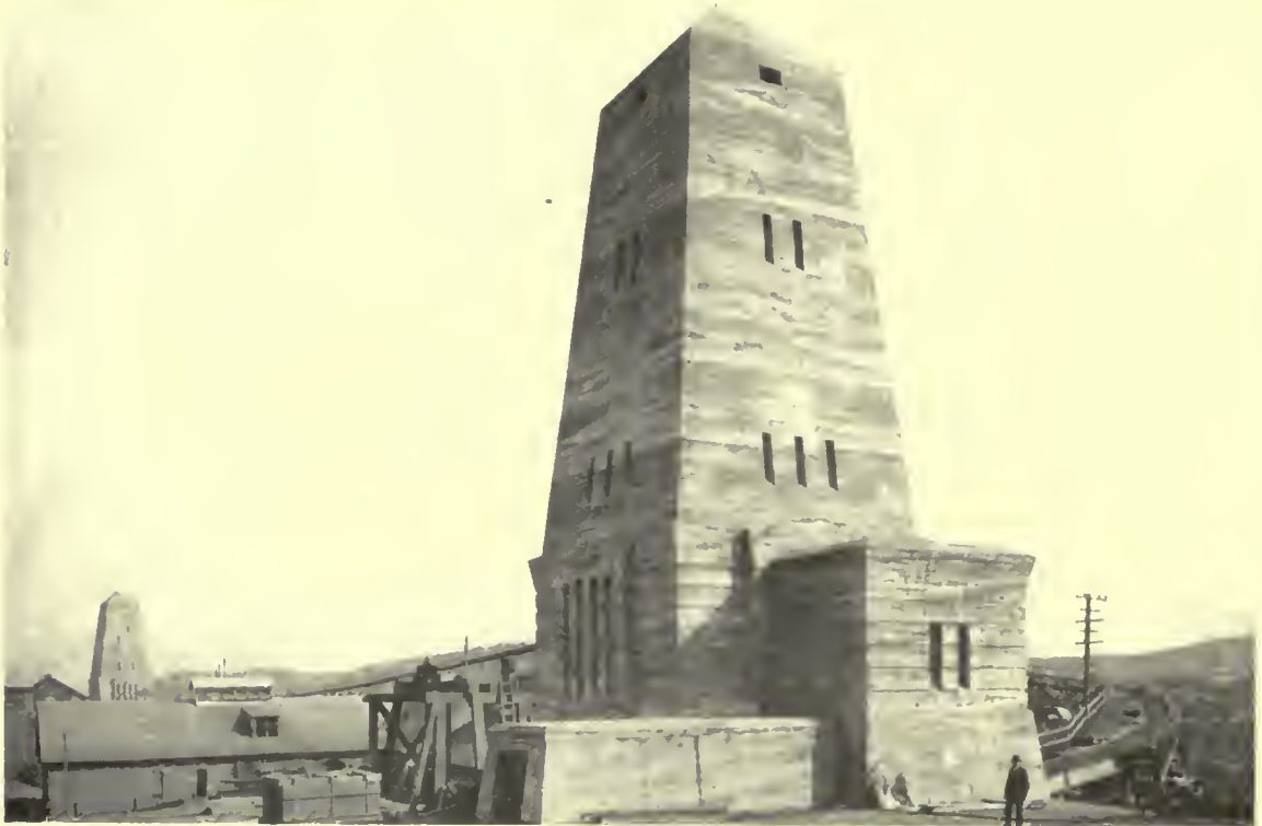
SHAFT HOUSE B. HOUSE A IN DISTANCE
