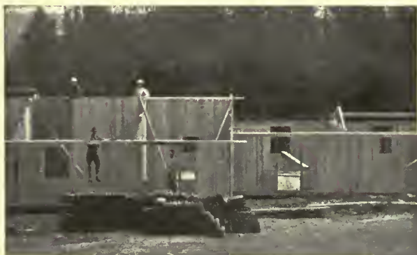
READY FOR THE ROOF—SECTION BARRACKS FOR REHOUSING IN THE "REGION LIBEREE"
