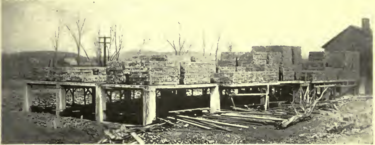
TEST SLAB UNDER FINAL LOAD
