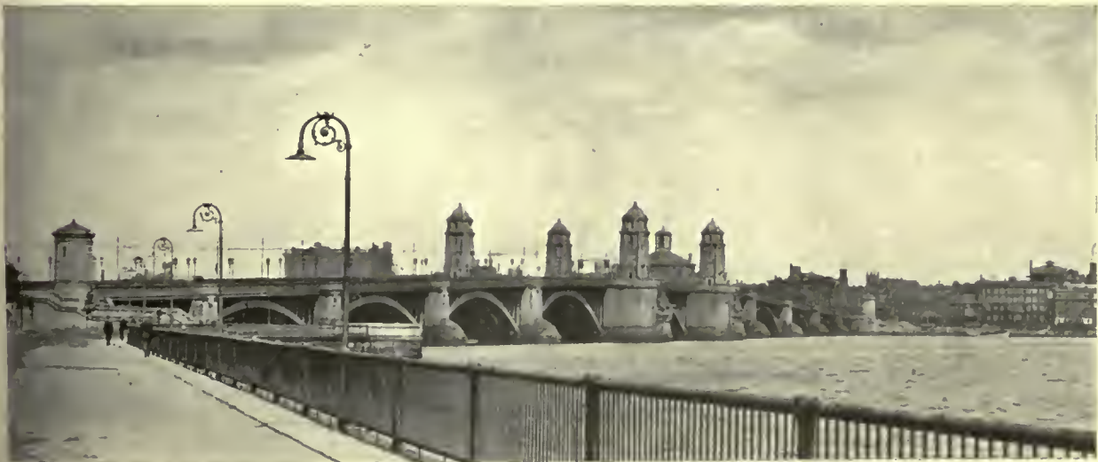
THE WEST BOSTON BRIDGE
