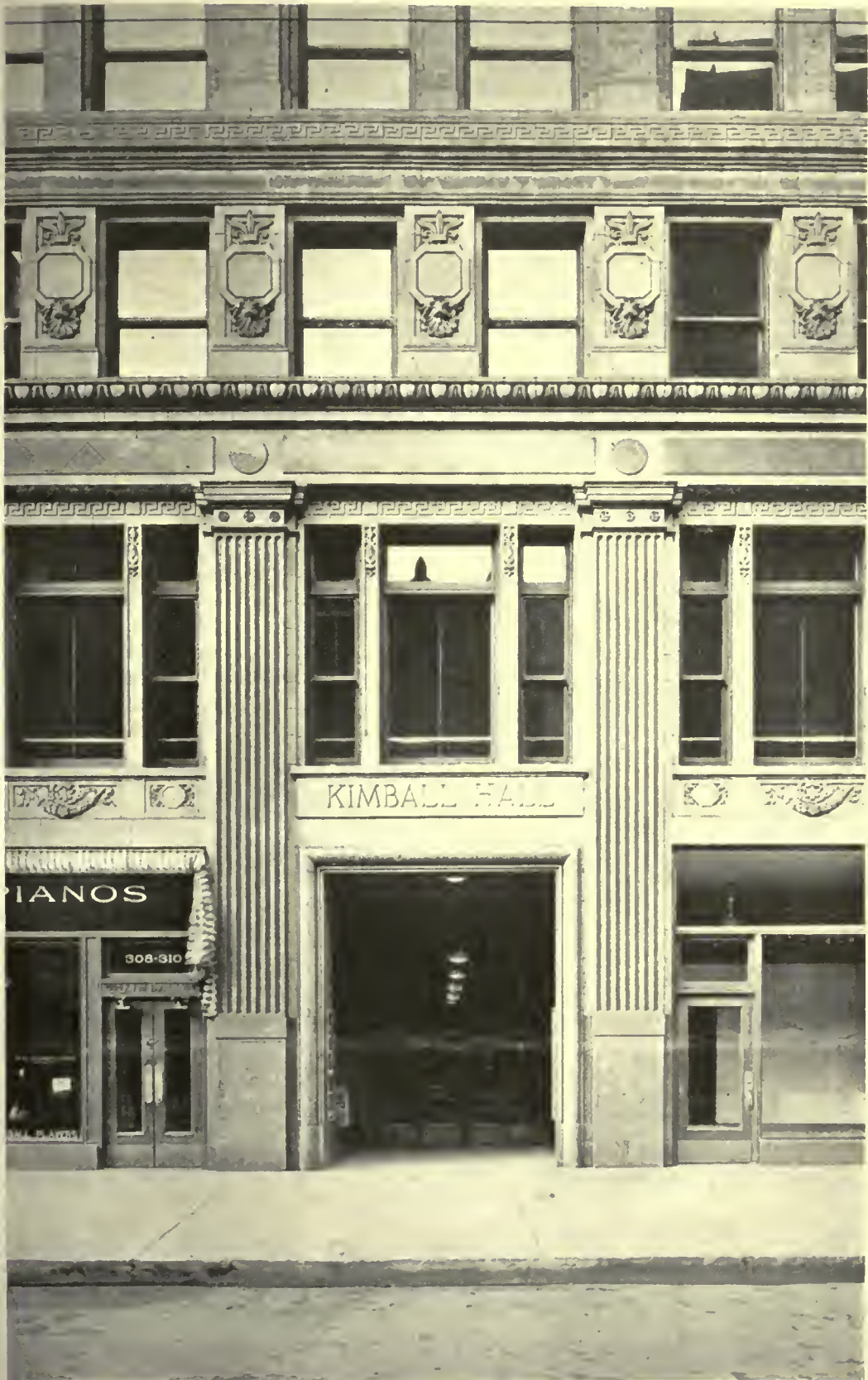
DETAIL OF LOWER STORES KIMBALL HALL BUILDING, CHICAGO, ILL. GRAHAM, ANDERSON, PROBST & WHITE, ARCHITECTS
