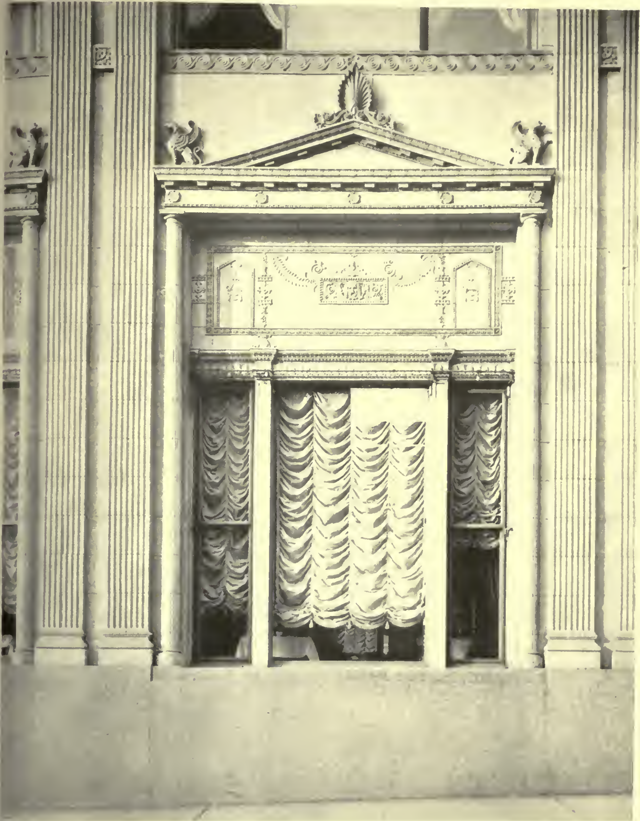
EXTERIOR DETAIL OF FIRST STORY HOTEL DESHLER, COLUMBUS, OHIO HOLABIRD & ROCHE, ARCHITECTS
