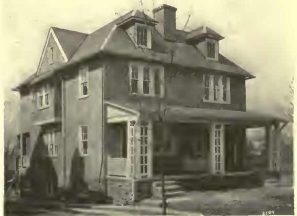
FIG. 7. OUTSIDE STUCCO WORK IN PLACE. BUILDING COMPLETED.
