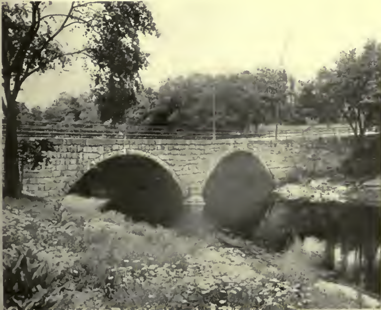
GREEN STREET BRIDGE, IPSWICH, MASS.
