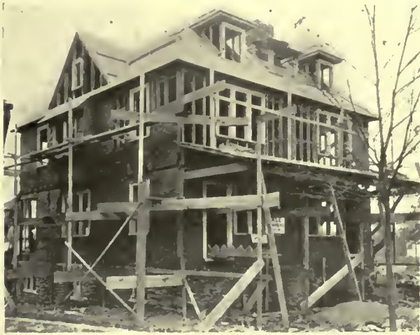
FIG. 5. TIMBER FRAMEWORK COMPLETE
