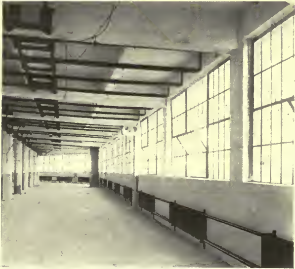
FACTORY BUILDING—THOMAS A. EDISON, INC., ORANGE, N. J. Wall radiators used throughout
