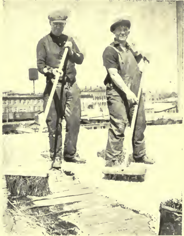
PLACING FELT, TAR AND SLAG ROOF OVER CONCRETE SLABS
