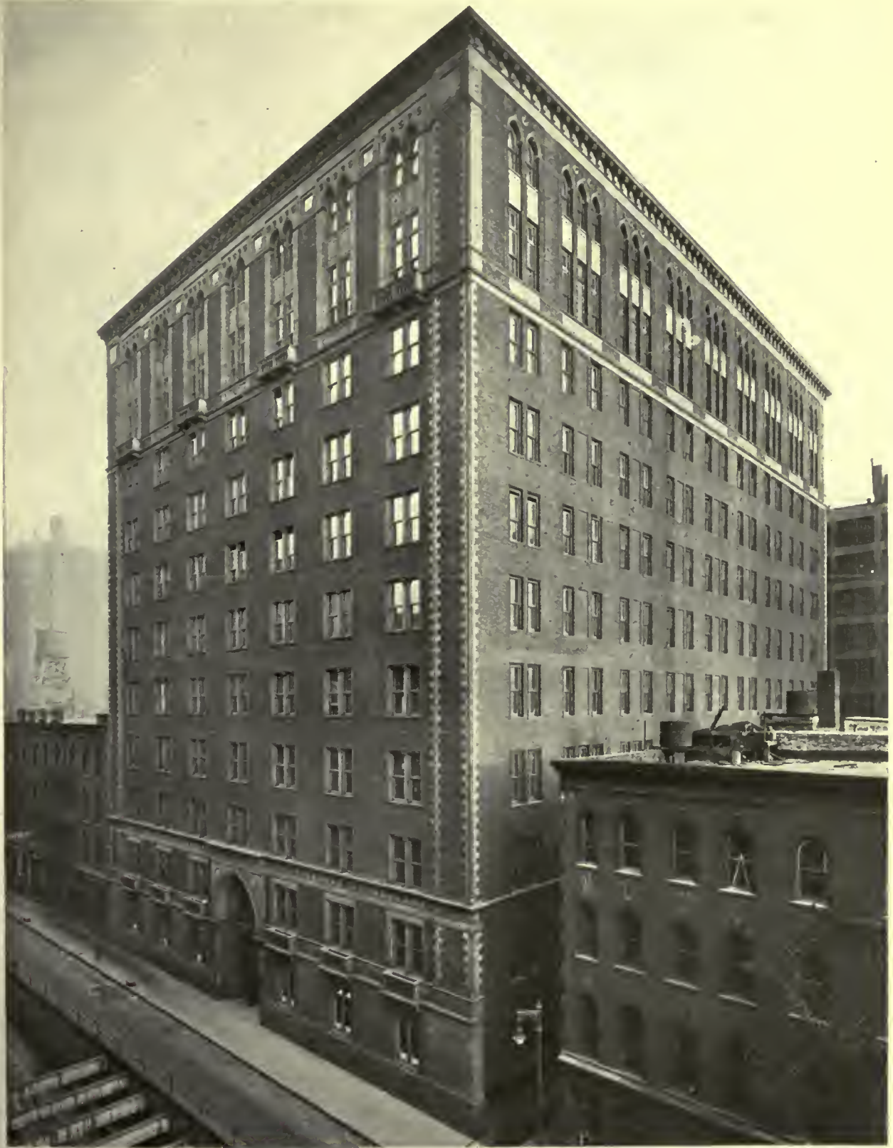
FRANKLIN EXCHANGE, CHICAGO TELEPHONE COMPANY HOLABIRD & ROCHE, ARCHITECTS
