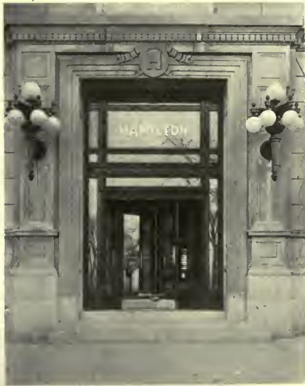
AN APARTMENT HOUSE INSTALLATION
