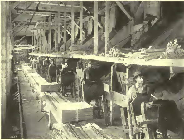
FIG. 6. THE SHINGLES ARE BUNDLED AND CONVEYED TO FREIGHT CARS
