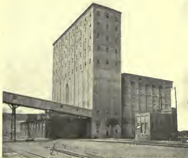
CONCRETE GRAIN ELEVATOR WITH CAPACITY OF 1,000,000 BUSHELS
