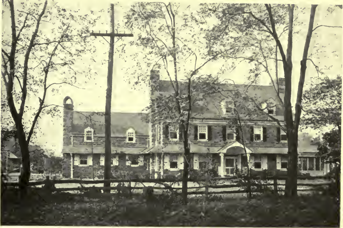
HOUSE OF ROYAL F. HAMMETT, GERMANTOWN, PA. CARL A. ZIEGLER, ARCHITECT
