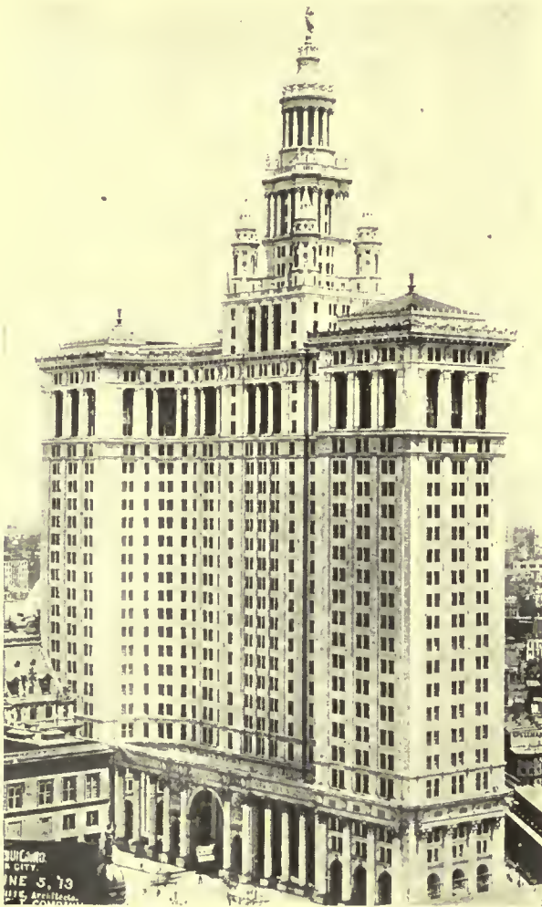
WEST ELEVATION, MUNICIPAL BUILDING, NEW YORK CITY
