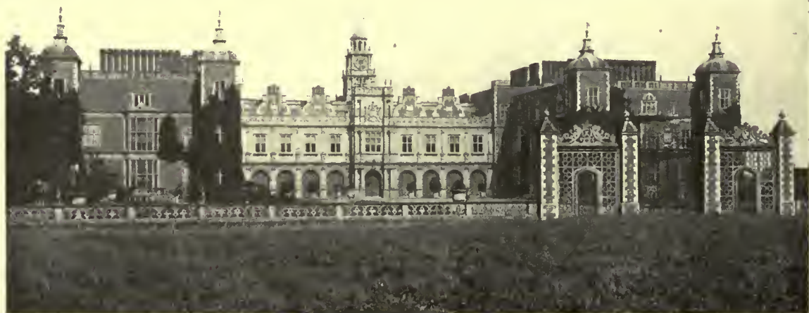
SOUTH FRONT, HALFIELD HOUSE, HERTS, ENGLAND
