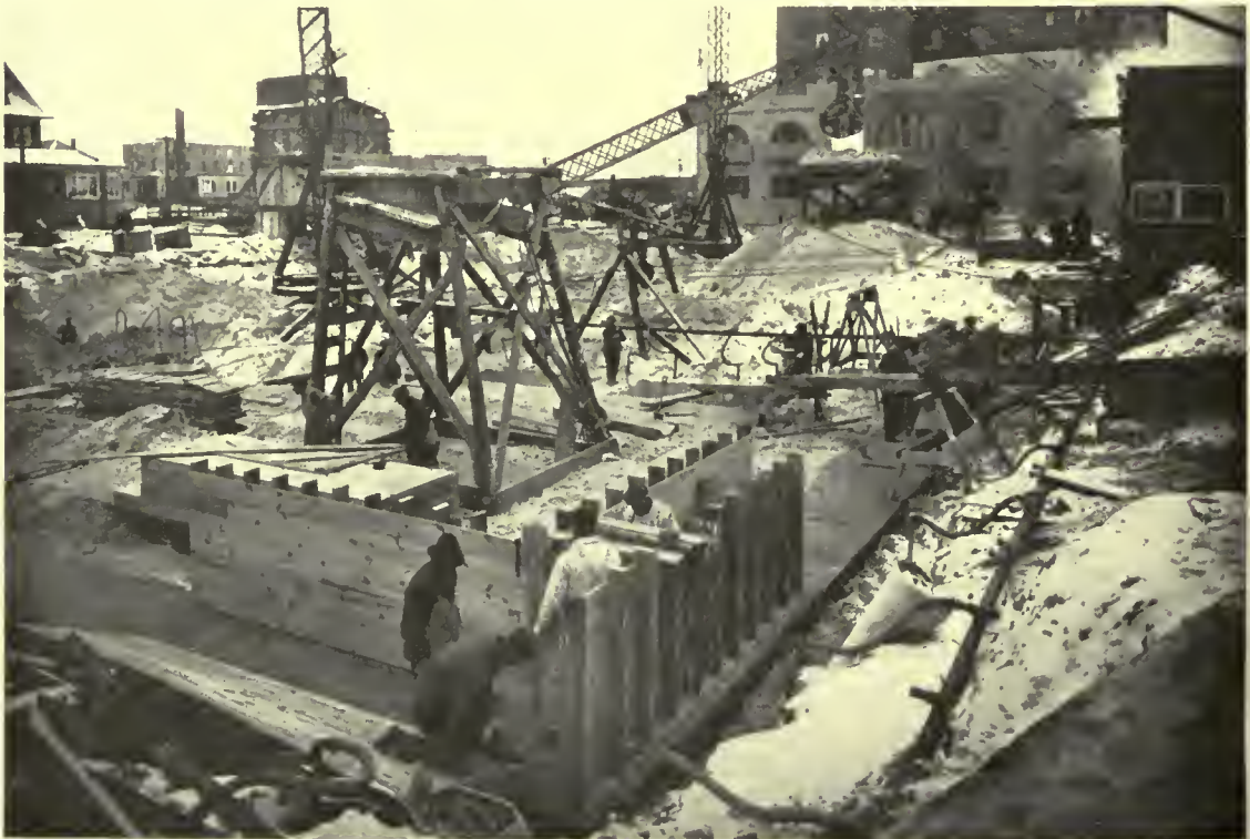
WALL FOOTINGS IN PLACE. SETTING FORMS FOR CONCRETE BASEMENT WALLS
