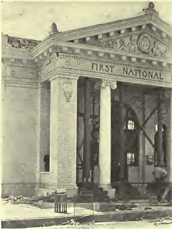
VIEW SHOWING SHORING OF PORTICO OF FIRST NATIONAL BANK BUILDING.
