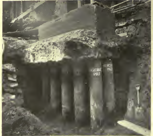
GROUP OF TUBULAR PILES PARTIALLY EXPOSED
