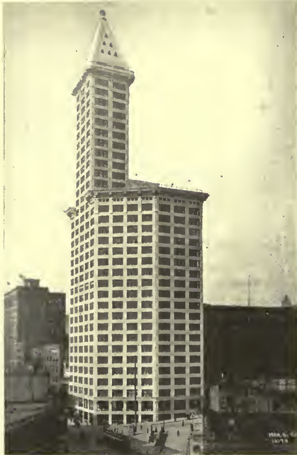
THE L. C. SMITH BUILDING, SEATTLE, WASH. GAGGIN & GAGGIN, ARCHITECTS This building, 40 stories to top of tower, is the tallest structure supported by a pile foundation
