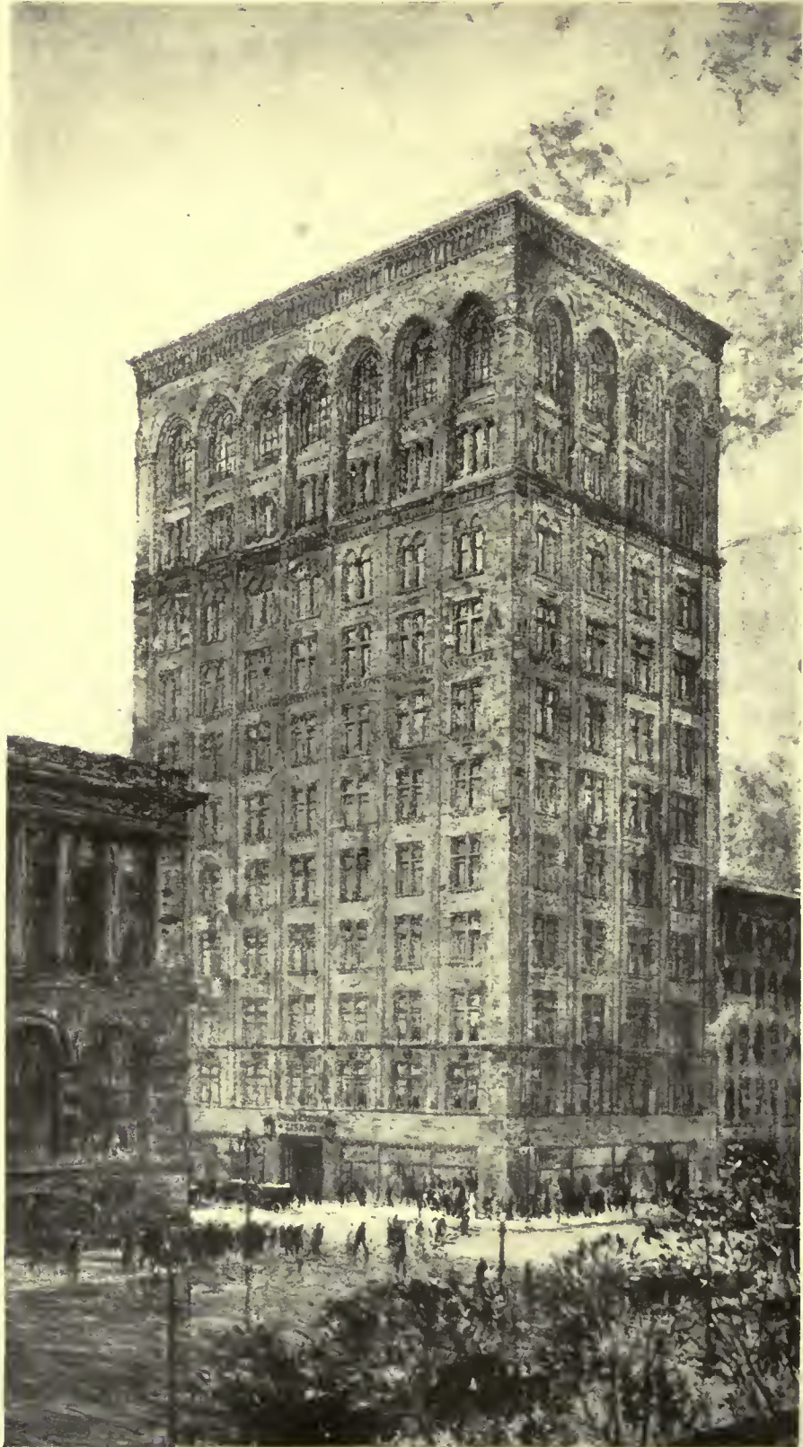
THE JOHN CRERAR LIBRARY, CHICAGO, ILLINOIS HOLABIRD & ROCHE, ARCHITECTS.
