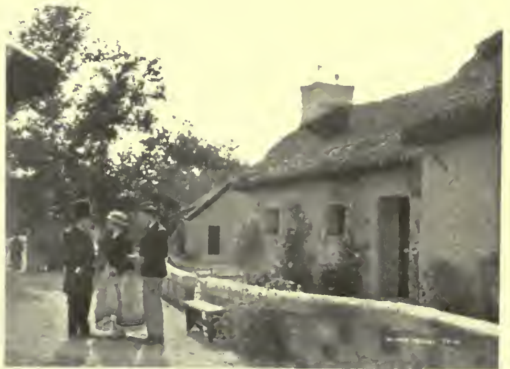
THE MODERN MOVING PICTURE "SET" IS AS STRUCTURAL IN ITS PRODUCTION AS A PRACTICAL BUILDING
