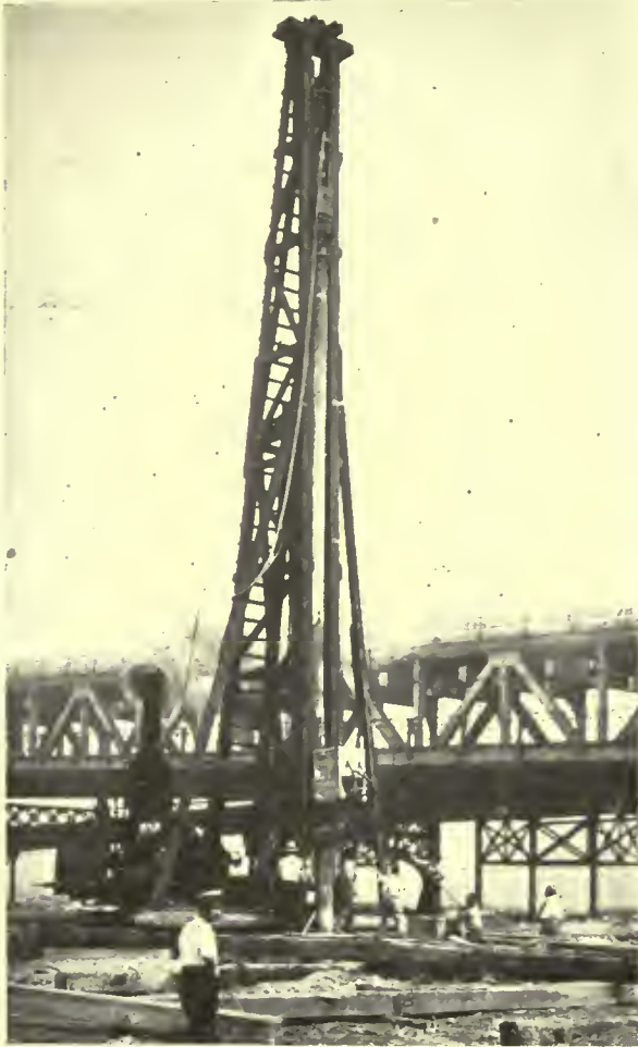
APPARATUS USED IN DRIVING PEDESTAL PILES
