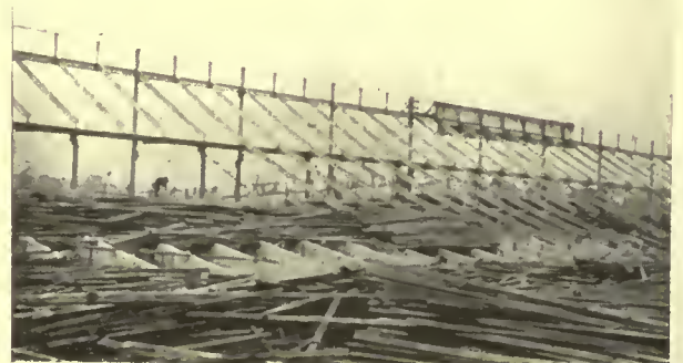
A VIEW OF THE TWO-MILE TRACK, WITH TIMBER SURFACE REMOVED
