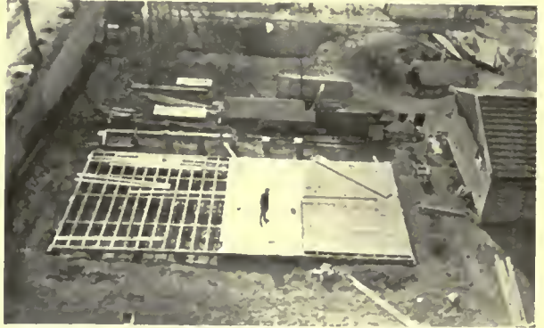
THE BEGINNING OF A BARRACK, CHALONS
