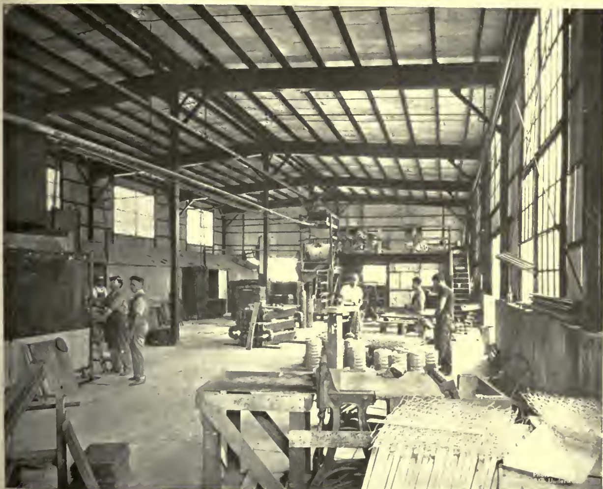
INTERIOR VIEW OF PLANT SHOWING WALL AND ROOF CONSTRUCTION
