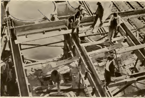
VIEW LOOKING DOWN. DOUBLE WALL CONSTRUCTION CAN BE CLEARLY SEEN
