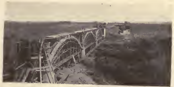
CONSTRUCTION OF CONCRETE BRIDGE
