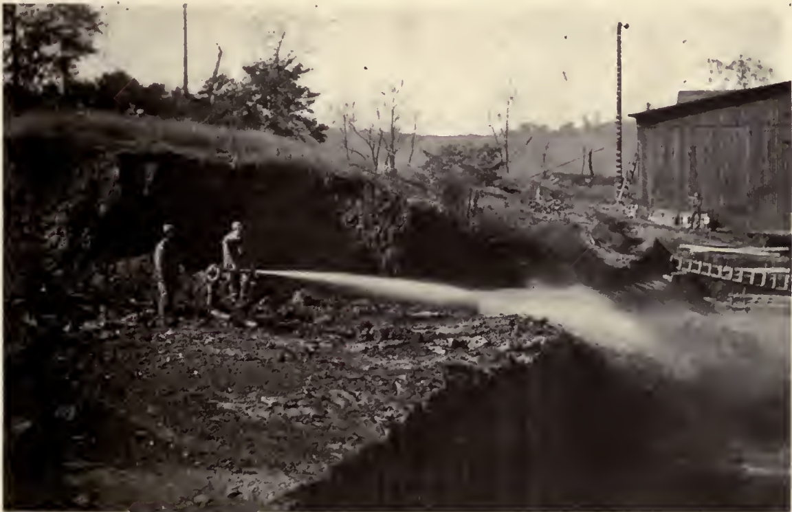
HYDRAULIC STRIPPING IN QUARRY
