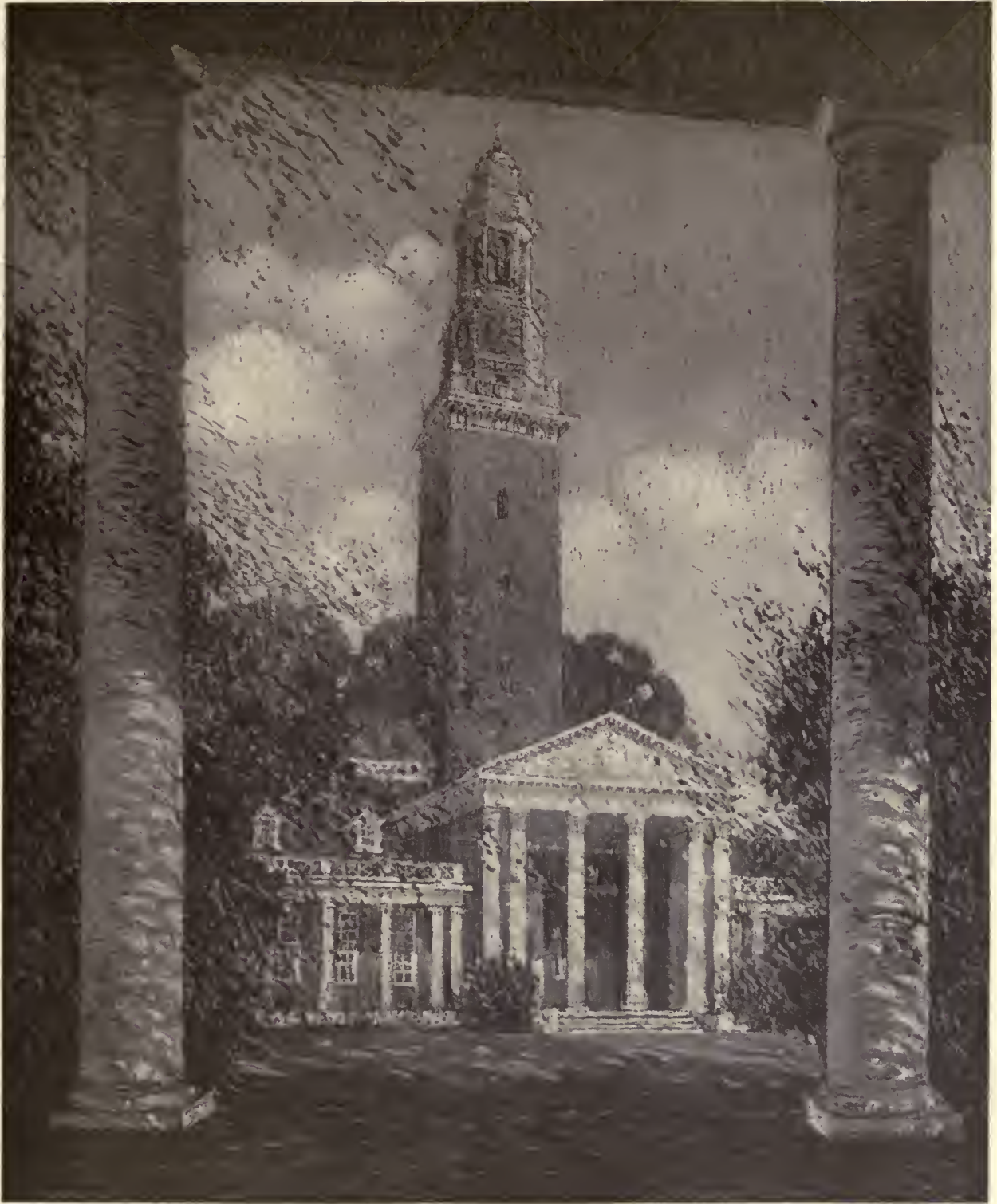
MEMORIAL TOWER, HOTCHKISS SCHOOL, LAKEVILLE, CONNECTICUT CASS GILBERT, ARCHITECT
