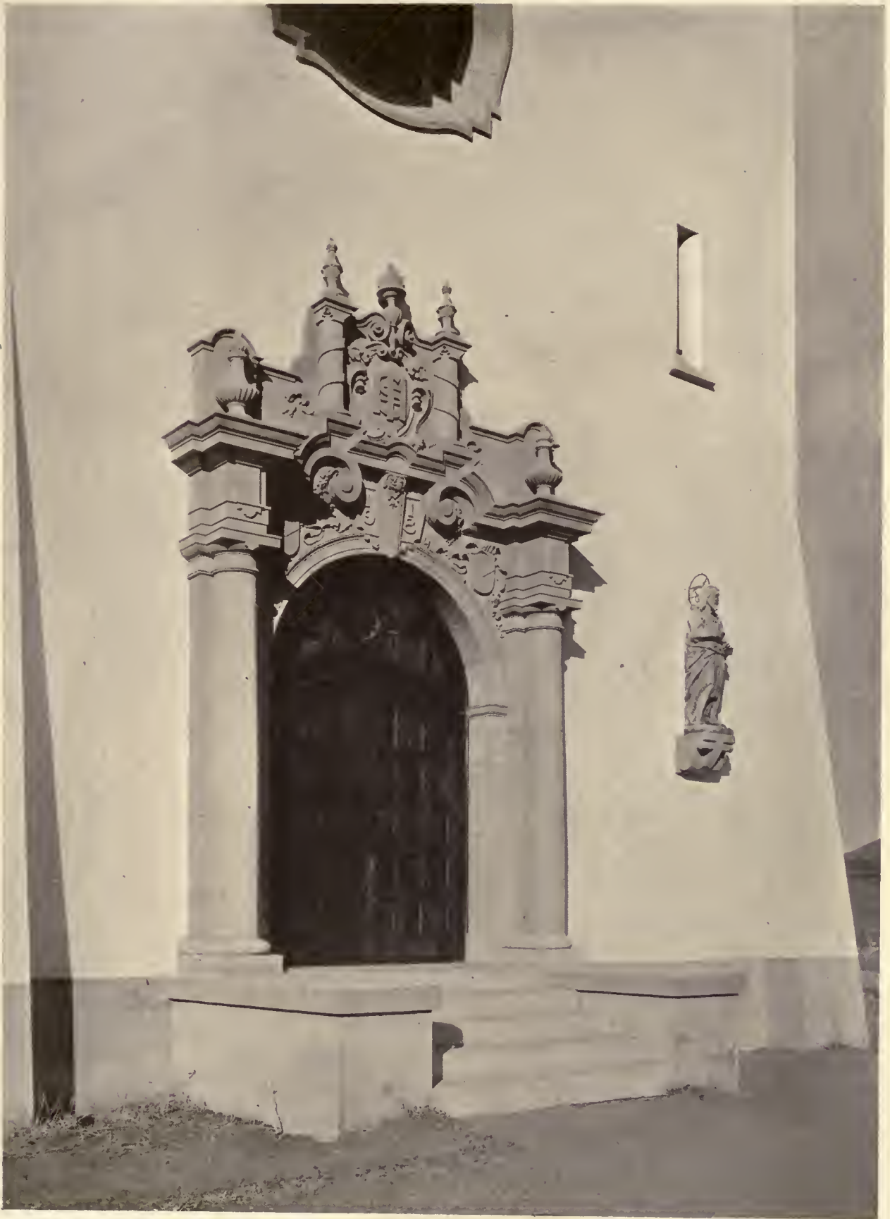
DETAIL MAIN DOORWAY ROMAN CATHOLIC CHAPEL, COLORADO SPRINGS, COLO. MacLAREN & HETHERINGTON, ARCHITECTS
