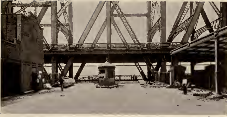
VIEW LOOKING FROM TRAFFIC CONCOURSE ON ROOF OF STOREHOUSE BUILDING TOWARDS BRIDGE. GUARDHOUSE SEEN IN CENTER
