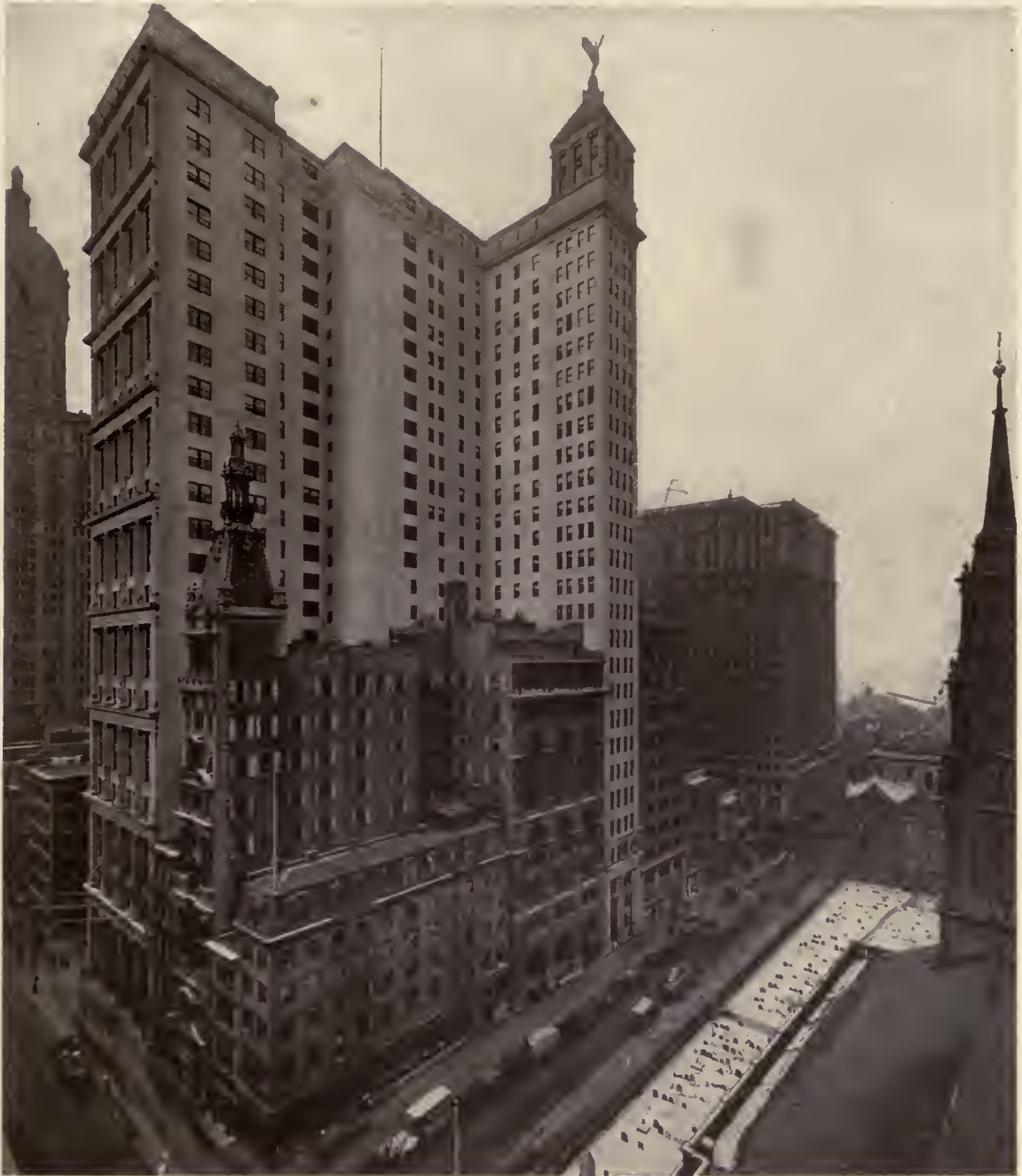
VIEW SHOWING PRESENT CONDITIONS
