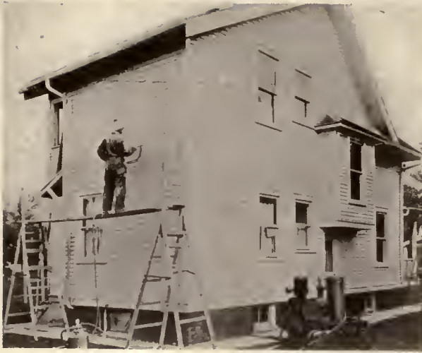
SPRAYING METHOD APPLIED TO SPRING HOUSE PAINTING
