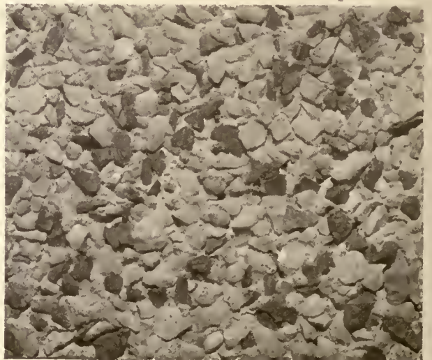
DASH FINISH USED WITH MAGNESITE STUCCO
