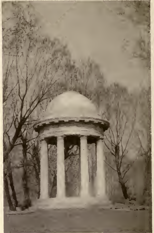
TEMPLE OF LOVE, CAST STONE. DOME IS MADE MONOLITHIC BY SETTING EIGHT RIBS AND PANELS AGAINST CROWN AND FORMING REINFORCED CONCRETE COVERING. ROSEMONT, PENNA.
