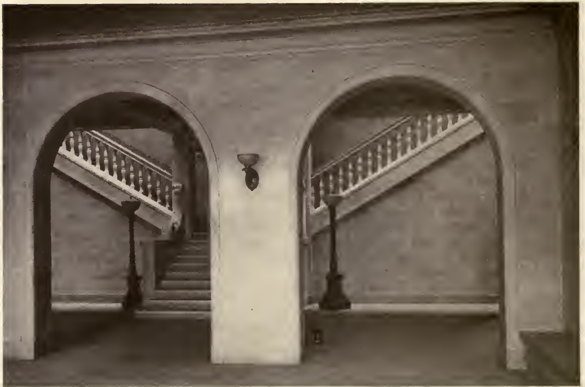
VIEW OF GROUND FLOOR LOBBY FROM THE VESTIBULE PREBLE COUNTY COURT HOUSE, EATON, OHIO H. H. HIESTAND AND RICHARDS, McCARTY & BULFORD, ASSOCIATED ARCHITECTS
