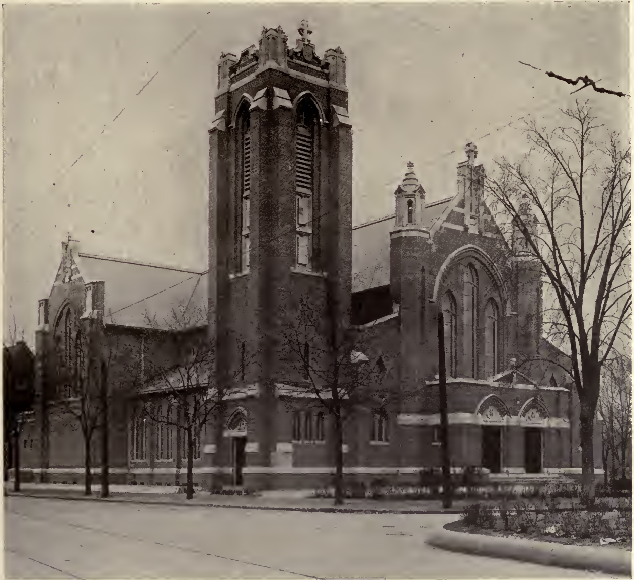
ST. STEPHEN'S CHURCH, WORCESTER, MASS.
