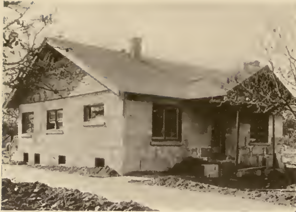
THE DOUBLE WALLED BUNGALOW READY FOR STUCCO FINISH
