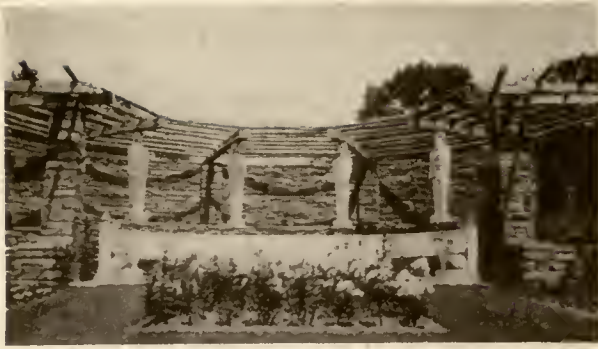
EXEDRA SEAT, 25-FOOT RADIUS "FOUR SEASONS" SUPPORTS IN CAST STONE. ROSEMONT, PENNA.
