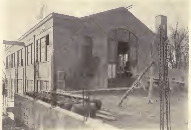
REAR ELEVATION. NOTE HOISTING BEAM AND LARGE OPENING OF OPERATING ROOM FOR PLACING EQUIPMENT
