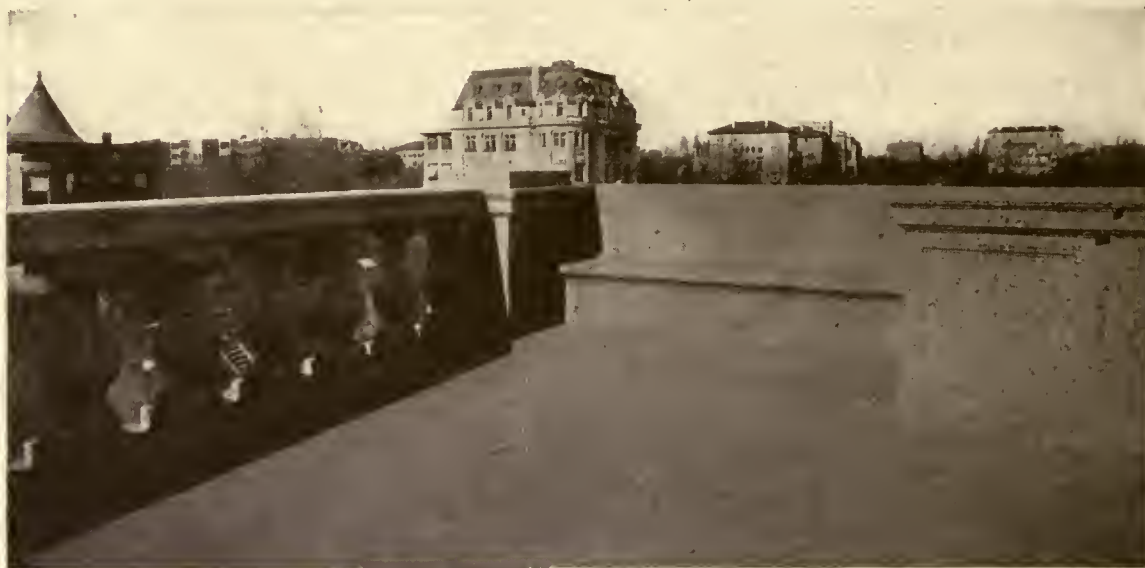
FIG. 1. PRECAST CONCRETE WORK AT MERIDIAN HILL PARK
