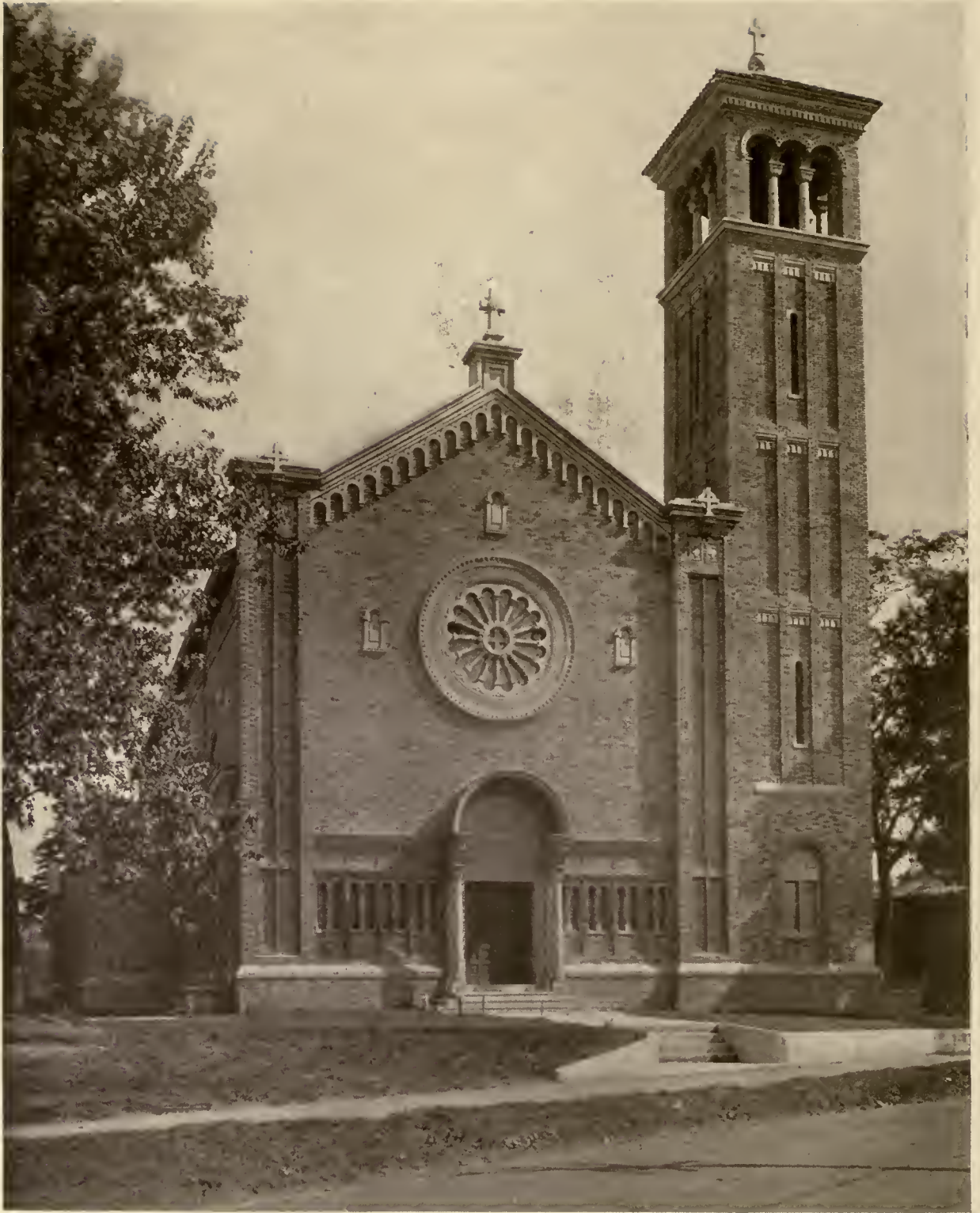
ST. JOHN'S CHURCH, NORTHAMPTON, MASS. JNO. WM. DONOHUE, ARCHITECT
