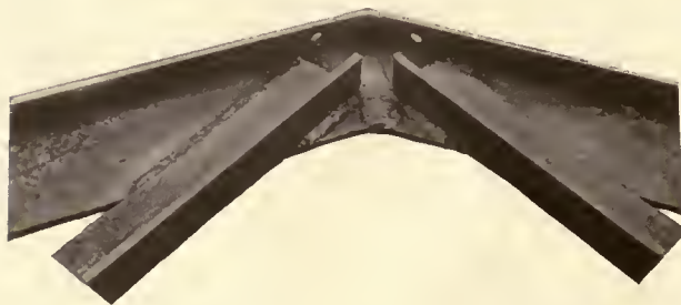
WELDED CONNECTION AT PEAK OF TRUSS
