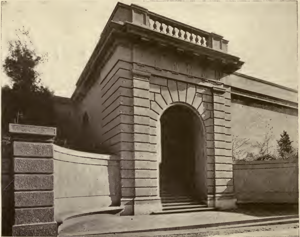
FIG. 4. ENTRANCE TO MERIDIAN HILL PARK, WASHINGTON, D. C., SHOWING EXPOSED AGGREGATE SURFACES
