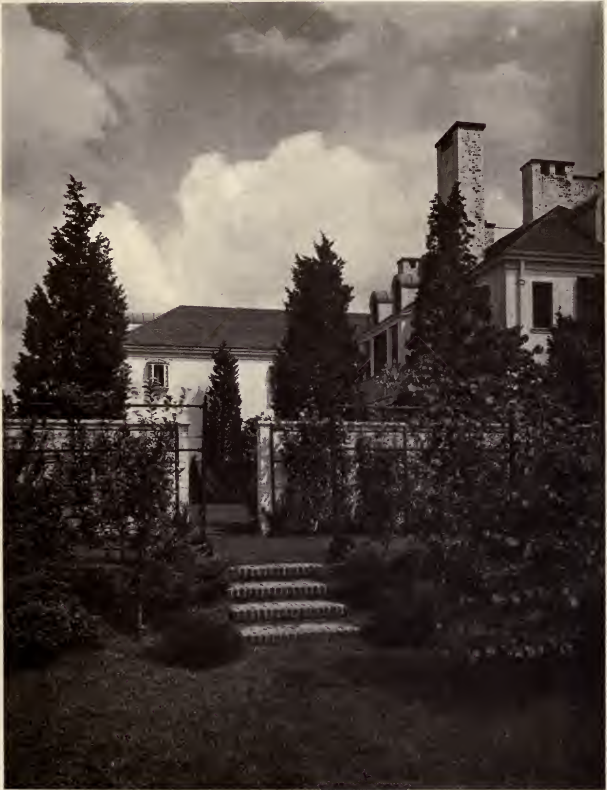
HOUSE OF ROBERT L. BACON, JR., AT WESTBURY, L. I. JOHN RUSSELL POPE, ARCHITECT
