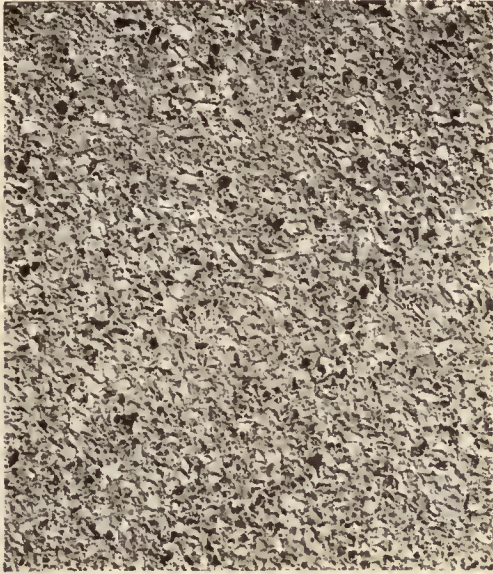
FIG. 2. A CLOSE-UP VIEW OF CONCRETE SURFACES BY EARLEY-PEARSON METHODS
