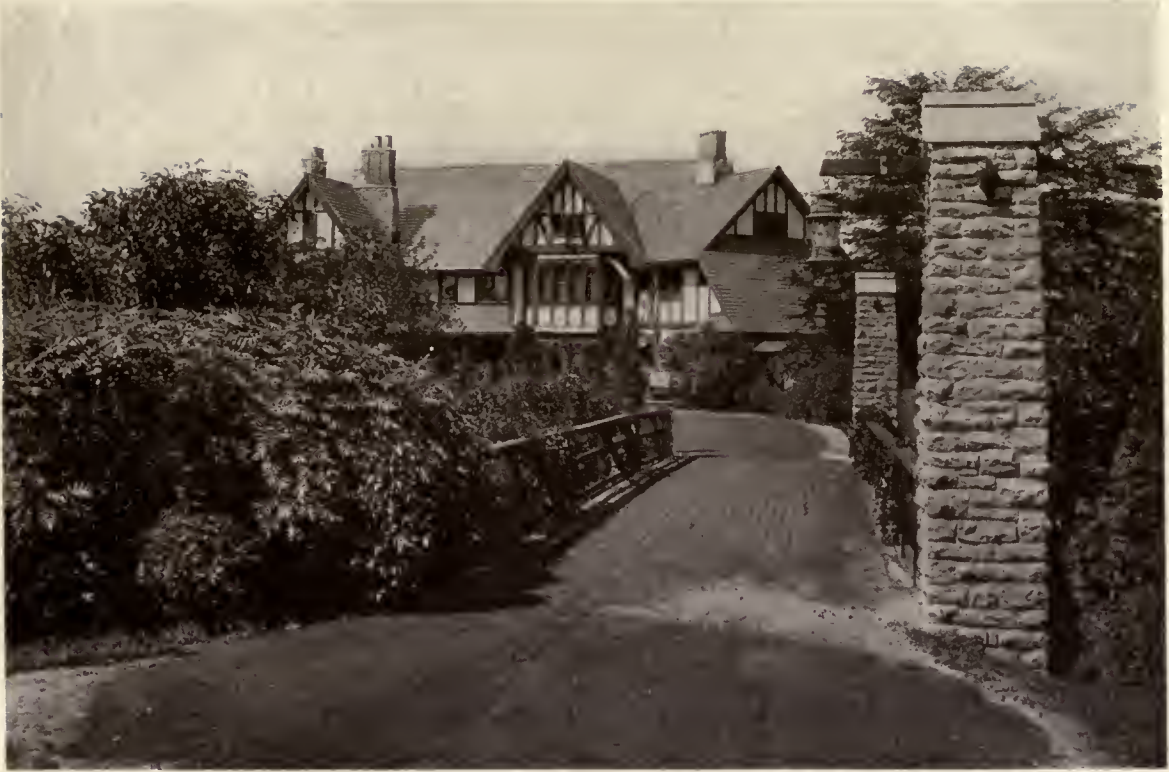
ENTRANCE DRIVEWAY, ESTATE OF WILLIAM S. WALBRIDGE, TOLEDO O.
