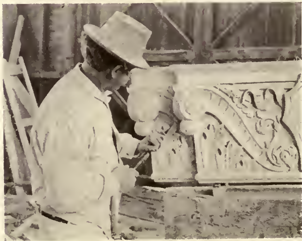
CARVING PILASTER CAPITOL. CARVER IS USING AIR-HAMMER
