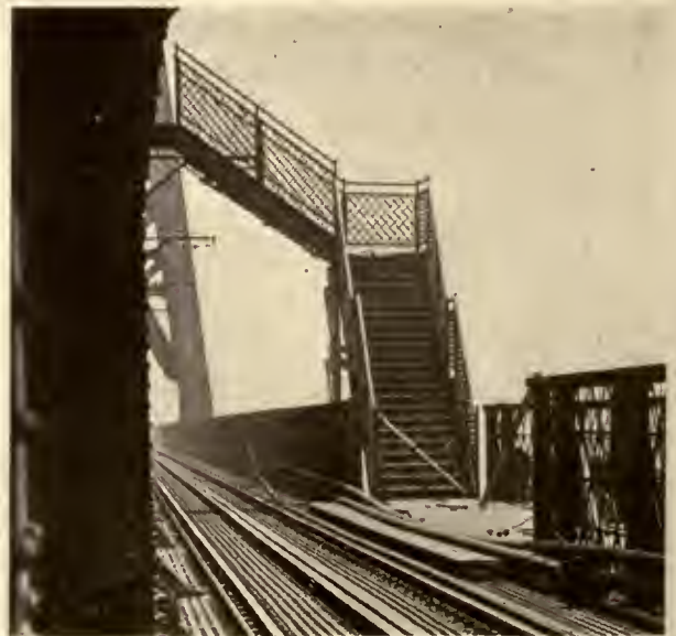
STAIRWAY ON SOUTHERLY SIDE FROM PROMENADE LEVEL, AND CONNECTING WITH HANGING BRIDGE BELOW TRACK LEVEL, BY WHICH ACCESS TO BUILDING IS HAD
