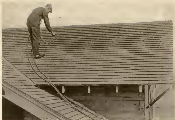
SPRAY PAINTING A SHINGLE ROOF Such surfaces often prove difficult for brush work
