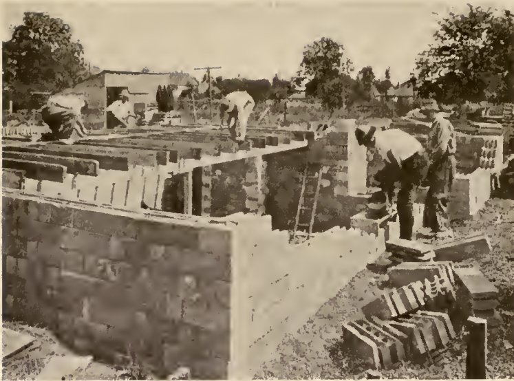
WALLS BEING CONSTRUCTED OF THE INTERLOCKING TYPE OF CONCRETE BLOCK
