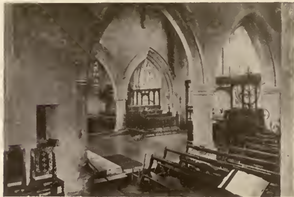
VIEW ACROSS CHANCEL, PARISH CHURCH AT CIRENCESTER
