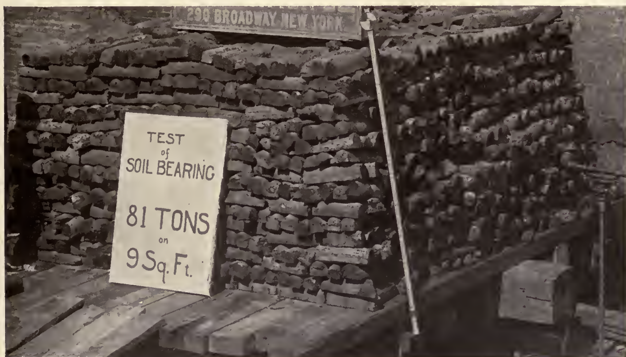
TESTING THE SOIL
