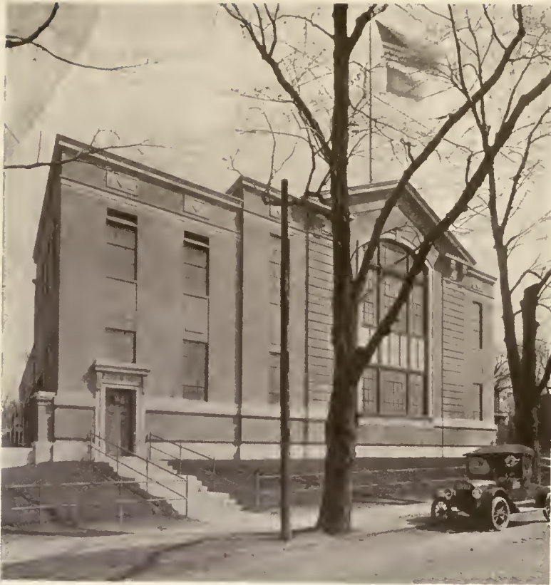
FRONT ELEVATION, FLUSHING SUB-STATION, N. Y. & QUEENS ELECTRIC LIGHT & POWER CO. WILLIAM W. KNOWLES, ARCHITECT
