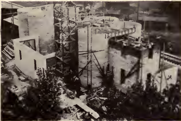
DOUBLE WALLS BUILT IN SUCCESSIVE TIERS
