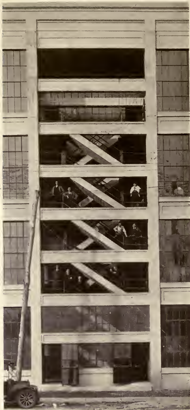
KAHN TAILORING COMPANY BUILDING, INDIANAPOLIS. A DOUBLE STAIRWAY EXIT ON STREET FRONT
