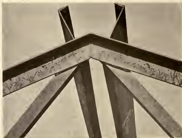
ROOF PURLINS WELDED TO TOP CHORD OF TRUSS
