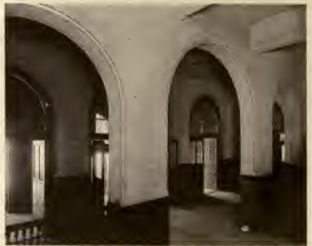
OLD FIRST FLOOR HALL AND VESTIBULE
