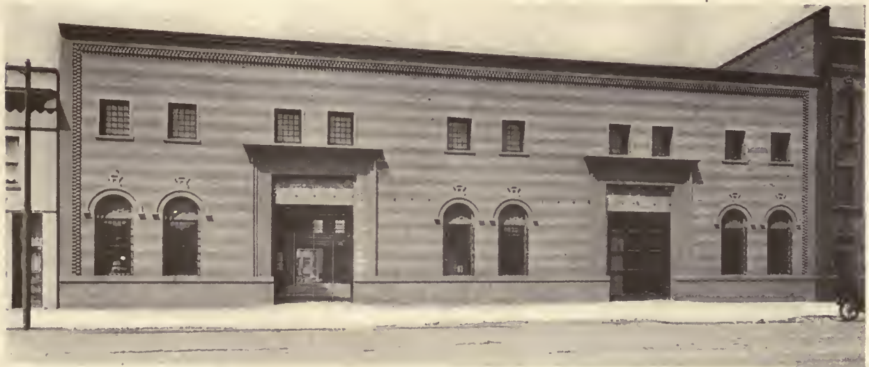
COTTAGE GROVE AVENUE ELEVATION. GARAGE FOR MANDEL BROTHERS, CHICAGO I. S. STERN, ARCHITECT. L. J. MENSCH, ENGINEER
