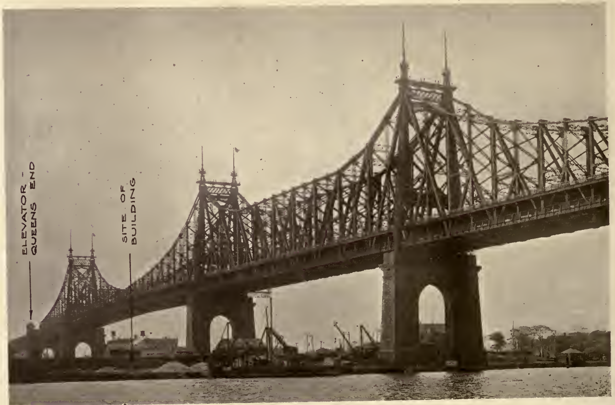
VIEW OF QUEENSBORO BRIDGE FROM MANHATTAN SIDE. THE TWO CENTER BRIDGE PIERS ON BLACKWELLS ISLAND ARE 630 FEET APART
