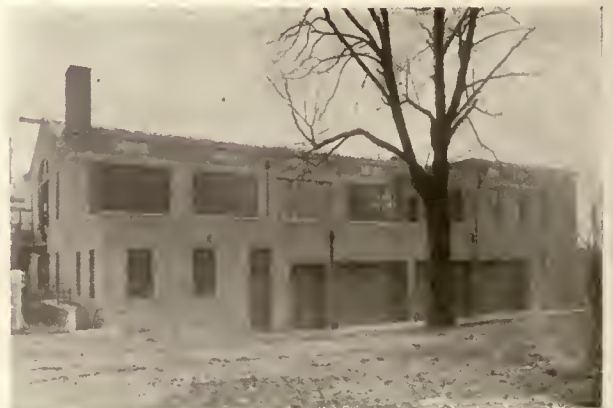
NORTH ELEVATION, SHOWING EMERGENCY TRUCK ENTRANCES
