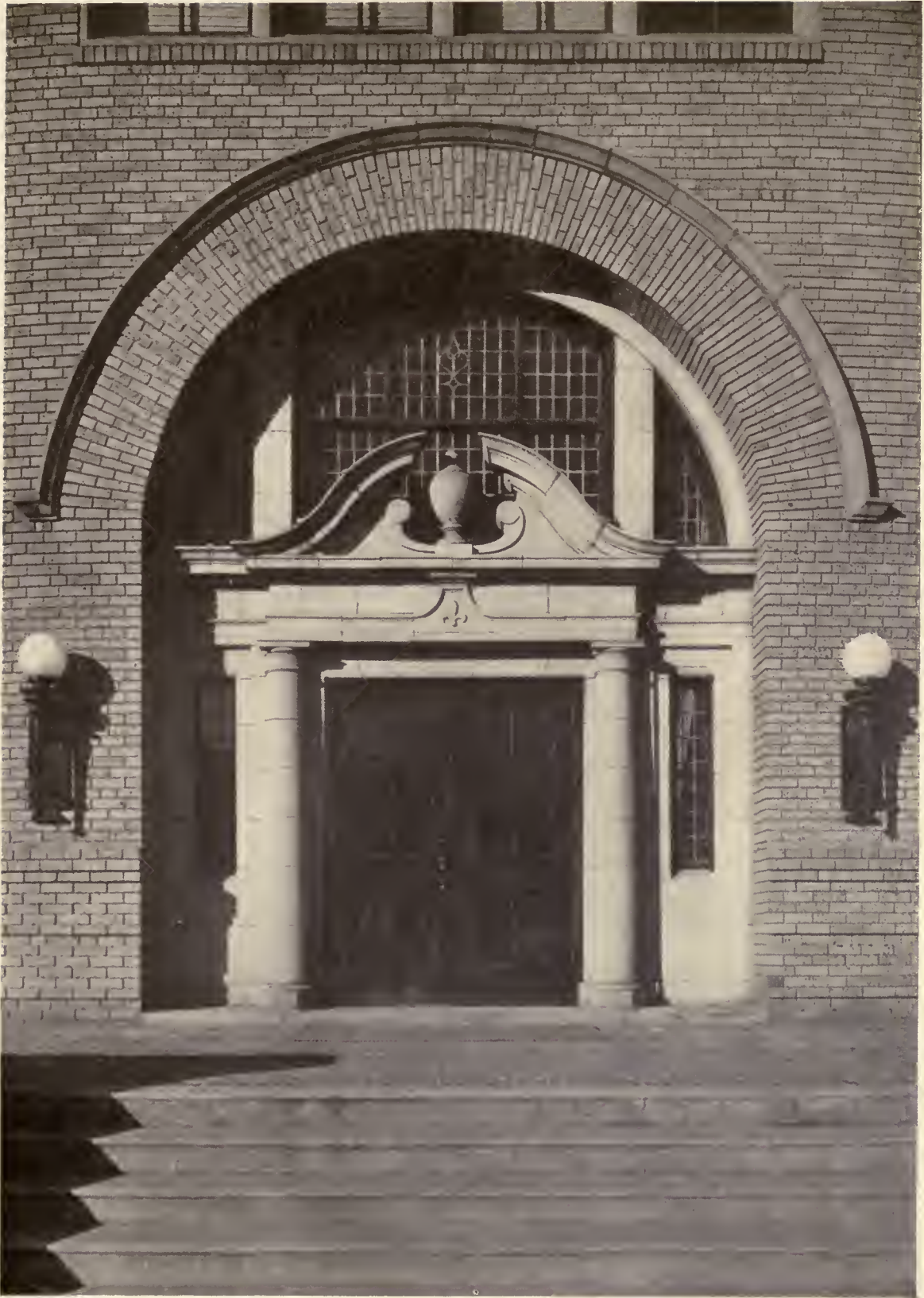
ENTRANCE DETAIL HIGH SCHOOL, DURANGO, COLORADO CHARLES E. THOMAS, ARCHITECT
