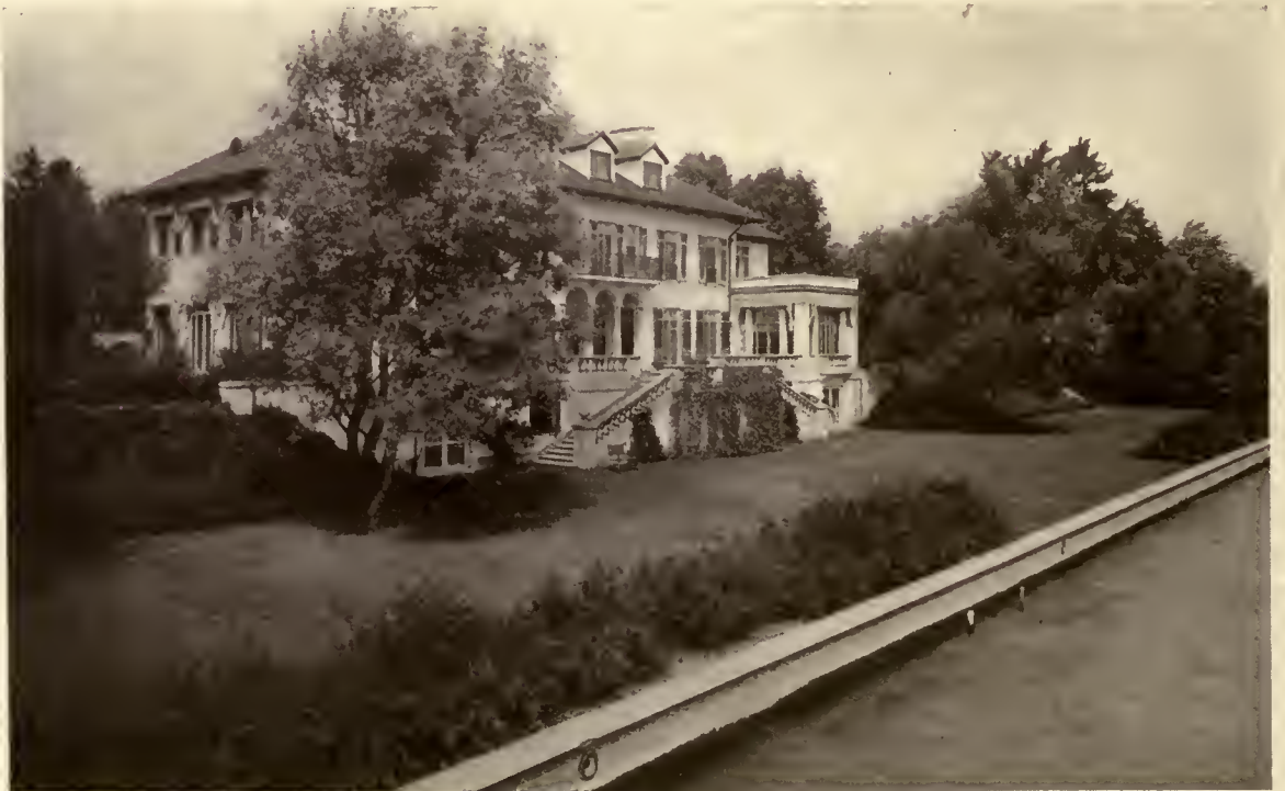
LAKEFRONT, HOUSE OF C. G. EDGAR, GROSSE POINTE, MICH. WILLIAM PITKIN, JR., LANDSCAPE ARCHITECT
