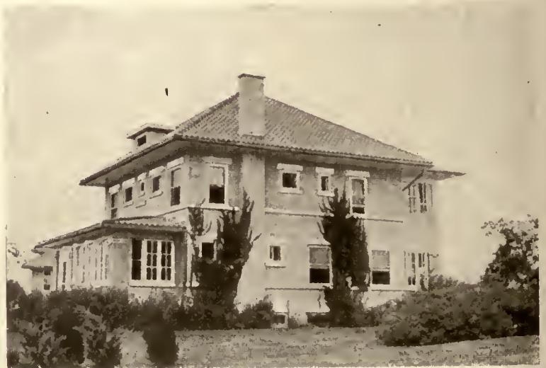
AN ATTRACTIVE HOUSE CONSTRUCTED WITH WALLS OF CONCRETE BLOCK AND STUCCO FINISH
