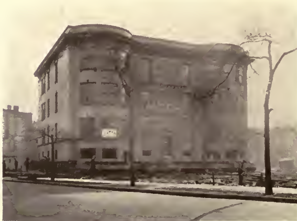
SECTION 2 TURNED ABOUT \frac{3}{4} OR 67\frac{1}{2} DEG. AND FACING N.W. NOW IN CENTER OF IRVING AVENUE. ORIGINAL POSITION IMMEDIATELY IN FRONT OF PRESENT POSITION AND FACING JACKSON BOULEVARD WHICH IS IN THE FOREGROUND
