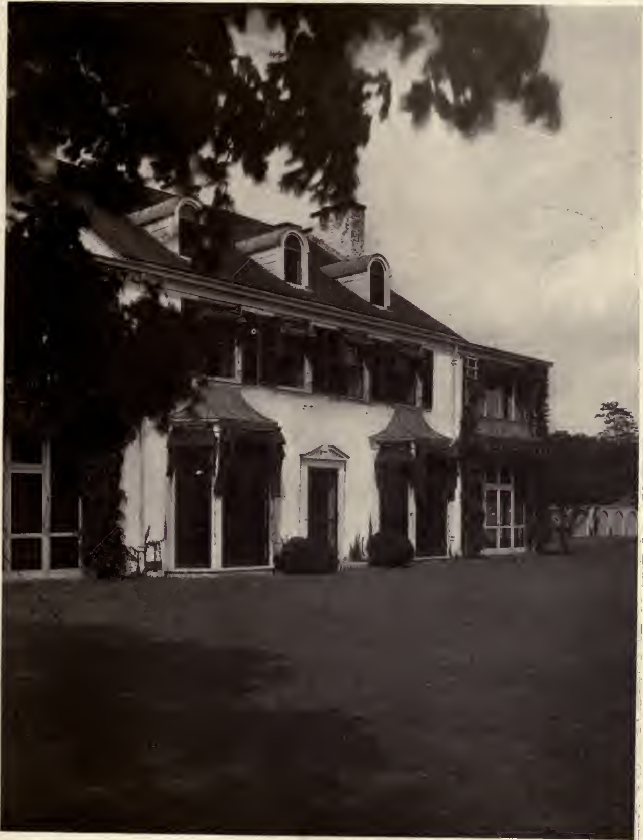
HOUSE OF ROBERT L. BACON, JR., AT WESTBURY, L. I. JOHN RUSSELL POPE, ARCHITECT
