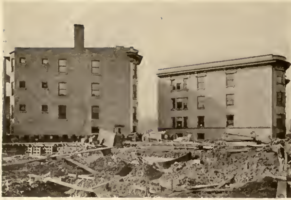
SECTION 1 TURNED ABOUT \frac{3}{4} OR 135 DEG. AND FACING N.W. SECTION 2 AT RIGHT.
