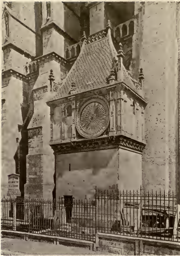
CATHEDRAL OF NOTRE DAME DE CHARTRES. CLOCK TOWER, NORTH SIDE
