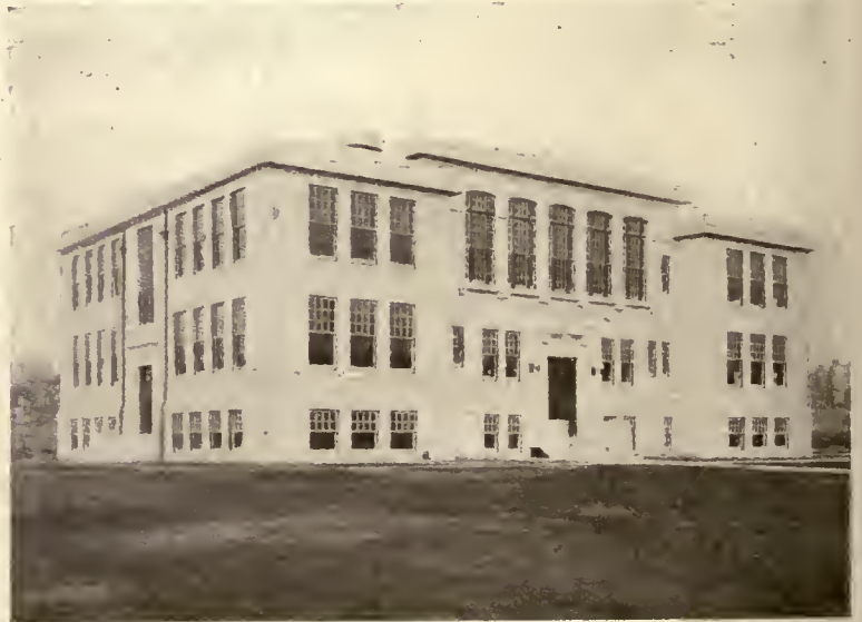
FIG. 9. REINFORCED CONCRETE SCHOOL BUILDING. NOTHING TO BURN IN CONSTRUCTION; MAINTENANCE COSTS AT A MINIMUM; DEPRECIATION NEGLIGIBLE
