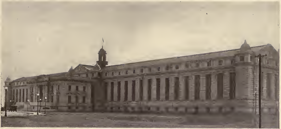
VIEW OF ADMINISTRATION AND MAIN CELL BUILDING
