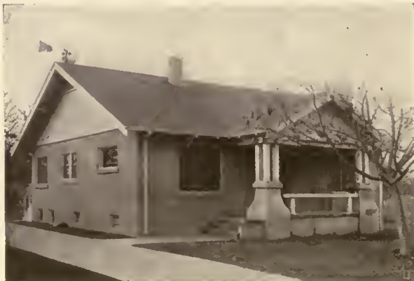
STUCCO WORK COMPLETED
