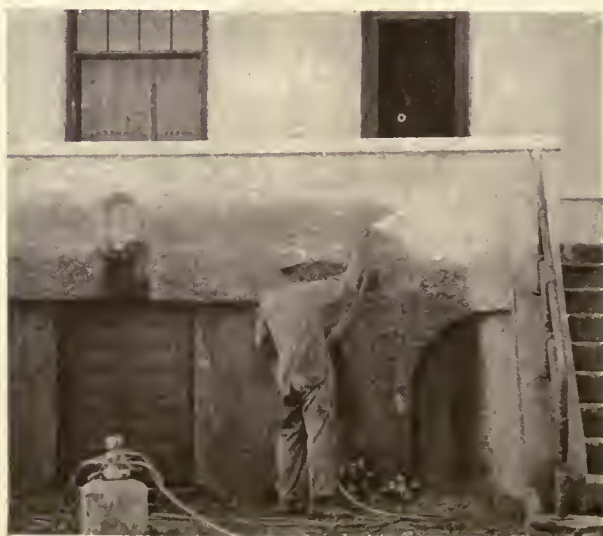
AN EXCELLENT WAY TO PAINT ROUGH CAST CEMENT STUCCO
