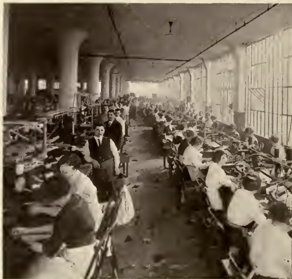
TYPICAL INTERIOR VIEW, KAHN TAILORING COMPANY BUILDING, INDIANAPOLIS. IN WORKSHOP GENERAL ARTIFICIAL ILLUMINATION IS PROVIDED, SUPPLEMENTED BY INDIVIDUAL ILLUMINATION AT THE WORK.
