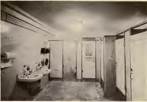
INTERIOR VIEW, PUBLIC CONVENIENCE STATION AT SCRANTON, PA.
