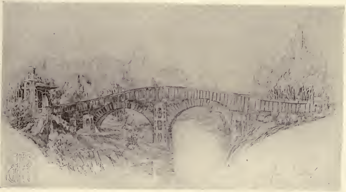
FOOT BRIDGE, BRONXVILLE, N. Y. CHARLES W. STOUGHTON, ARCHITECT
