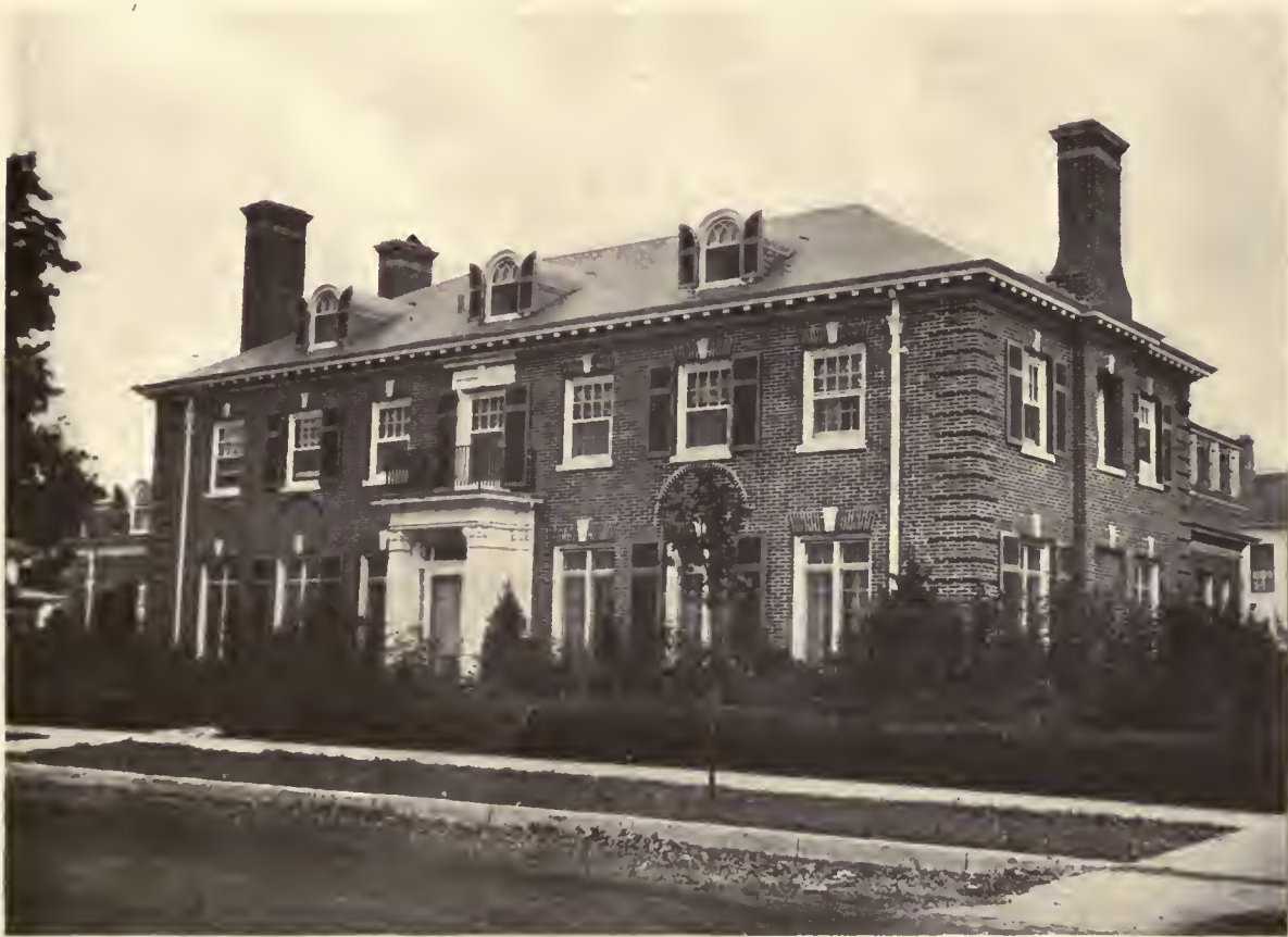
RESIDENCE OF MRS. ALICIA OATMAN, DUNDEE, ILLINOIS CHILDS & SMITH, ARCHITECTS Thirty-third Annual Joint Chicago Architectural Exhibition
