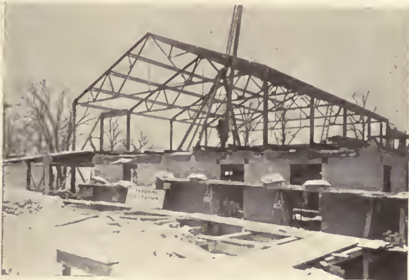
NO. 3. THREE WEEKS LATER. STEEL ERECTION COMPLETED. MASONRY WORK IN PROGRESS
