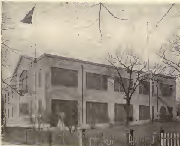
SOUTH ELEVATION SHOWING LOUVRE CONSTRUCTION INSTALLED IN LARGE OPENINGS OF TRANSFORMER COMPARTMENTS
