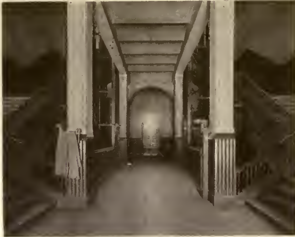
OLD FIRST FLOOR LOBBY
