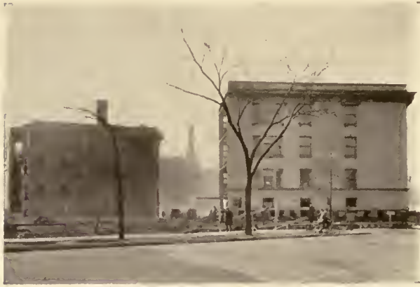
TURNING OF SECTION 2 ALMOST COMPLETED AND READY TO BE MOVED BACK INTO FINAL POSITION. SECTION 1 AT LEFT AND UNDERPINNED WITH BRICK ON NEW FOUNDATIONS. SECTION 2 STILL IN IRVING AVENUE, JACKSON BOULEVARD IN FOREGROUND.
