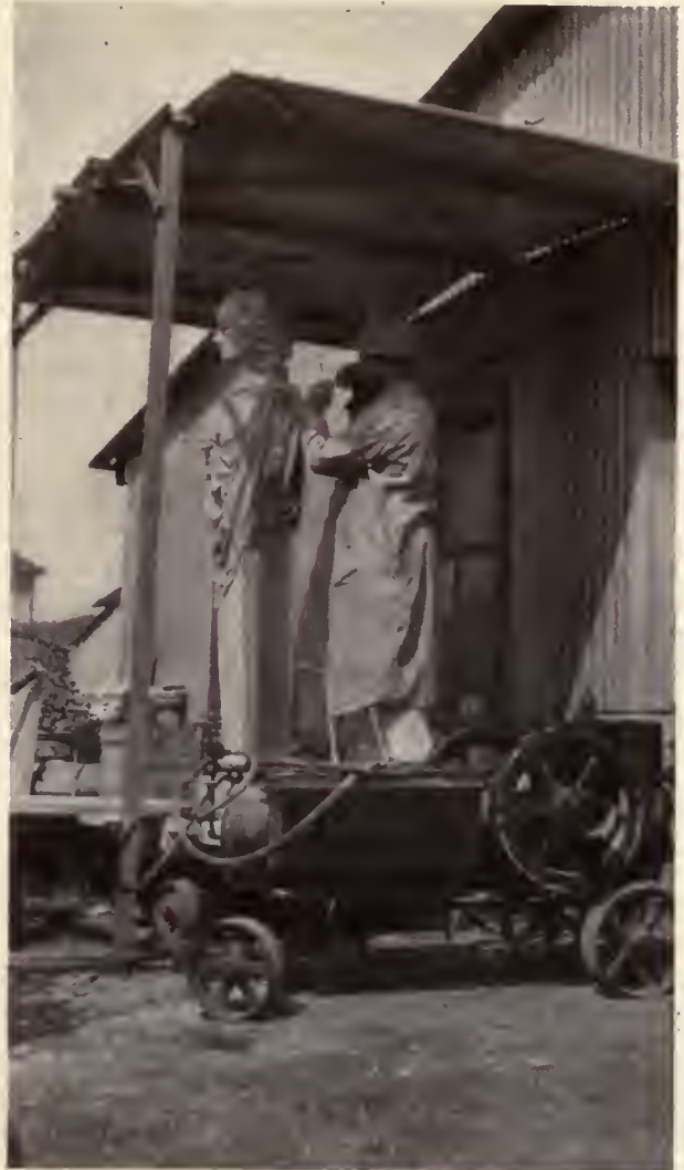
CAST STONE TERMINAL BEING RETOUCED WITH PNEUMATIC TOOL
