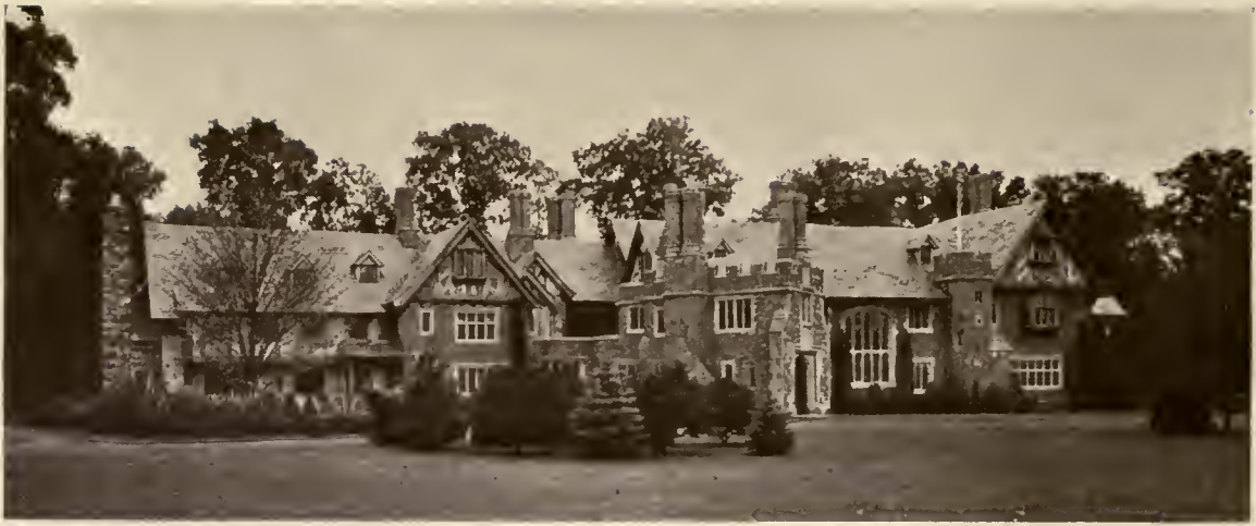
HOUSE OF GEORGE MARSHALL ALLEN, MORRISTOWN, N. J. CHARLES I. BERG, ARCHITECT
