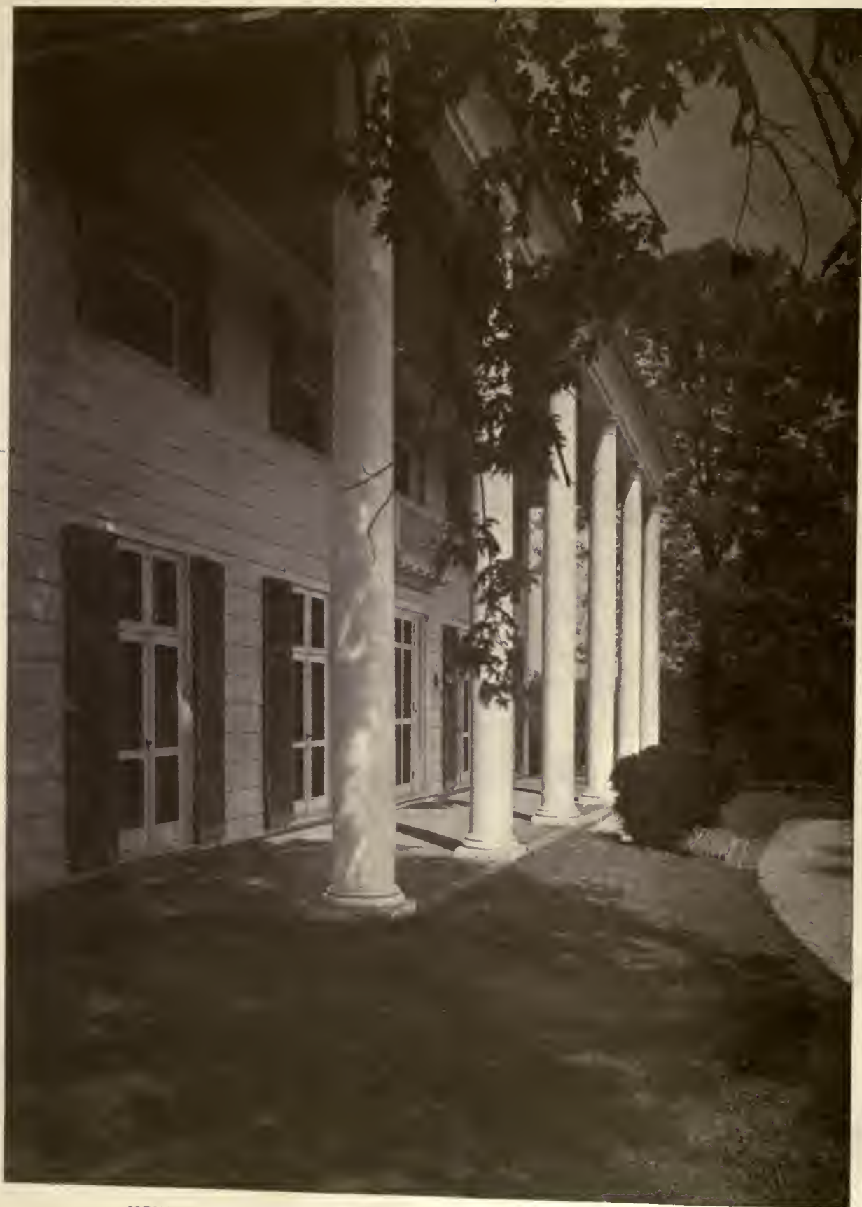
HOUSE OF J. RANDOLPH ROBINSON AT WESTBURY, LONG ISLAND JOHN RUSSELL POPE, ARCHITECT
