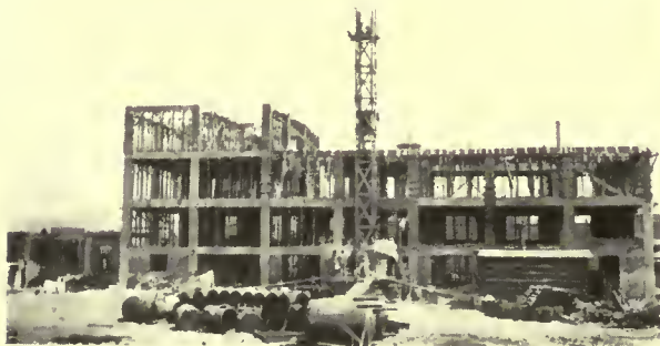
Building 1 under construction.
