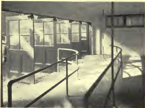
Entrance to ramp showing hand rails for preventing congestion.
