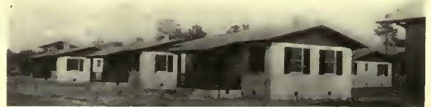
Jacksonville, Fla. H. J. Klutho, Architect. 158 houses. Work started Aug. 28, 1918; photograph taken Dec. 16, 1918.
