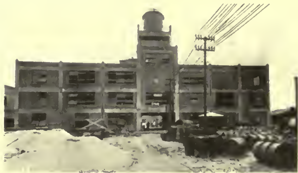
View of Building 10A, 10B, 10C, from the north, showing the main thoroughfare through the first story. Hydrant and hose house in the foreground.
