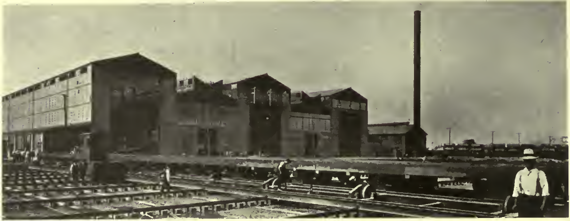
Exterior view showing the large doors for passage of hulls and the transfer table to transport the hulls to the fitting basin.
