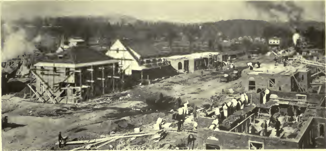
Newburgh, N. Y. Branch of Design, Housing Department and Ludlow & Peabody, Architects. 127 houses, 76 apartments and 2 stores in 13 apartment buildings. Work started Oct. 9, 1918; photograph taken Dec. 1, 1918.
