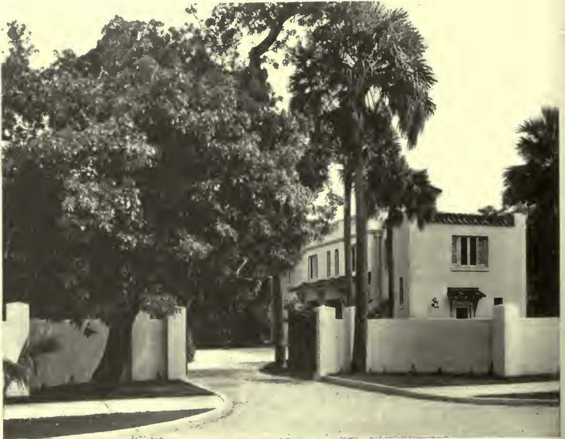
MAIN ENTRANCE AND GARAGE
