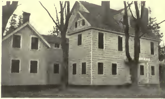
HOUSE BEFORE ALTERATIONS
