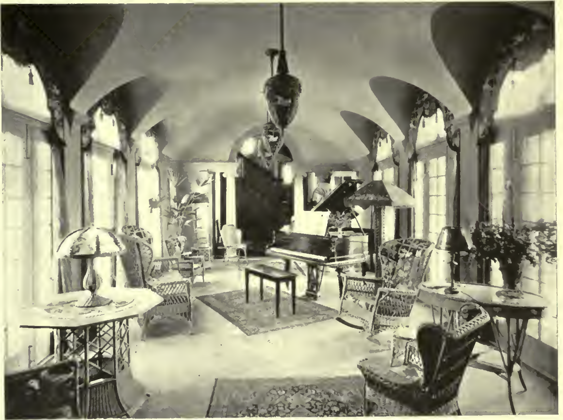
FIRST FLOOR LOGGIA
