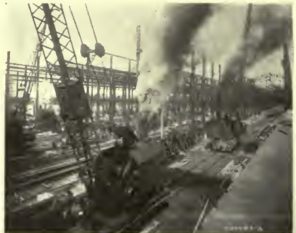
Erecting frame with locomotive cranes.
