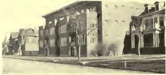
AN APARTMENT BUILDING IN THE HEART OF THE RESIDENCE DISTRICT
