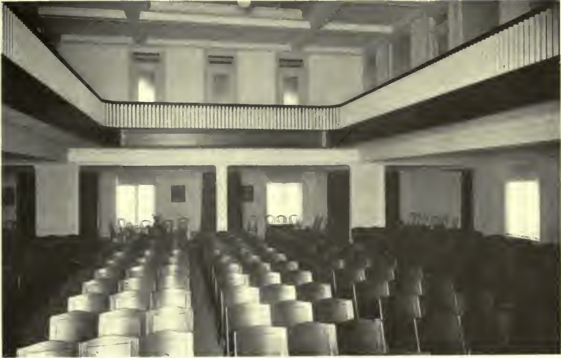
SUNDAY SCHOOL ASSEMBLY ROOM
