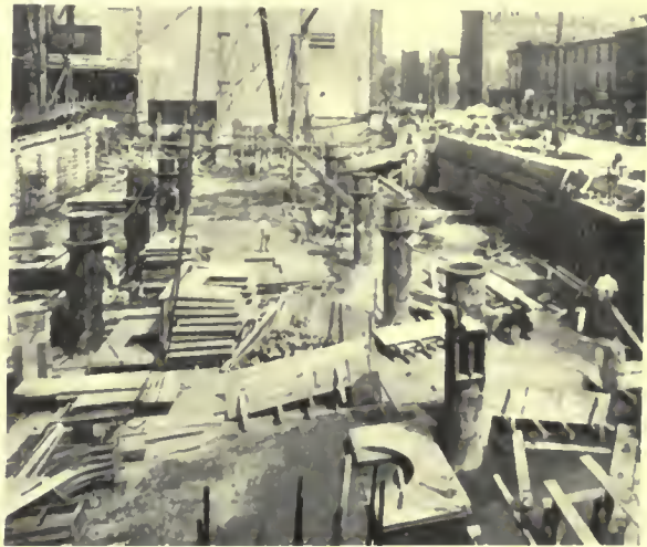
Basement columns in position with slab form material ready for erection
