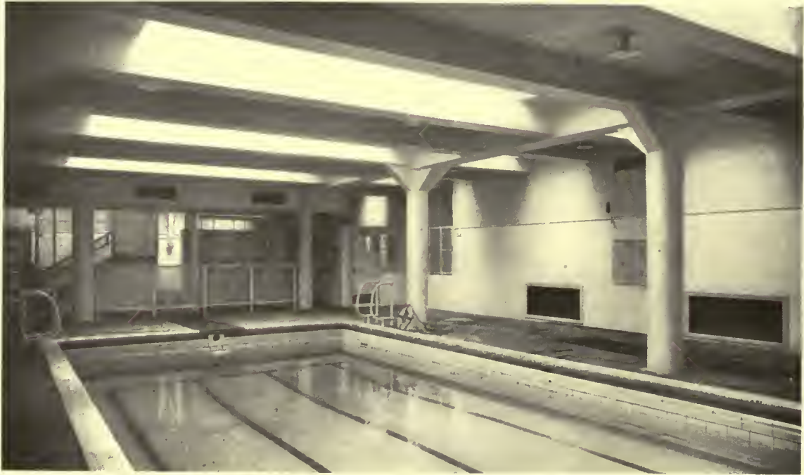
Fig. 7. General view of the pool and natatorium facilities in Public School No. 66, Borough of Brooklyn. The plan of this pool is shown in Fig. 2. Note the guide lines on the floor of the pool, also the generous register openings for fresh air supply and ventilation.
