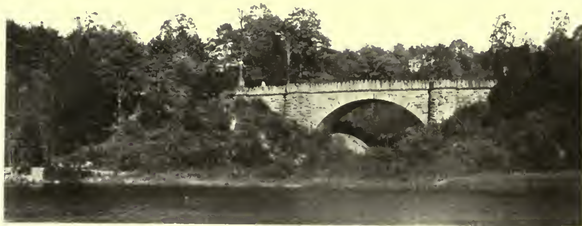
A BRIDGE SPANNING A RAVINE
