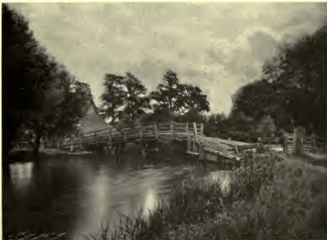
FLATFORD BRIDGE, ENGLAND. AN EXCELLENT TYPE OF SIMPLE WOODEN BRIDGE
