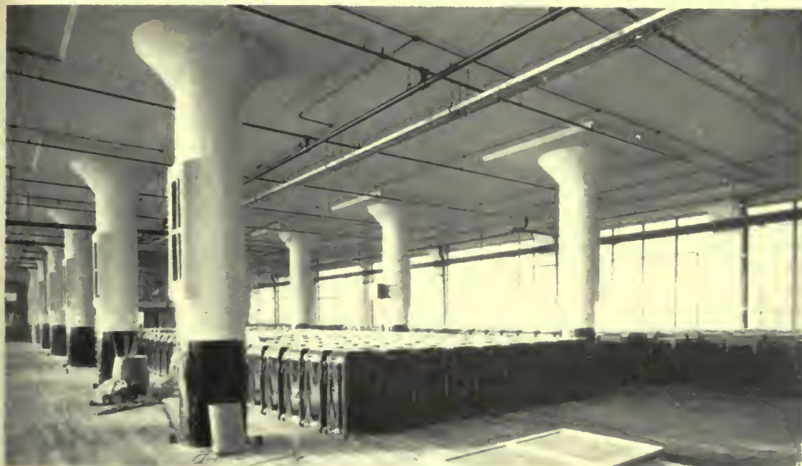
View of a finished story, except that the hot air registers are not yet in place.
