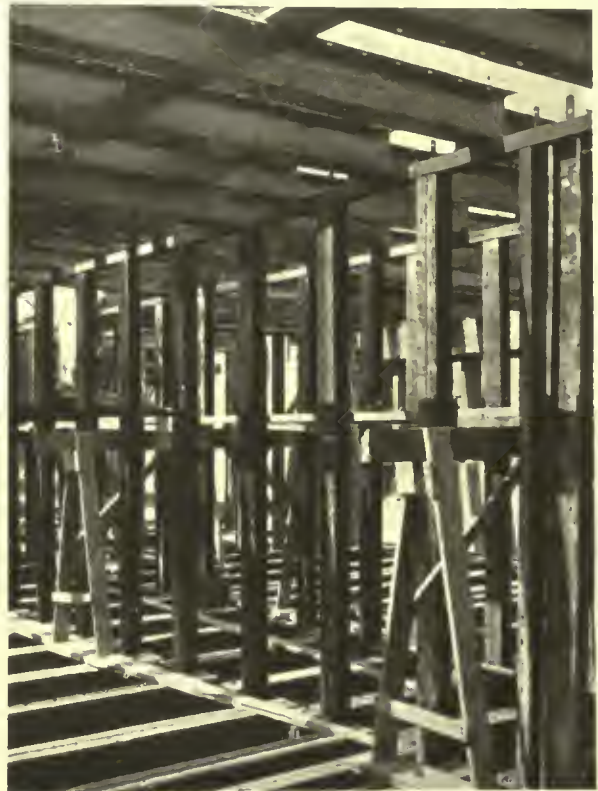
Apartment house construction, showing metal floor joists, studs, cap and sill plates.
