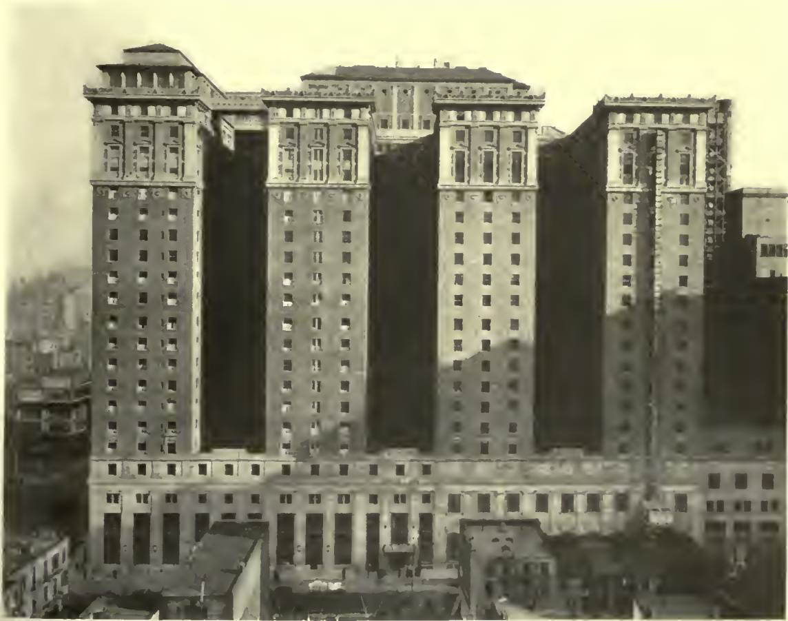
SOUTH, OR THIRTY-SECOND STREET FRONT
