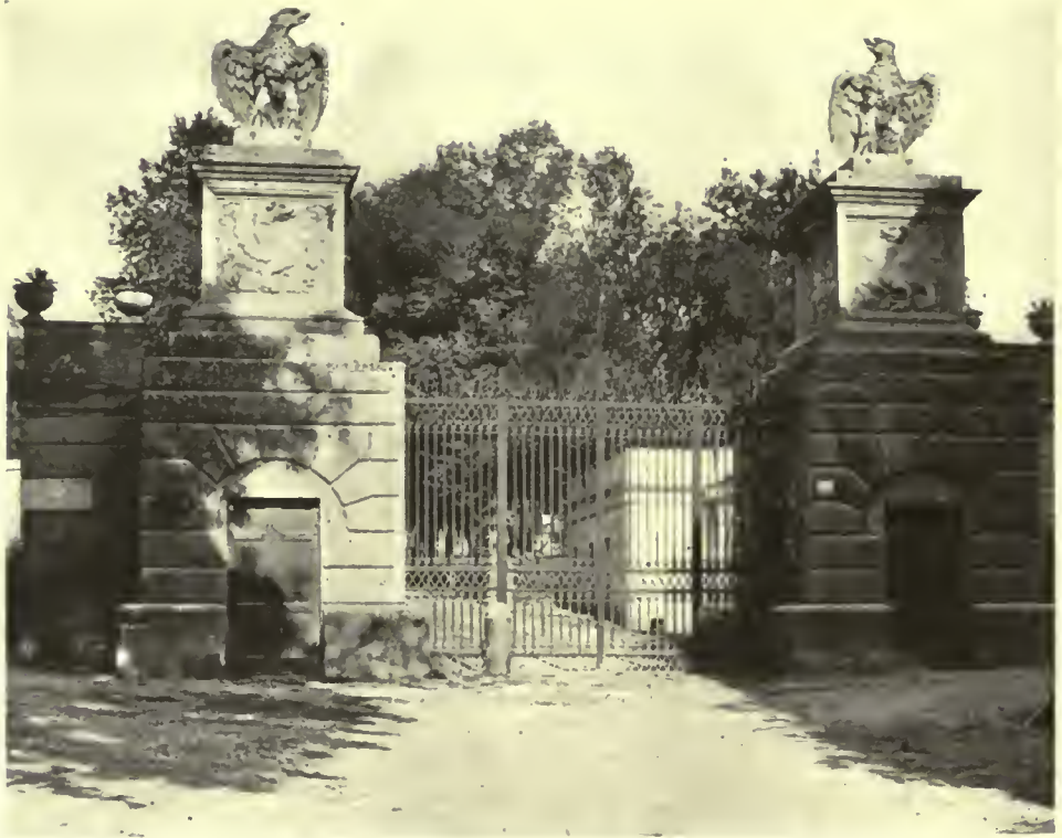
ENTRANCE, VILLA BORGHESE, ROME
