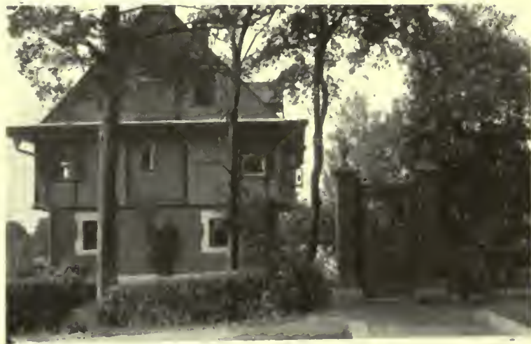
NORTH ELEVATION AND GATE, RABBIT HOUSE
