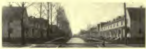
St. Helena, Md. E. L. Palmer, Jr., Architect. 296 houses, mess hall and kitchen and power house. Started May 15, 1918; photograph taken Nov. 15, 1918.
