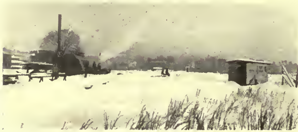
Site of the improvement on December 19, 1916.
