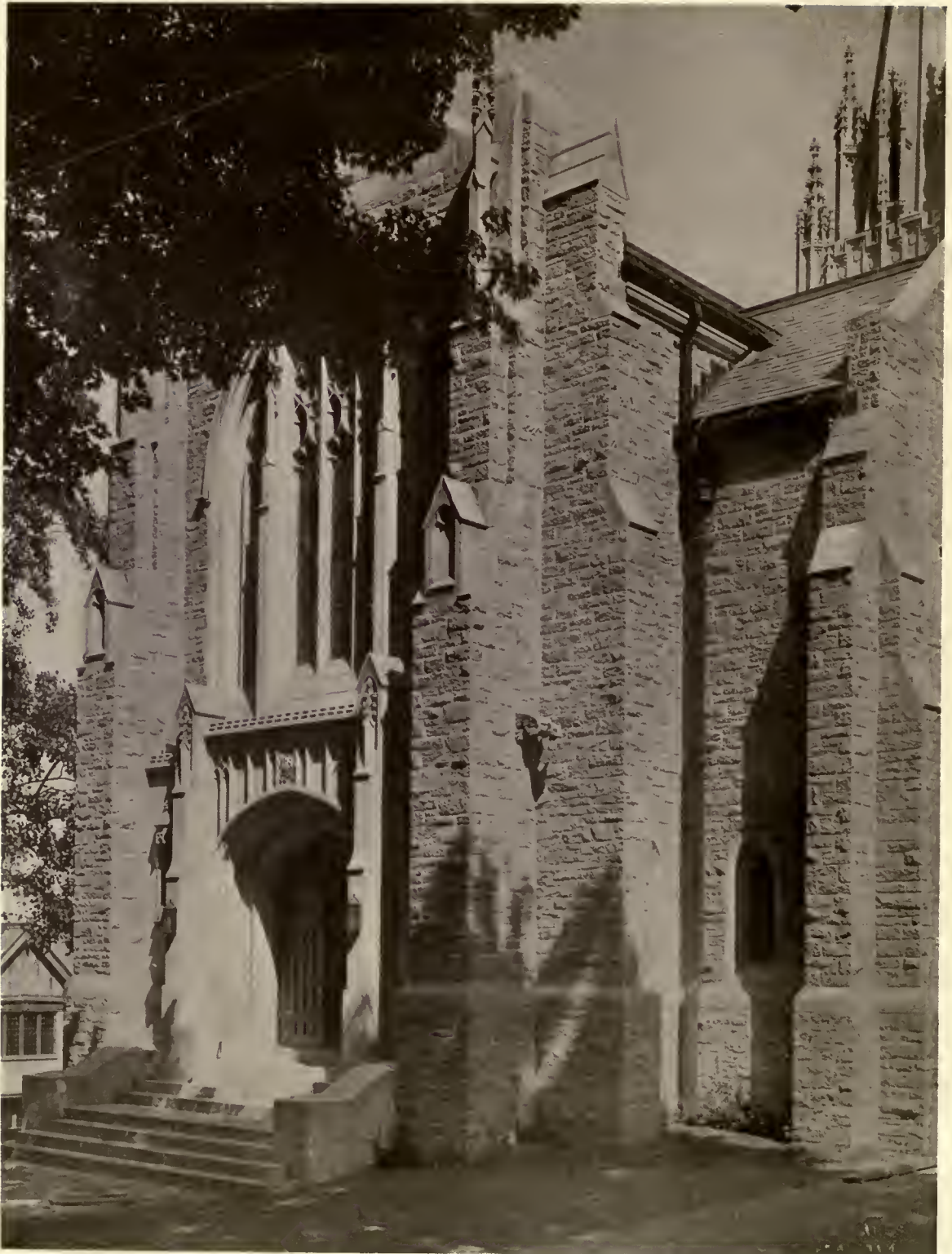
SECOND CHURCH IN NEWTON—WEST NEWTON, MASS. MESSRS. ALLEN & COLLENS, ARCHITECTS
