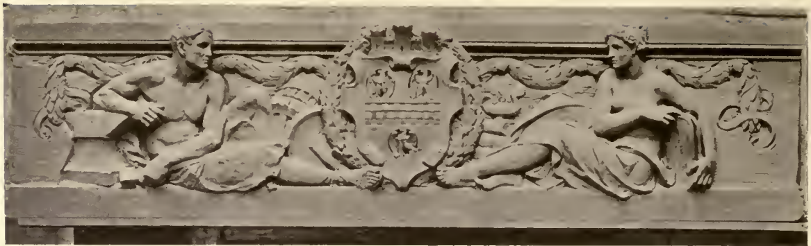
DECORATIVE PANEL, CITY AND COUNTY BUILDING, PITTSBURGH, PA. MR. CHARLES KECK, SCULPTOR MR. EDWARD B. LEE AND MESSRS. PALMER, HORNBOSTEL & JONES, ASSOCIATED ARCHITECTS THIRTY-SECOND ANNUAL EXHIBITION, ARCHITECTURAL LEAGUE OF NEW YORK
