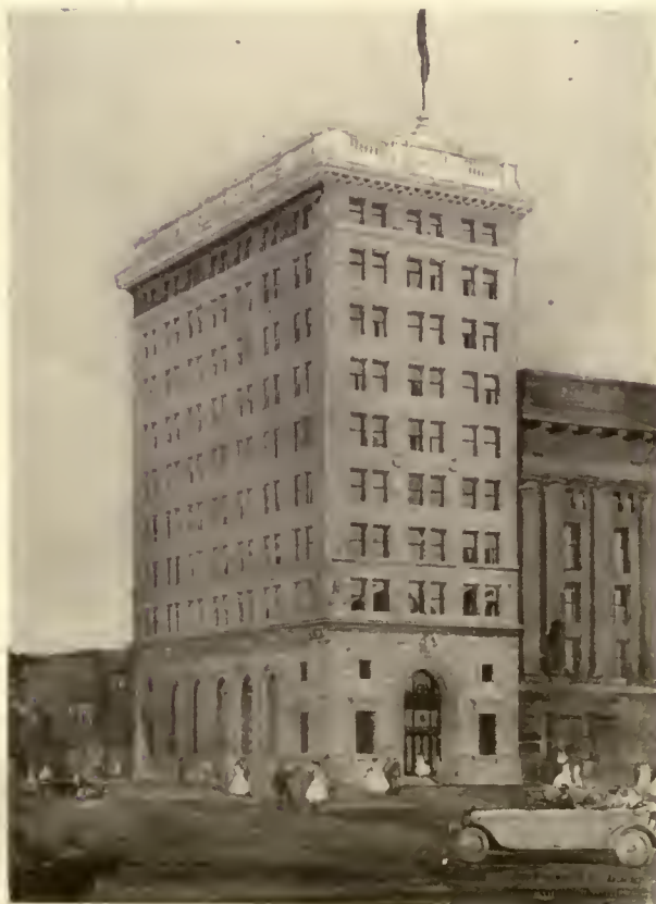
BANK OF HAMILTON, WINNIPEG, MANITOBA MESSRS. H. C. INGALLS AND F. B. HOFFMAN, JR., ARCHITECTS
