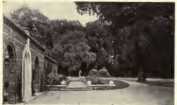
PART OF UNFINISHED CARRIAGE COURT SHOWING WALL OF CLOISTER GARDEN; THE SMALL ARCHES ARE FILLED WITH FRENCH TREILLAGE
