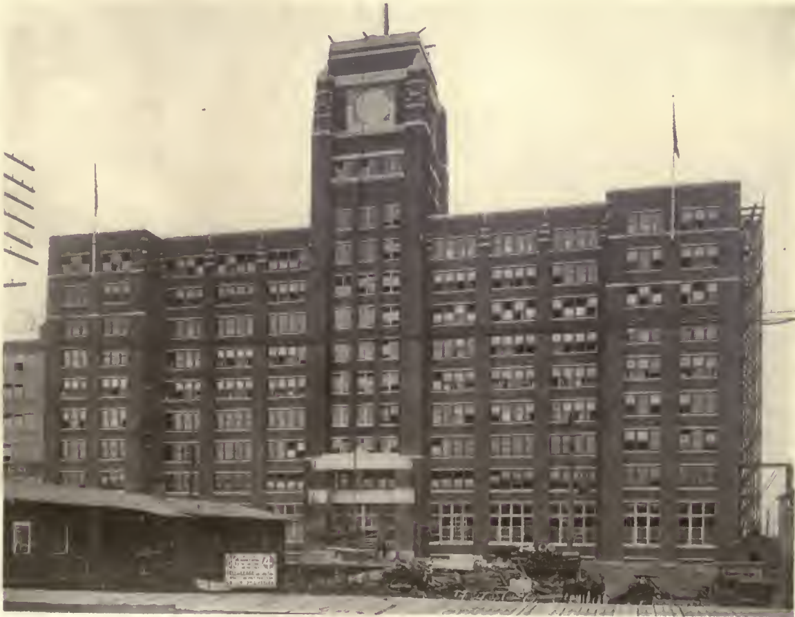
SEATTLE PLANT, SEARS, ROEBUCK & CO. MR. GEORGE C. NIMMONS, ARCHITECT
