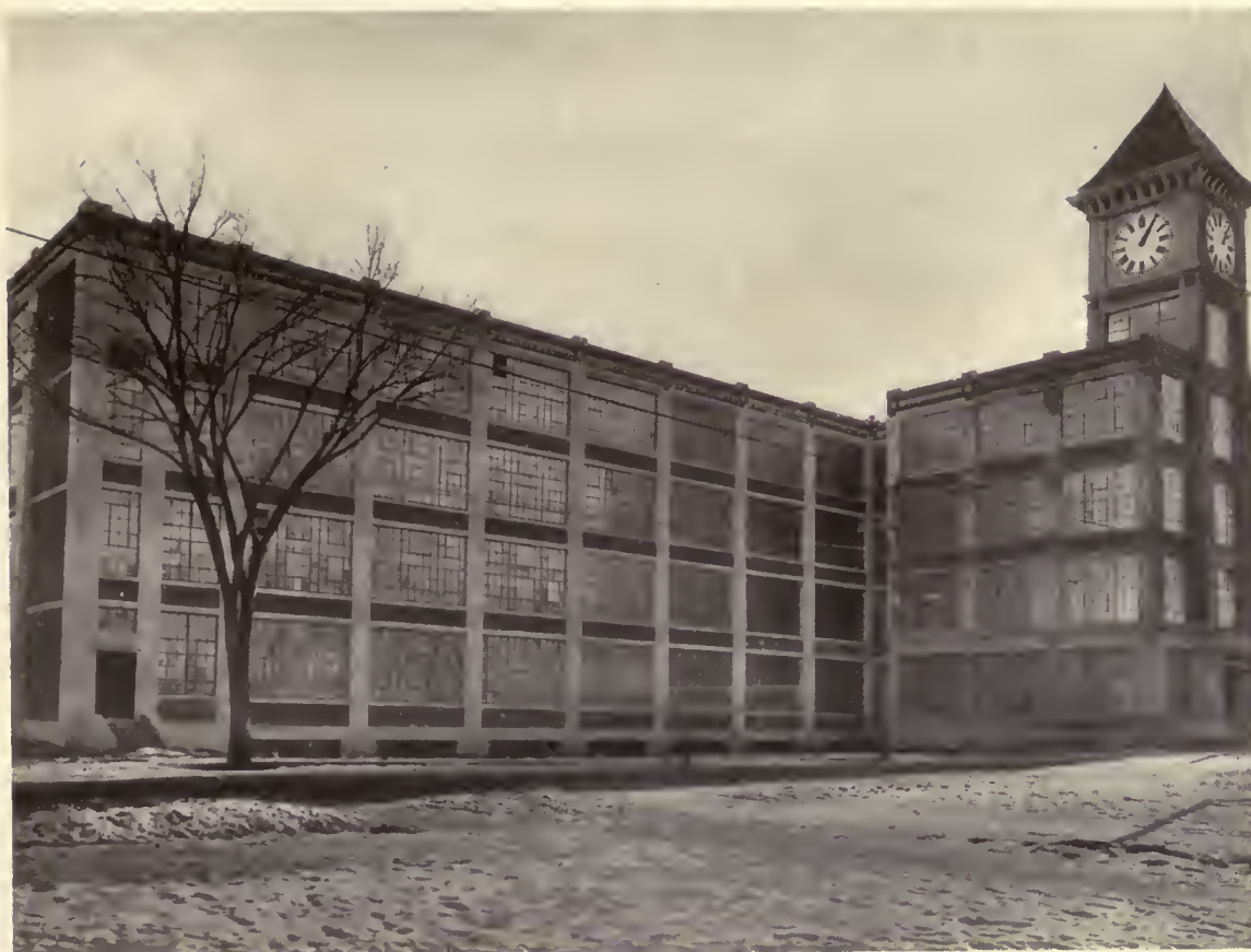
FACTORY, SETH THOMAS CLOCK CO., THOMASTON, CONN. MESSRS. LOCKWOOD, GREENE & CO., ARCHITECTS
