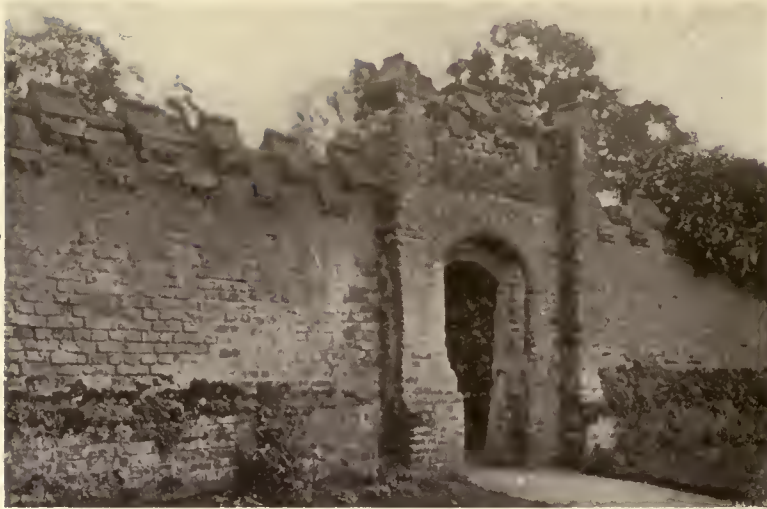
FIG. 1—FORE COURT WALL AND GATEWAY, BRECCLES HALL, NORFOLK
