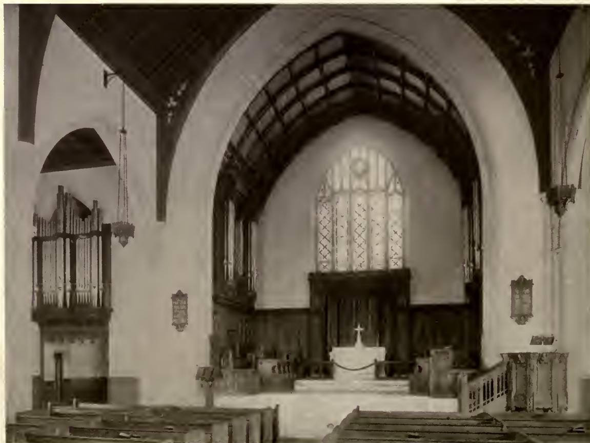
SECOND CHURCH IN NEWTON—WEST NEWTON, MASS. MESSRS. ALLEN & COLLENS, ARCHITECTS
