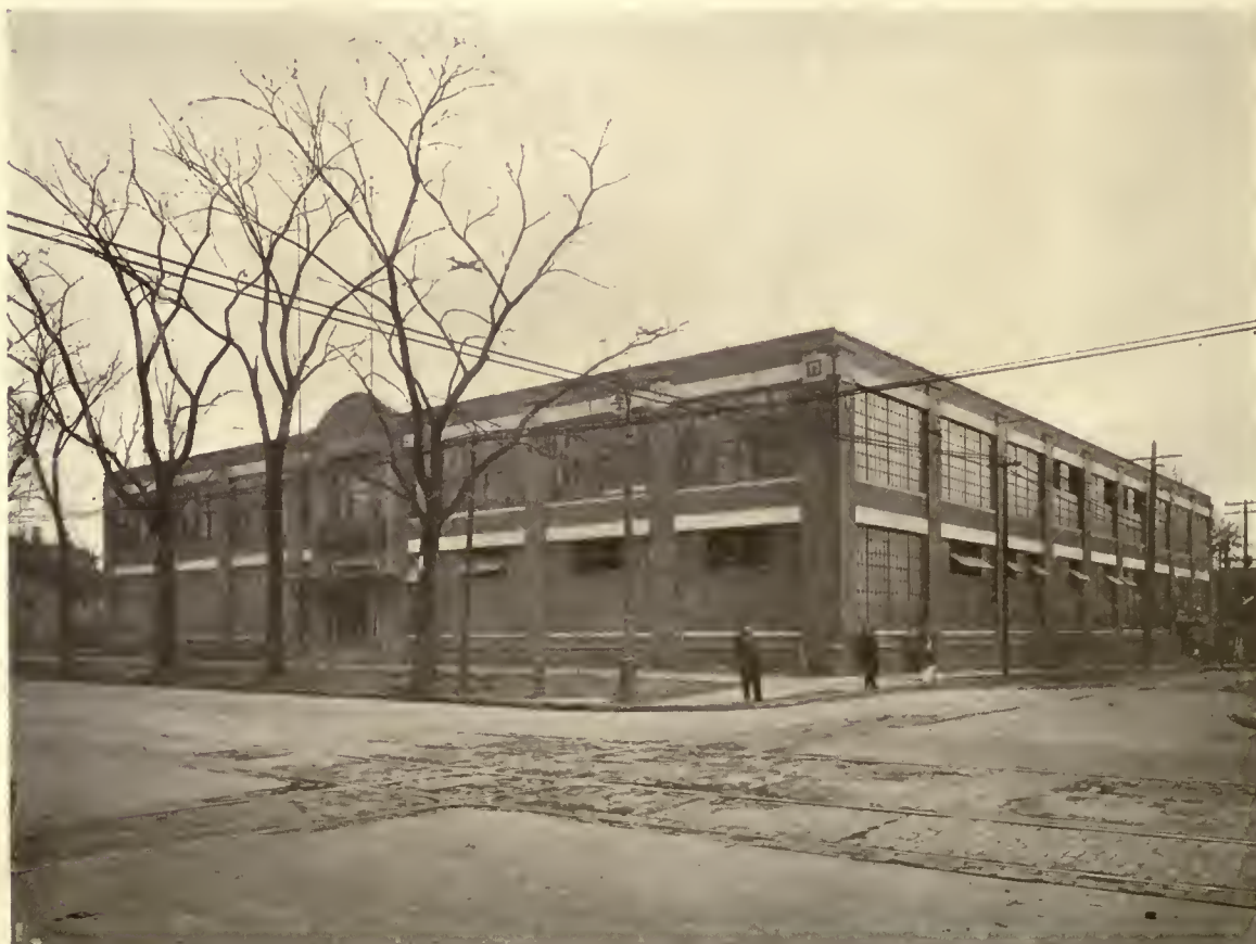
BUILDING OF ARTHUR COLTON CO., DETROIT, MICH. MESSRS. MILDNER & EISEN, ARCHITECTS
