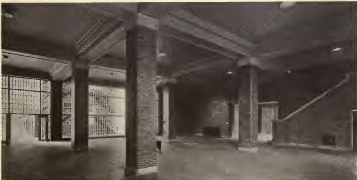
MAIN CORRIDOR SHOWING ENTRANCE TO CELL HOUSE
