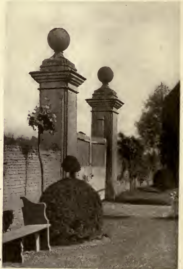
FIG. 6—GATE PIERS, WATER EATON MANOR
