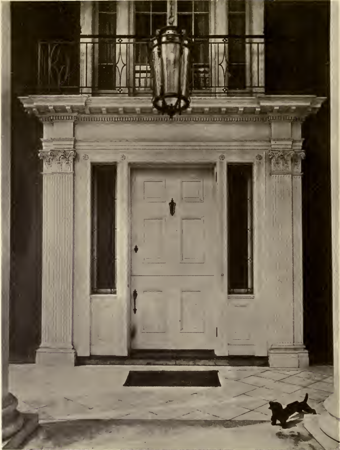
DETAIL OF ENTRANCE, EAST FRONT
