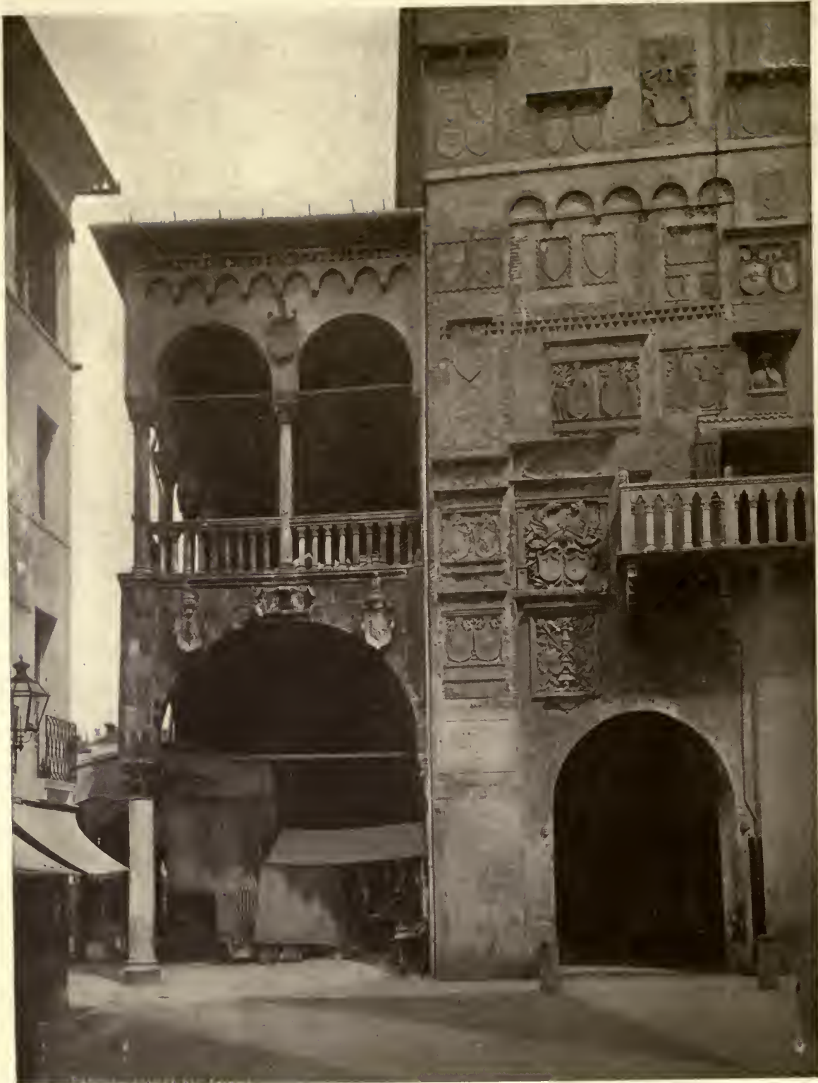
HOUSE IN PADUA, ITALY
