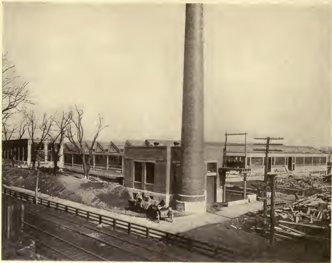
POWER PLANT, CINCINNATI-BICKFORD TOOL CO., CINCINNATI, O. MESSRS. DAY & ZIMMERMANN, ARCHITECTS AND ENGINEERS
