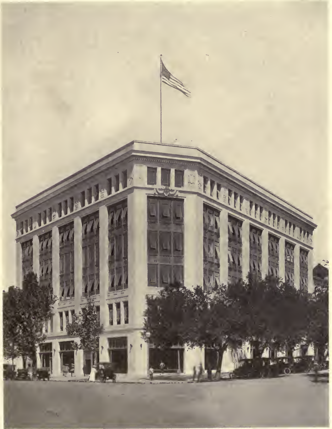
SERVICE BUILDING, FORD MOTOR CO., WASHINGTON, D. C.
