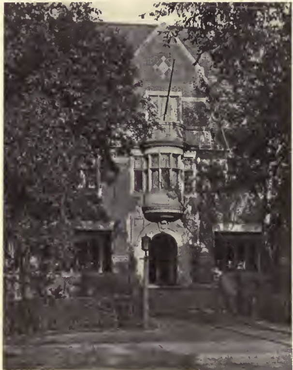
DETAIL OF ENTRANCE FRONT KITCHI GAMMI CLUB, DULUTH, MINN. CRAM, GOODHUE & FERGUSON, ARCHITECTS New York Office
