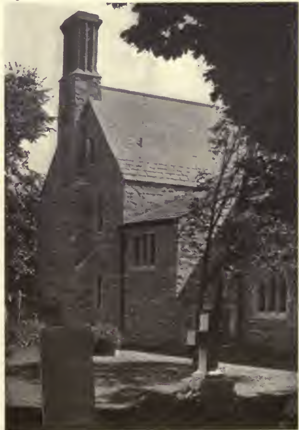
MORRISTOWN PARISH HOUSE, MORRISTOWN, N. J.
