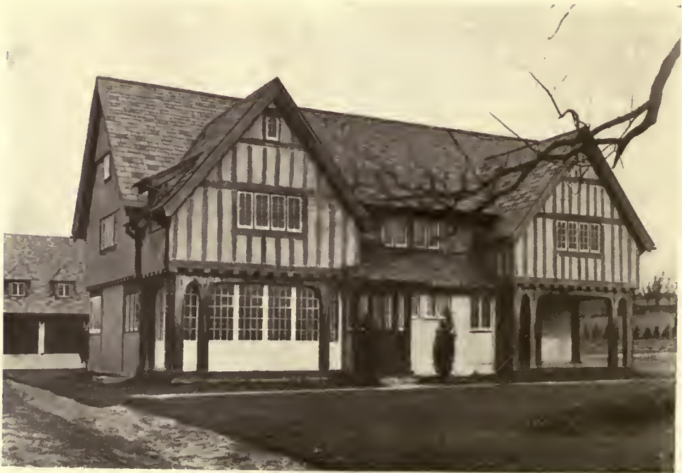
FARM BUILDINGS, GREENWICH, CONN. MR. W. F. DOMINICK, ARCHITECT
