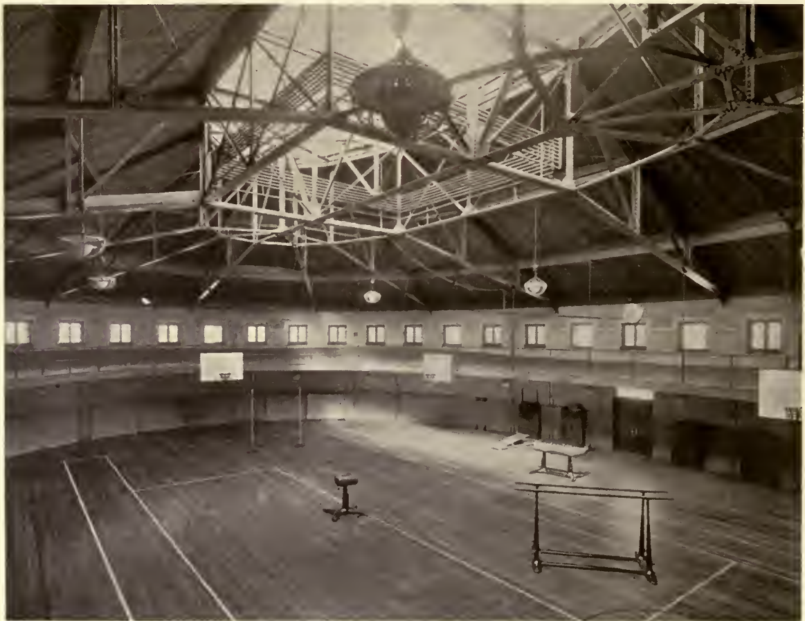
INTERIOR OF GYMNASIUM
