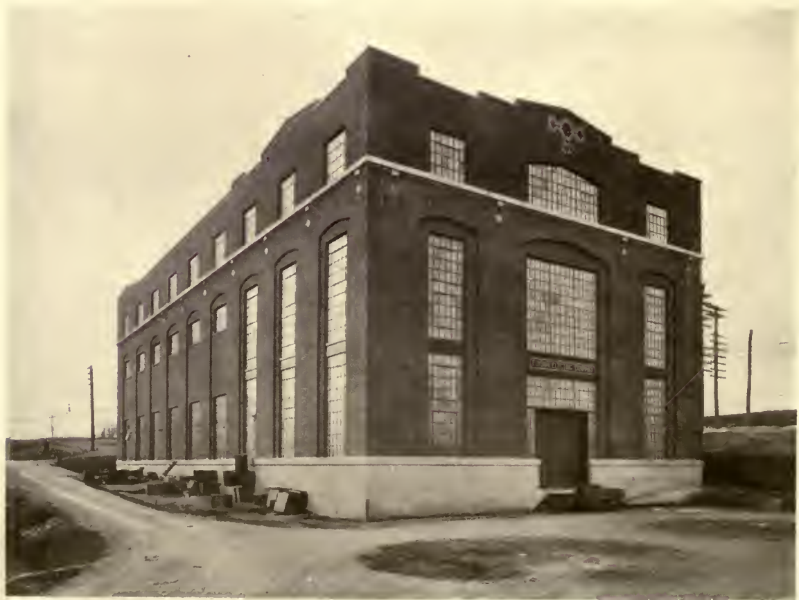
SUB-STATION, EDISON ELECTRIC CO., LANCASTER, PA.
