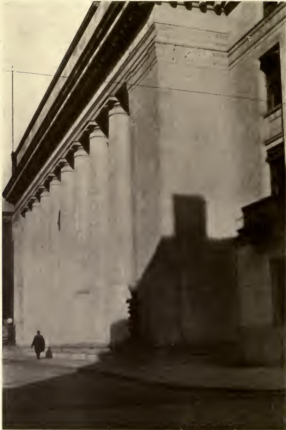
LEHIGH VALLEY TERMINAL, BUFFALO, N. Y. MR. KENNETH M. MURCHISON, ARCHITECT
