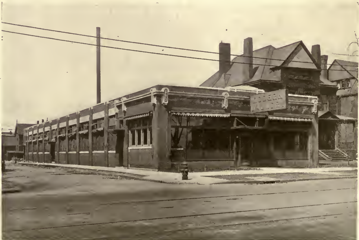
LAUNDRY BUILDING, DETROIT, MICH. MESSRS. MILDNER & EISEN, ARCHITECTS
