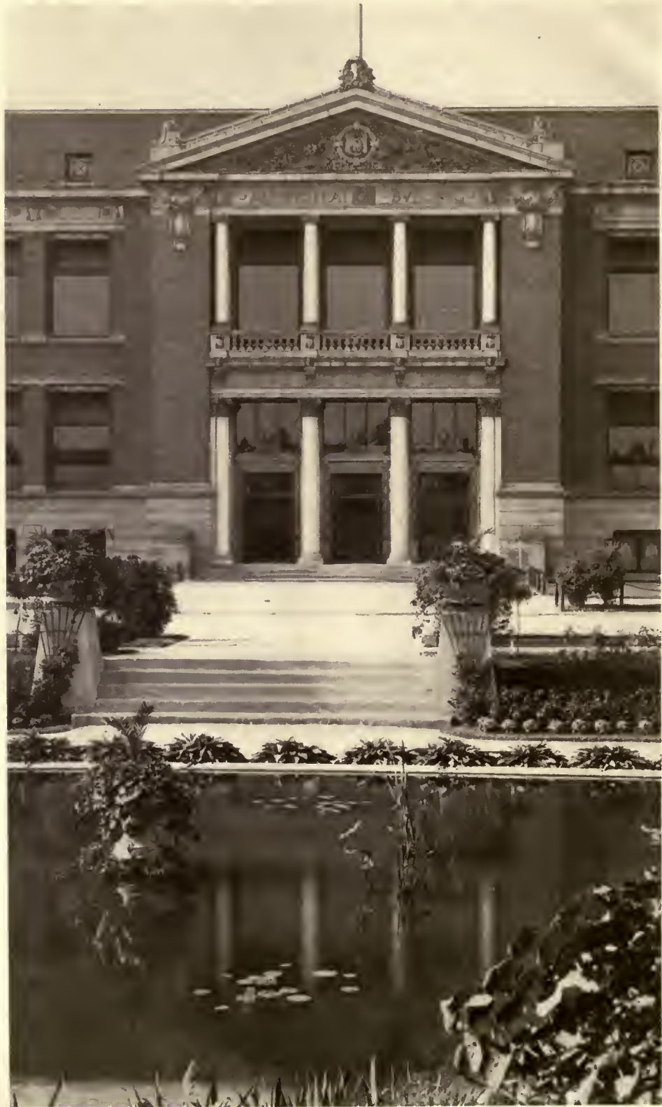
MAIN ENTRANCE, ADMINISTRATION BUILDING, SEARS, ROEBUCK & CO., CHICAGO
