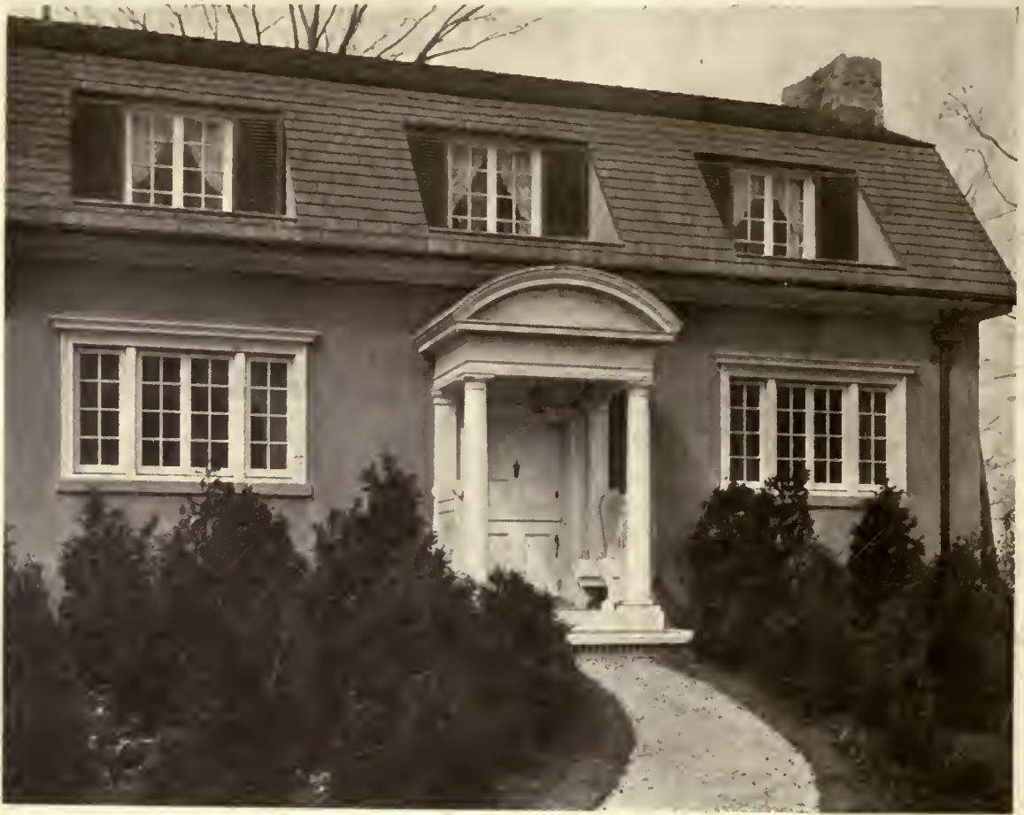
DETAIL OF NORTH WING
