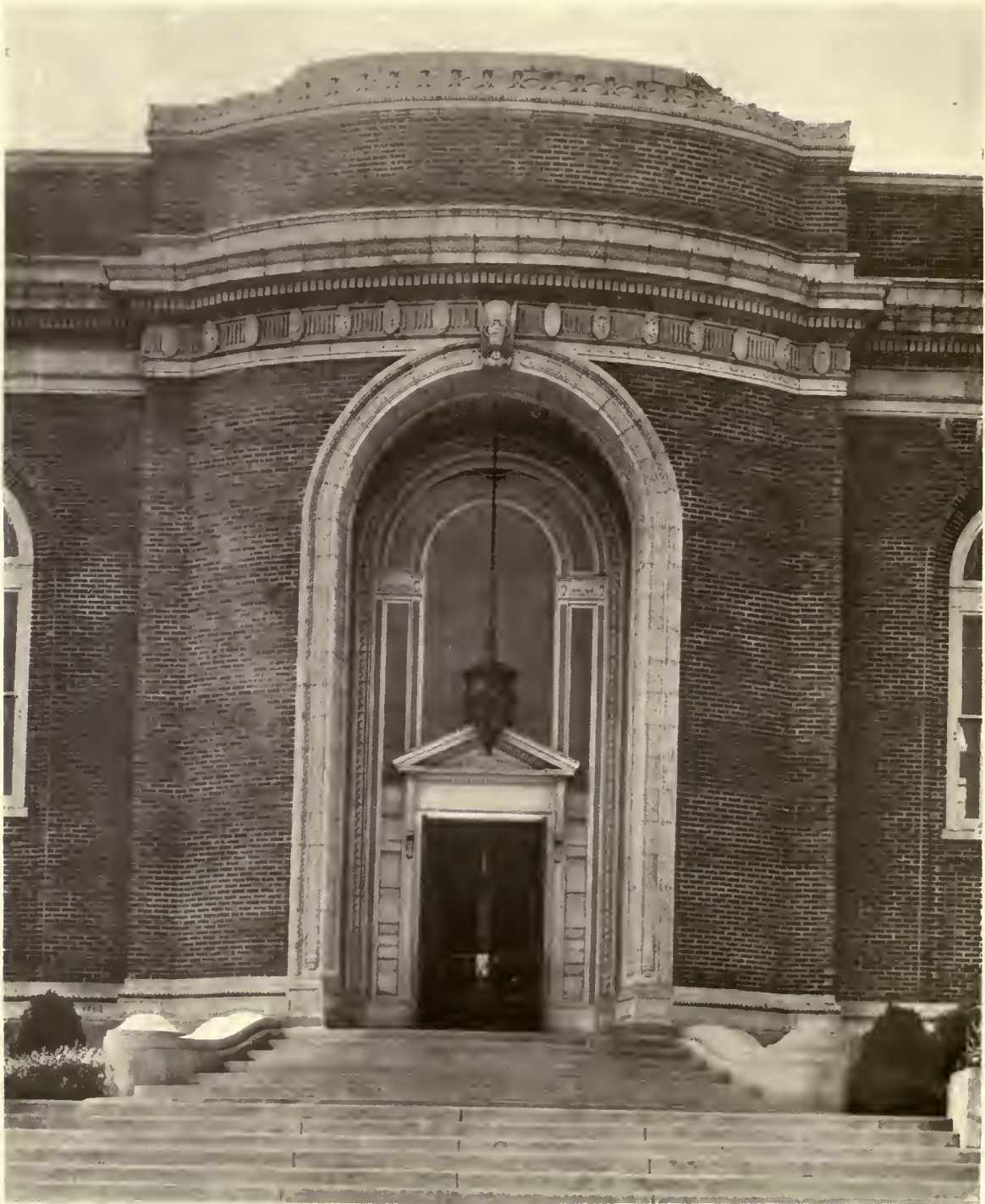
ENTRANCE TO HADDINGTON BRANCH LIBRARY, PHILADELPHIA, PA.
