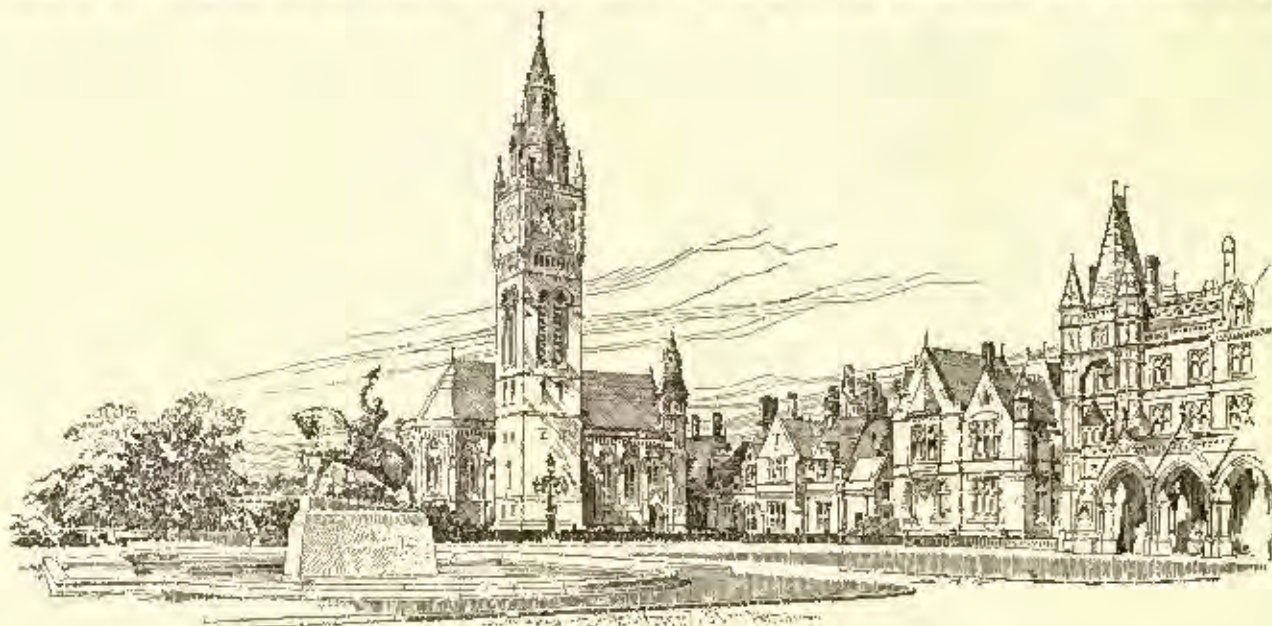
Easton Hall, Chester. Alfred Waterhouse, R. A., Architect.
