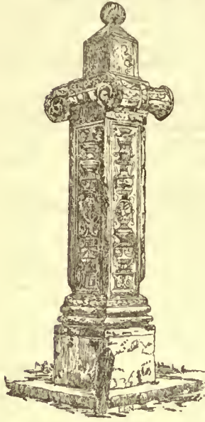
Column at Ravenna.
