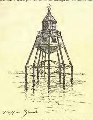
there is much running ice, it has been found advisable to protect these structures against the impact of the ice, either by a wall of riprap, or by ice-breakers detached from the foundation.
