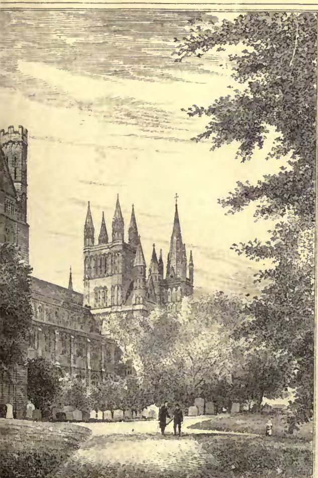
THE CENTRAL TOWER NOW BEING DEMOLISHED 1883
