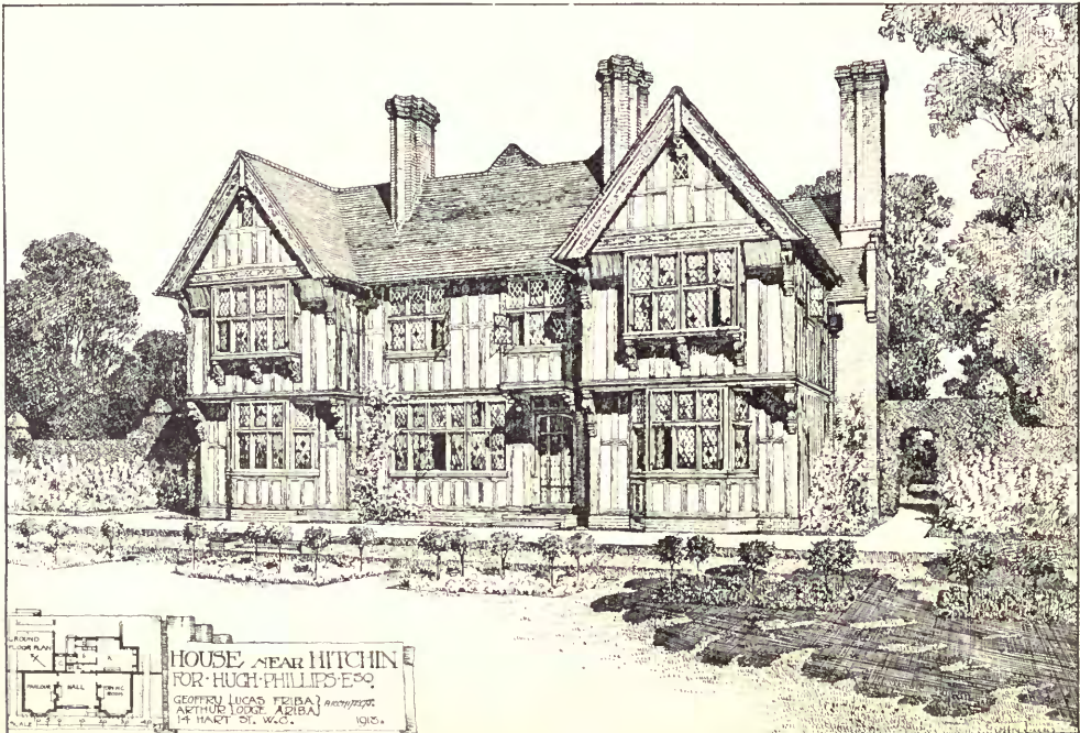
House near Hitchin, LUCAS & LODGE, Architects. Contractor : WILLMOTT & SONS, Hornsey, London, N.
