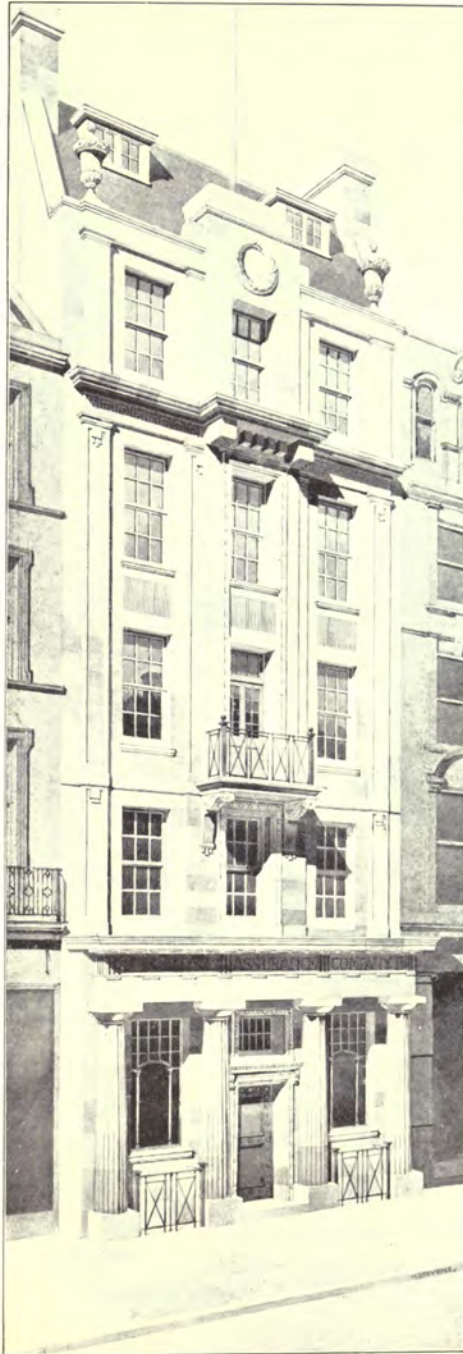
Prudential Assurance Buildings, Belfast, PAUL WATERHOUSE, M.A., Architect.
