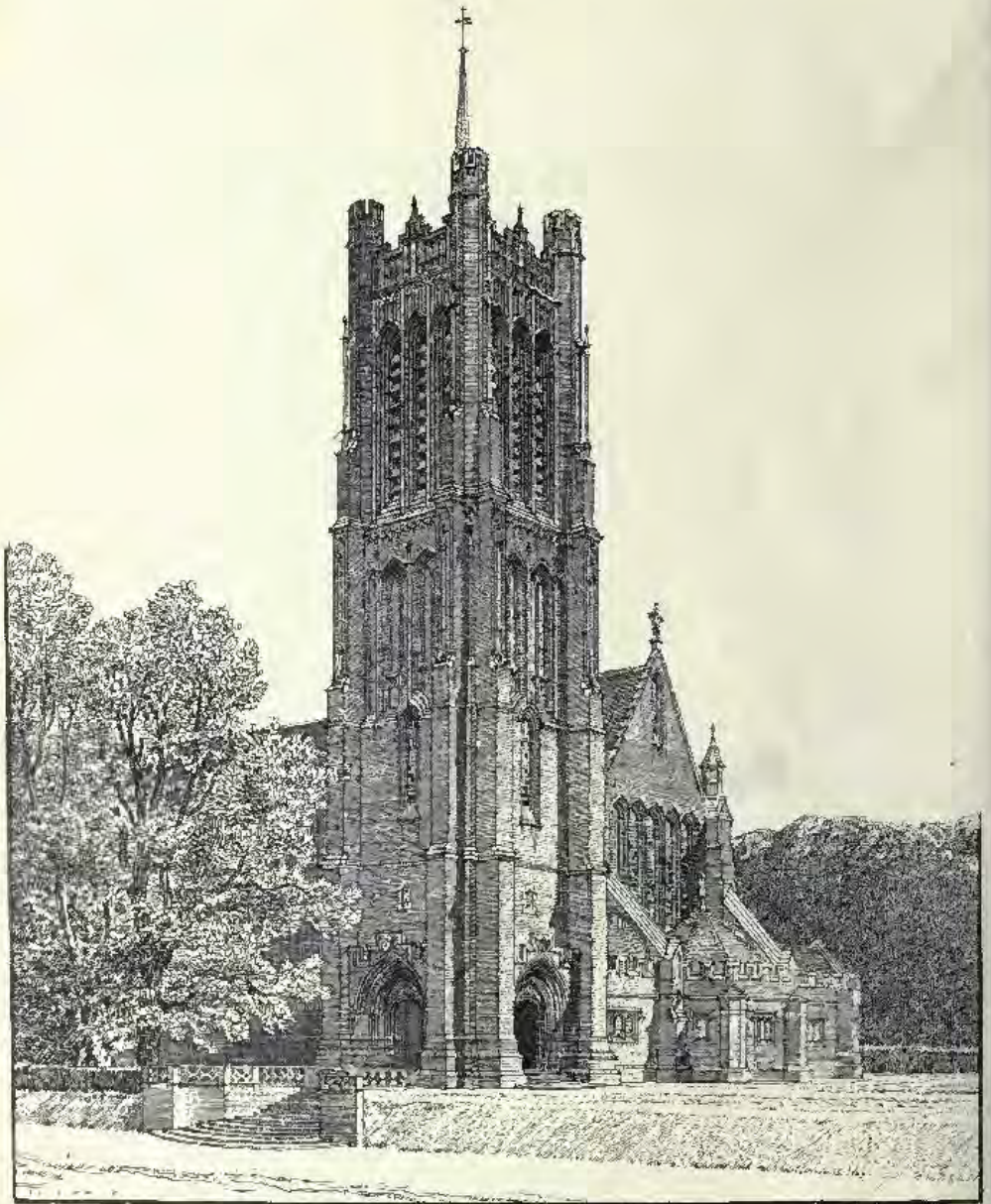
Christ Church, Sutton, Surrey, New Tower, Baptistry, and Northex, DOUGLAS G. ROUND, Architect.
