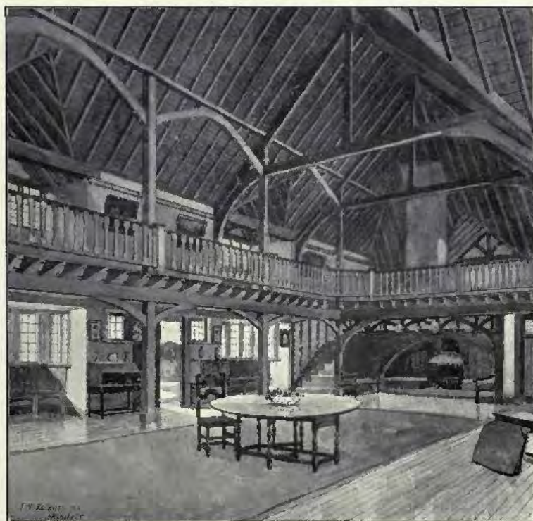
A Studio at Richmansworth, FRANK NORMAN RECKITT, Architect. General Contractor : A. J. Bellow, 16 and 16a Highbury Place, London, N. Sanitary Appliances and Plumbing : Davis, Bennett & Co. Westminster Sanitary Works, London, S.W.
