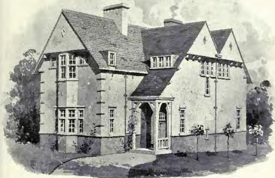
House in the Imley Road, Oxford, J. H. BEART FOSS, Architect.
