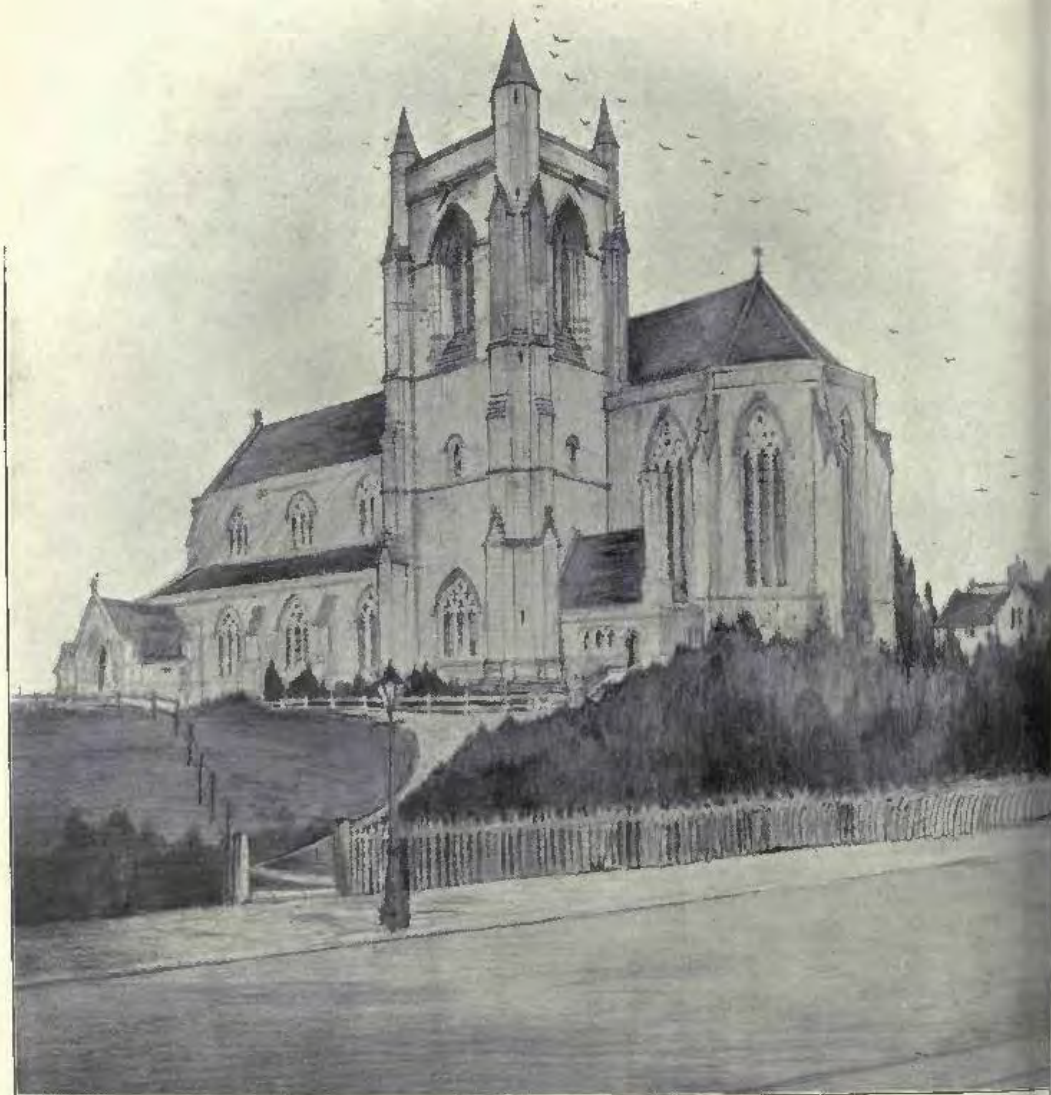
St. Alban's Church, Cheetwood. Manchester, Completion of the Tower, JOHN GIBBONS & SON, Architects. Contractors: DEAKIN & GREENWOOD, Long Street, Elton Street, Lower Broughton, Manchester.
