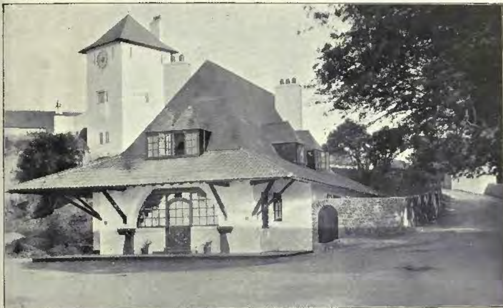
The Village Shop and St. Martin's Tower, Monastery Buildings, Caldey, J. COATES CARTER, Architect.
