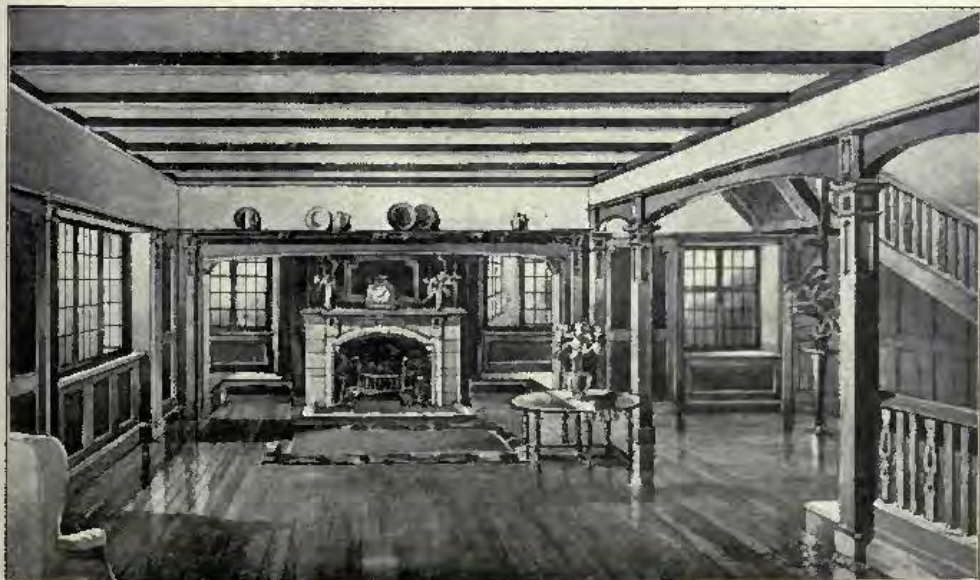
The Living Hall, The Lodge, Portishead, W. HENRY WHITE, Architect.
