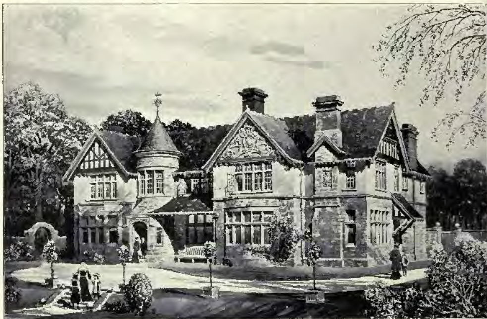
House at Caerw, Maesteg, Glam., E. W. BURNETT, Architect.
