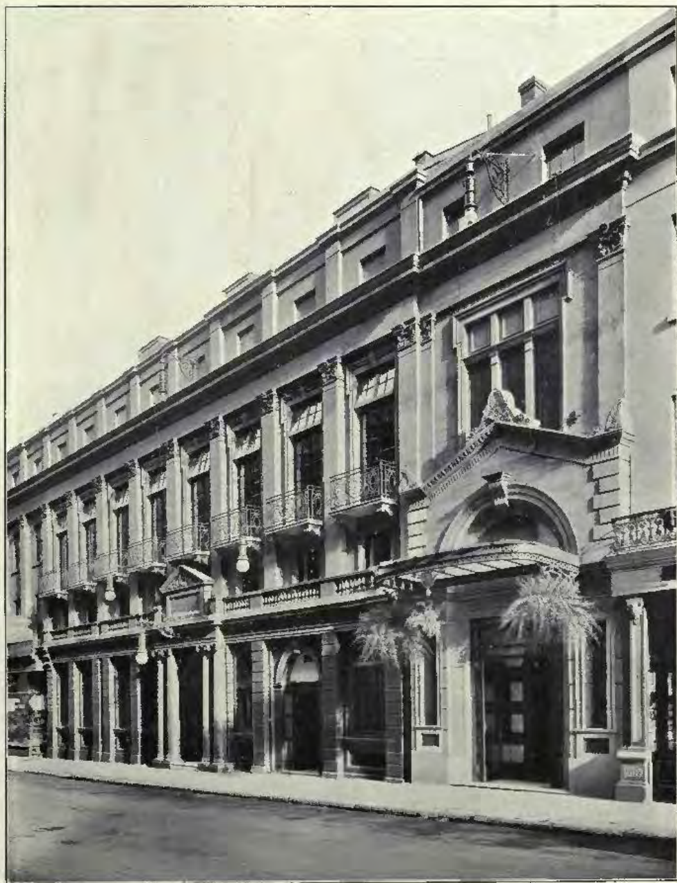
Royal Adelaide Gallery, Messrs. A. & S. Gatti, Ltd., OSWALD C. WYLSON, Architect Electric Tight Fittings, Wrought Iron Staircase and Shelters, Heating and Ventilation: STRODE & Co., 48, Osnaburgh Street, London, N.W.
