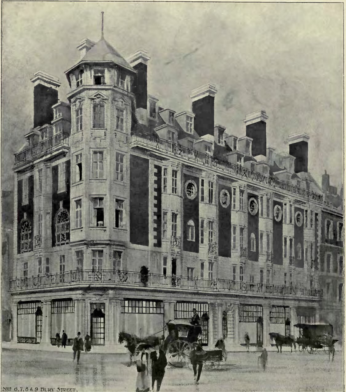
No s 6, 7, 8 & 9 BURY STREET.
