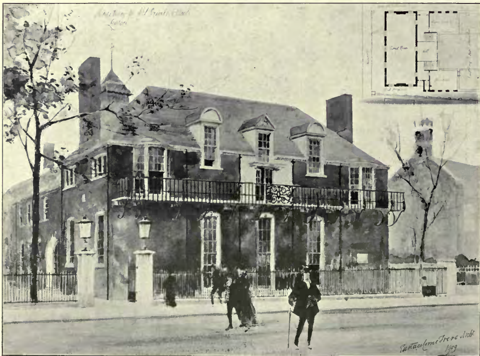
1402. Additions to All Saints' School, Leyton, EUSTACE C. FRERE, Architect. General Contractors: J. and J. Dean, 32, Addison Road, Walthamstow.
