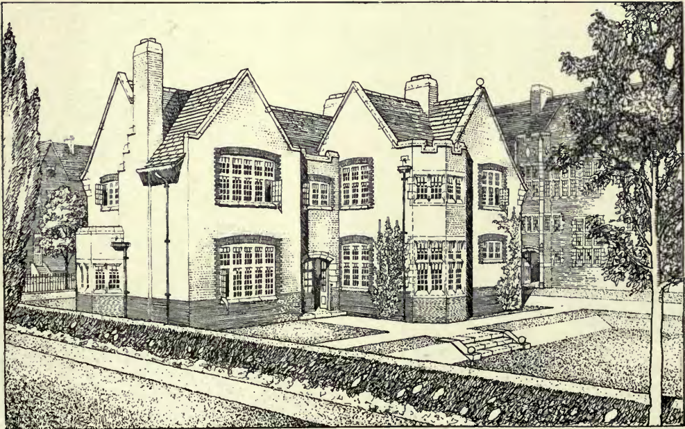
Mistress's House, Godolphin and Latymer School, Hammersmith, GREENAWAY AND NEWBERRY, Architects.
