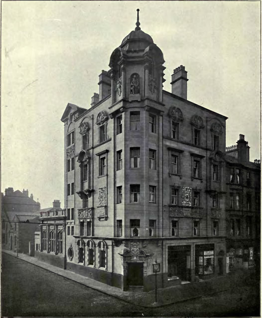
357. Glasgow Savings Bank, Parkhead Branch , HONEYMAN, KEPPIE AND MACKINTOSH, Architects. (For Plans, see p. 92.)
