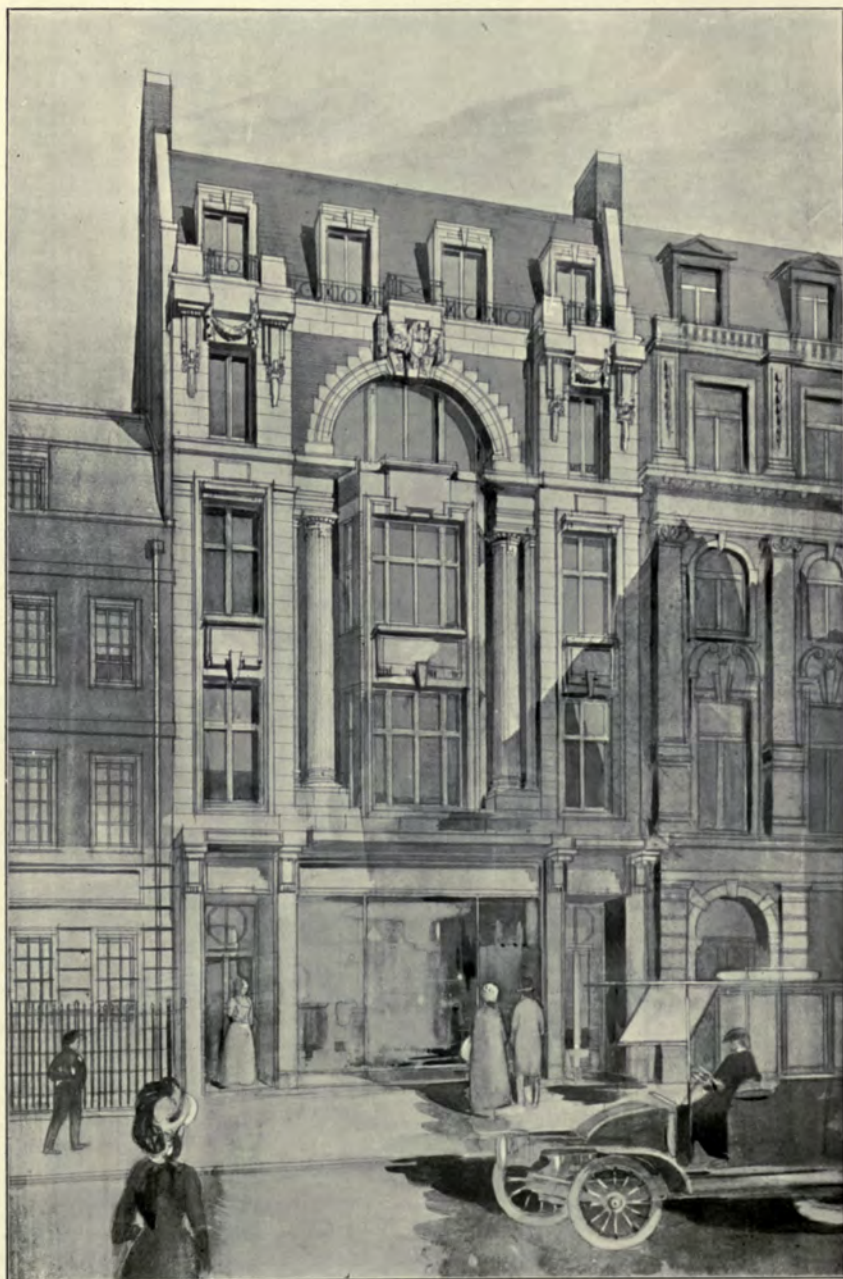
1714. No. 28 Margaret Street, W., JOHN BELCHER, A.R.A., Architect. Contractors: G. Godson and Sons, Pembroke Works, Kilburn Lane, W. Steelwork: G. Aston and Sons, Limited, 46 Eagle Wharf Road, N. Stone Carving: E. J. and A. T. Bradford, 62A Borough Road, S.E. (Tel. 2384 Hop.)
