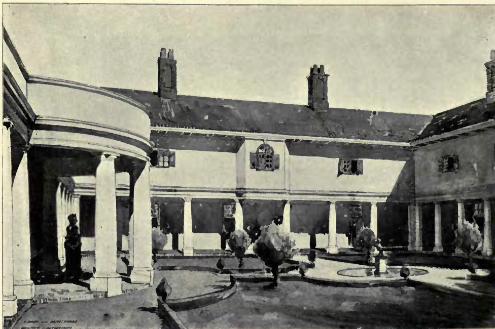
1606. Courtyard, New Government Buildings, Bloemfontein, BAKER AND MASEY, Architects.
