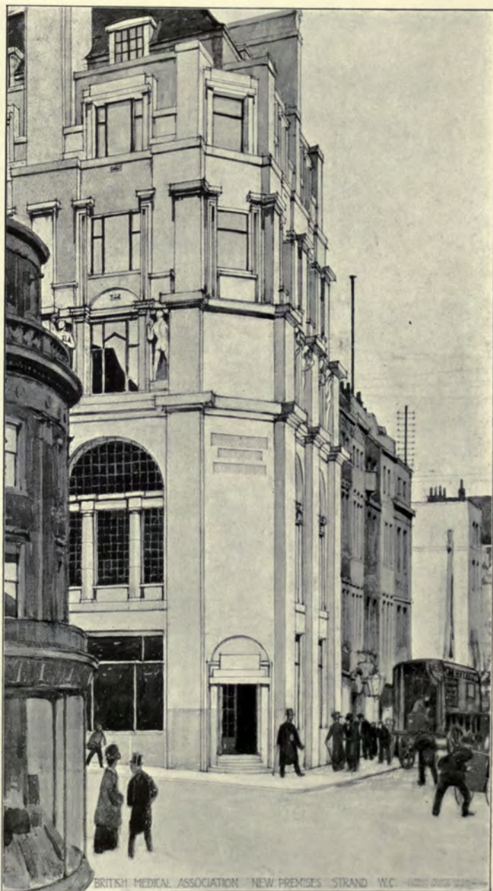
BRITISH MEDICAL ASSOCIATION NEW PREMISES STRAND W.C. 1908 1569. Premises for the British Medical Association, Strand, H. PERCY ADAMS AND CHARLES HOLDEN, Architects. Constructional Steelwork and Fireproof Flooring by: Messrs. Homan and Rodgers, 17 Gracechurch Street, E.C.
