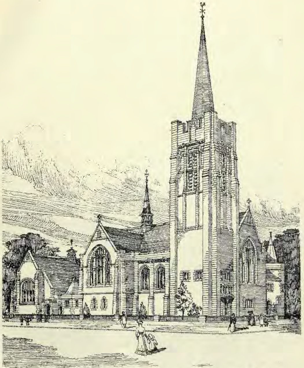
620. St. Mungo's Parish Church, Easter Road, Edinburgh, DUNN AND FINDLAY, Architects.
