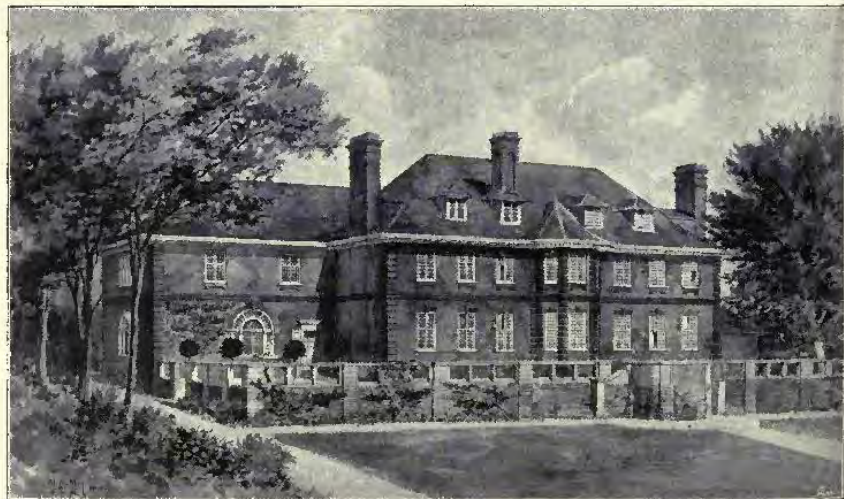
1790. Fritthwood House, Northwood , MERVYN E. MACARTNEY, Architect. (For Plans, see p. 29.)
