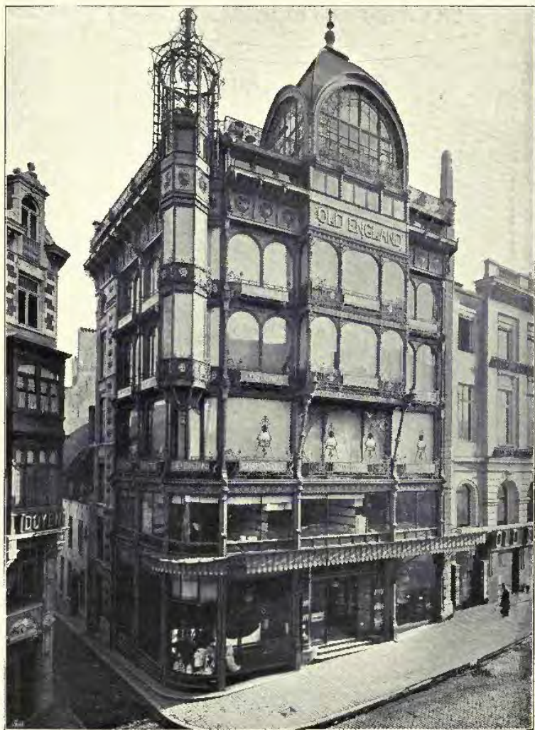
Magasin Old England, Brussels, PAUL SAINTENOIS, Architect, Brussels. (In collaboration with MM. DE BECKER, Architect, and WYLIOWSKI, Engineer.)]
