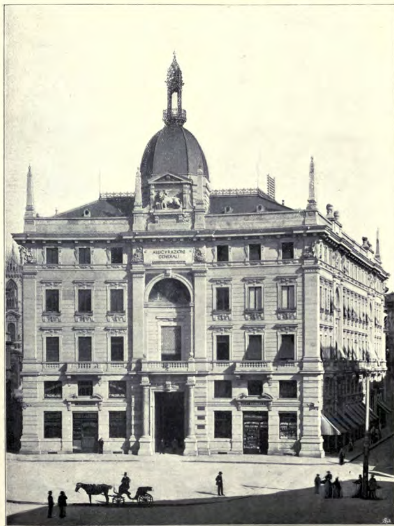
Business Premises in Milan of the Assicurazioni Generali, "Venezia," LUCA BELTRAMI, Hon. Corr. Mem. R. I. B. A., Architect, Milan.
