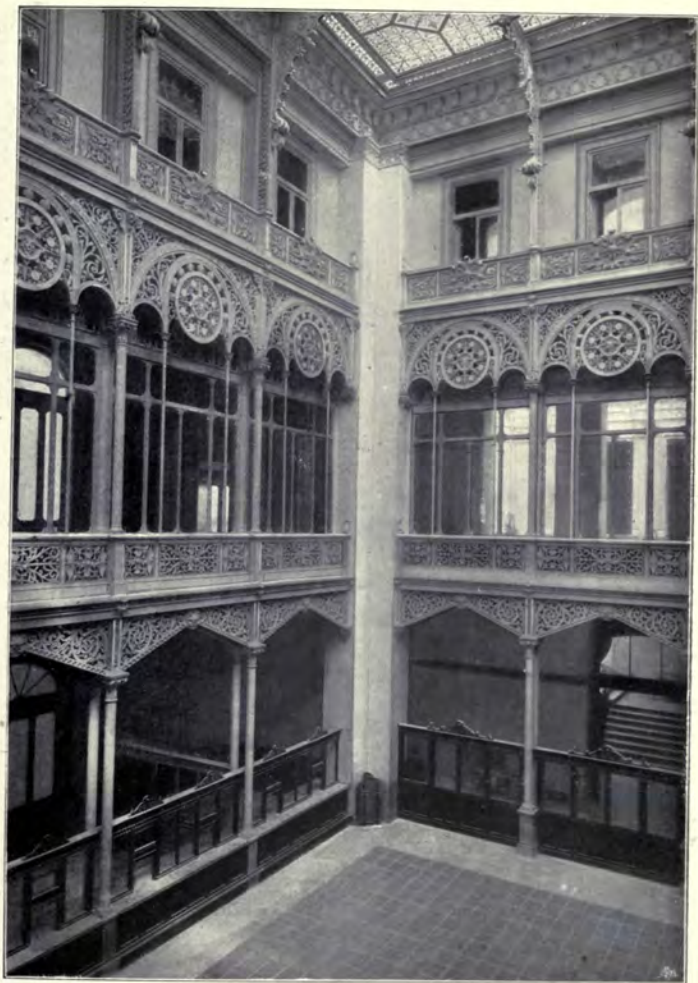
Bank of Spain, The Moorish Court, EDUARDO DE ADARO, Architect, Madrid.
