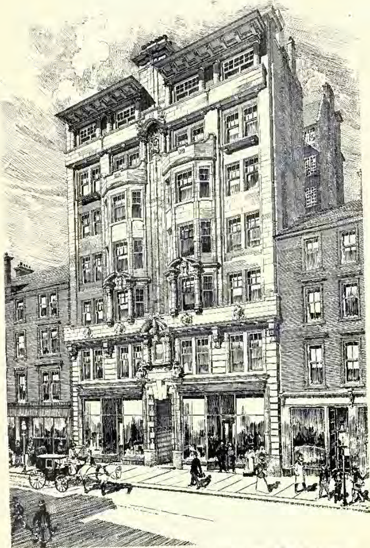
757. Atlantic Chambers, Glasgow , JOHN JAMES BURNET, A.R.S.A., Architect. (For Plans, see p. 104.)
