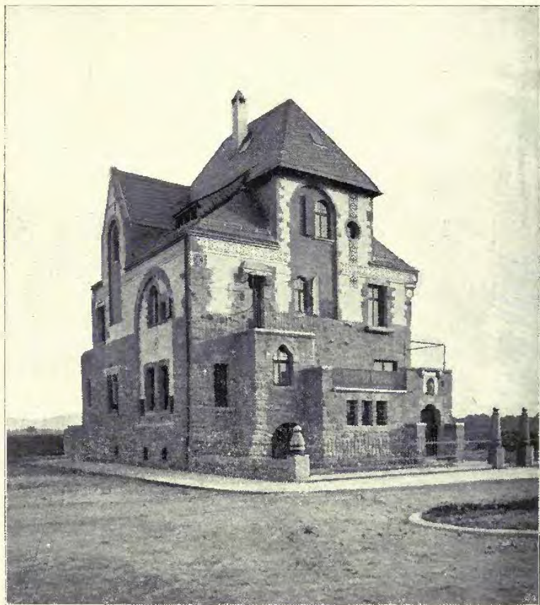
Haus Billing, Eisenlohr Strasse, Karlsruhe, HERMANN BILLING (BILLING AND MALLEPFEIN), Architect, Karlsruhe. (For Plans, see p. 123.)
