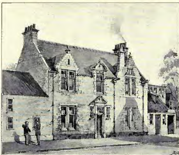
536. Offices at Dunfermline, T. HYSLOP URE, Architect. (For Plans, see p. 93.)
