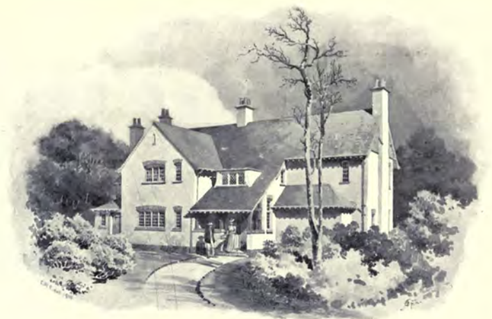
1721. A House at Warlingham, Surrey , HARRISON AND WARD, Architects. (For Plans, see p. 48.)
