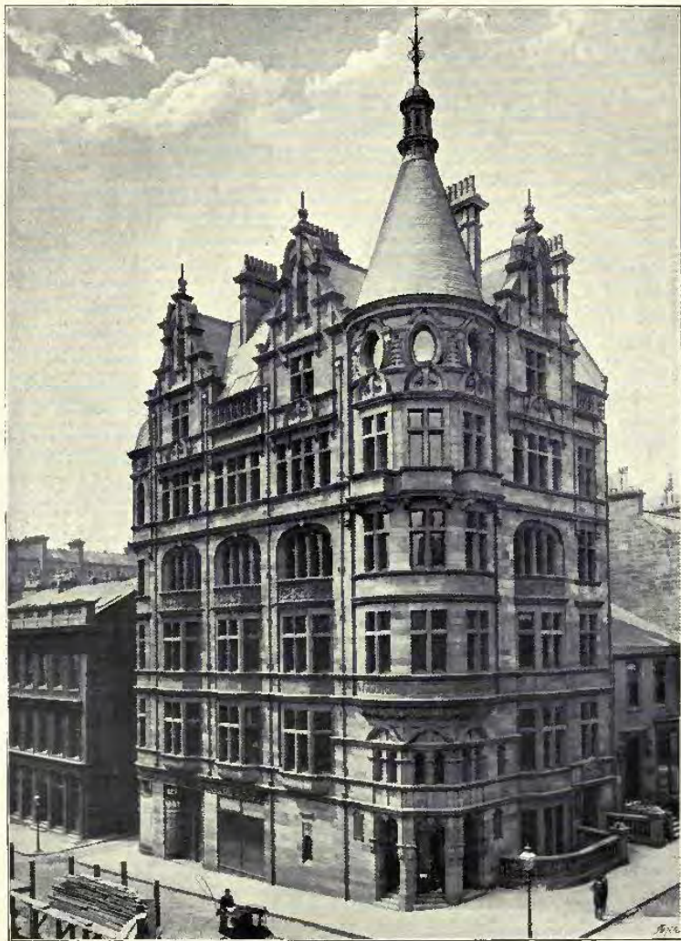
523. Norwich Union Chambers, Glasgow, JOHN HUTCHISON, F.R.I.B.A., Architect.
