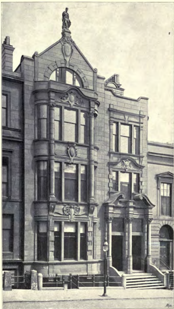
703. Business Premises, St. Vincent Street, Glasgow, FRANK BURNET AND BOSTON, Architects.
