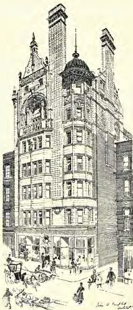
700. The British Workman's and General Assurance Company's Premises, 166, Buchanan Street, Glasgow, JOHN A. CAMPBELL, Architect.
