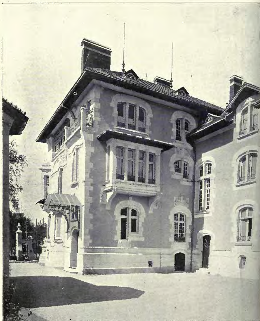
Villa Schiltzenberger, Strassburg i/E, BERNINGER AND KRAFFT, Architects, Strassburg. (For Plans, see p. 134.)
