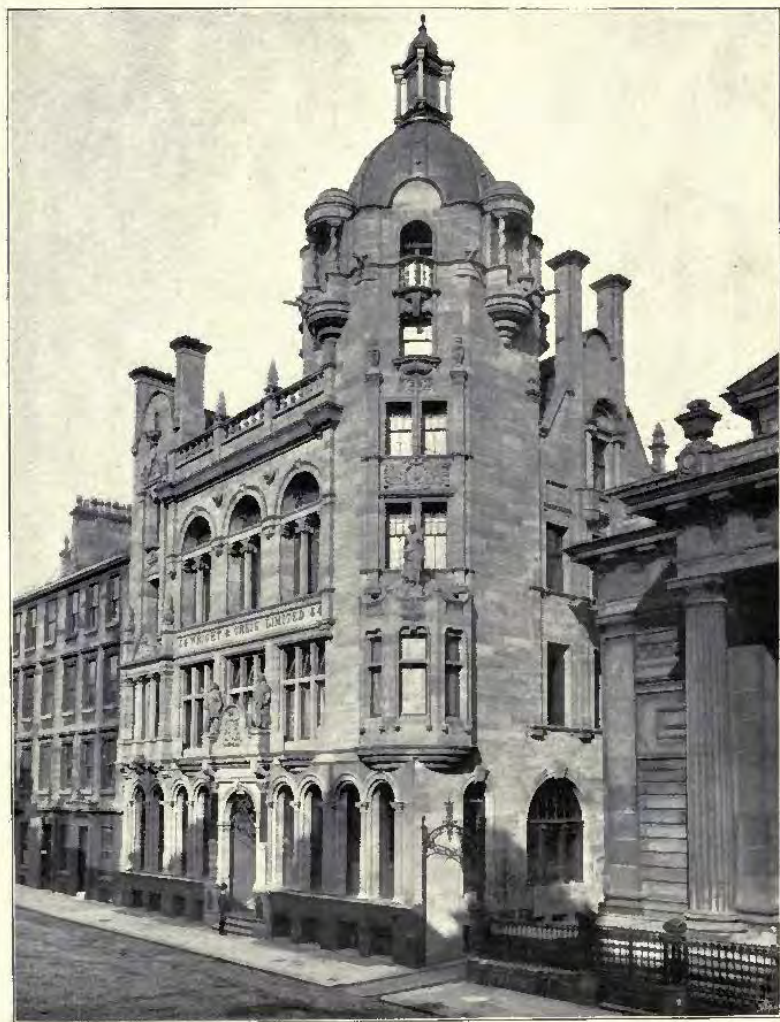
531. Business Premises for Messrs. Wright and Greig, Ltd., JAMES CHALMERS, I.A., Architect.
