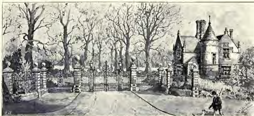
Lodge and Entrance Gates, Childwick Bury, St. Albans, ROBERT W. EDIS, F.S.A., Architect.
