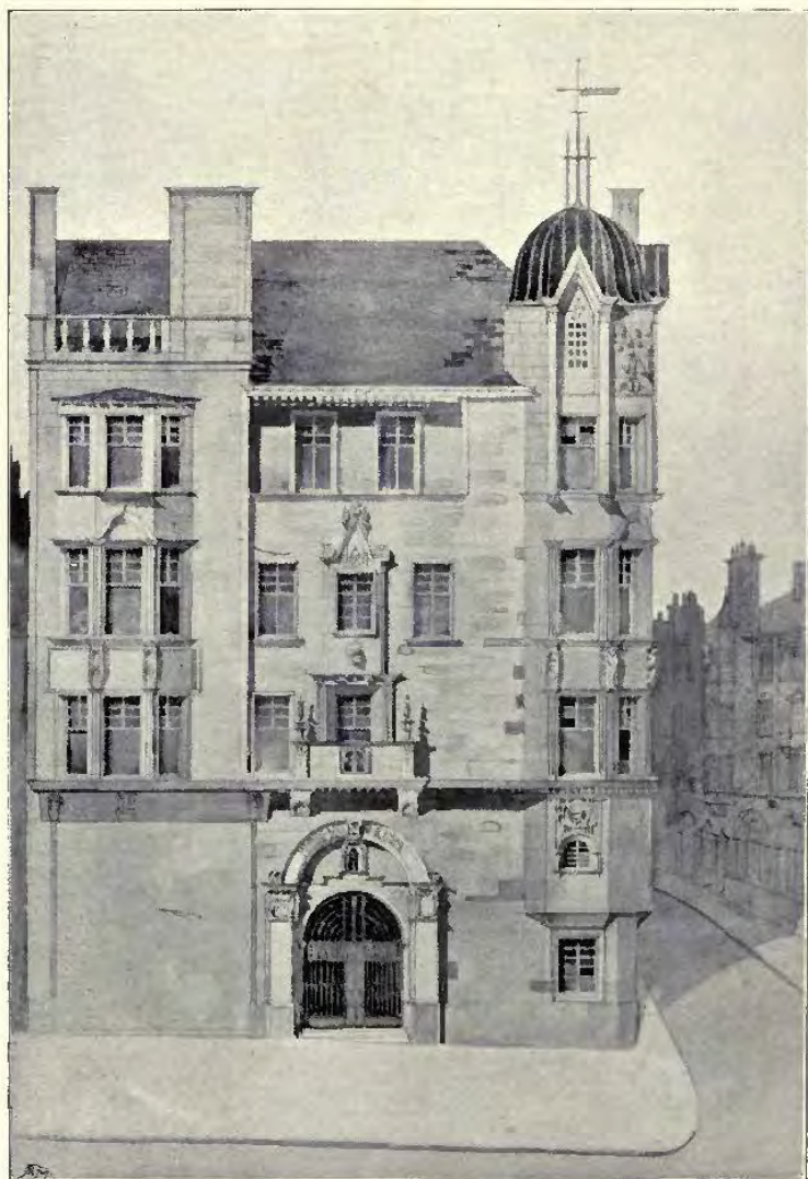
511. Savings Bank, Anderston, Glasgow, JAMES SALMON AND SON, Architects.
