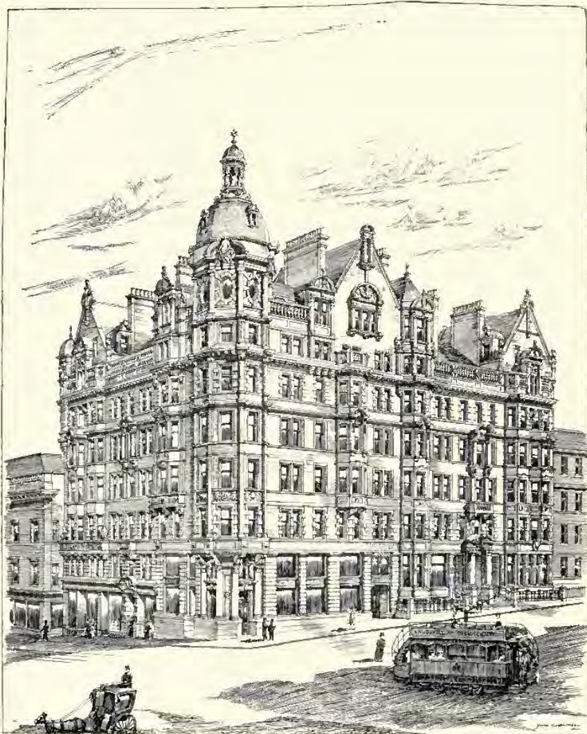
566. Business Premises, Renfield Street and West Regent Street, Glasgow, FRANK BURNET AND BOSTON, Architects.
