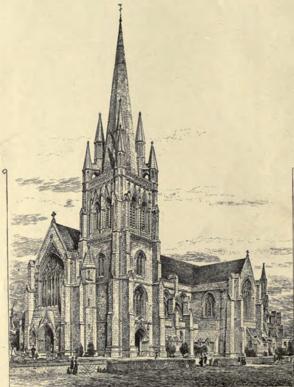
St. Alban's Church, Blackburn, EDWARD GOLDIE, Architect.
