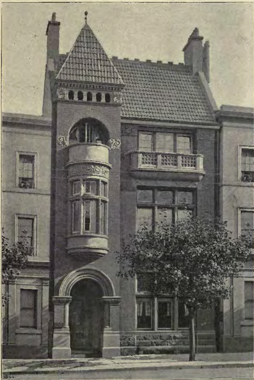
Doctor's Residence, Collins Street, Melbourne, NAHUM BARNET, Architect, Melbourne.
