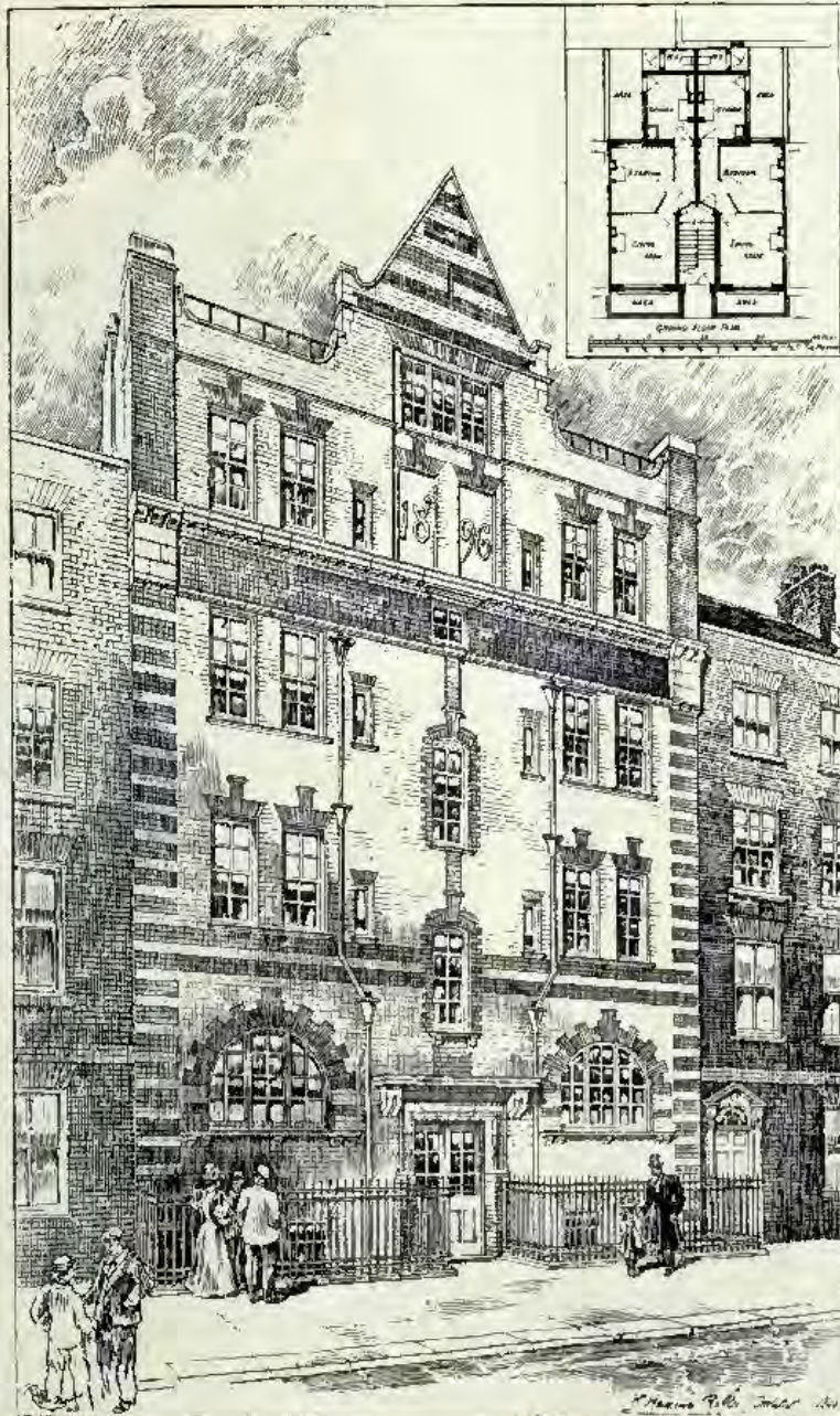
Nos. 9 & 10, Gosfield Street, London, W., W. HARGREAVES RAFFLES, Architect. (For Plan, see p. 66.)
