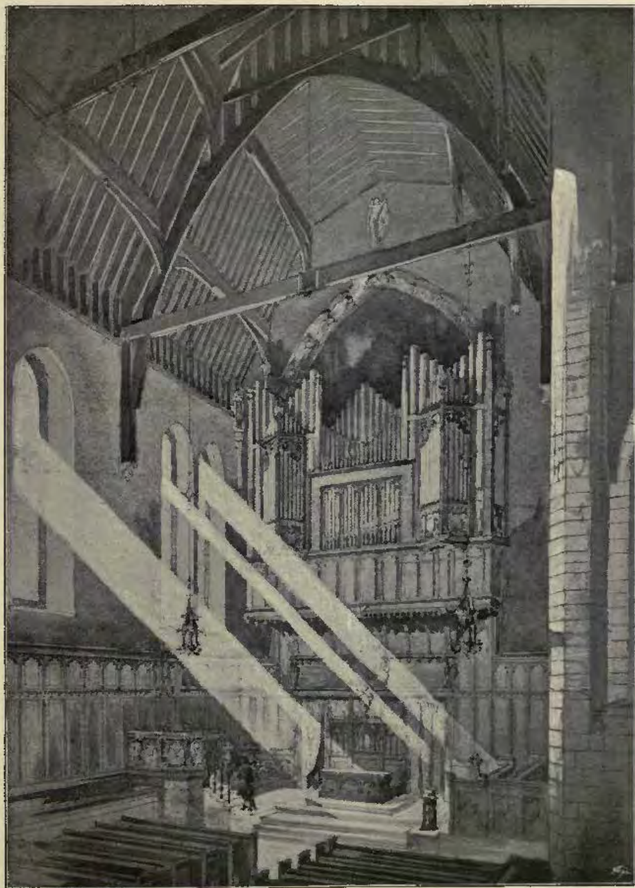
283. Parish Church, Arbroath, Chancel , JOHN JAMES BURNET, A.R.S.A., Architect. (For Exterior View, see Vol. VII., p. 57.)
