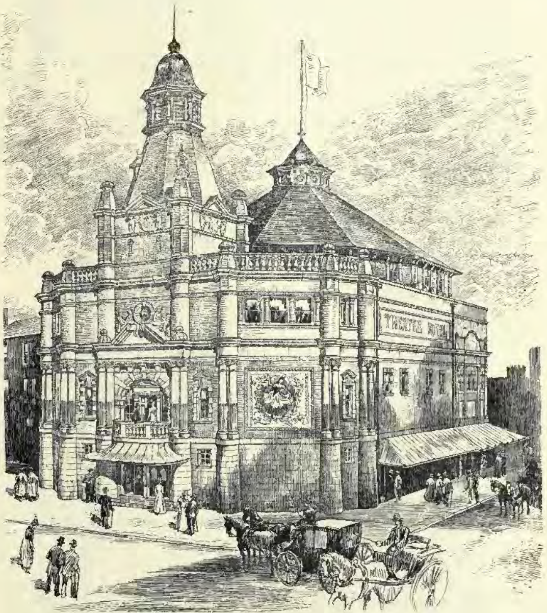
Theatre Royal, Southampton , W. HOPE AND J. C. MAXWELL, Architects. (For Plan, see p. 102.)
