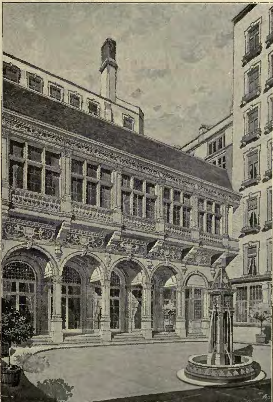
1850. Additions to the Savoy Hotel , T. E. COLICUTT, F.R.I.B.A., Architect.
