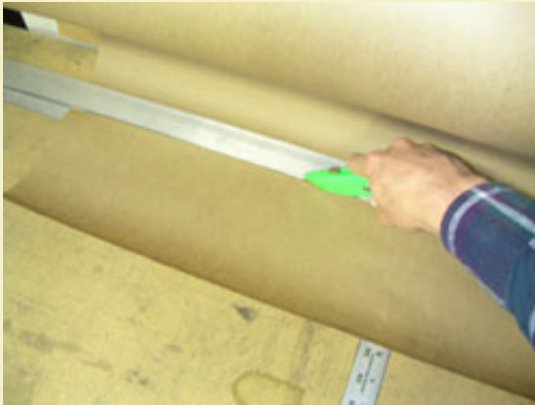
Figure 5: Cutting from a roll using a utility knife.
