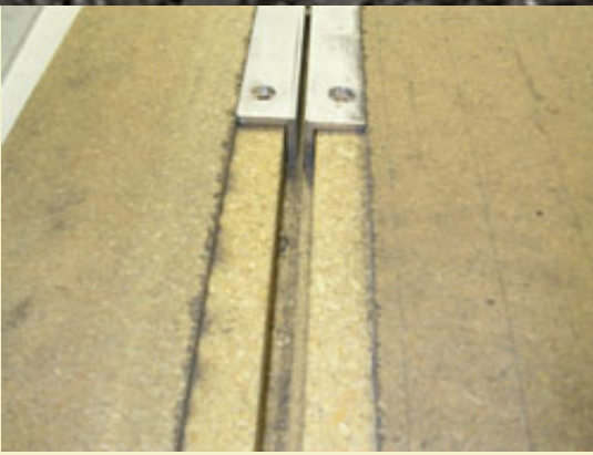
Figure 7: Closeup of angle aluminum fitted into cutting channel.
