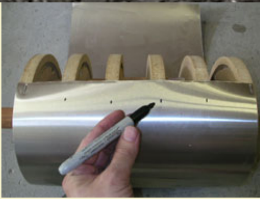
Figure 6: Marking the rib positions.
