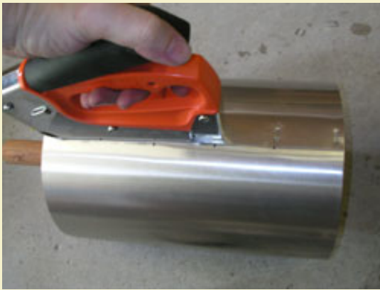
Figure 7: Securing the seam by stapling to the frame ribs.
