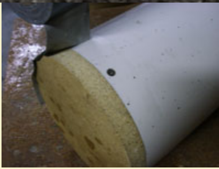
Figure 15: Attaching bottom with screws and sealing with duct tape.
