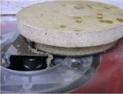
Figure 11: Using a router with a laminate bit to trim the excess overhang.
