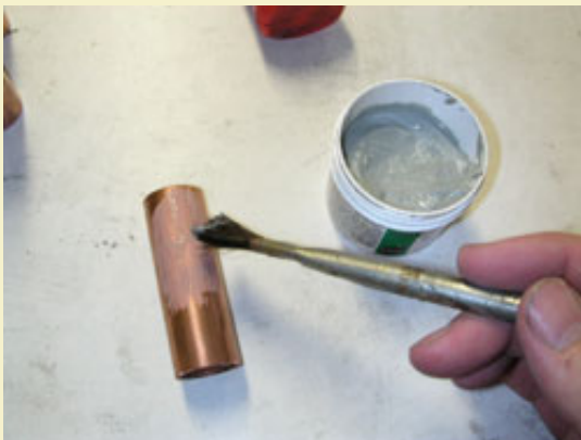
Figure 1: Brushing flux onto a pipe segment before soldering.
