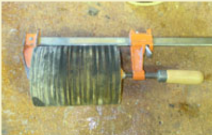
Figure 2: Laminating plywood disks to form the rammer.
