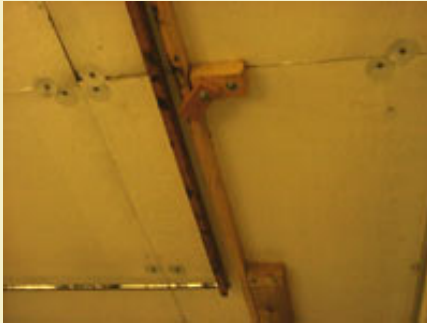
Figure 5: Clamps holding frame against the ceiling.
