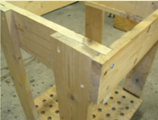
Figure 5: Joining details of the container frame.
