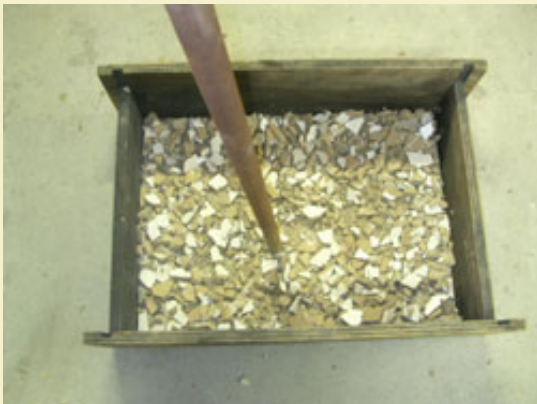
Figure 7: Grinding up floor tiles with a steel rod in a box to reduce flying shards.
