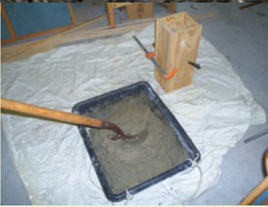
Figure 5: Mixing 40 lbs of cement in a plastic tub using a shovel.
