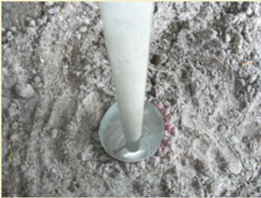
Figure 20: The nail end of the ramming rod is placed into the buried soda can, which is then filled to the top with lead.
