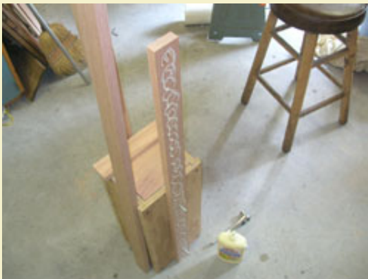
Figure 9: Using wood glue to laminate the 36" and 54" long frame members together.
