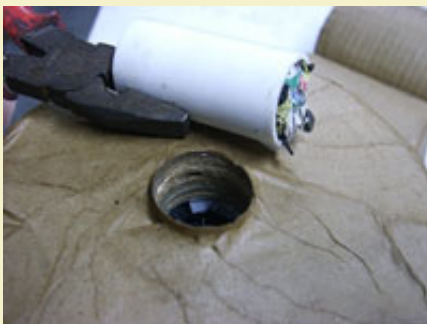
Figure 34 Removing the PVC plugs.
