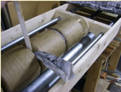
Figure 37: Ramming pasted newspaper between the breaks.
