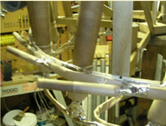
Figure 34: Side mounted lances are tied off and foiled over to protect the connection points.
