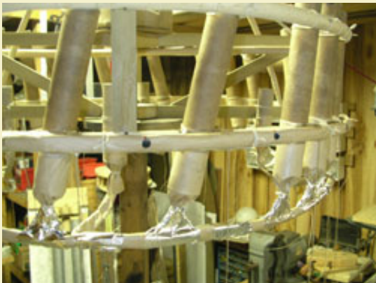
Figure 32: A ring of matched pipe is tied to the lower ring. Note the holes pre-punched where the lance fuses will connect.
